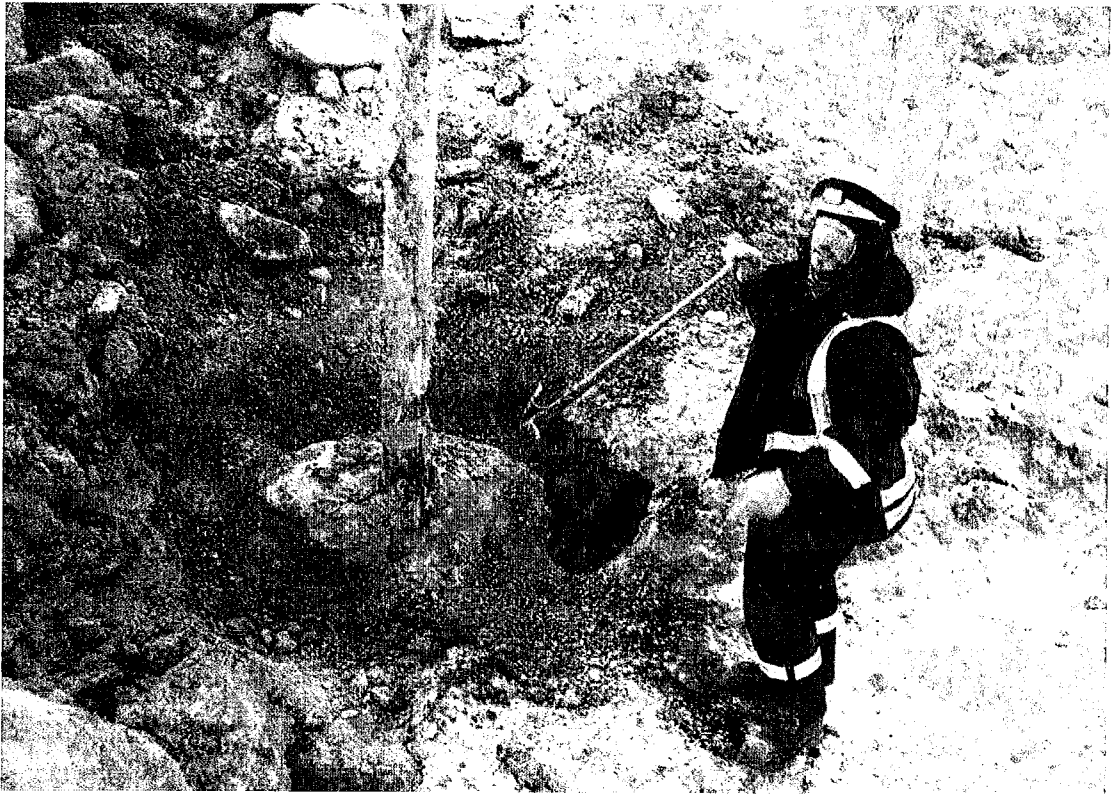
Photo 3 – Grout bulb with excavated ungrouted 'crush' fill adjacent
