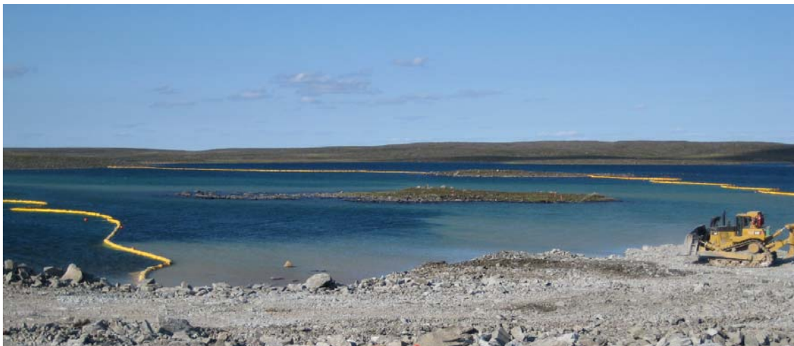
Photo 2-3. Elevated TSS appears to be contained by turbidity barriers - July 31.
