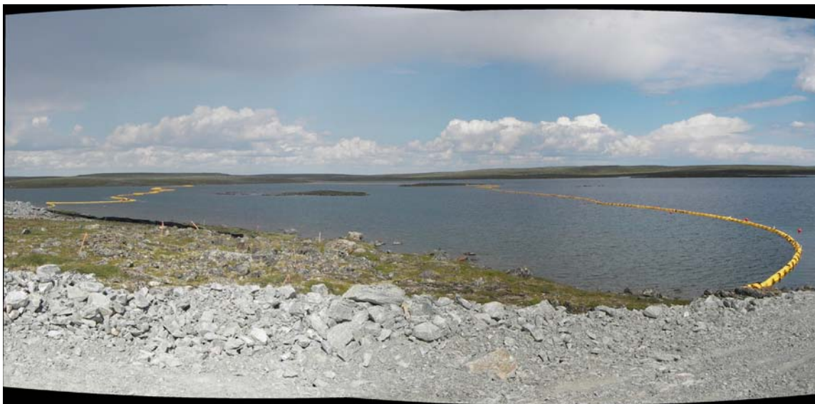
Figure 10: Turbidity Barriers at Second Portage Lake (July 24, 2008)
