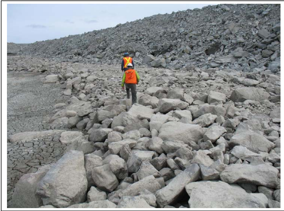
Photo # 7 East Dike, boulder field along downstream toe of dike
