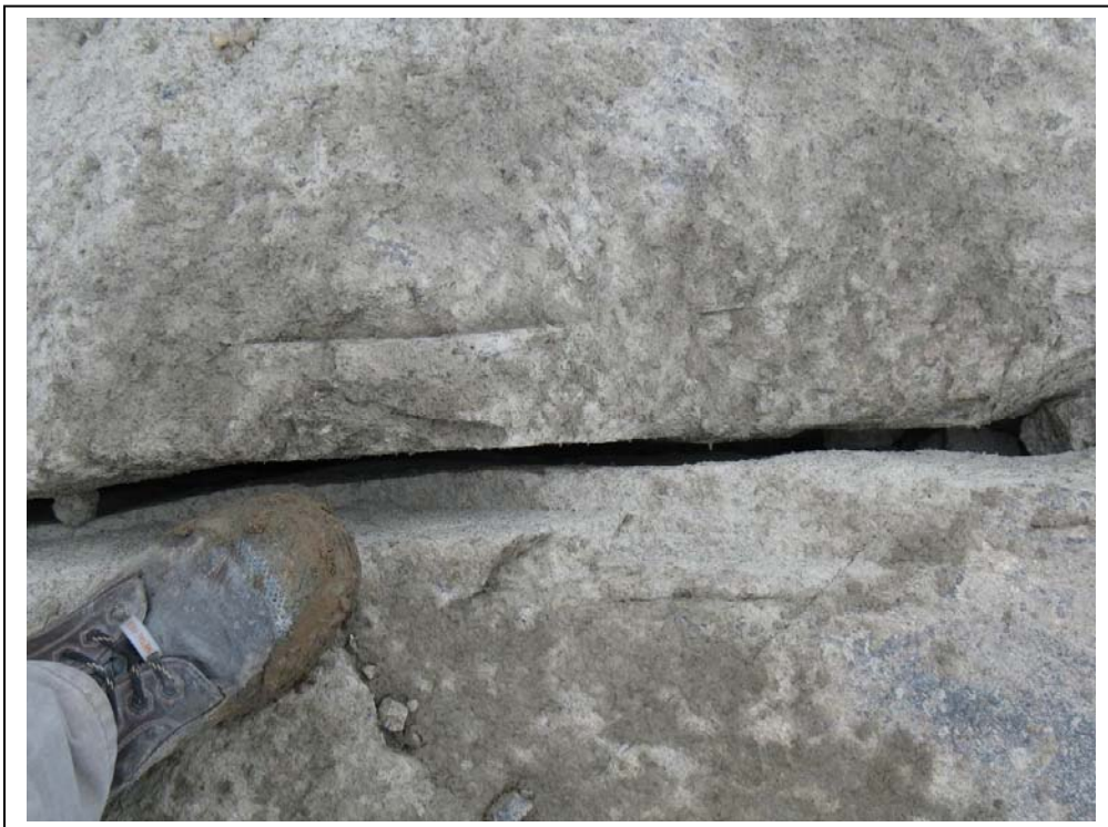
Photo # 12 Stormwater Dike, open joint in rock foundation
