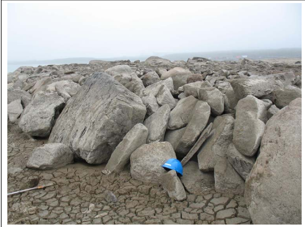
Photo # 13 Stormwater Dike, boulder accumulation along shoreline
