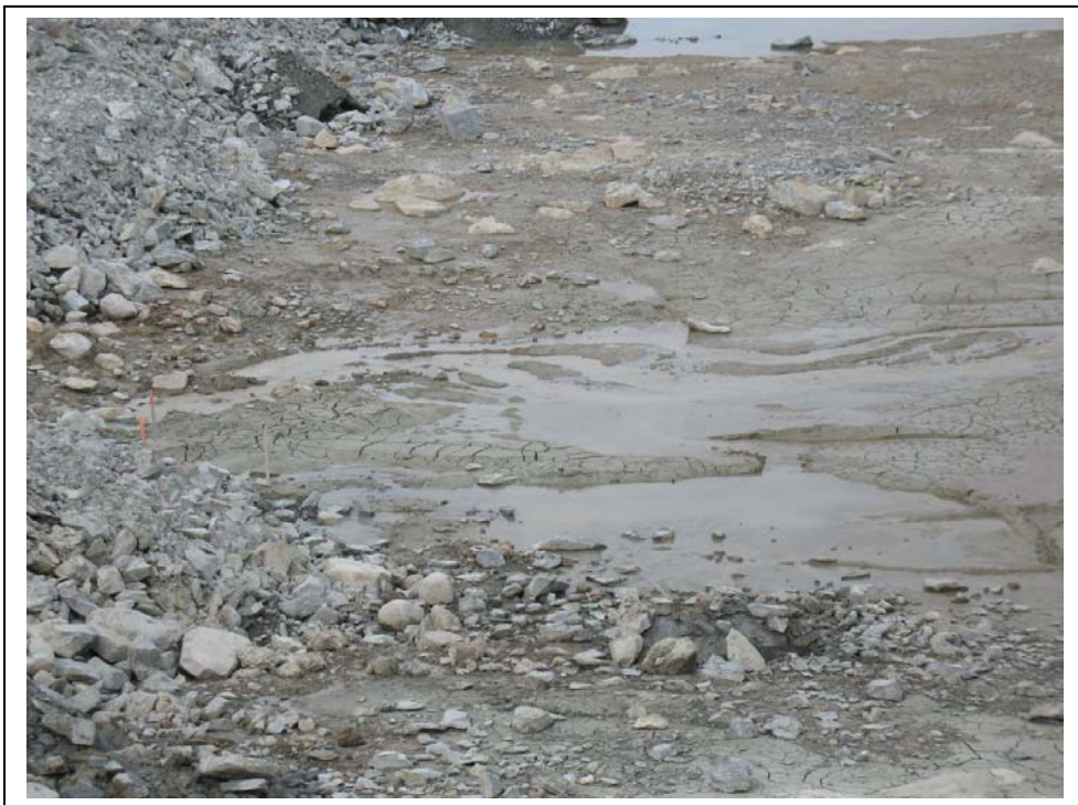
Photo # 4 East Dike, seepage to east of ramp
