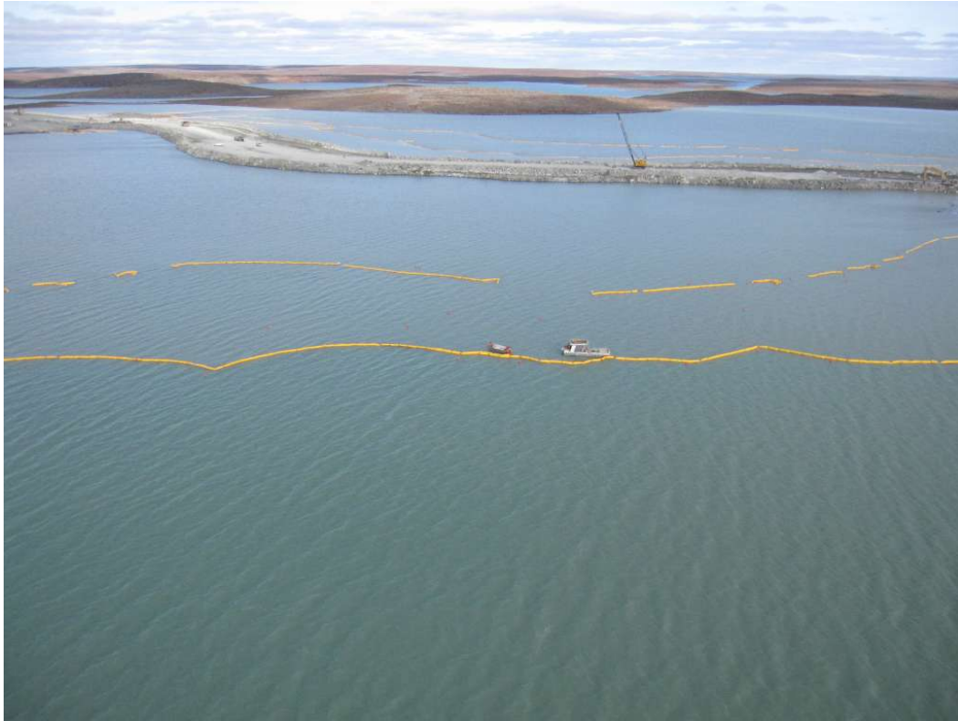
Reparation of the turbidity curtain Sept 11 2009
