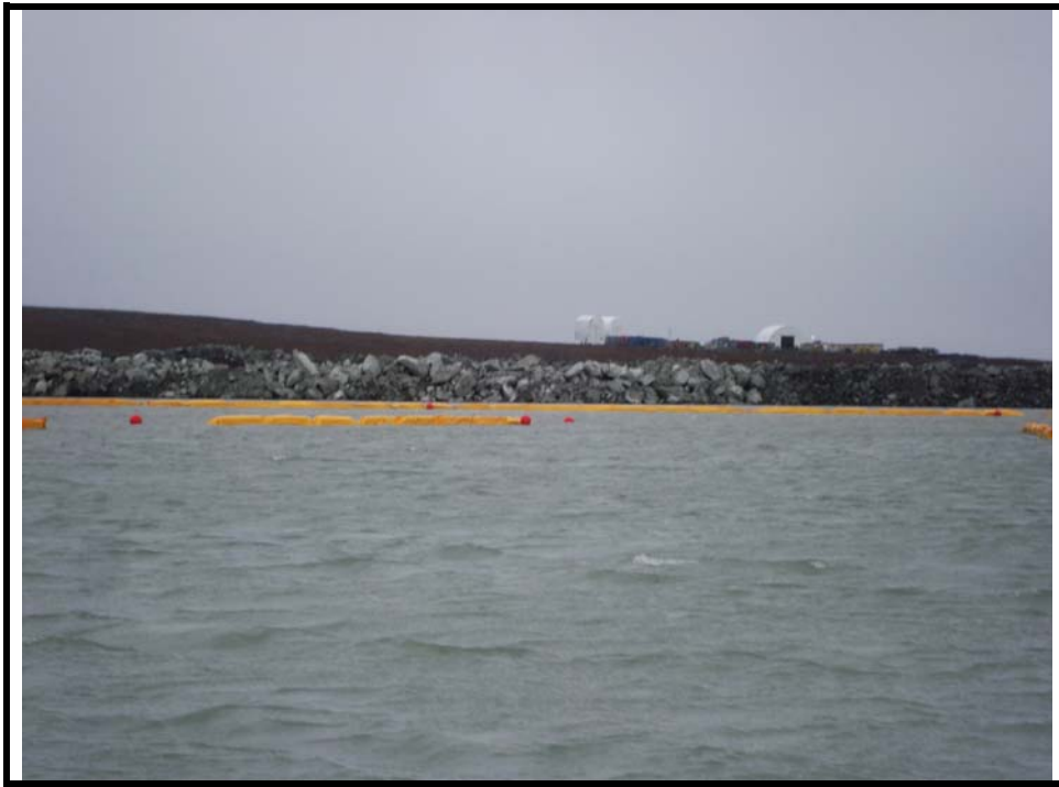
Photo 4 : Turbidity curtain East side.
