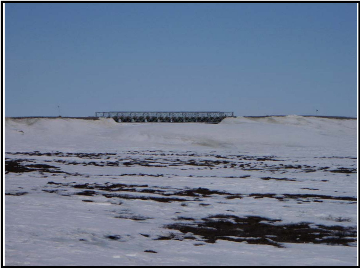
Photo No 2: R02 prefreshet erosion inspection. No erosional issues identified.
