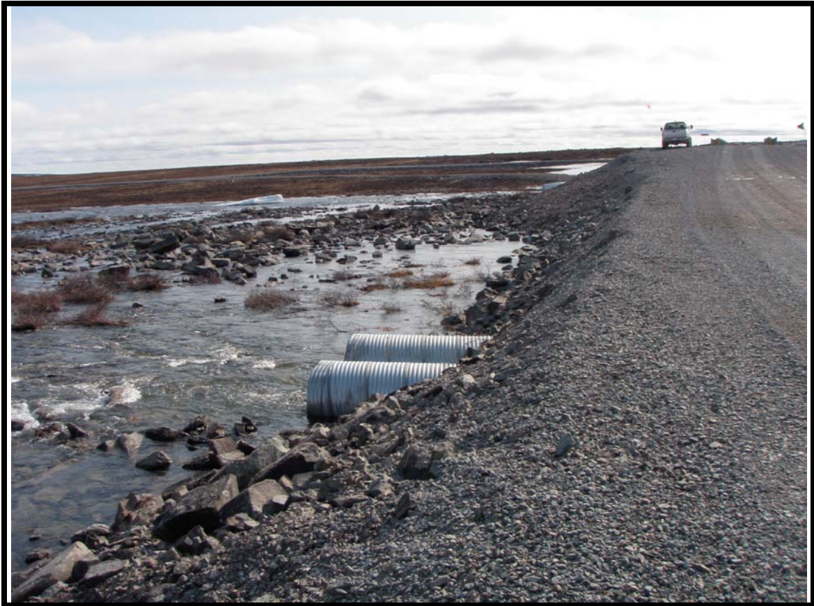
Photo No 6 : Downstream photo of R02 culverts
