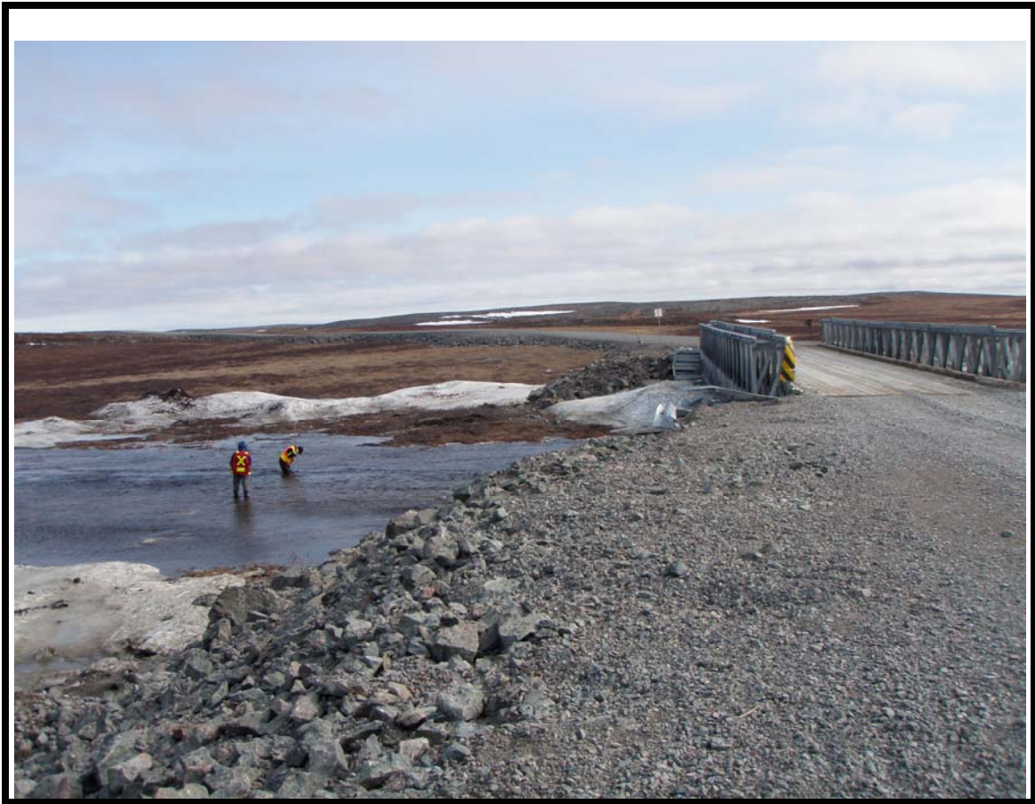
Photo No 5 : Turbidity and erosion monitoring at R05
