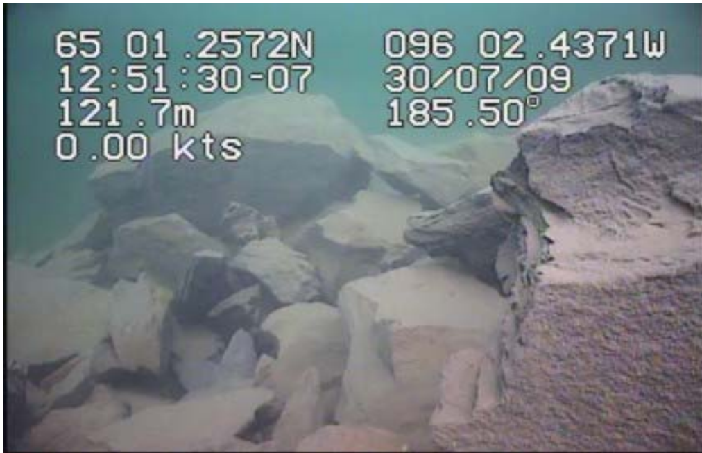
Photo C-1. (East Dike- midpoint) East Dike construction material primarily made of large jagged boulders.
