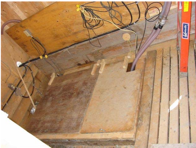
10. Inside of the Grease Station with panel over the trap.
