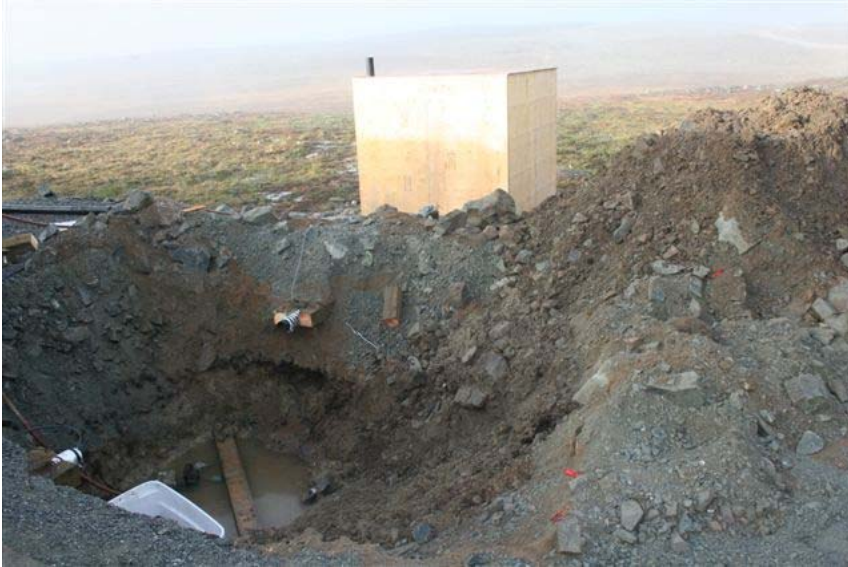
1. Construction of the new grease trap.
