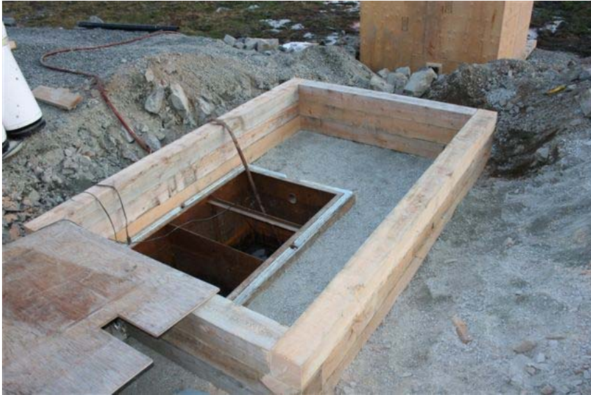
7. The base filled with 0-3/4''.
