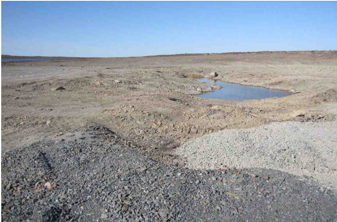
Photo 04: After completion of the haulage the area have been levelled with the loader. The banks (non-contaminated material) were pushed to make sure there are no steep slopes – September 4 th 2009.
