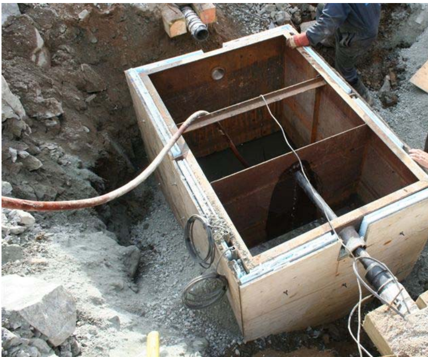
4. excavation and installation of the grease trap
