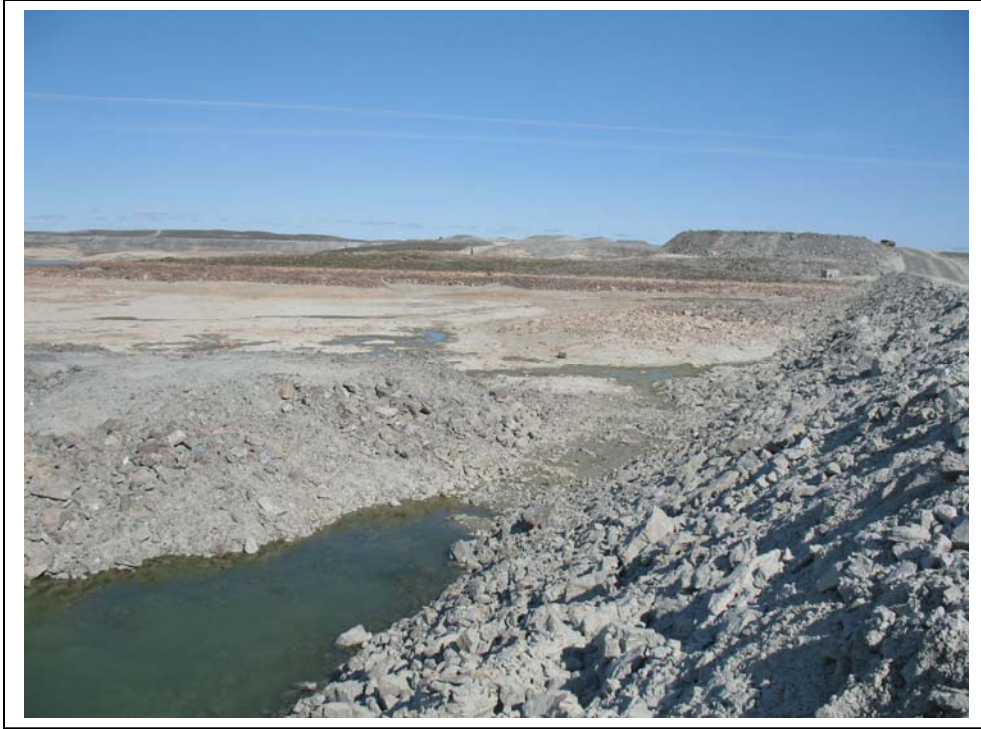
Photo # 1 East dike, seepage areas in North Channel
