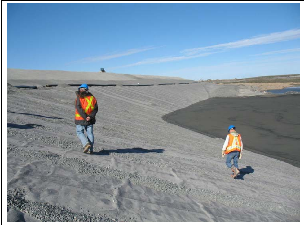
Photo # 11 Stormwater dike, Coletanche liner minor wrinkles
