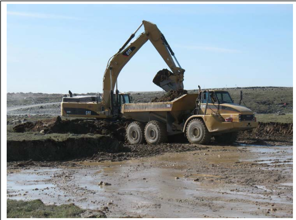
Photo # 18 Saddle dam SD2, excavation of ice rich soils
