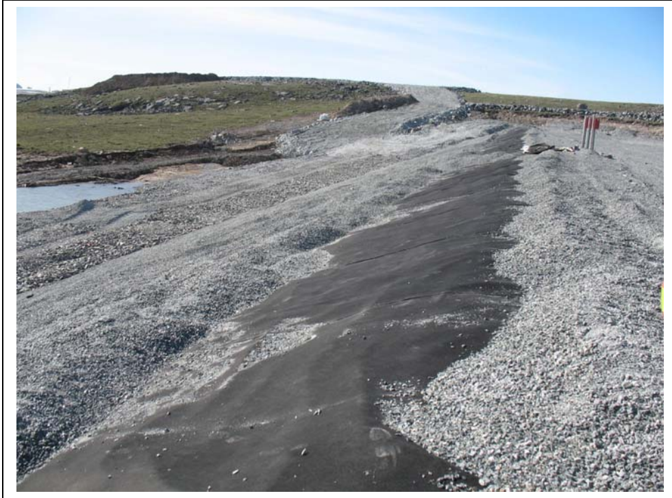
Photo # 15 Saddle dam SD1, LLDPE liner with geotextile cover
