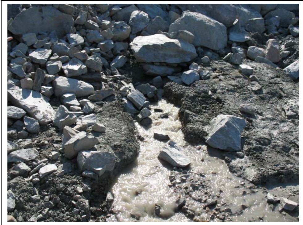
Photo # 5 East dike, flow from toe of dike in South Channel
