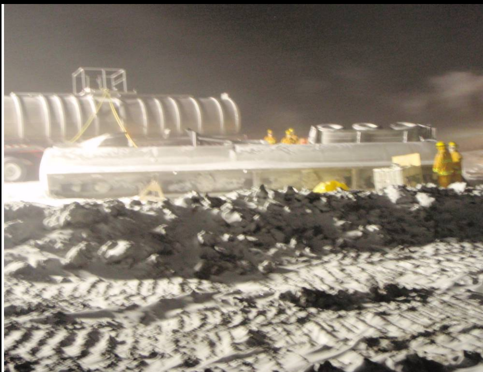
Photo No 4 : ERT organizing pumps to transfer to another tanker; berm in foreground constructed of local muck and lined with \frac{3}{4} inch gravel on the inside
