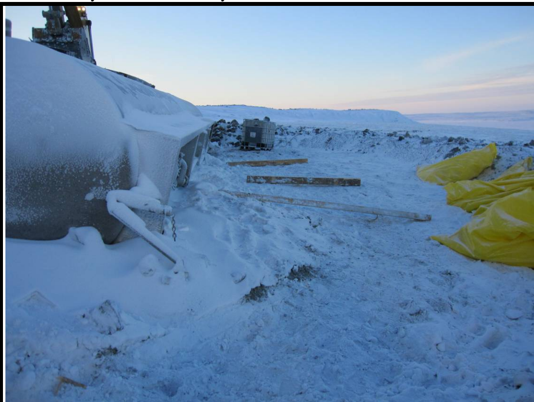
Photo No 8: Secondary containment berm and HDPE hazardous spill bags
