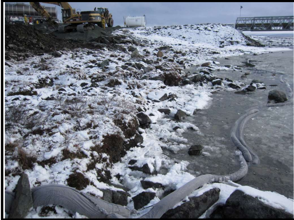
Photo No 4 : Booms installed in the river to prevent the river contamination.
