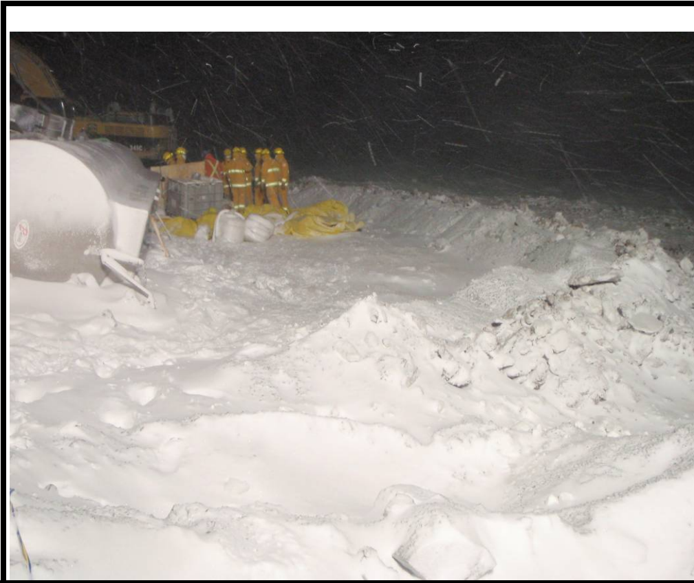
Photo No 3 : Secondary berm constructed with the large excavators
