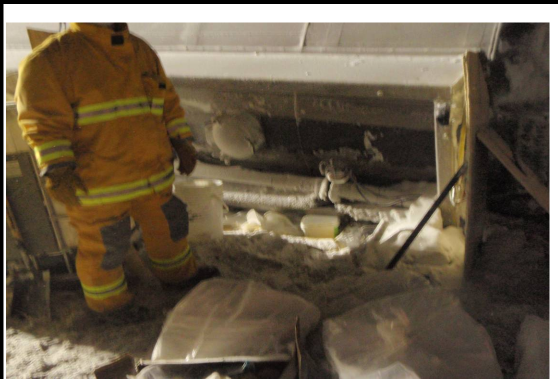
Photo No 5 : Yellow insta-berm, absorbent pads and buckets used to contain and recover leaking release valve. No other apparent spills.
