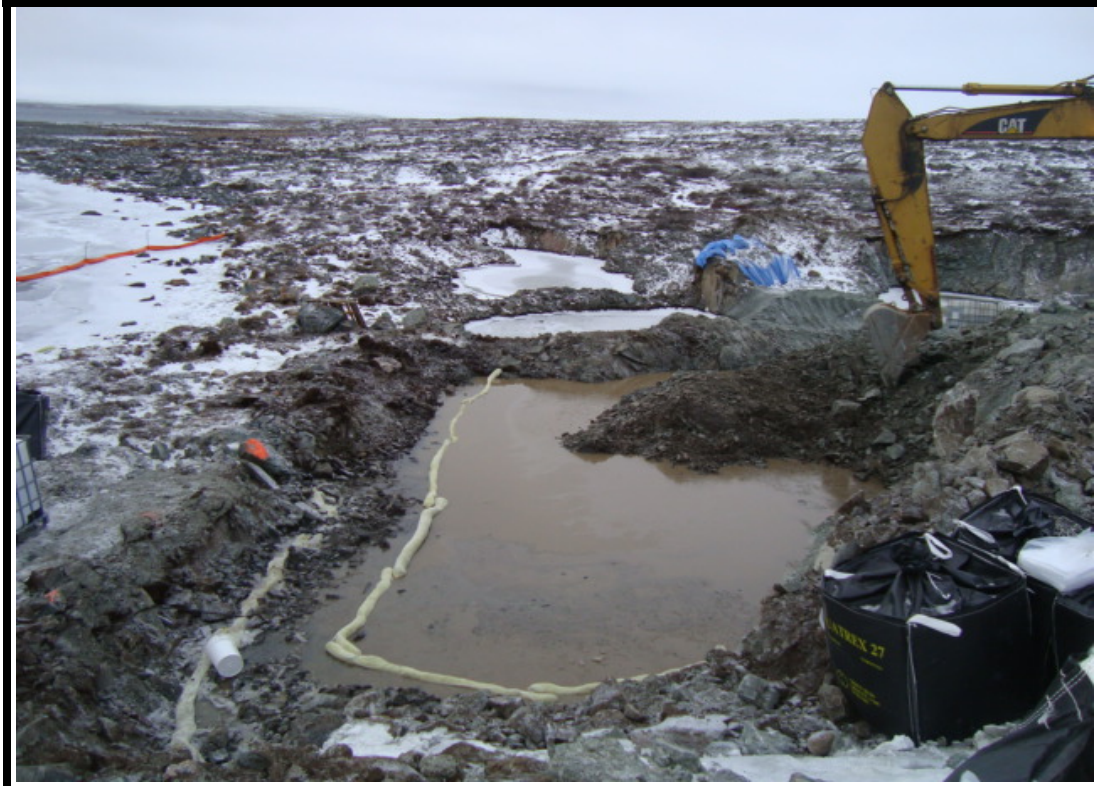
Photo No 10 : Excavation between the abutment of the bridge and the first ditch.
