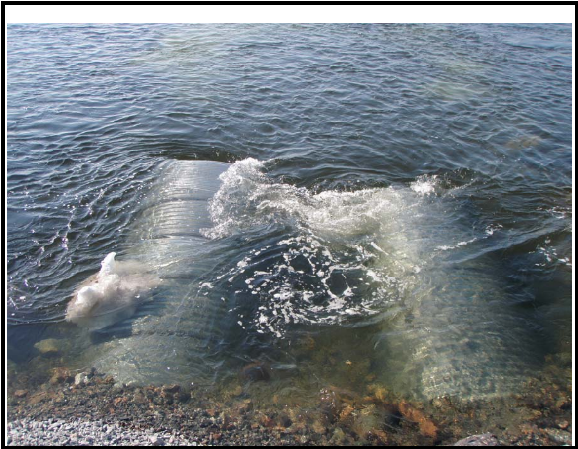
Photo No 5 : R02 water level at permanent culverts (June 15,2010)
