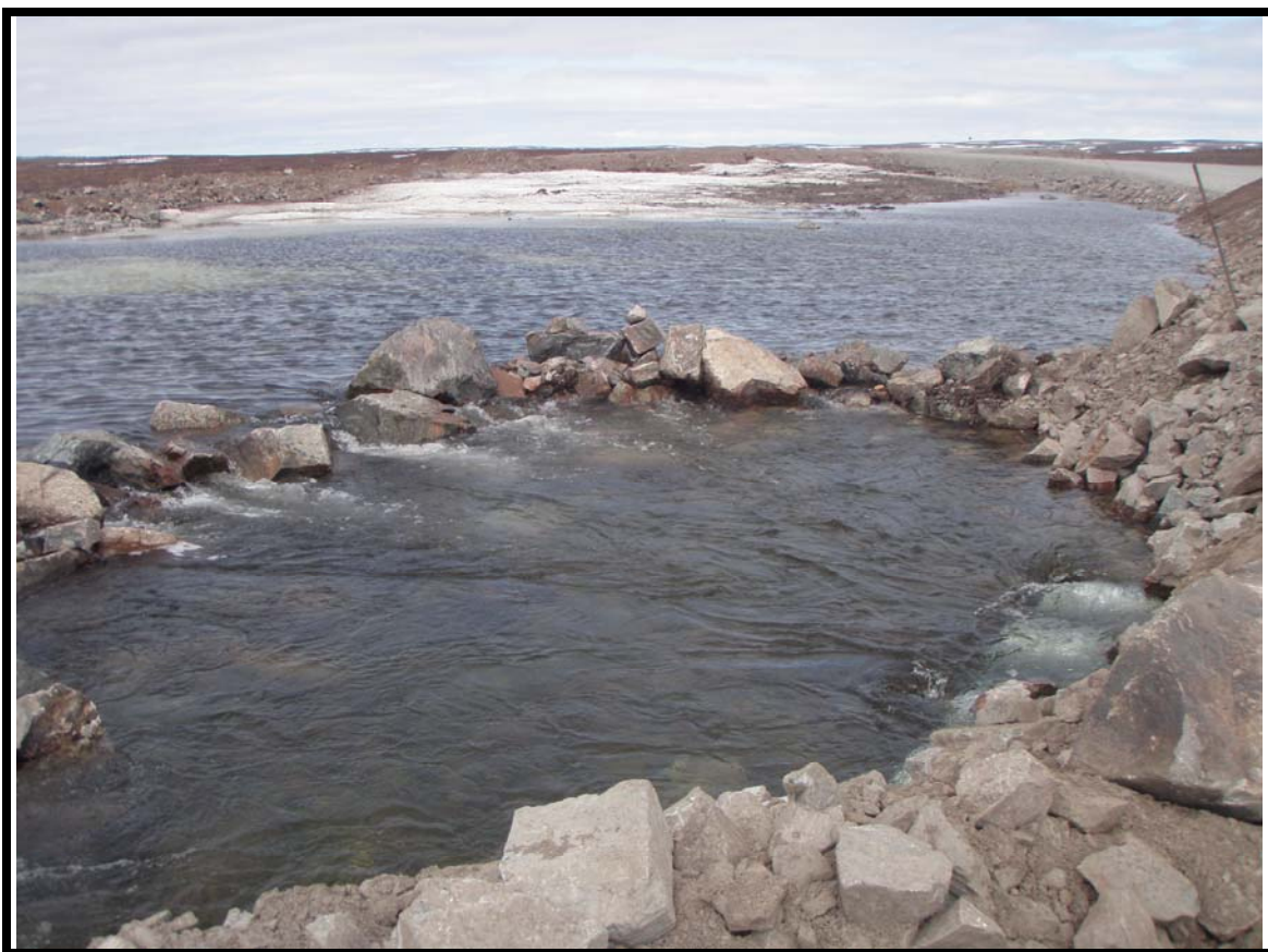
Photo No 8 : R02 temporary culverts with upstream clean boulder berm to reduce flows on temporary culverts (June 16, 2010).
