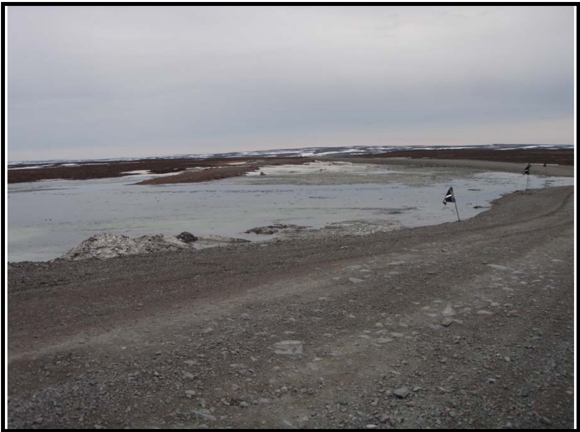
Photo No 2 : Upstream of R02- water level increasing and advancing over the road potentially causing a road washout. No observed turbidity downstream. (June 14, 2010)
