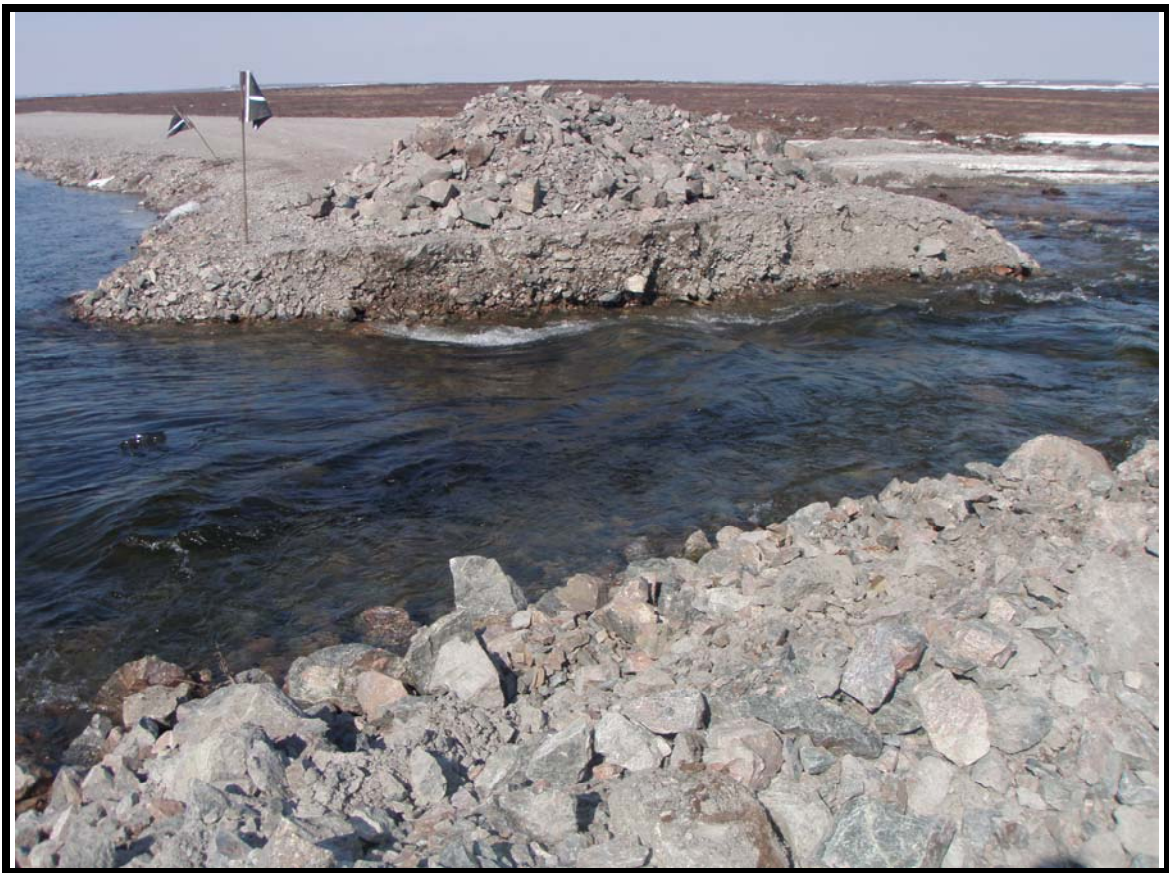
Photo No 4: R02 emergency excavation completed above the high water mark to prevent the road from washing out (June 15, 2010).
