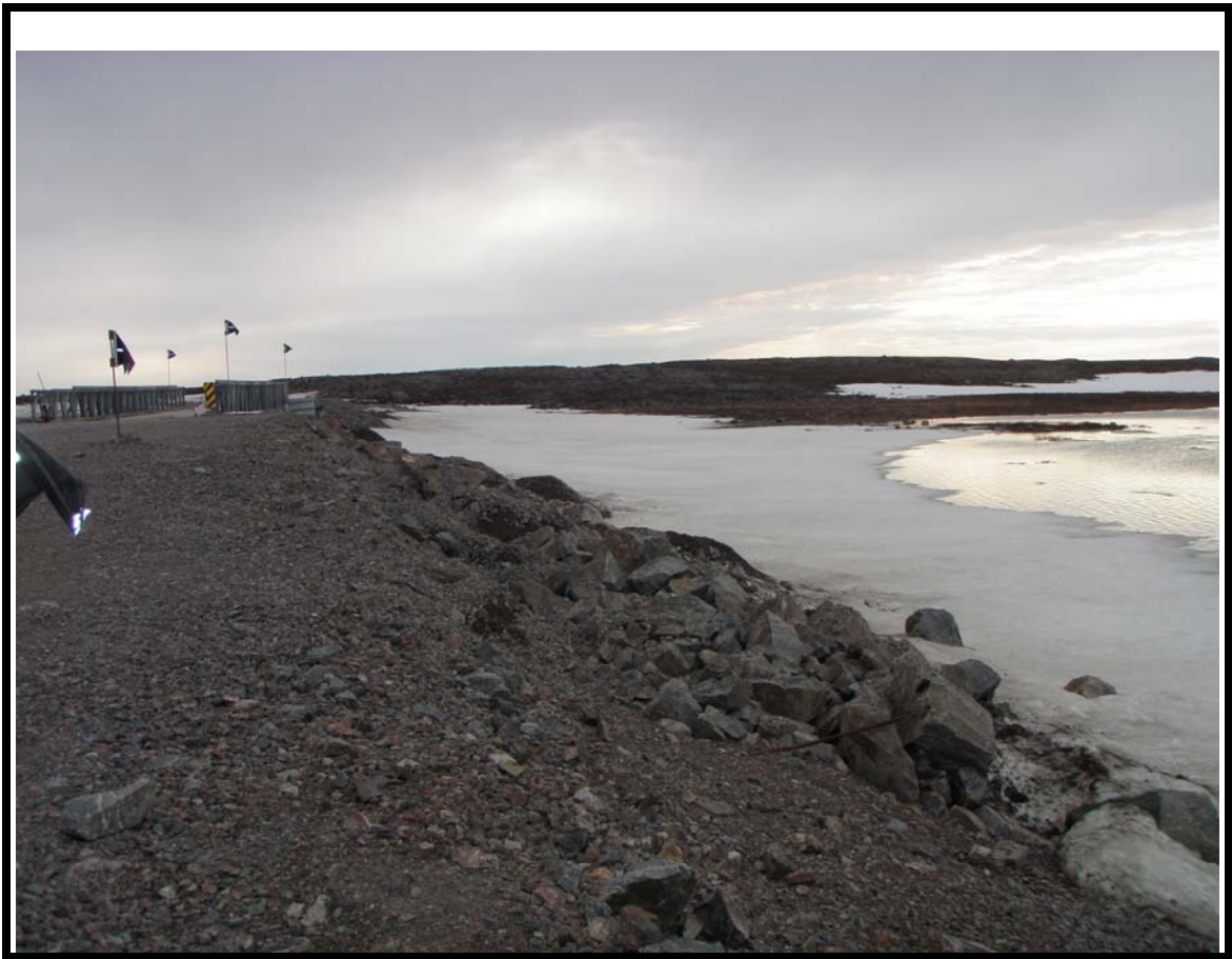
Photo No 1 : Upstream of R02- ice and snow blocking the bridge (June 14, 2010)
