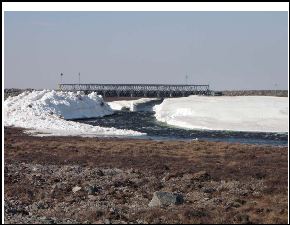
Photo No 3: R02 downstream following excavation of accumulated snow and ice below the bridge (June 15, 2010)
