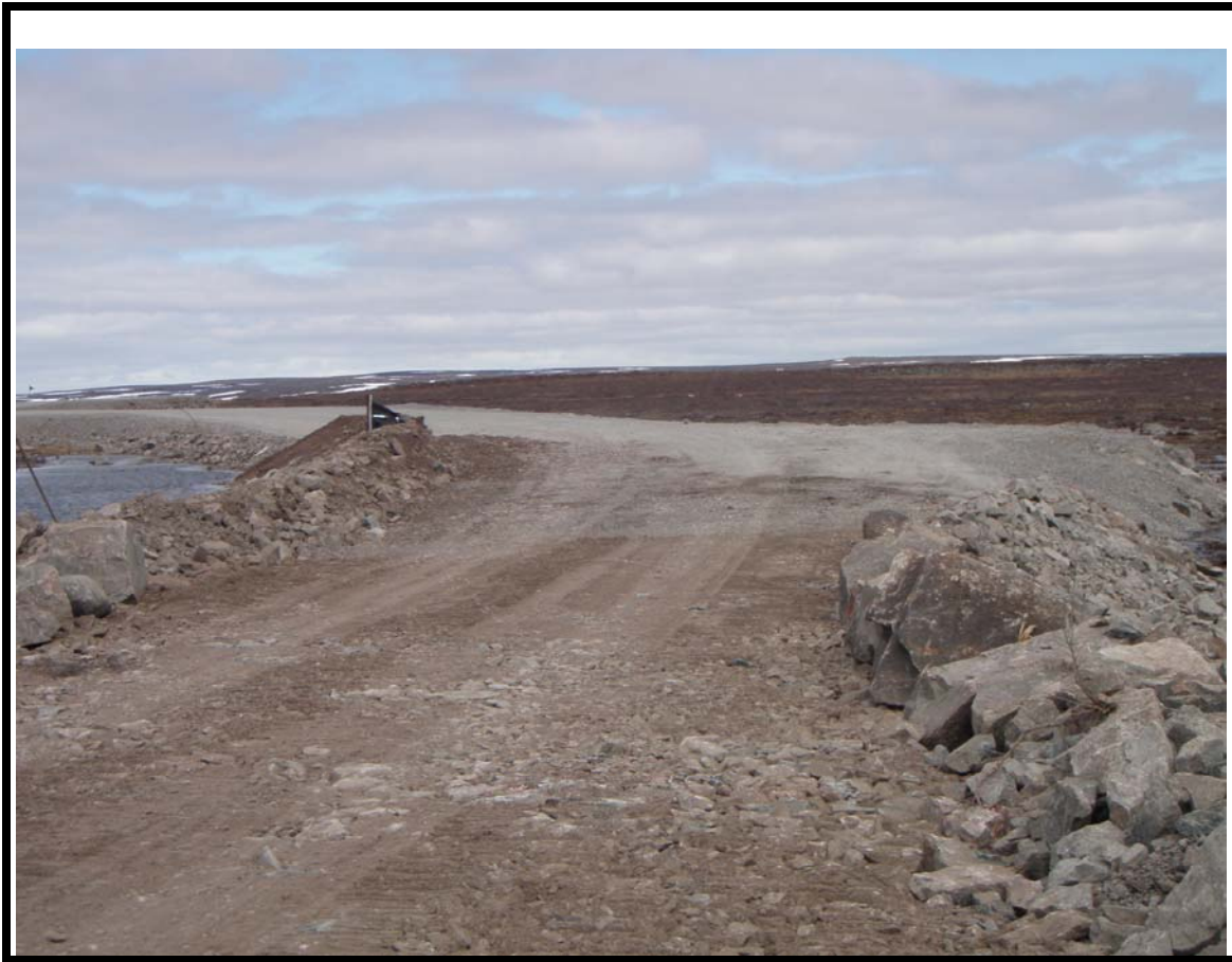
Photo No 7 : R02 temporary culverts installed on June 16, 2010 above the ordinary high water mark to accomodate freshet water flows.
