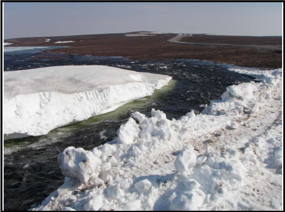
Photo No 6: Water flowing below the bridge following excavation of snow accumulated under the bridge (June 15, 2010).
