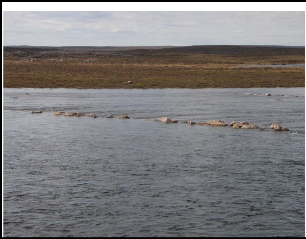
Photo No 9 : R02 berms post freshet- water level maintained from late June until mid July. Note water cascading over most of the berm
