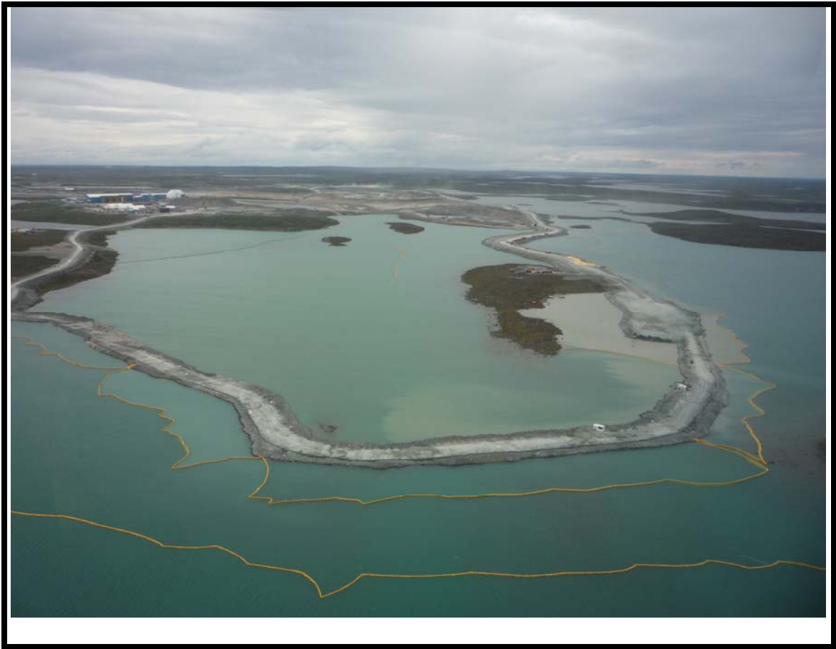
Photo No 3: July 21st - 2 layers of turbidity curtains; one anchored by the causeway, the other deployed in shallower areas
