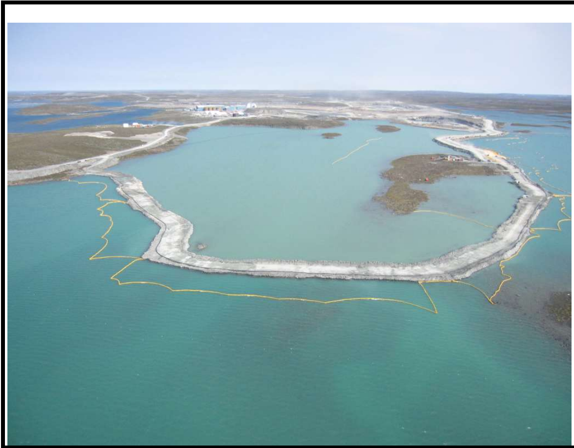
Photo No 1 : July 17th aerial photo of Bay-Goose Dike construction
