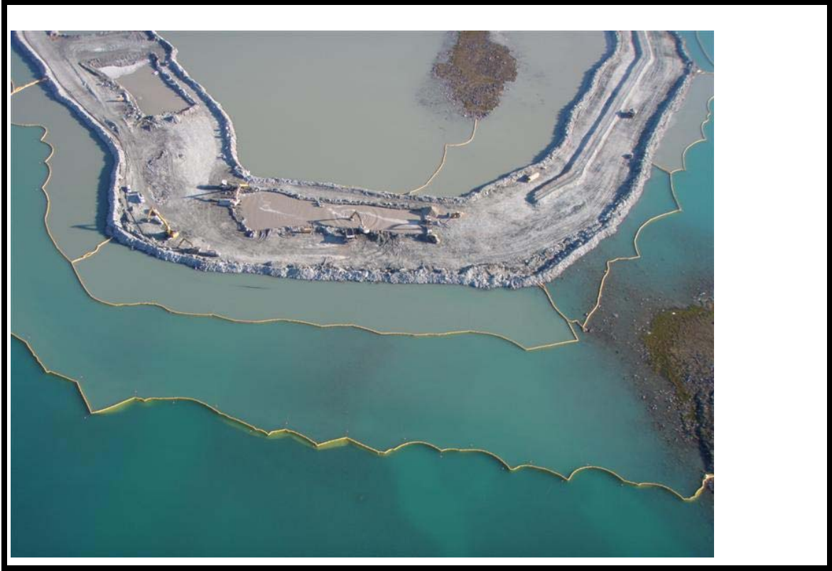
Photo No 9 : August 9th Trenching in the deepest zone of Bay-Goose Dike phase II
