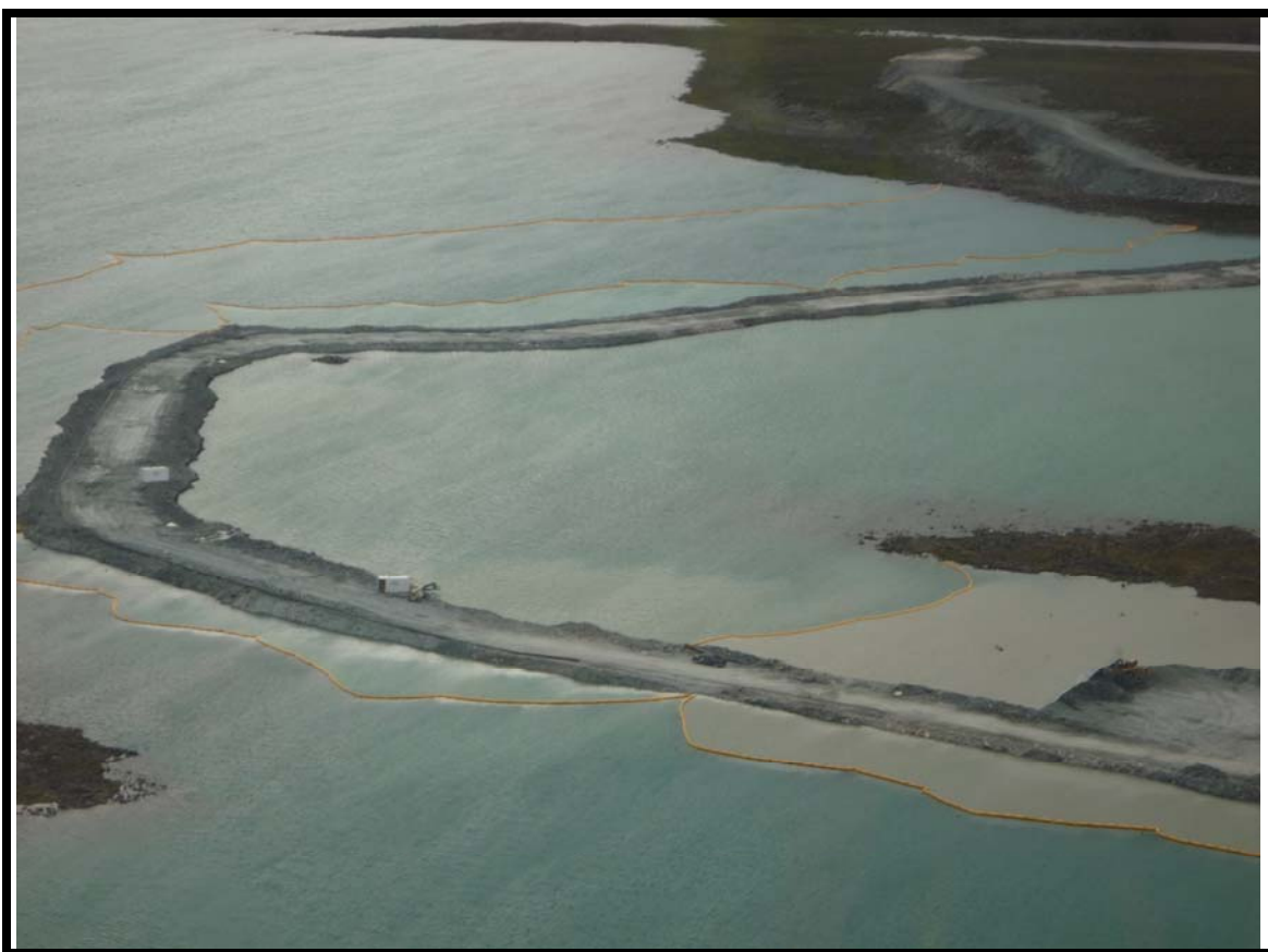
Photo No 2 : July 21, 2010 -platform advancement along causeway (bottom right hand corner)
