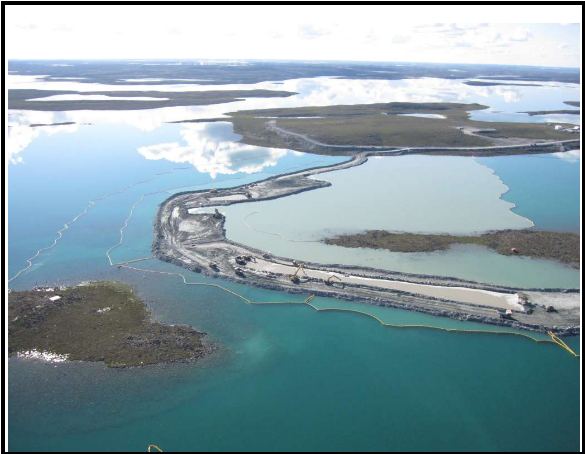
Photo No 7 : August 1st- dike and trenching advancement
