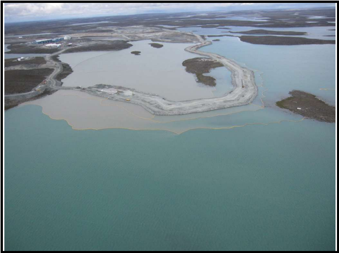
Photo No 10 : August 20 th aerial photo
