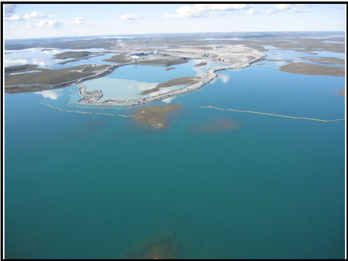
Photo No 8 : August 1st aerial photo of the entire Bay Goose dike construction area
