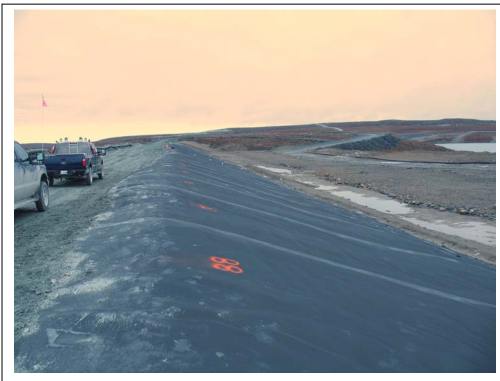
Photo #10 Saddle dam No. 2. LLDPE liner
