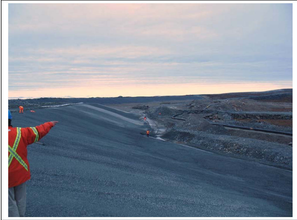
Photo #11 Stormwater Dike. Preparation of upstream slope to receive Coletanche liner
