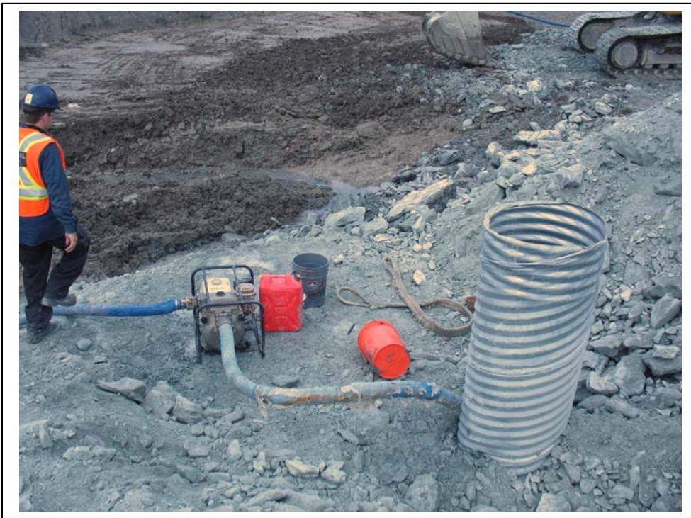
Photo #16 Cofferdam. Second sump in rockfill under construction.
