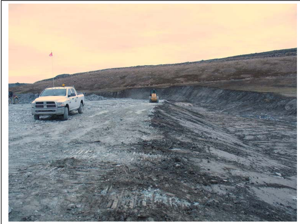
Photo #13 Cofferdam. Start of placement of impervious till zone
