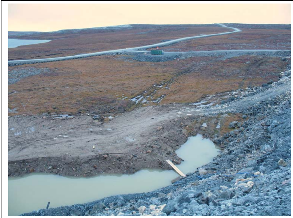
Photo #9 Saddle Dam No.1. Ponded water at downstream toe
