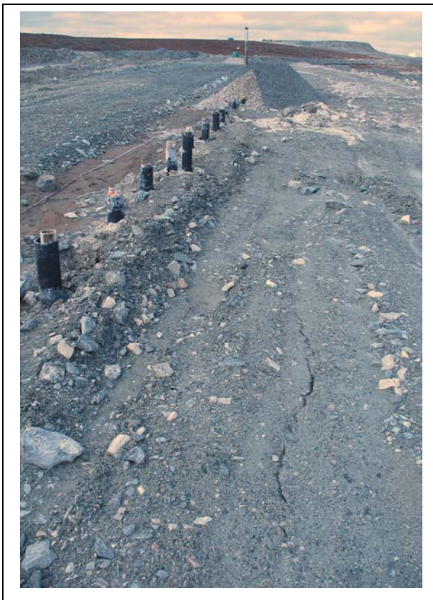
Photo #3 Rough surface of dike crest which may prevent identification of movement
