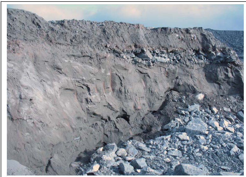
Photo #5 Portage Pit wall situated downstream of East Dike. Note contrast between overburden on left and rock on right
