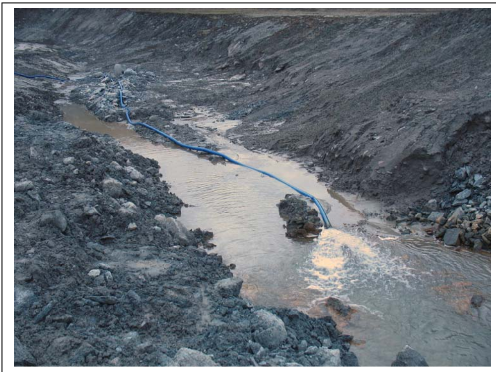
Photo #14 Cofferdam. Water pumped from sump inside rockfill.
