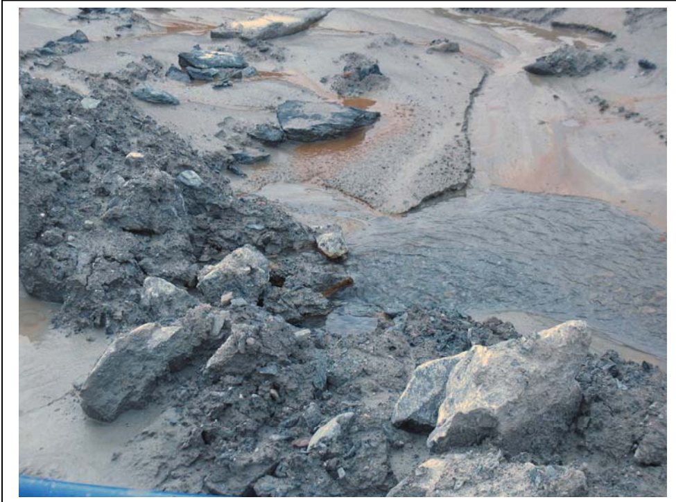
Photo #15 Cofferdam. Water welling up from un-grouted investigation borehole
