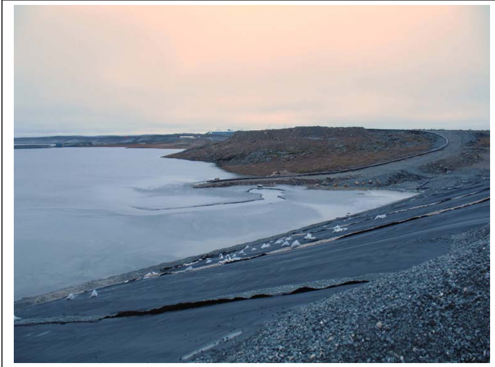
Photo #7 Saddle Dam No.1. Tailings deposit at left abutment
