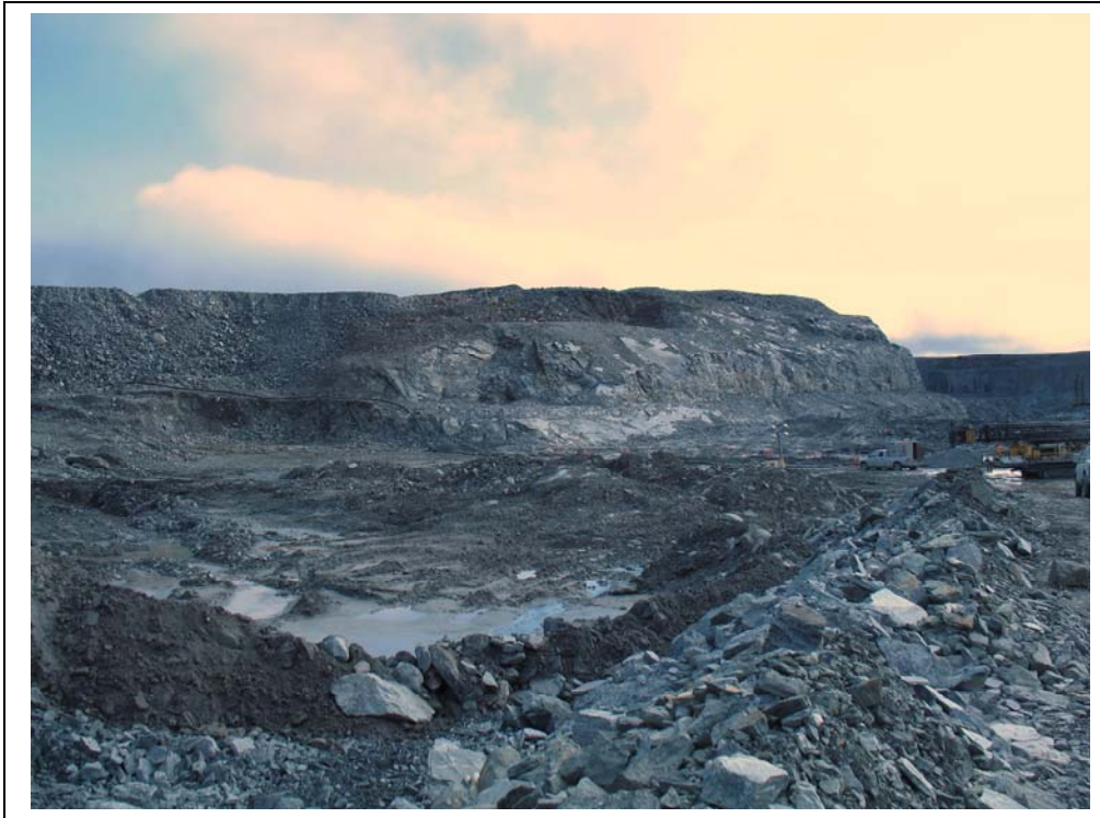
Photo #5 Portage Pit wall situated downstream of East Dike. Note contrast between overburden on left and rock on right
