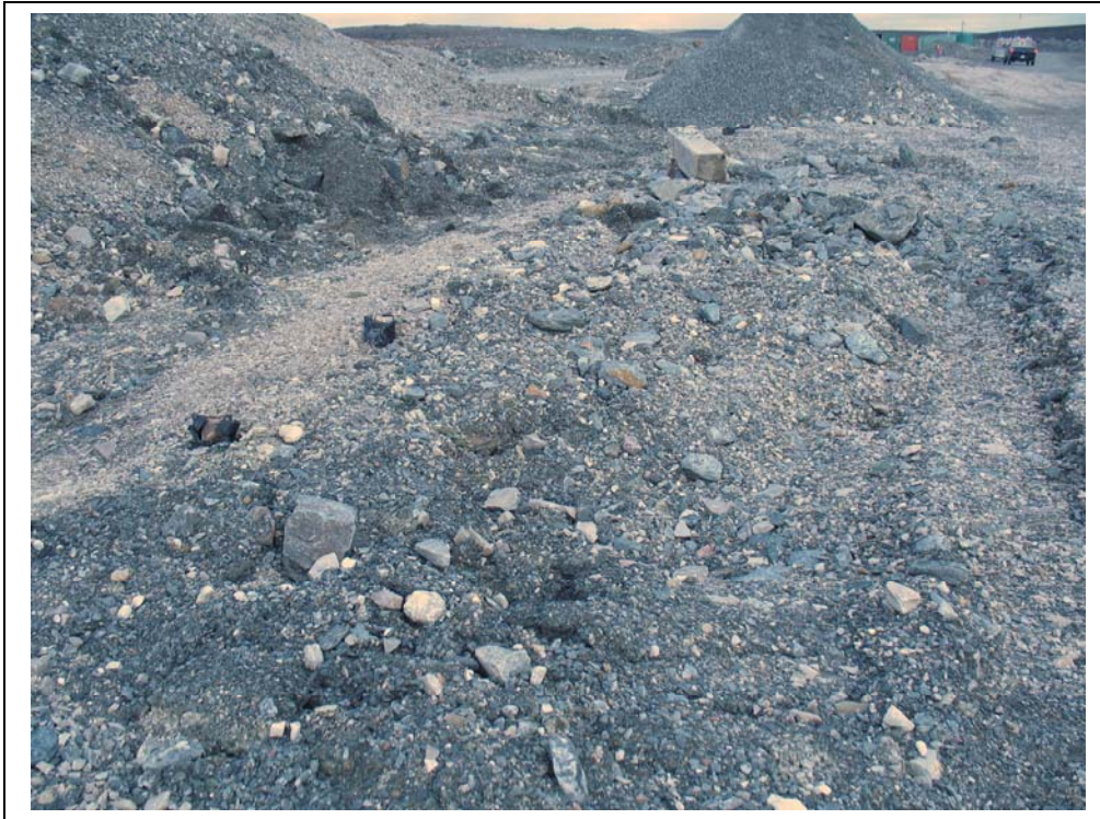
Photo #3 Rough surface of dike crest which may prevent identification of movement
