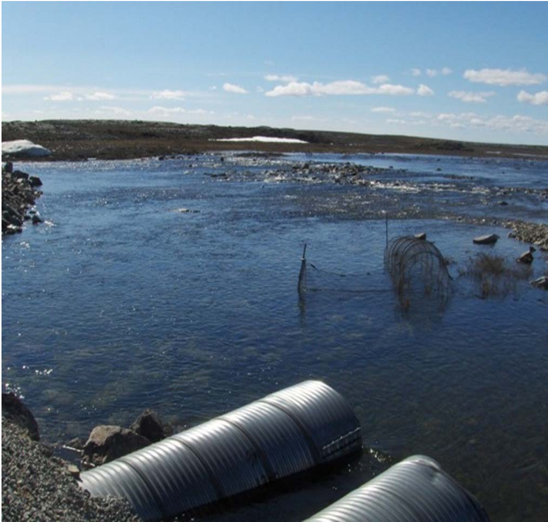
R02 Culverts – June 26, 2011
