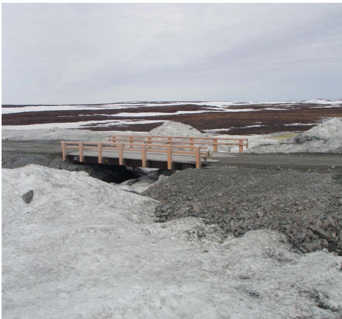
R09 (KM 49) DS of Bridge – June 15, 2011
