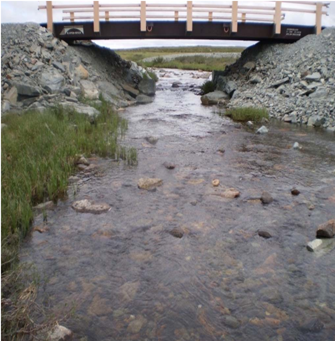
R09 (KM 49) DS of bridge – July 16, 2011
