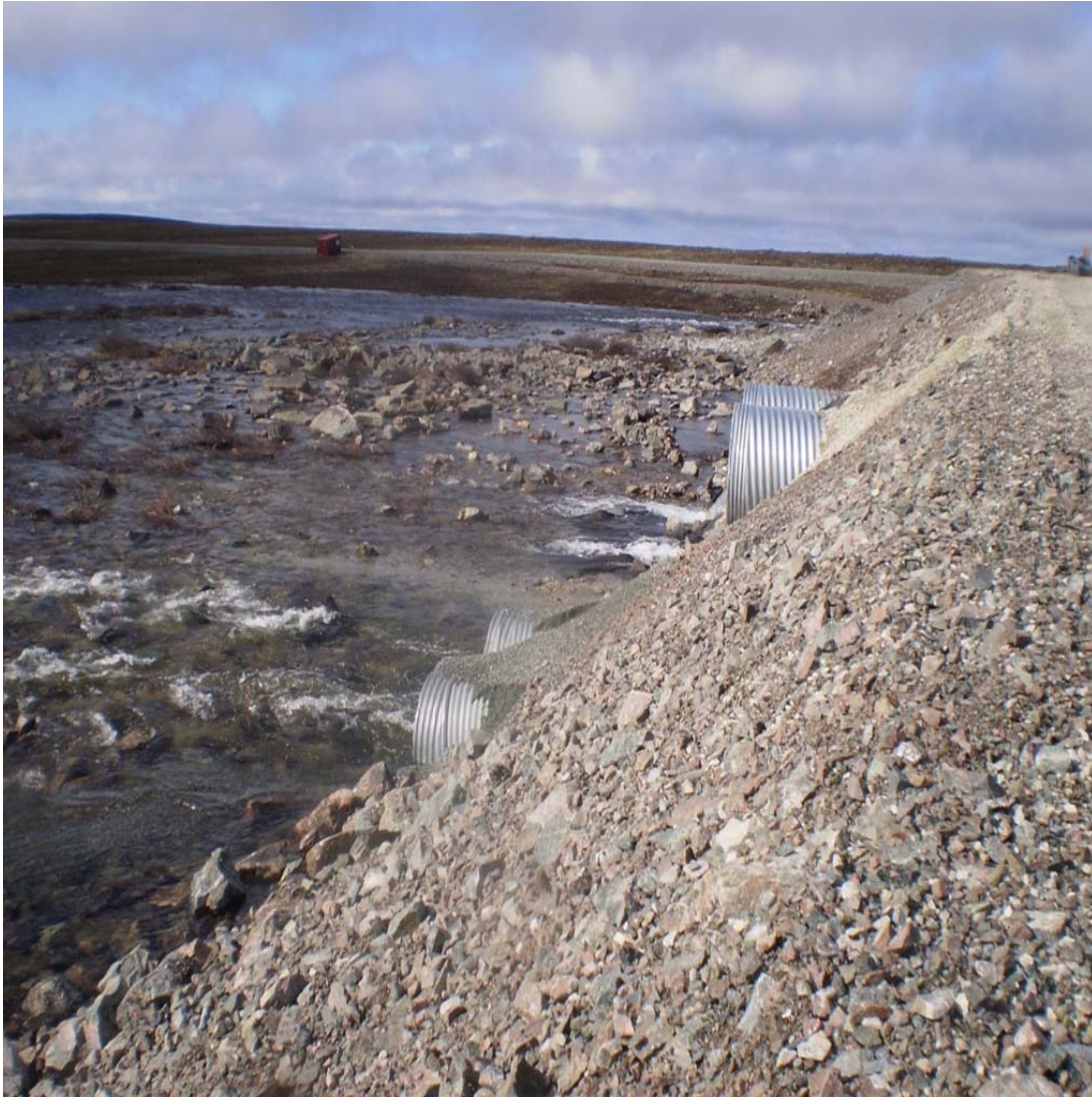
R02 DS Culverts – June 26, 2011
