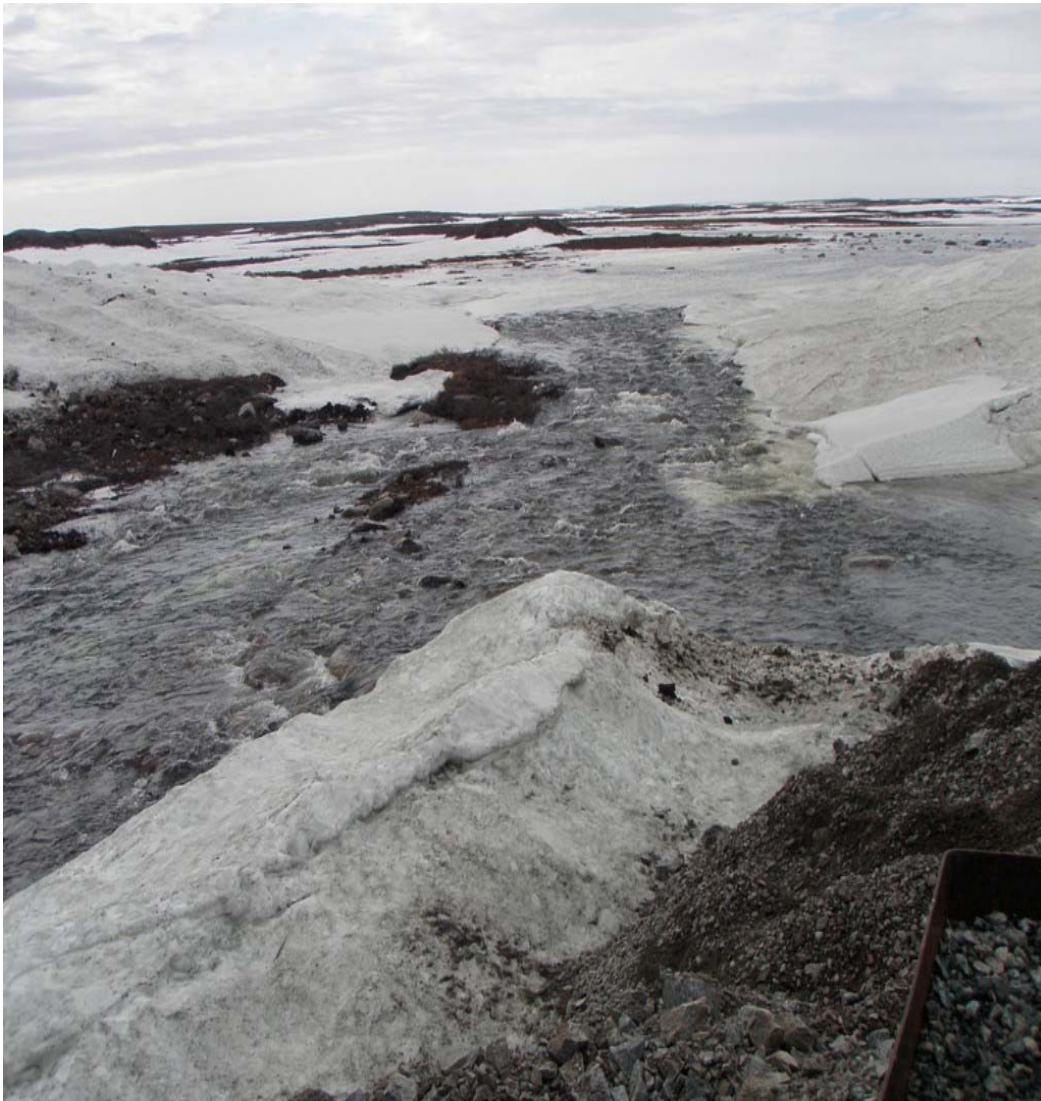
R02 US of Bridge – Upstream flow at R02 – June 15, 2011
