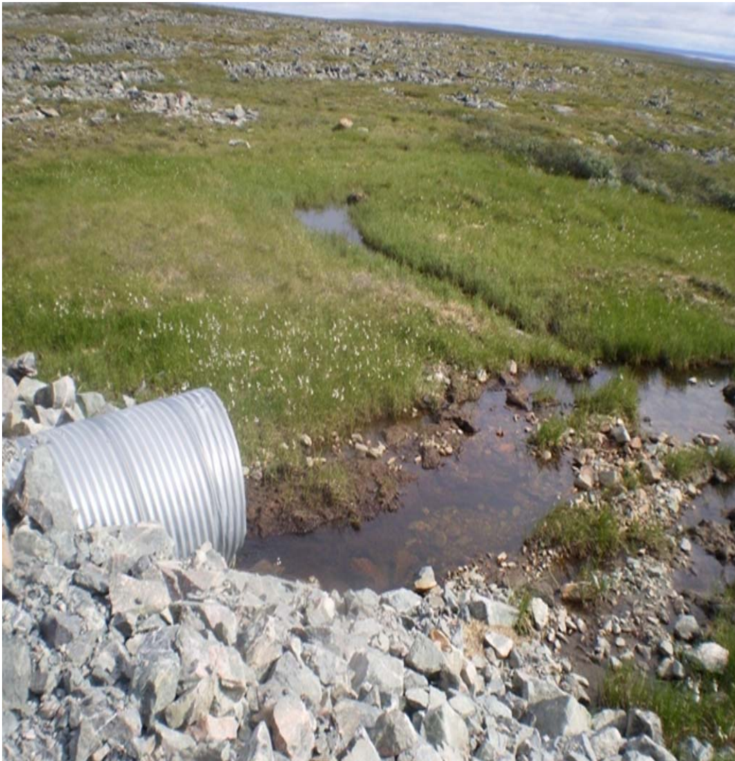
Water levels continue to recede – Culvert at KM 26 – July 16, 2011
