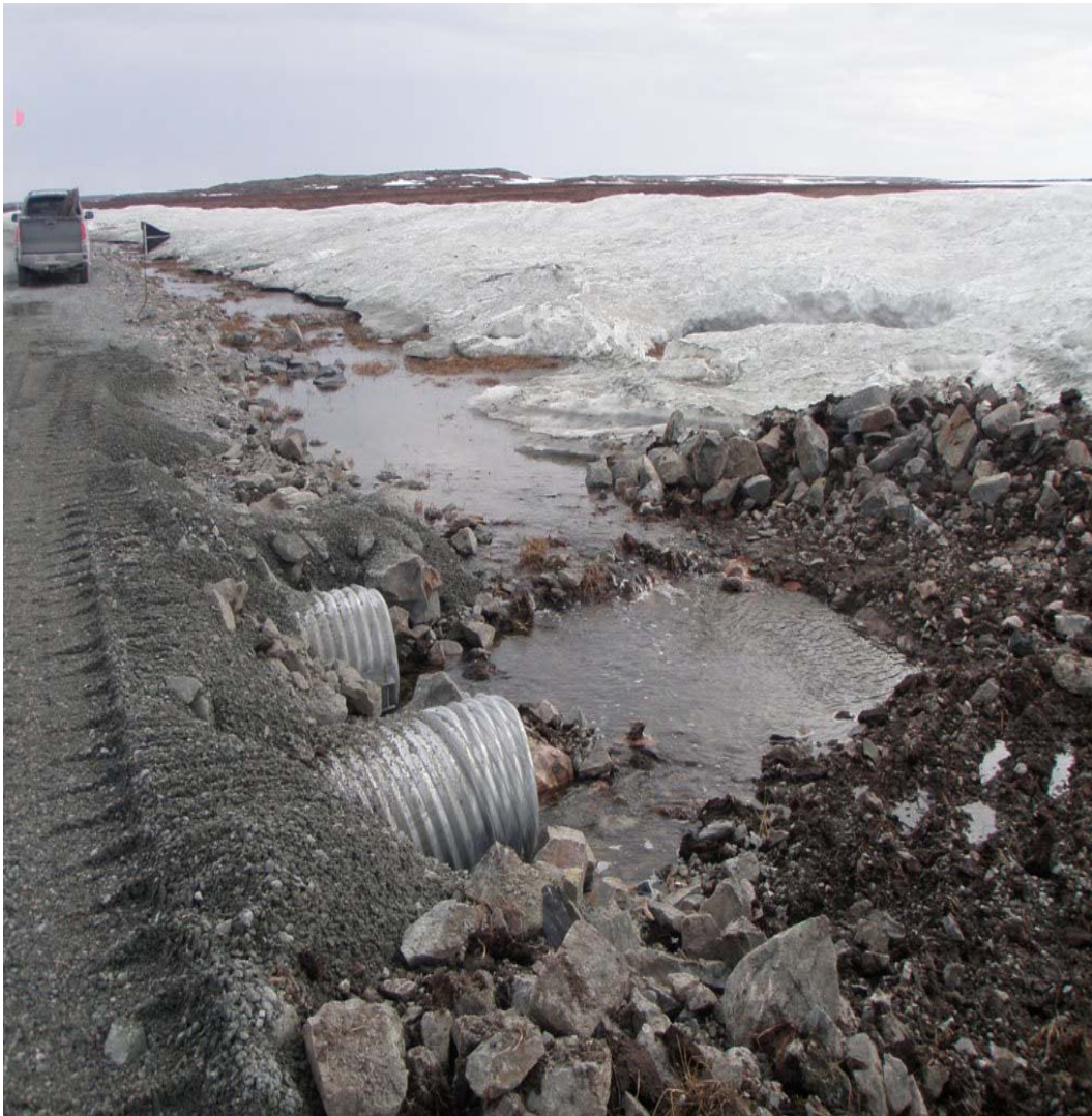
Culvert at KM 22 collecting run off – June 15, 2011
