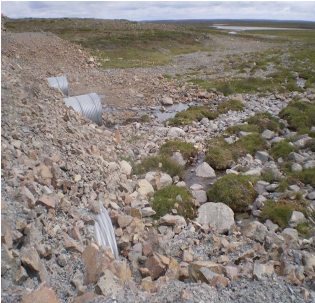
Nearly dry culvert at KM 68 – July 16, 2011
