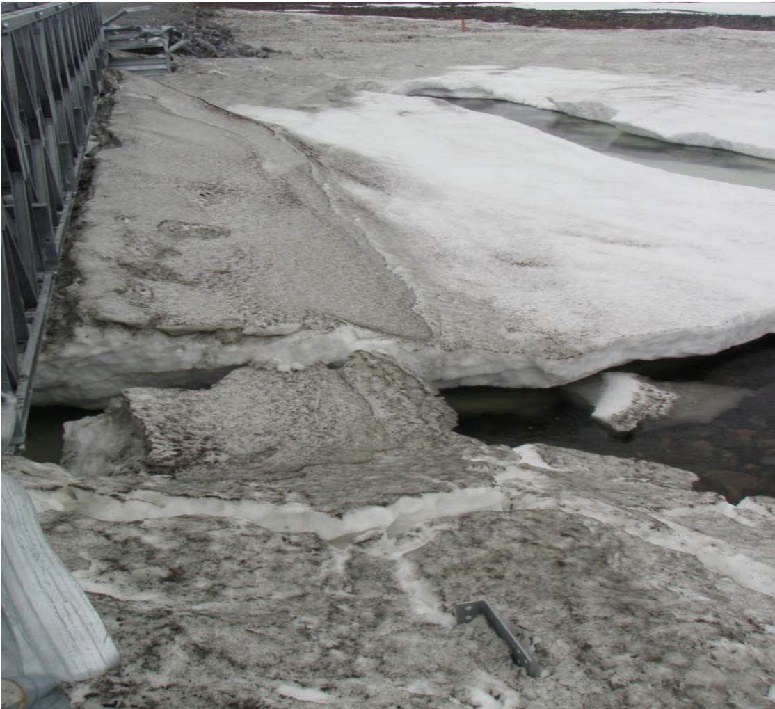
R15 Bridge (KM 70) Snow covering bridge abutments – June 15, 2011
