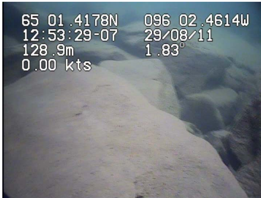
Photo D.1-2. SP-ED-1; North end of East Dike. Thin layer of sediment on boulders is also evident.
