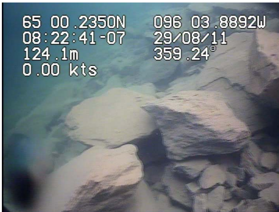
Photo D.3-10. TPE-BGS-5; Southwest end of Bay Goose Dike South. Some sediment is evident on surfaces of angular boulders.
