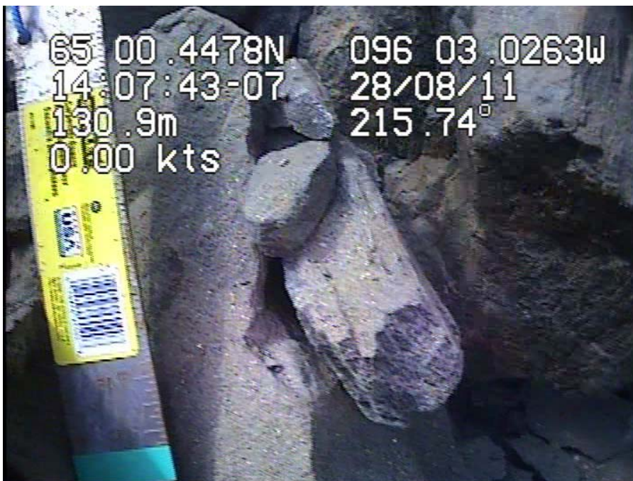
Photo D.2-10. TPE-BGN-5; South end of Bay Goose Dike North. No periphyton visible on any surfaces; reference gauge along angular boulders.
