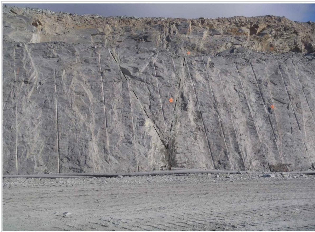
Photograph 33: Bench scale wedge formed by south dipping joint and north dipping sheared joint in the east wall of the Goose Pit. Viewed from 5,116 RL.
