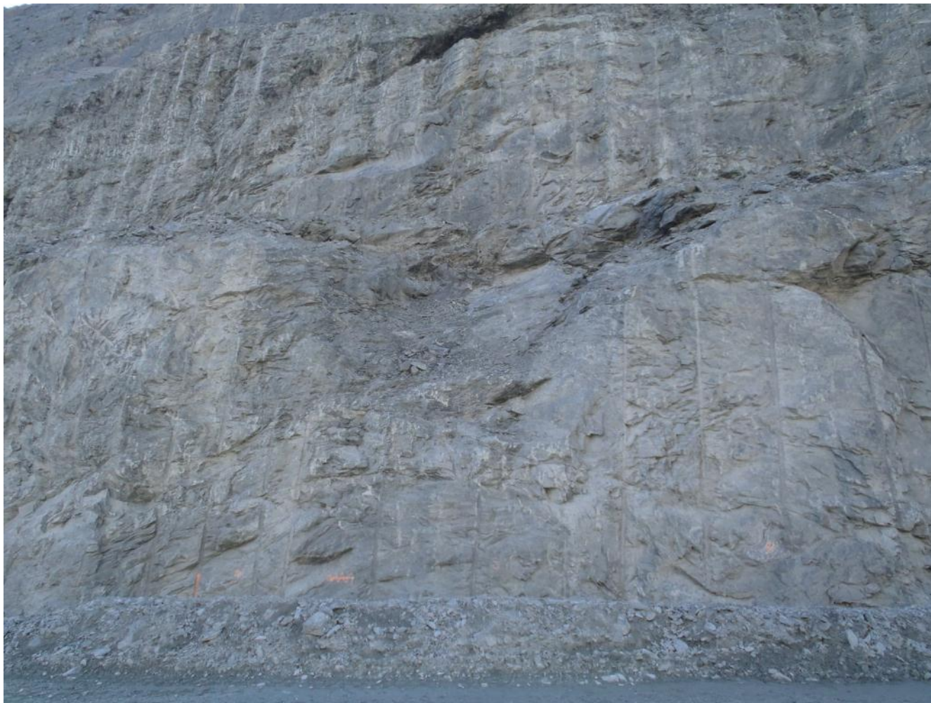
Photograph 24: Scallop-type structure in the west wall of Pit E, adjacent to ramp, with containment berm at base
