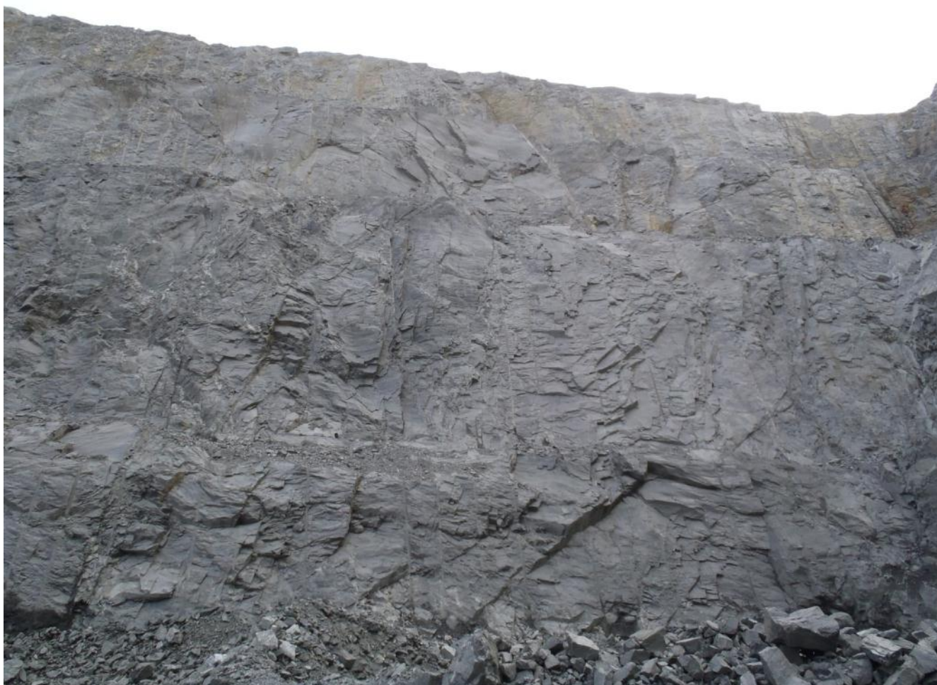
Photograph 28: Pit E east wall showing bench faces breaking to foliation
