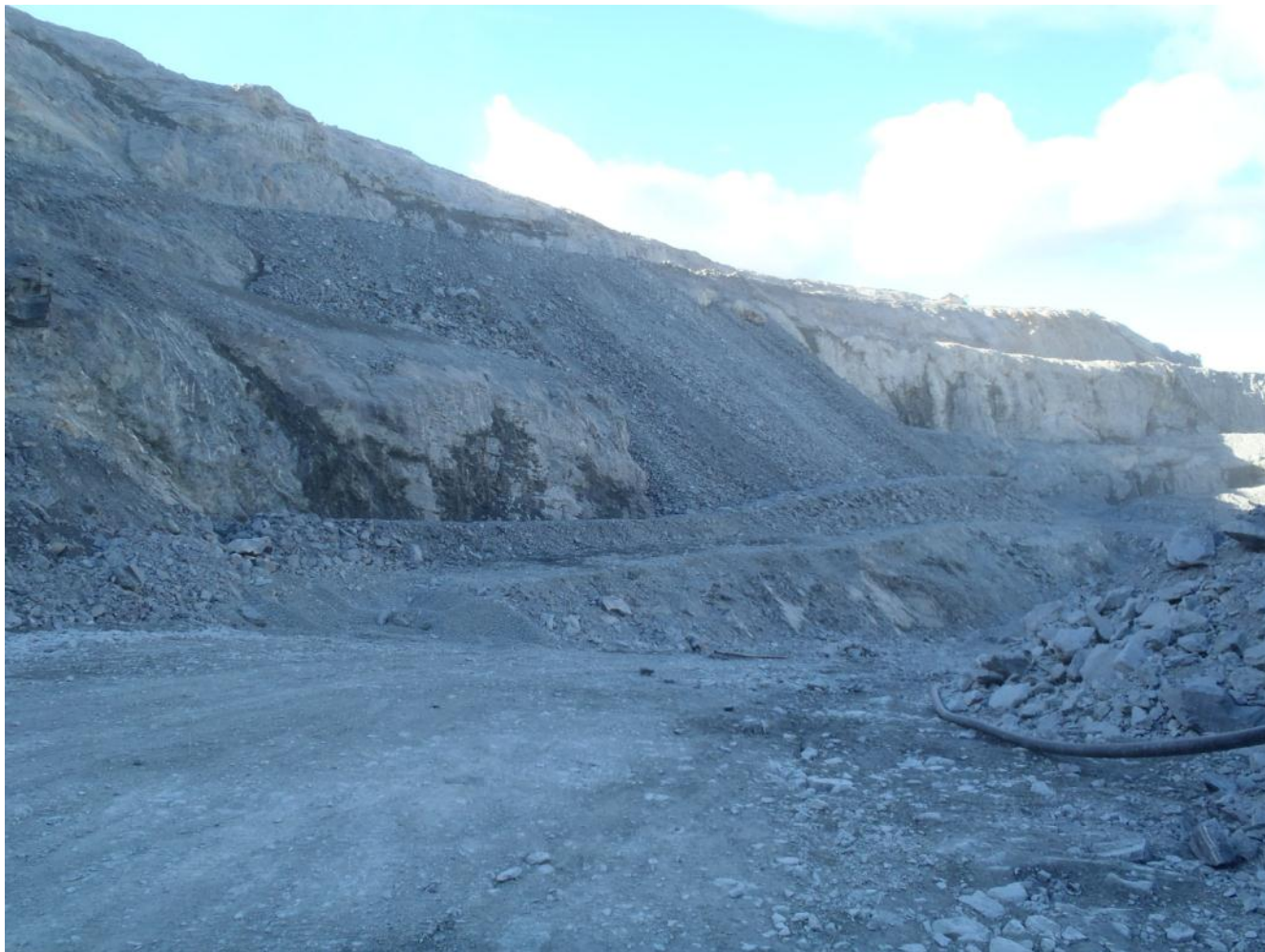
Photograph 18: Buttrressing of slope below ramp on the west wall of Pit D
