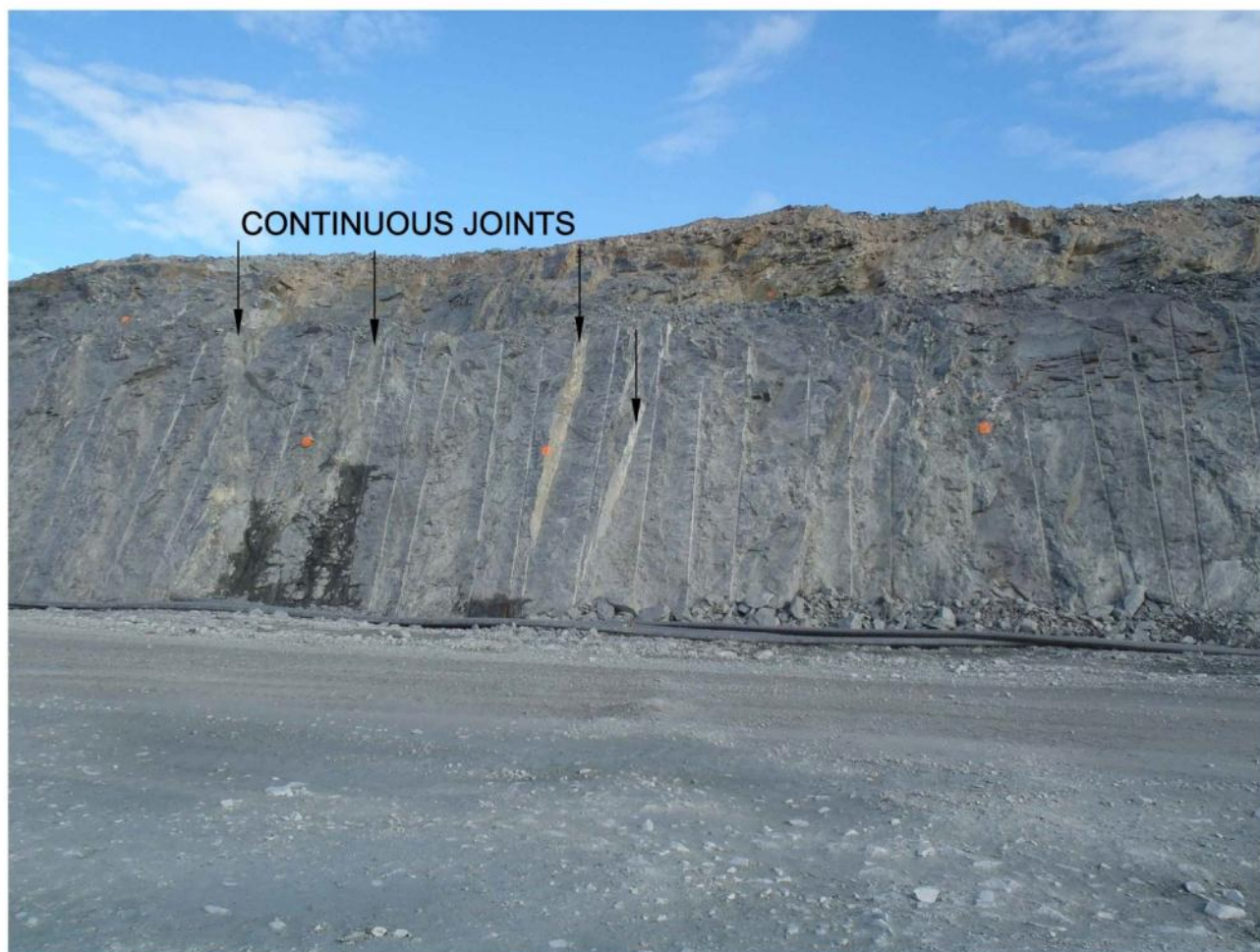
Photograph 38: Steep north- and south-dipping continuous joints exposed in east wall (potential side release planes)
