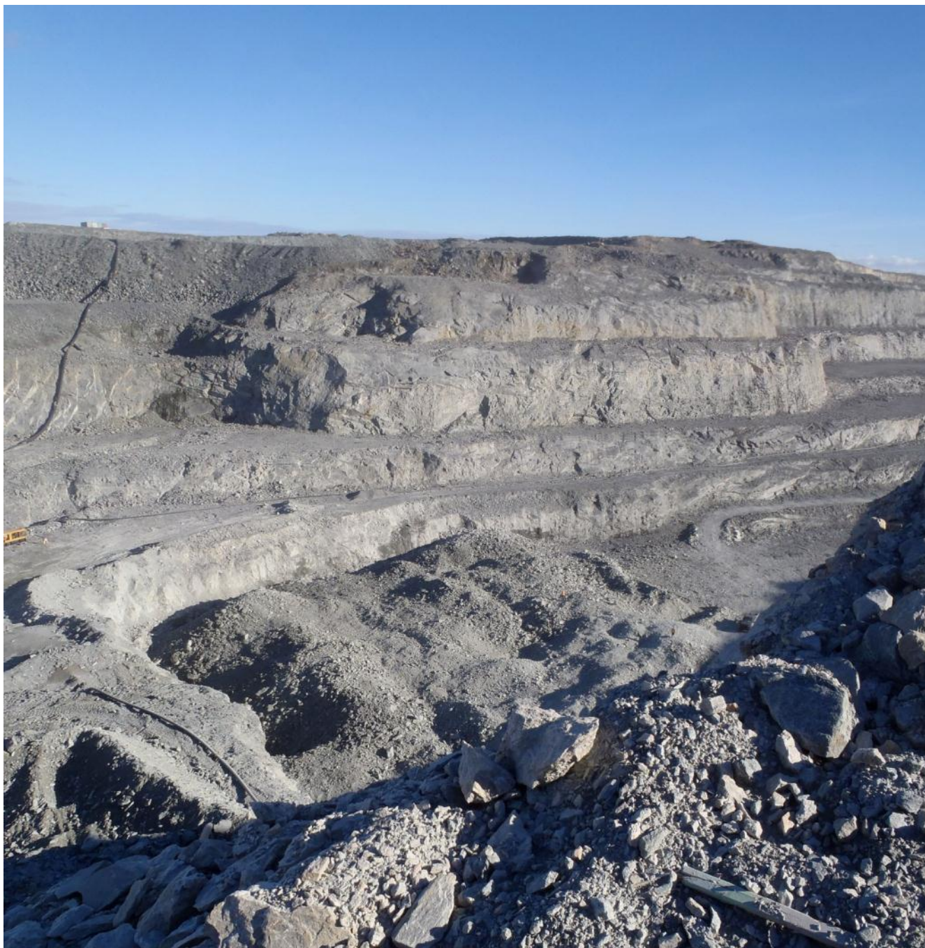
Photograph 20: East wall of Pit D showing loss of catchment looking southeast
