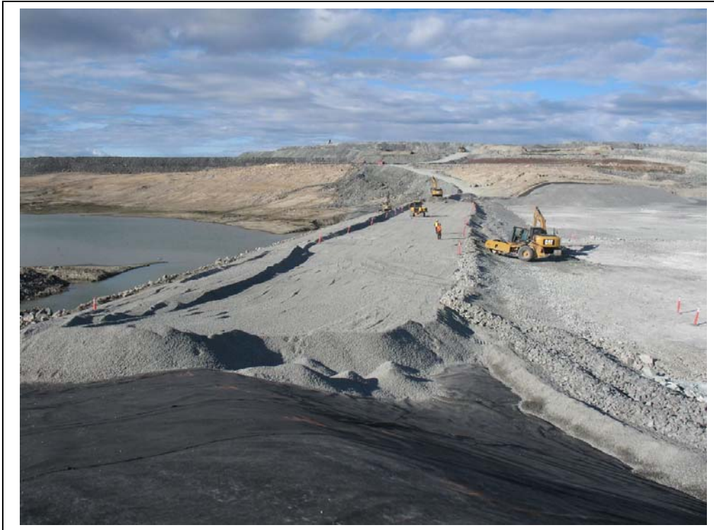
Photo #1 Central Dike, fill over U/S cofferdam
