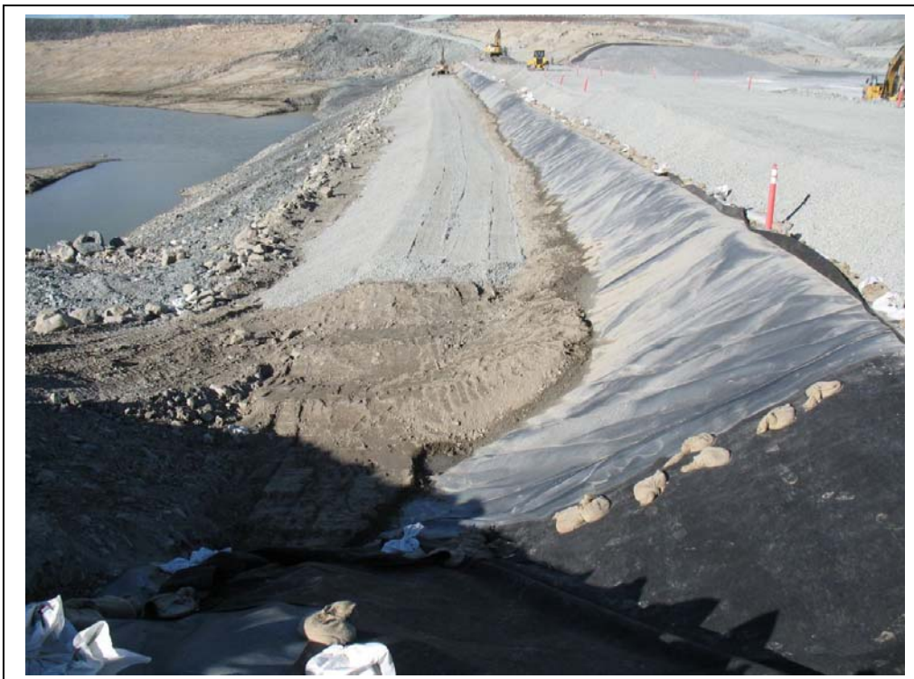
Photo #2 Central Dike, liner extension tied into cofferdam fill
