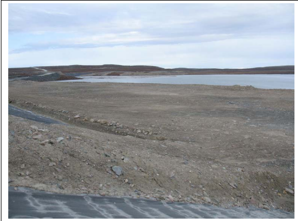
Photo #11 Saddle Dam #2, till placed as beach
