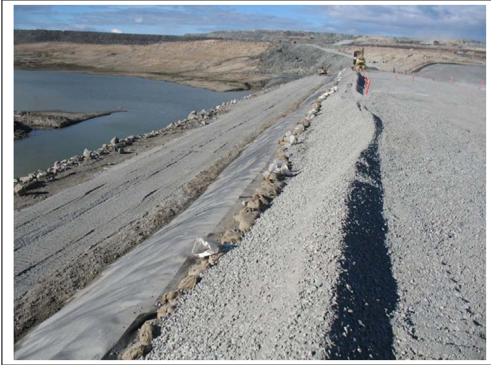
Photo #3 Bench to tie in U/S face liner. Too narrow.
