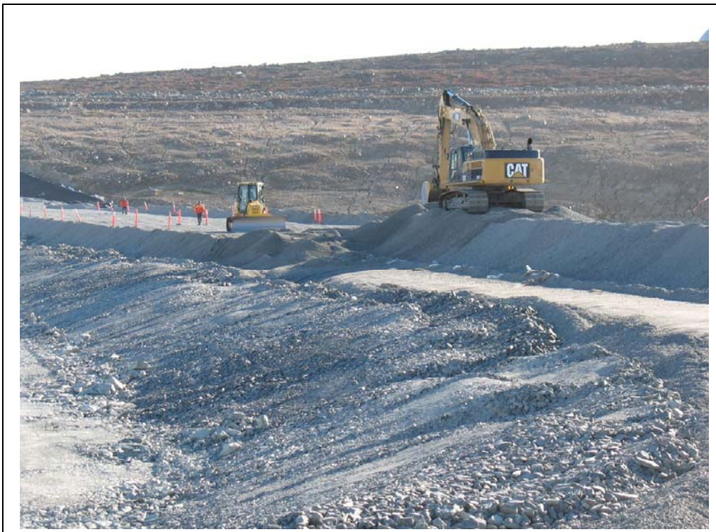
Photo #4 Redistribution of filter layer from thick layer designed to protect liner
