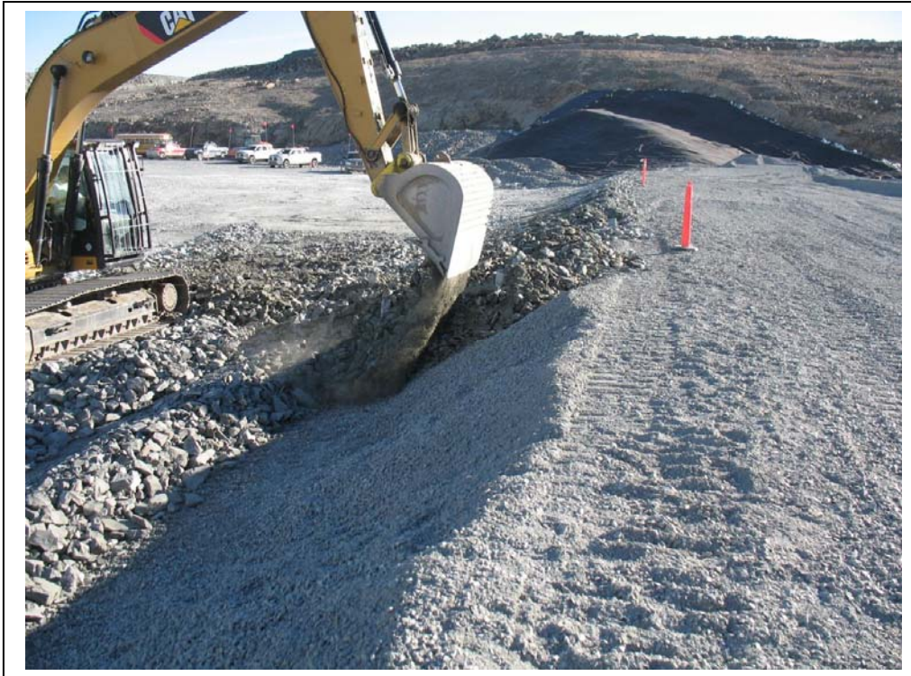
Photo #5 Placing of coarse filter
