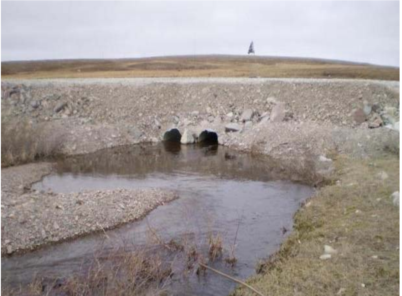
LFP2APL DS Culverts – June 24, 2012
