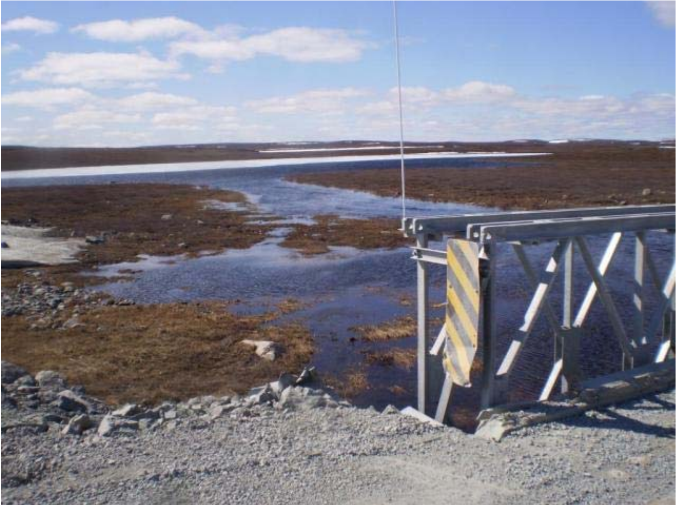
Upstream view of R05 Bridge at KM 17 – June 18, 2012
