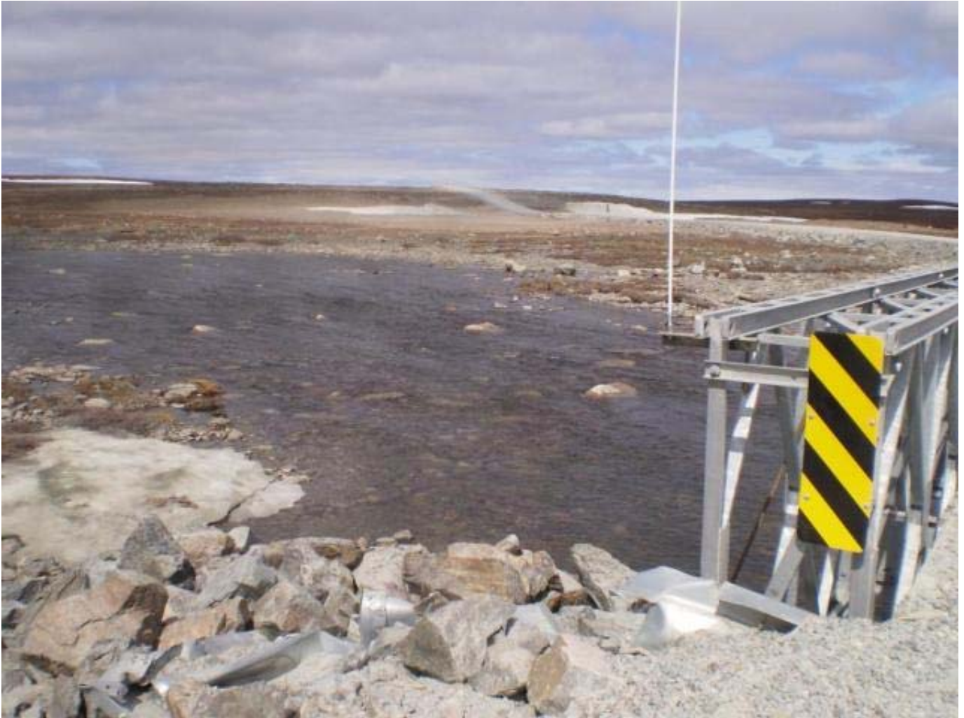
Upstream view of R15 Bridge – Jun 18, 2012
