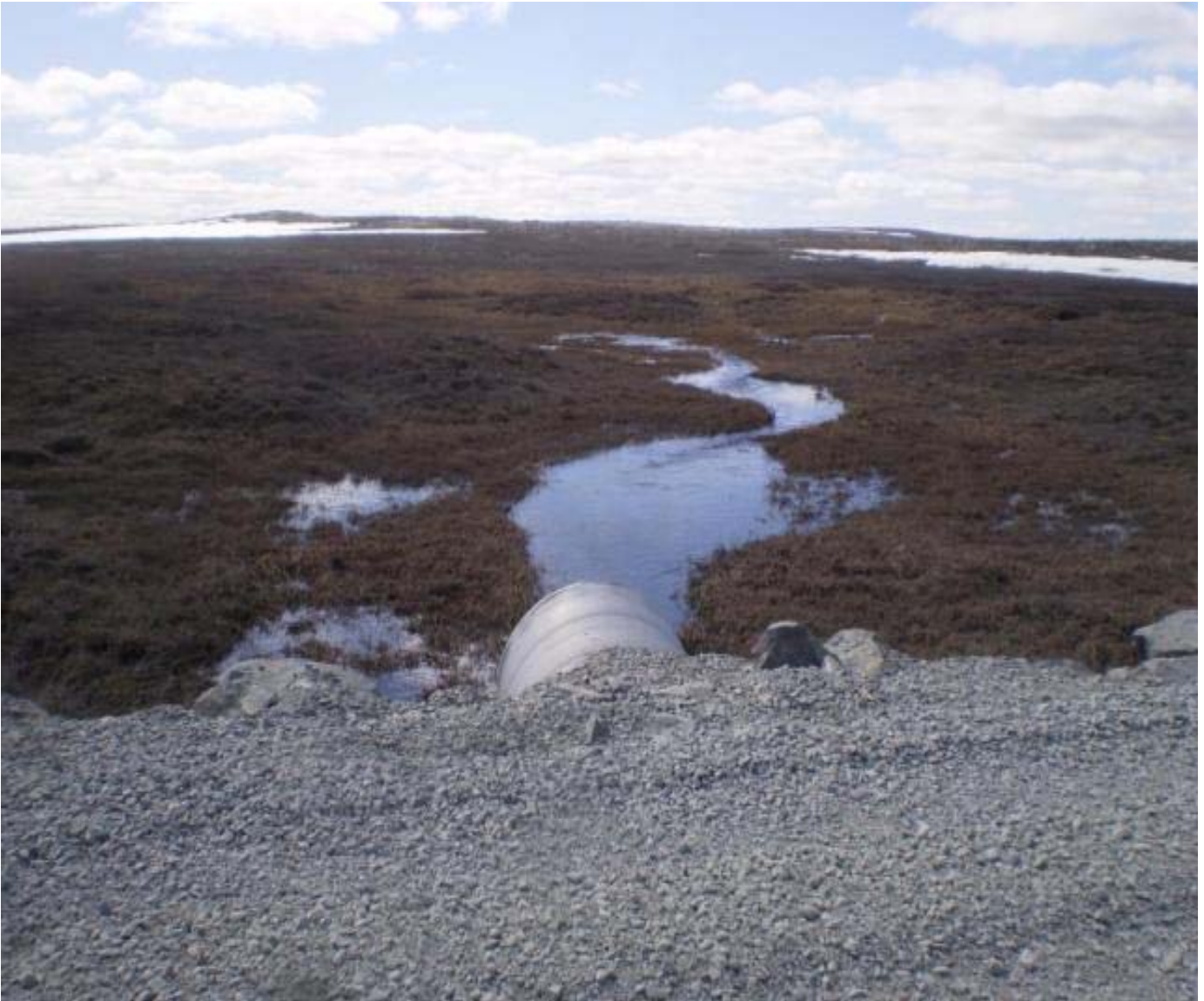
KM 25 US Culverts – June 18, 2011
