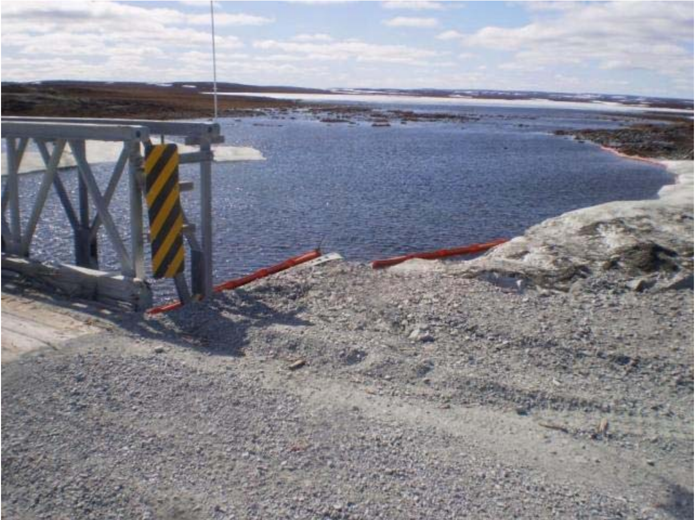
Upstream view of R06 Bridge at KM 22/23 – June 18, 2012
