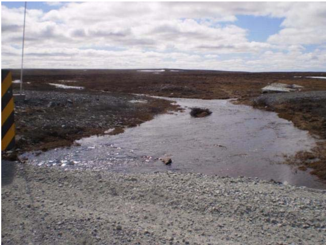
Upstream of R09 Bridge at KM 49 – June 18, 2012
