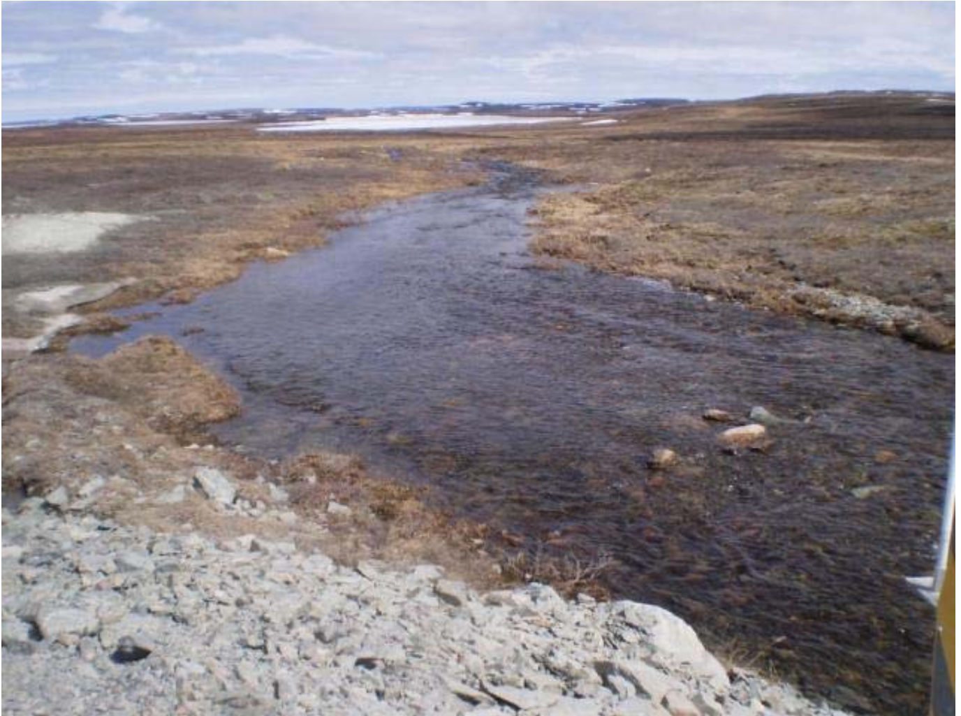
Downstream view of R09 Bridge at KM 49 – June 18, 2012
