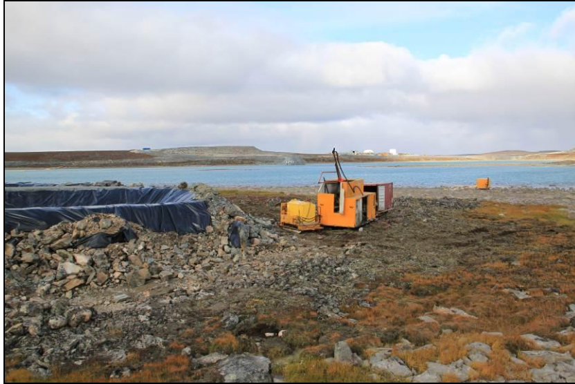
Photo 16: Drilling of groundwater well, near Bay-Goose basin (photo taken September 2011)
