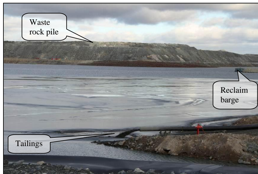
Photo 12: Tailings storage facility – north cell
