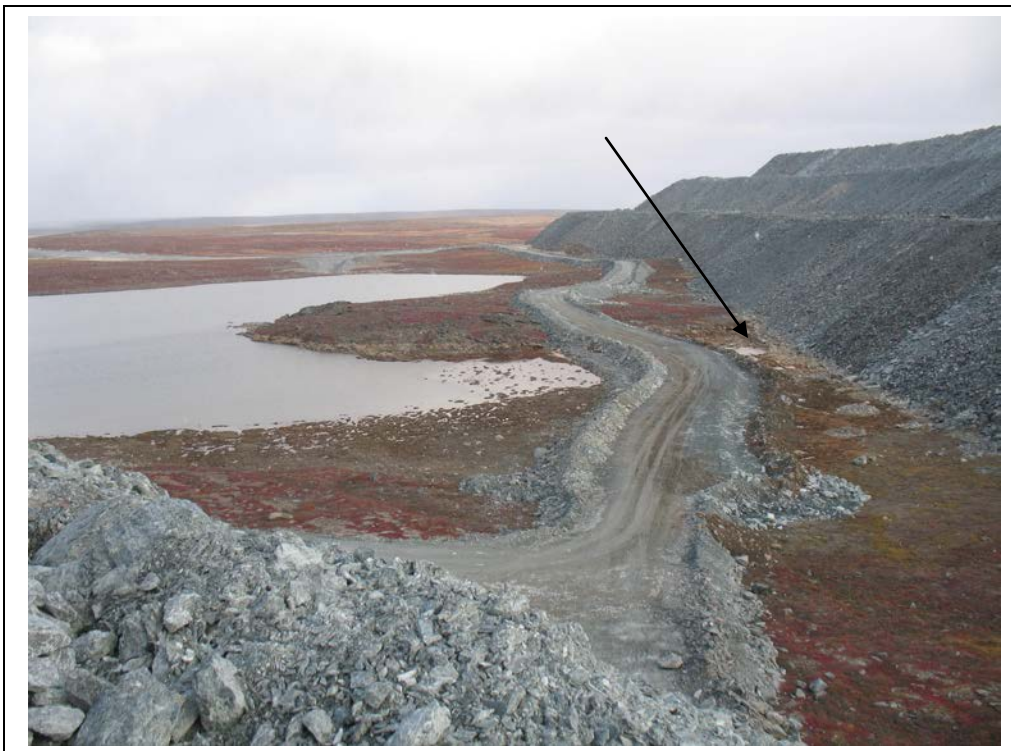
Photo #4 Site of seepage observations at waste rock pile. Pond RP-2
