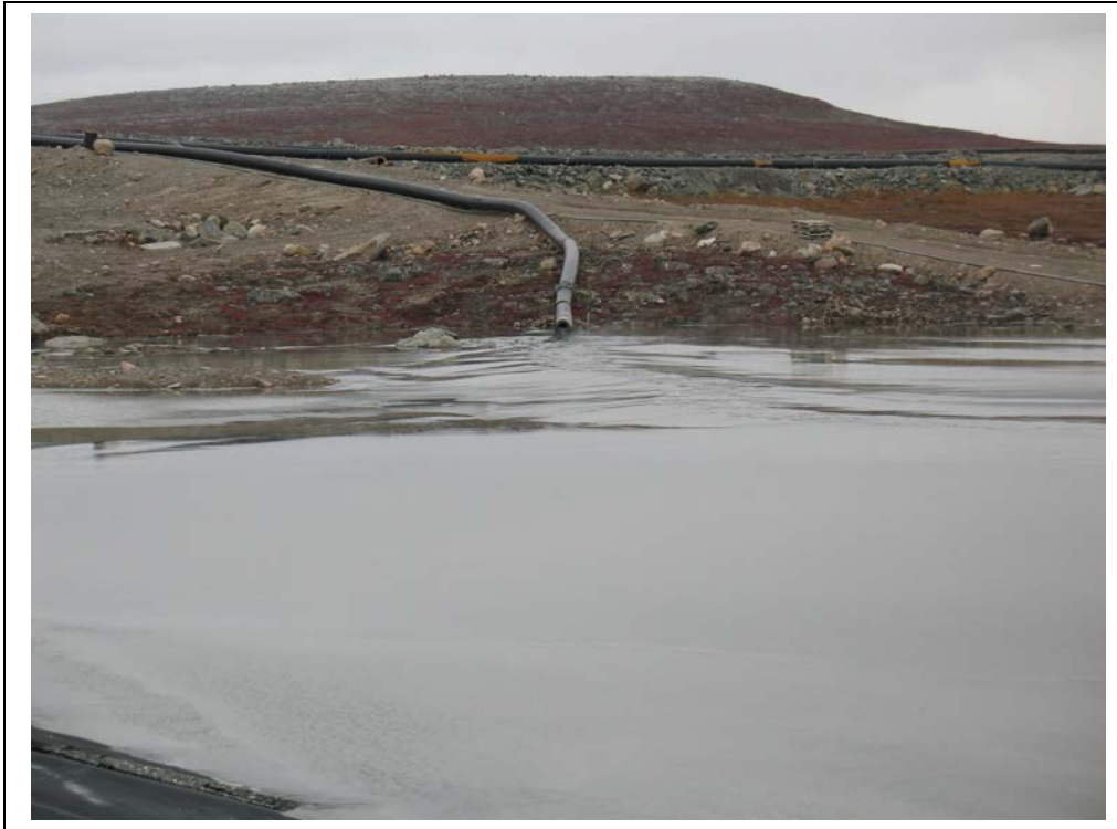
Photo #1 Saddle Dam No. 1 Note single large diameter tailings outfall
