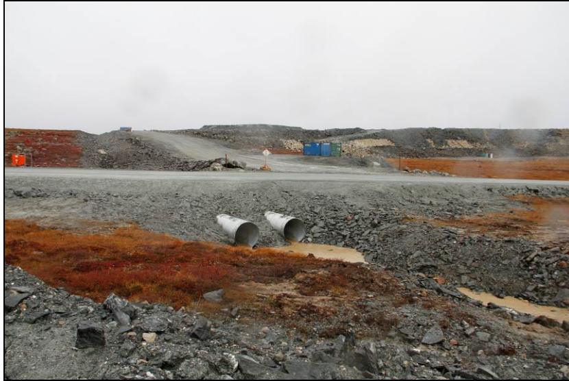
Photo 12: Diversion ditch around tailings facility
