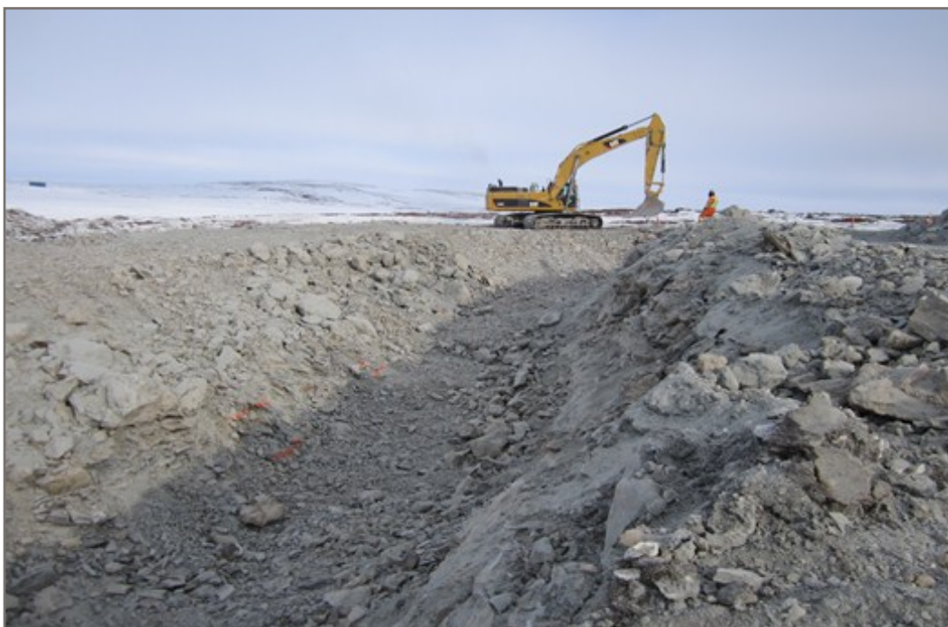
Photo 9: West End of Interception Trench Facing Northwest Trench Bottom Prior to Cleaning
