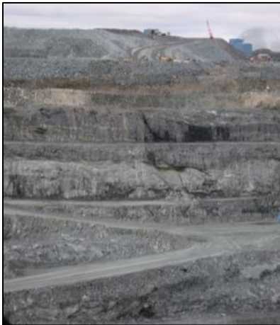
Photo 11: Moisture moving between the rock layers of the west wall of the South Portage pit
