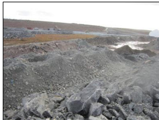
Photo 26: Berm around the landfarm site.
