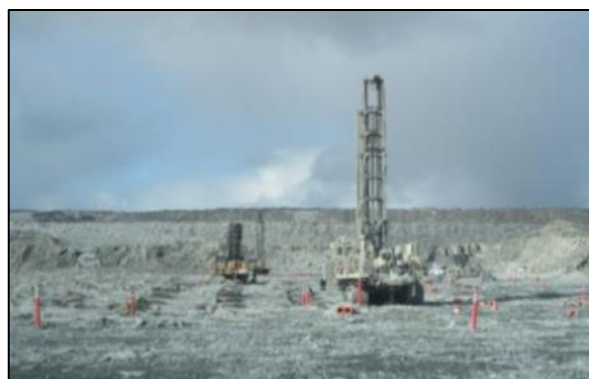
Photo 17: When drilling is completed, pylons will be overturned and placed in the holes.
