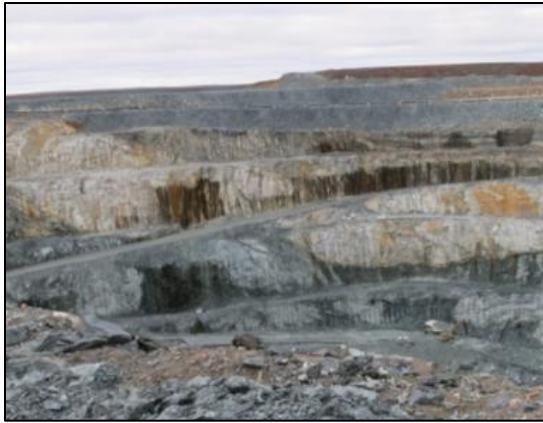
Photo 9: Moisture along southern wall of Bay-Goose pit.
