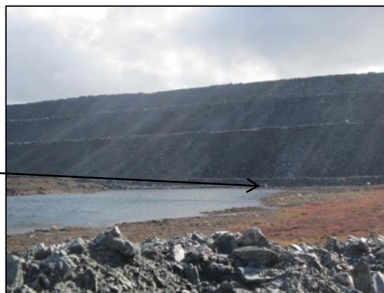
Photo 41: View of NP-2 Lake and the point of seepage at the Portage waste rock storage facility.
