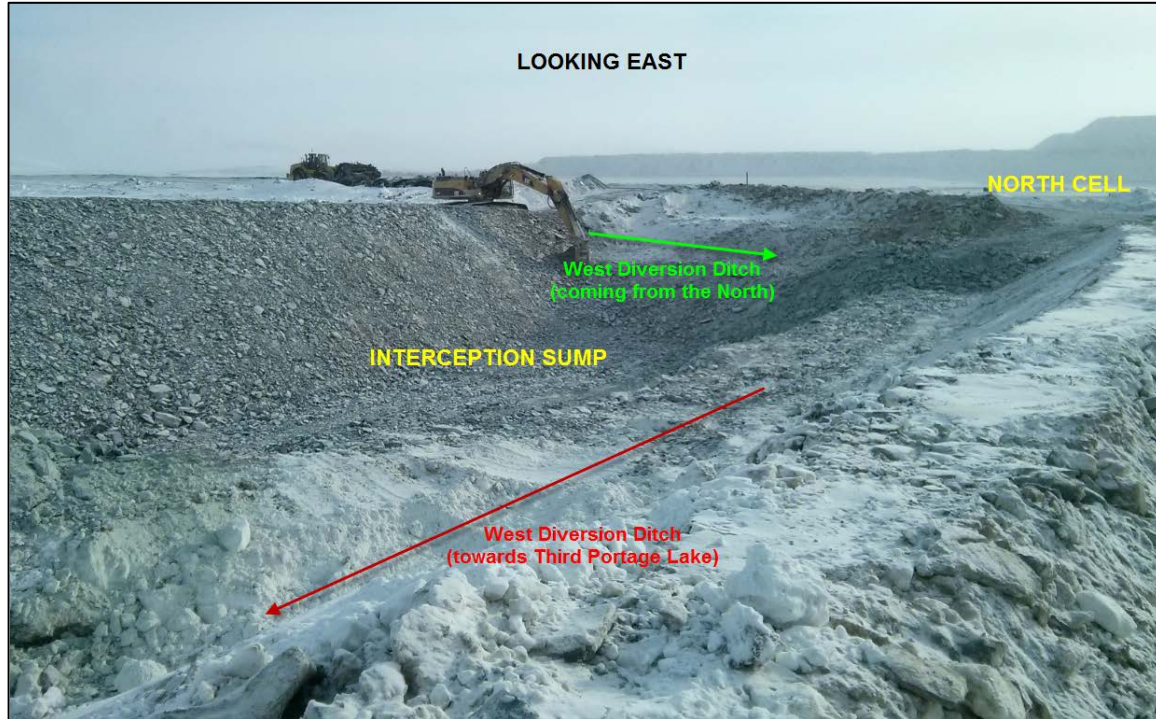
Figure 2-8: North Cell West Diversion ditch interception sump
