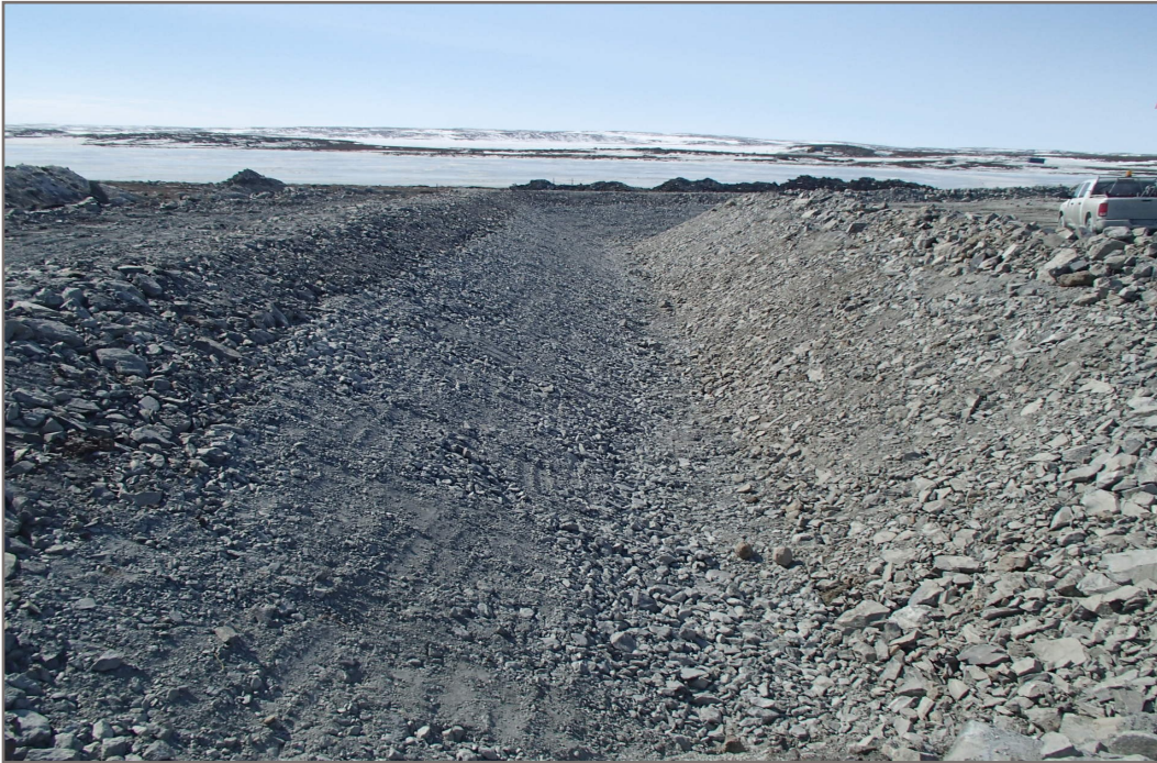
Photo 17: East End of Interception Trench Facing Southwest Completed Interception Trench Covered in Rockfill (Photo courtesy AEM)
