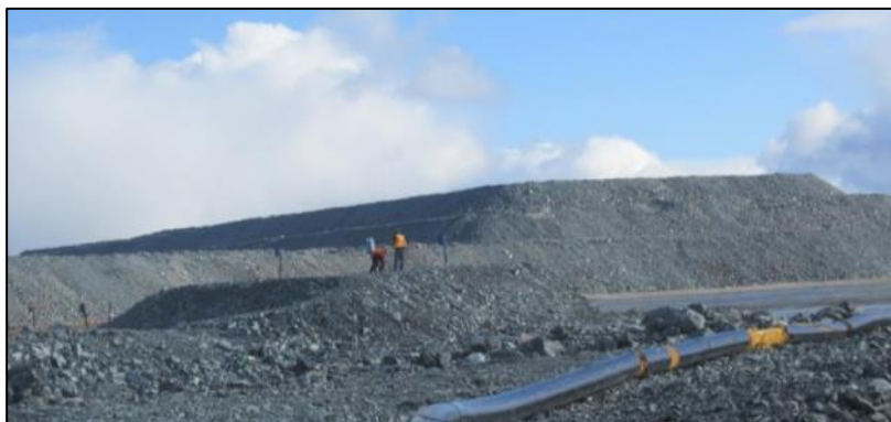
Photo 33: Test pads in the tailings storage facility for closure capping.
