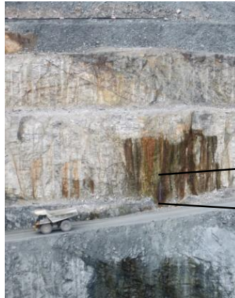
Photo 30: Seepage in the south wall of the Bay-Goose pit.
