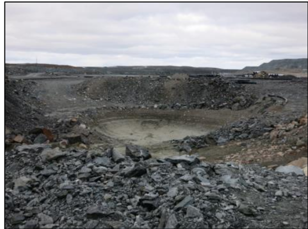
Photo 12: Slumping observed as water from Second Portage Lake seeps through the East dike.
