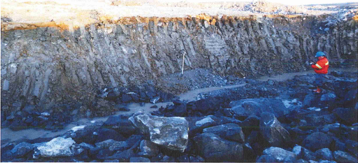
Figure 1: Granular channel observed in the in situ till of the Stormwater Dike foundation in 2009.
