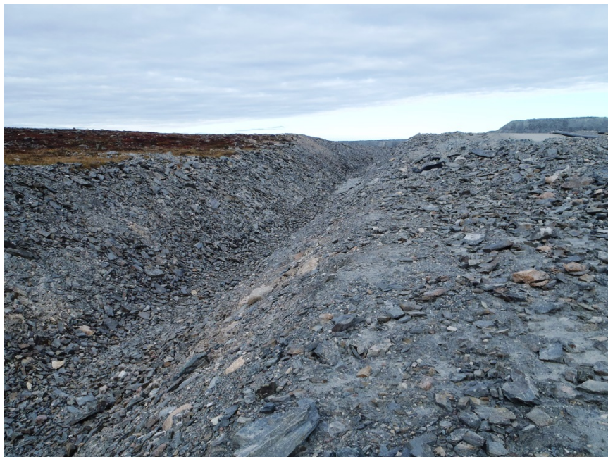
Photograph G2-13 Diversion Ditch and its Sediment and Erosion Protection Structure
