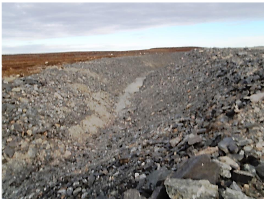
Photograph G2-4 Diversion Ditch and its Sediment and Erosion Protection Structure
