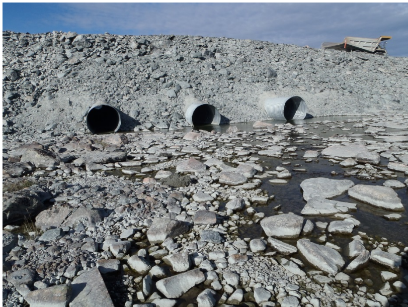
Photograph G1-4 Vault Road Culverts
