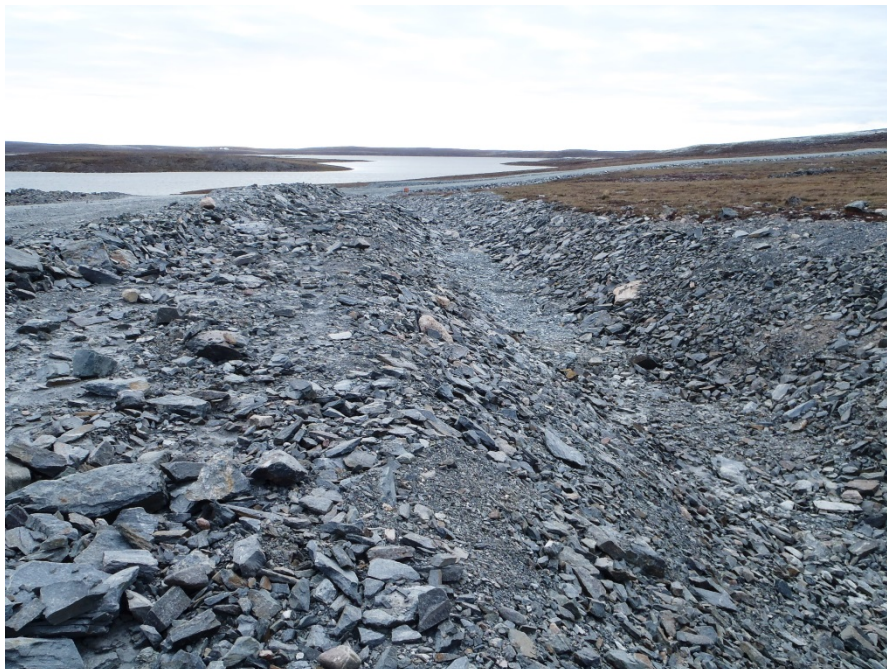
Photograph G2-14 Diversion Ditch and its Sediment and Erosion Protection Structure
