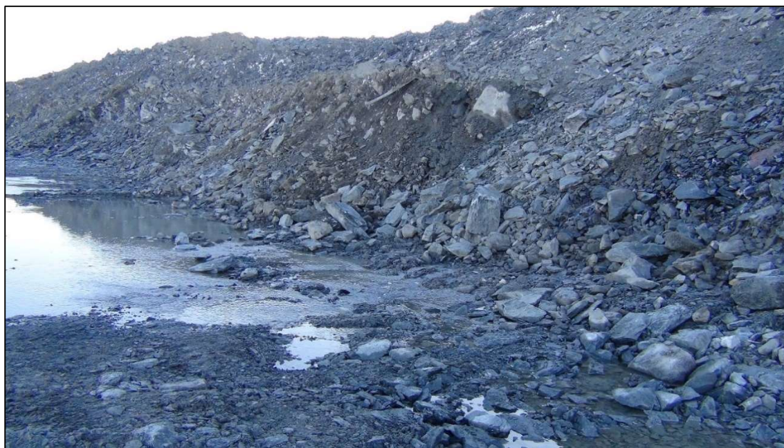
Photograph 8-12: Vault Pit flowing water from seepage face on downstream side of ring road (5130 mRL)
