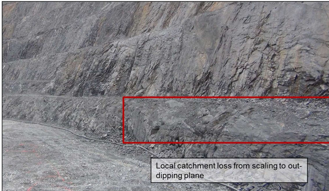
Figure 6-2: Example of catchment loss from scaling to out-dipping plane
