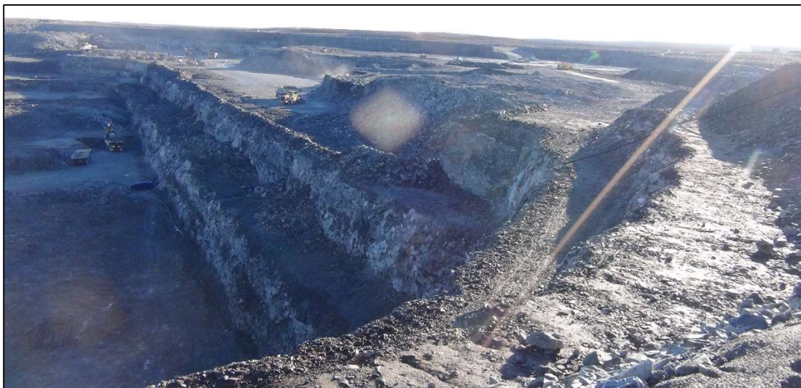
Photograph 8-7: Vault Pit grid south wall upper catch benches
