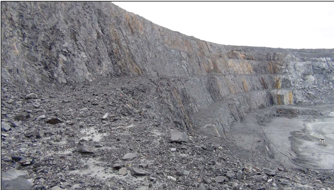
Figure 6-1: East wall showing good bench and wall performance
