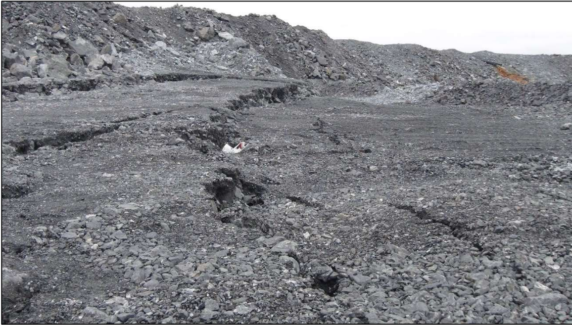
Photograph 7-6: Goose Pit dump tension cracks
