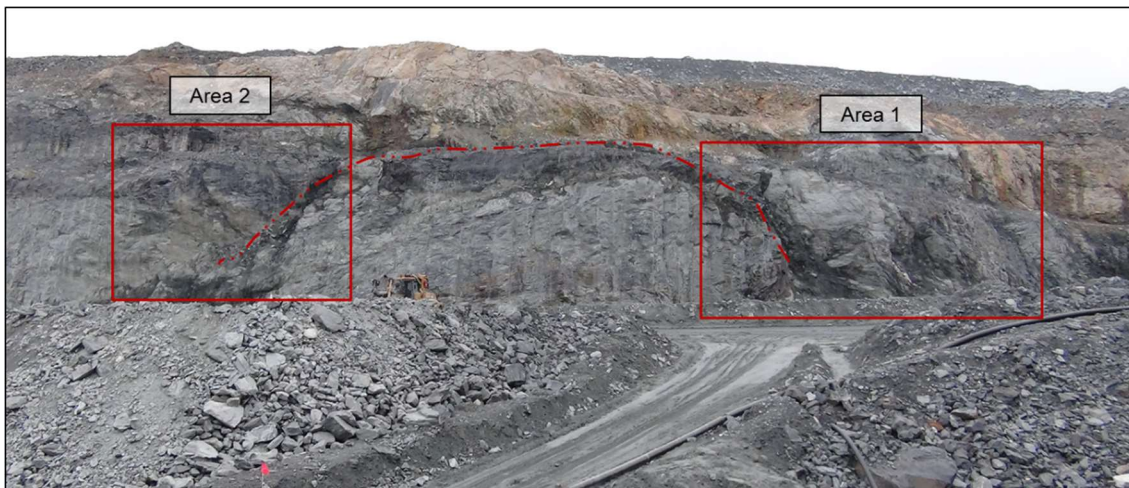
Photograph 6-7: Pit E3 Ramp Areas 1 and 2 - Bay Fault or splay
