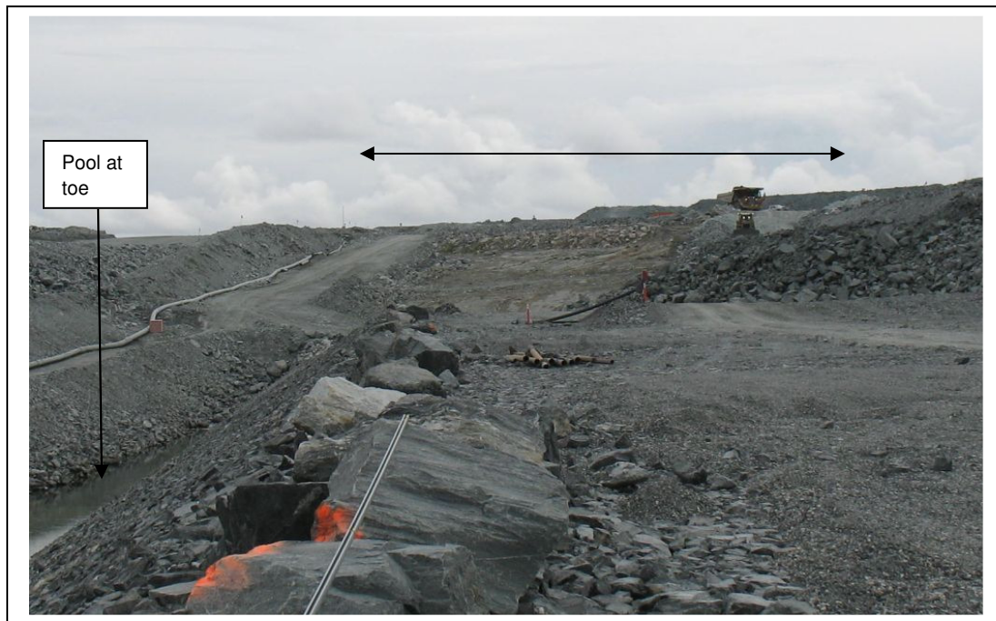
Photo #7 Central Dike, downstream toe, south catchment area extending to haul roads
