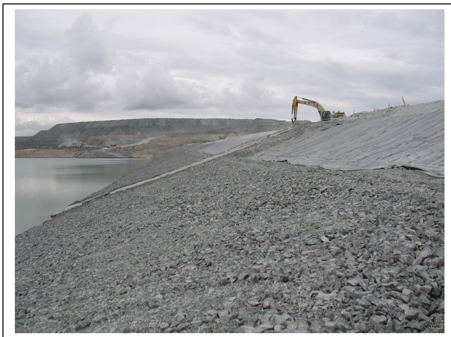
Photo #8 Central Dike, rockfill protection layer on LLPDE liner
