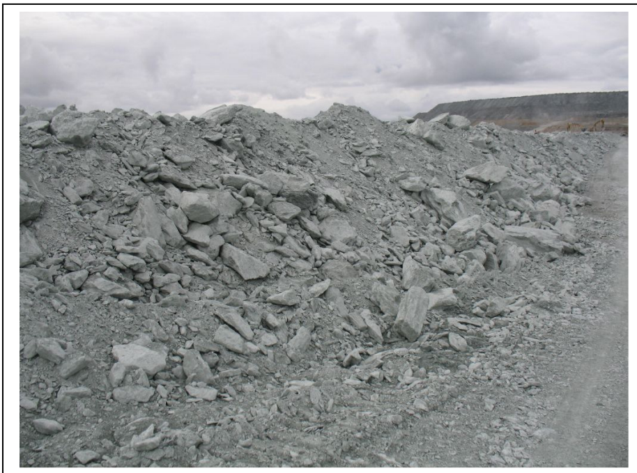
Photo #4 Central Dike, ultramafic soapstone rockfill
