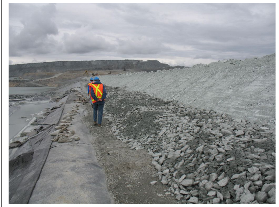
Photo #5 Central Dike, bedding and transition zones that confine the soapstone fill
