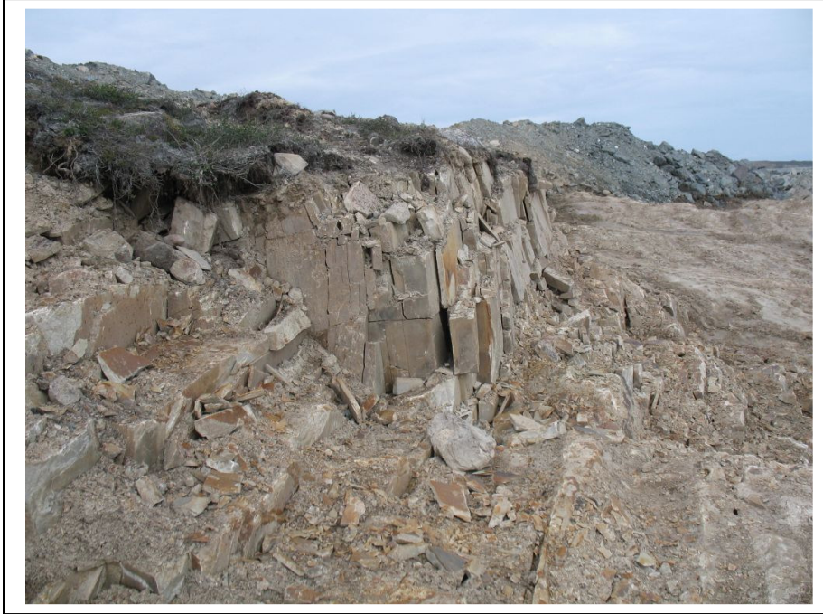
Photo #1 Saddle Dam 3, fractured rock of right abutment
