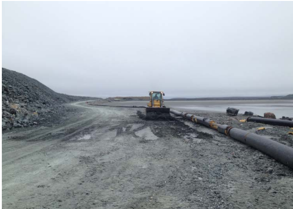
Photo 2 – Cleaning of the RF1 contaminated surface with the loader
