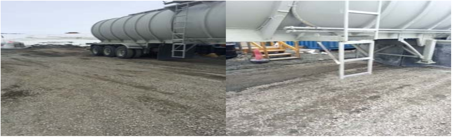
7. May 23rd – Area after new clean 0-20 mm granular material
