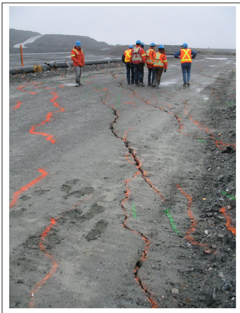
Photo no. 1 Cracking on Stormwater Dike Crest
