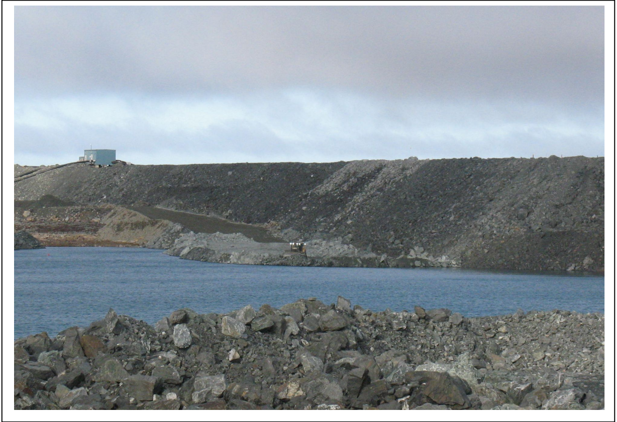
Photo no. 3 Construction of Stormwater Dike Toe Buttress
