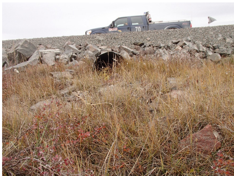
Photograph D1-22: PC-13 km 12+745
