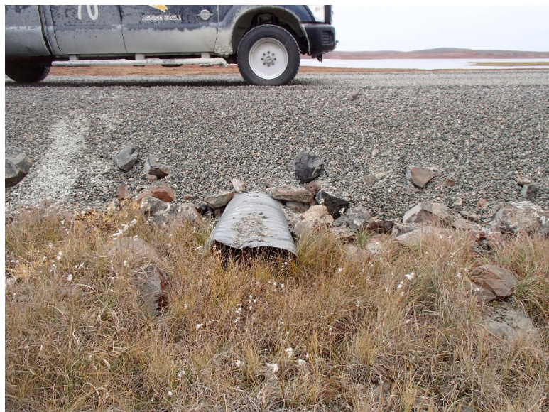
Photograph D1-21: PC-13 km 12+745
