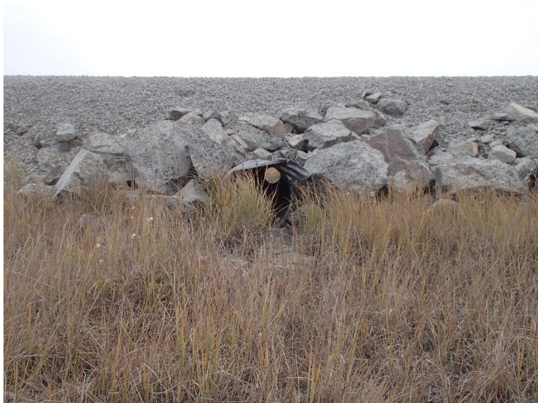
Photograph D1-33: PC-5 km 18+280
