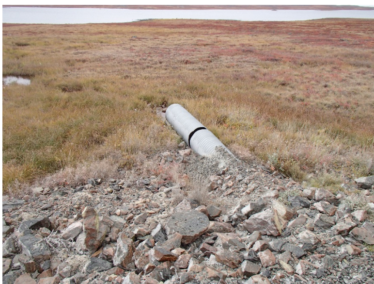
Photograph D1-26: PC-3 km 13+685
