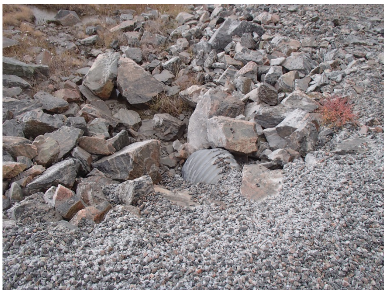
Photograph D1-30: PC-4 km 14+910
