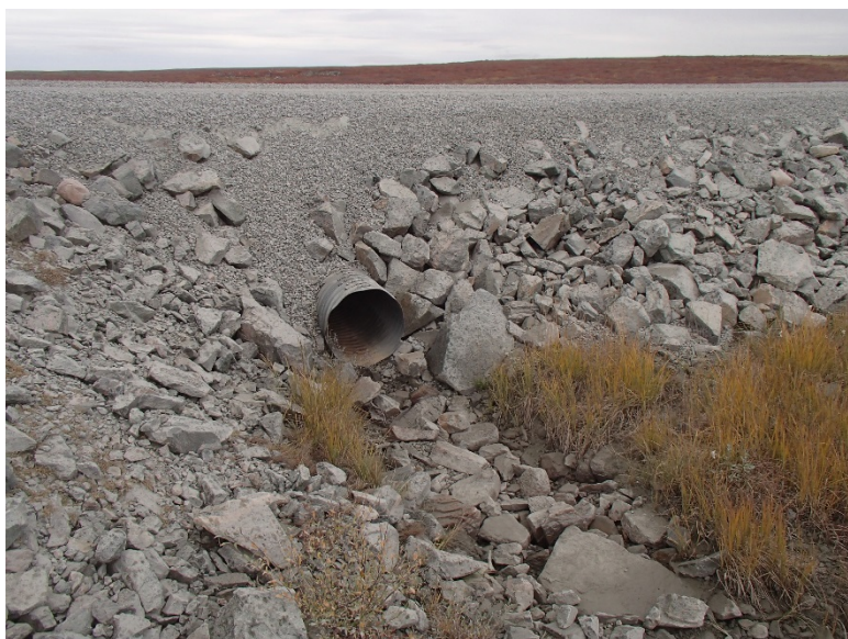
Photograph D1-34: PC-5 km 18+280
