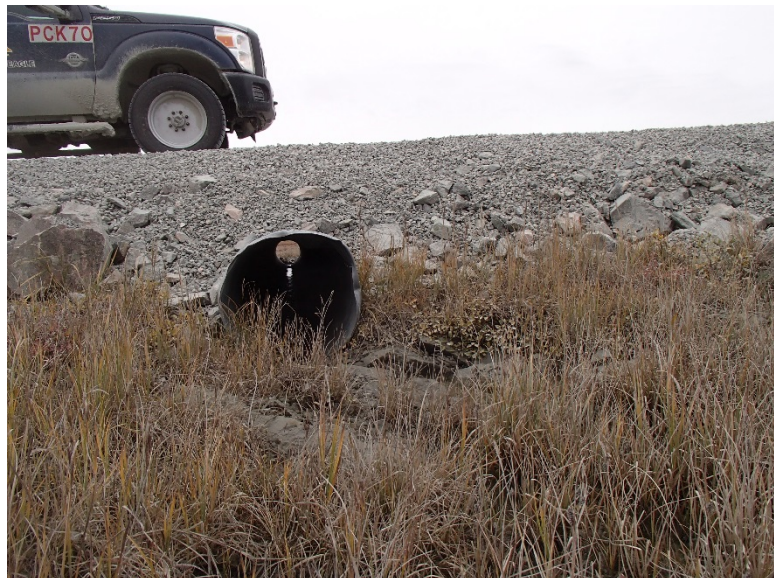
Photograph D1-39: PC-7 km 20+250
