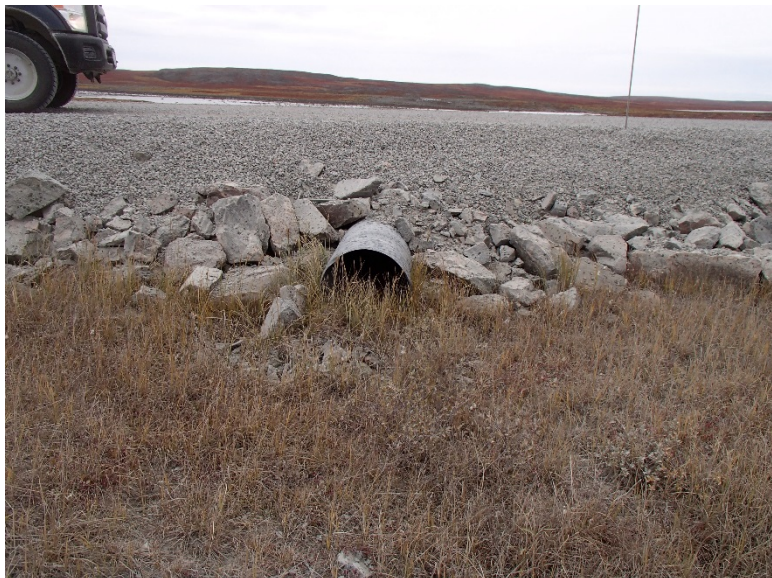
Photograph D1-35: PC-6 km 18+900
