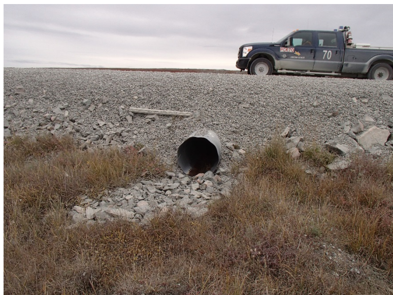
Photograph D1-40: PC-7 km 20+250
