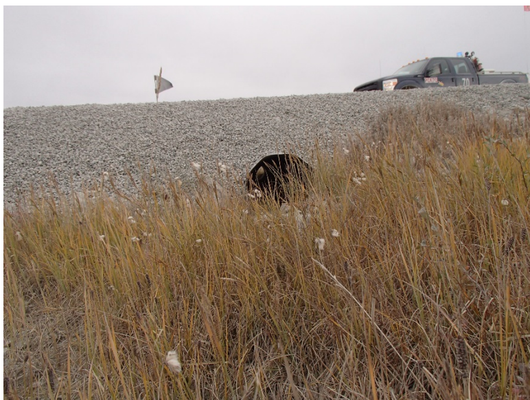
Photograph D1-36: PC-6 km 18+900
