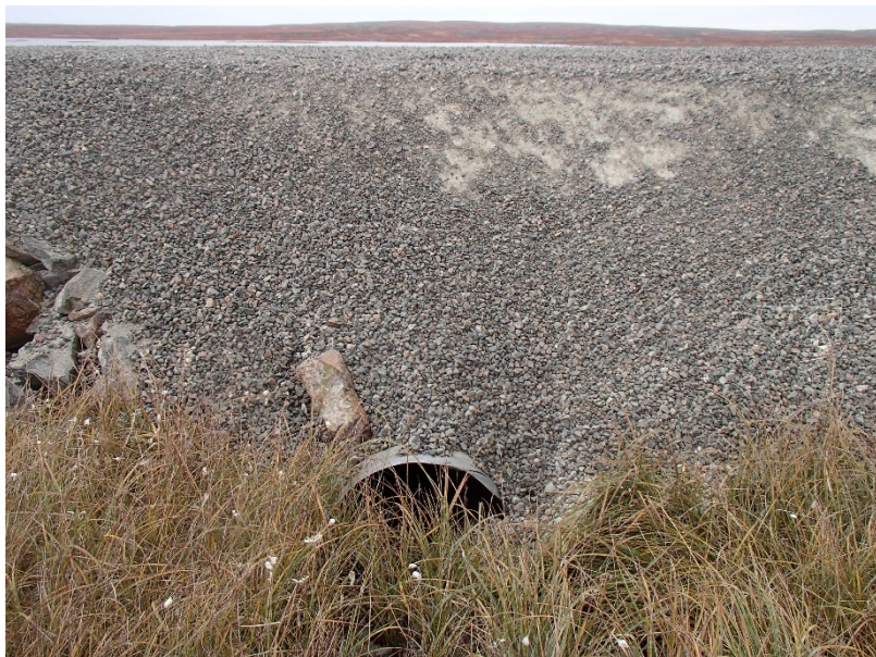
Photograph D1-25: PC-3 km 13+685
