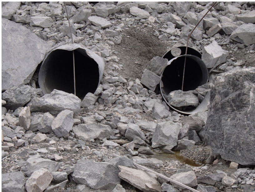
Photograph H1-5 Vault Road Culverts
