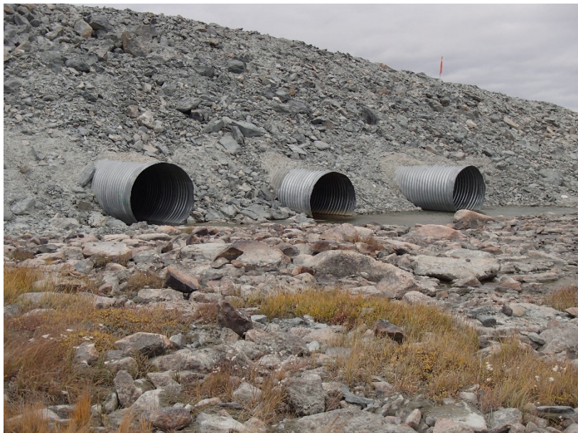
Photograph H1-1 Vault Road Culverts
