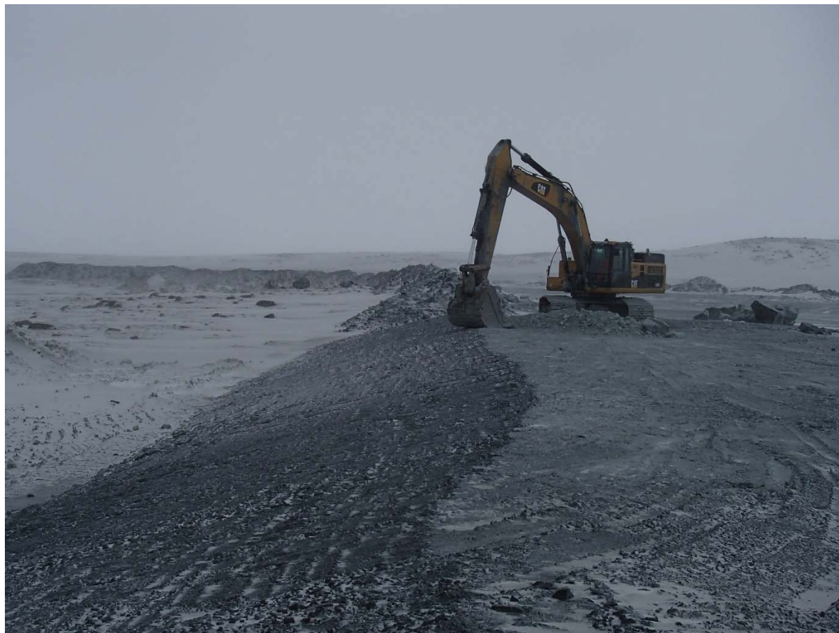
Photograph NCIS-019: From Sta. 2+100 m (approx.), looking SW. Profiling of the upstream slope (3H:1V) from El. 150 to 152 m with an excavator from Sta. 1+860 m to 1+678 m. The portion between Sta. 1+900 m and 1+800 m, where the structure is built on the natural ground, was not profiled.
