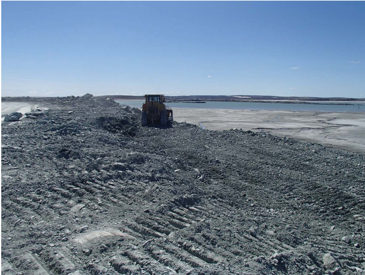
Photograph NCIS-057: From Sta. 3+010/-15 m (approx.), looking SW. Removing of UM rockfill material from the capping with a dozer to level the surface to El. 152 m from Sta. 2+980 m to 3+050 m (offset -30 to -20 m).
