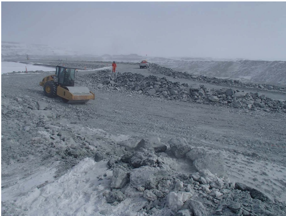
Photograph CD-1823: From Sta. 0+175/+8, looking NE. Compaction of the two 2 m lifts (approx.) of intermediate volcanic (IV) rockfill at El. 143 and at El. 145 m with a 10-tonne smooth-drum compactor with vibration (6 passes) from Sta. 40+720 m to 40+750 m (o.s. -10 to +10 m).
