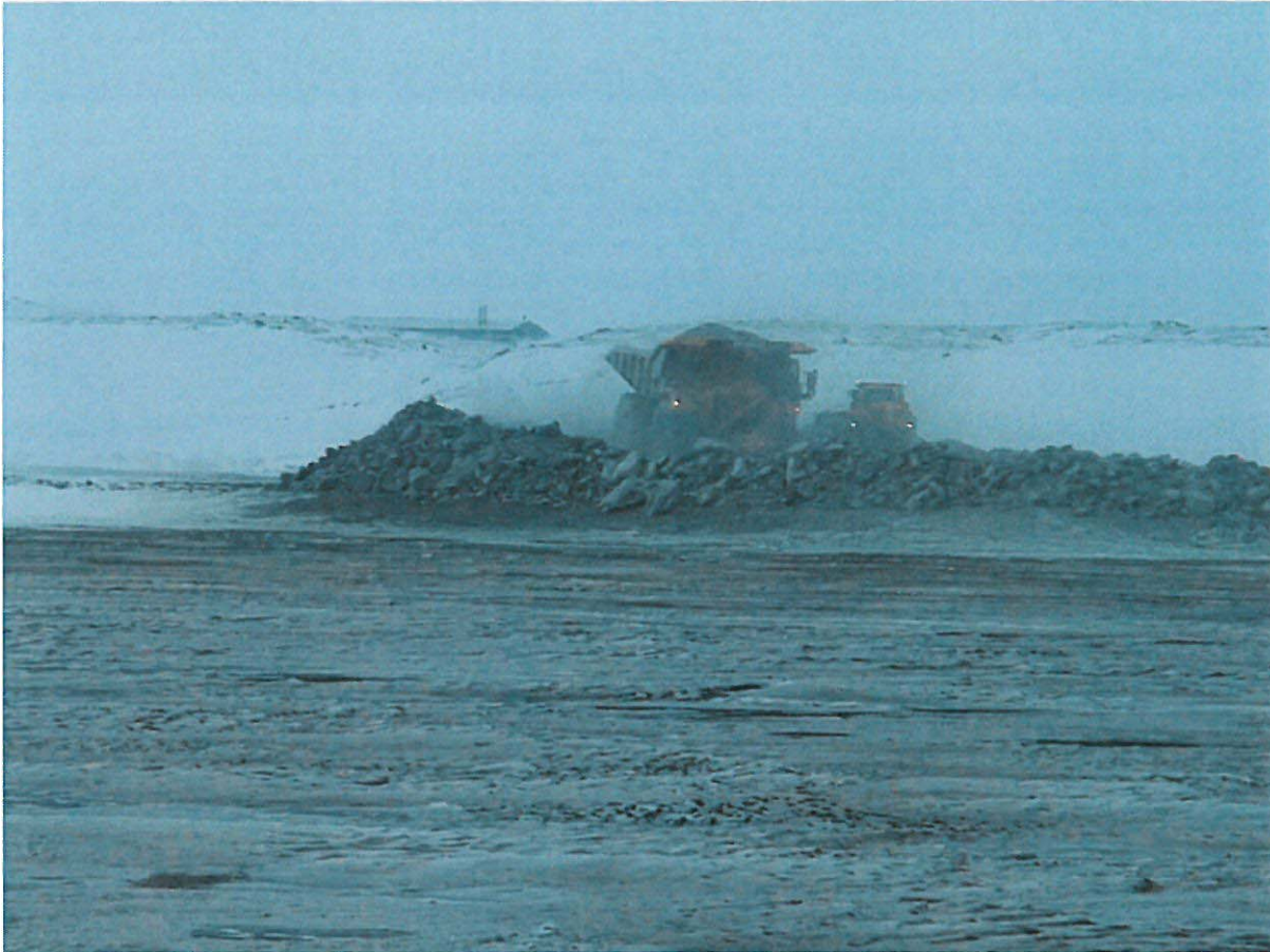
Photograph NCIS-008: Placement a 2 m thick (approx.) lift of UM rockfill from El. 150 m to El. 152 m (approx.) with a dozer. The material is of good quality and is well graded.
