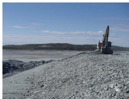
NCIS-102 (2018-07-20), looking W from Sta. 2+680/-21 m (approx.). Placement of a 0.5 m thick lift of coarse filter in the upstream slope from El. 152 m to 154 m with an excavator from Sta. 2+575 m to 2+710 m and from Sta. 2+411 m to 2+460 m.
