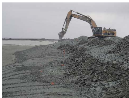
NCIS-079 (2018-07-05), looking SW from Sta. 1+280/-39 m. Placement of a 0.5 m thick lift of coarse filter in the upstream slope from El. 150 m to 152 m with an excavator from Sta. 1+300 m to 1+200 m.
