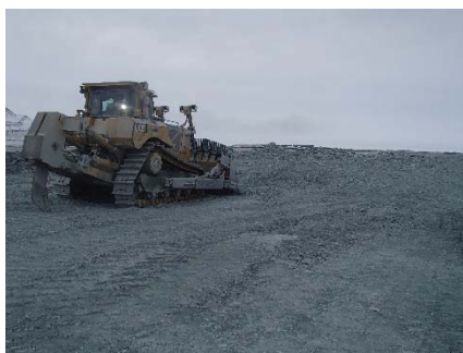
NCIS-020 (2018-05-27), looking S from Sta. 1+570 m. Placement a 2 m thick (approx.) lift of UM rockfill from El. 150 m to El. 152 m (approx.) with a dozer from Sta. 1+564 m to 1+535 m (o.s. unavailable).
