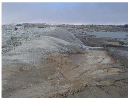
SD3-307 (2018-06-06), looking N from Sta. 20+800/-25 m. View of the liner bedding ready for geosynthetics installation.
