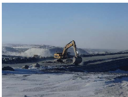
CD-1844 (2018-05-11), looking SE from Sta. 0+080/-49 m. Placement of a fourth 0.5 m thick lift of coarse filter from El. 144.5 m to 145 m with an excavator from Sta. 0+170 m to 40+730 m.
