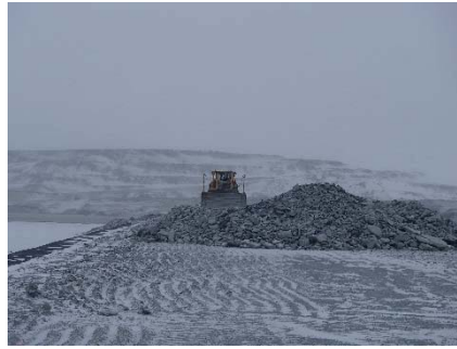
CD-1806 (2018-04-28), looking N from Sta. 0+800/-27 m. Placement a 2 m thick (approx.) lift of intermediate volcanic (IV) rockfill from El. 143 m to El. 145 m from approx. Sta. 0+710 to 0+760m (o.s. -28 to 3 m).
