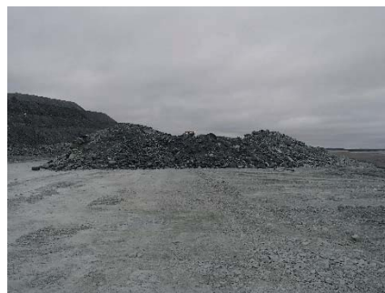
NCIS-090 (2018-07-13), looking SE from Sta. 2+440/-1 m (approx.). Placement of a 2 m thick (approx.) lift of UM rockfill from El. 152 m to El. 154 m (approx.) with a dozer from Sta. 2+455 m to 2+370 m (+4 m to -24 m).
