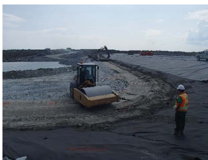
SD3-328 (2018-07-11), looking N from Sta. 20+820/-34 m. Compaction perpendicularly to the longitudinal axis of Saddle Dam 3 of the 0.5 m lift of low quality till (0-150 mm) at El. 142.5 m with a 10-tonne smooth-drum compactor without vibration (4 passes) from Sta. 20+615m to 20+635 m.
