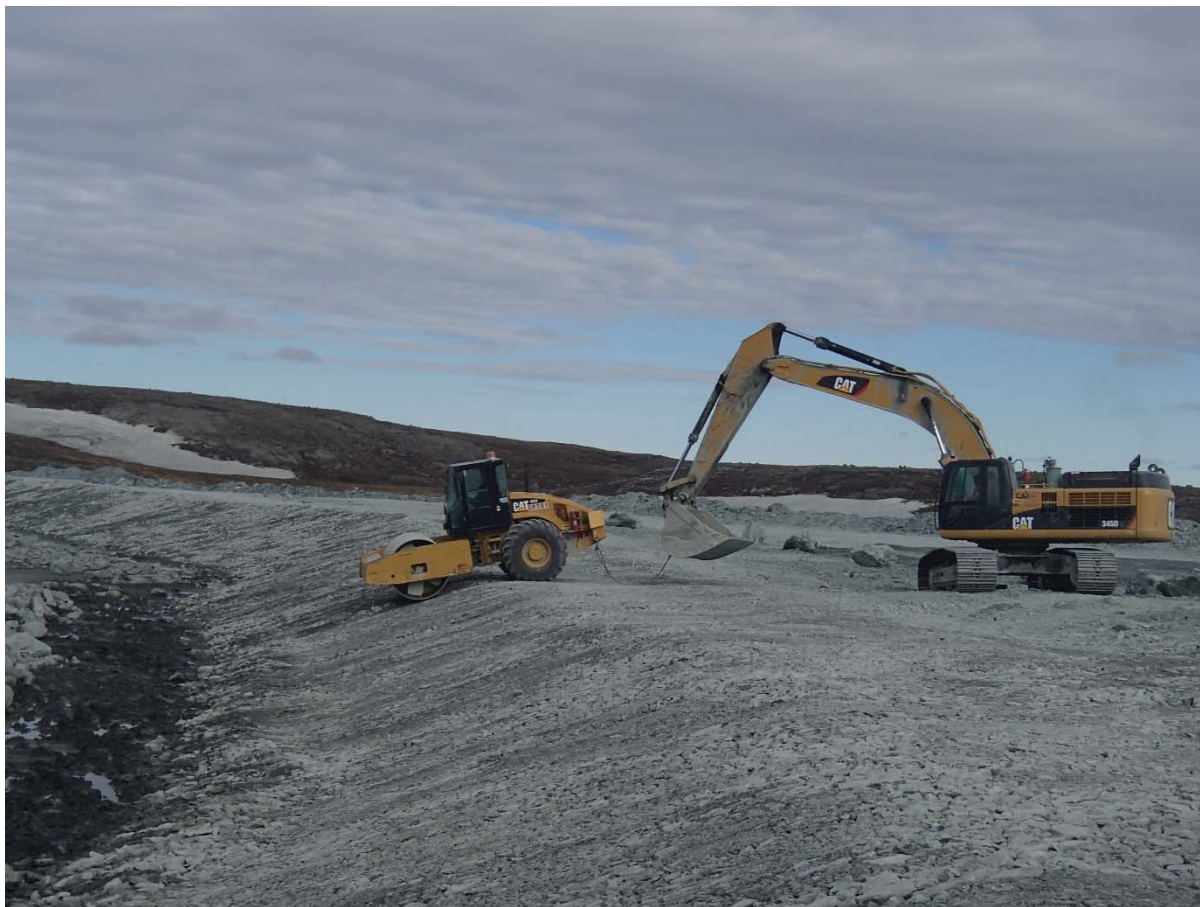
Photograph NCIS-037: From Sta. 1+550/-25 m (approx.), looking NW. Compaction of the 0.5 m lift (approx.) of coarse filter between El. 150 and 152 m with a 10-tonne smooth-drum compactor (4 passes) in the upstream slope from Sta. 2+450 to 1+805 m.
