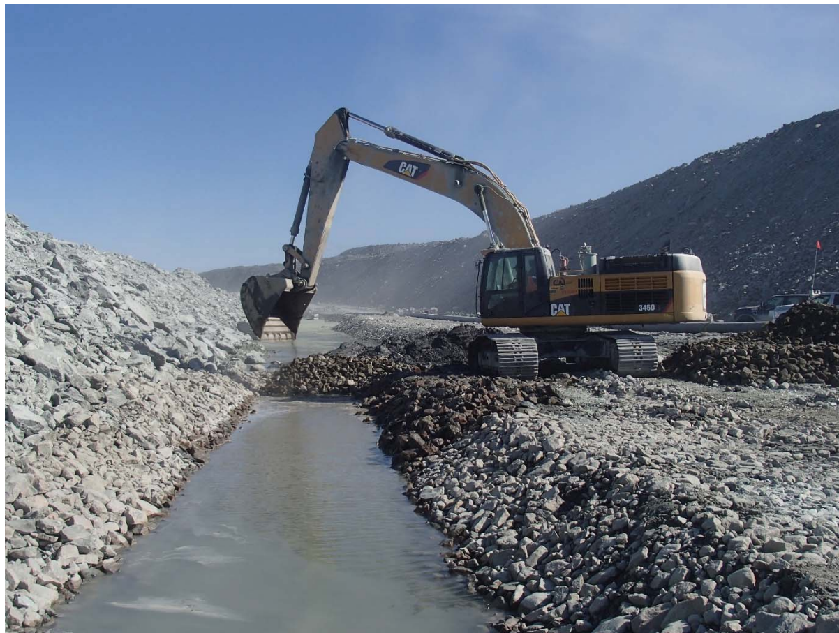
Photograph NCIS-125: From Sta. 3+050/+26 m (approx.), looking NE. Corrections to the north sump: removal of approx. 0.5 m of tailing and till sieving reject material on the bottom of the excavation. The erosion protection material was replaced.
