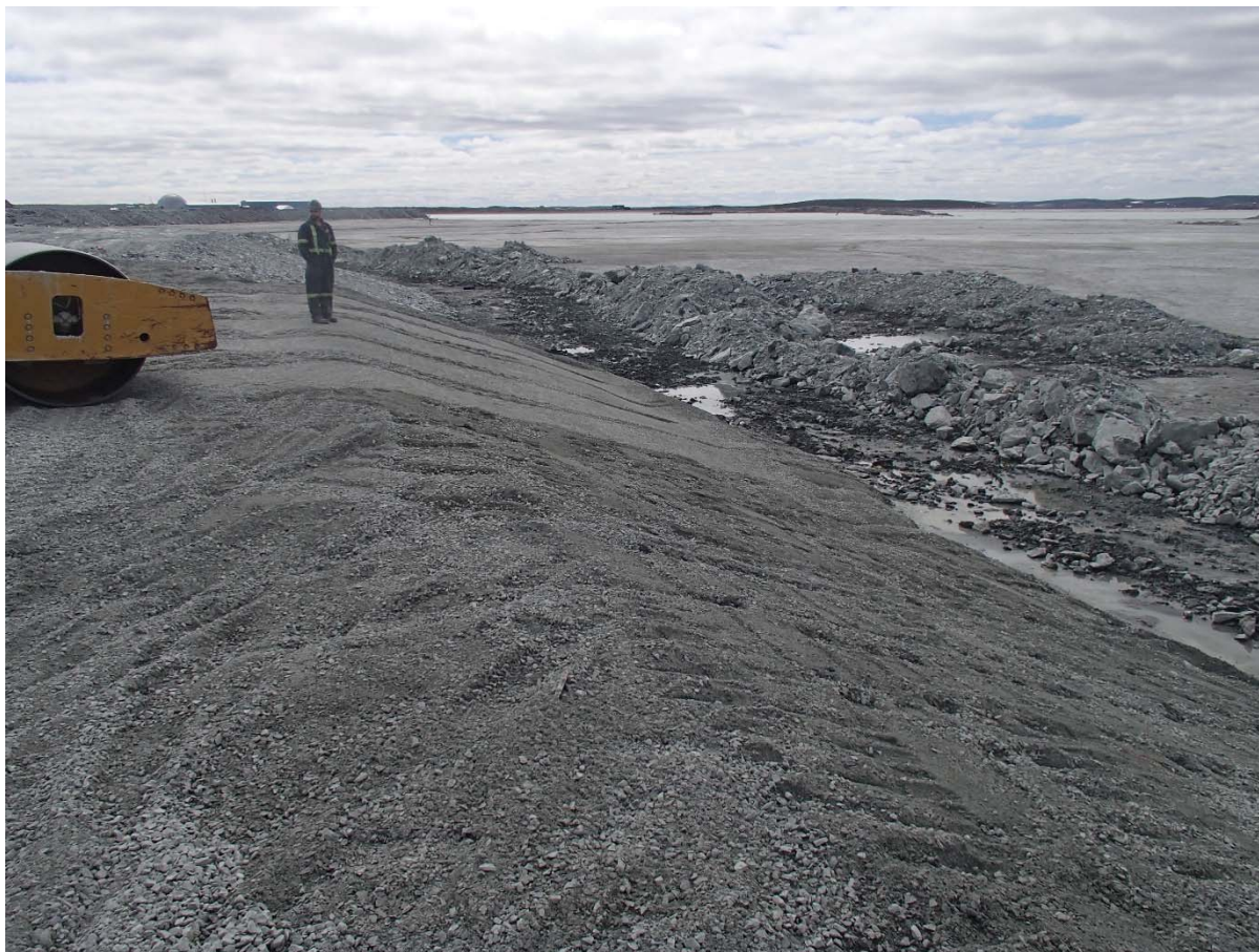
Photograph NCIS-038: From Sta. 2+510/-28 m (approx.), looking SE. Compaction of the 0.5 m lift (approx.) of fine filter between El. 150 and 152 m with a 10-tonne smooth-drum compactor (4 passes) in the upstream slope from Sta. 2+542 m to 2+475 m.
