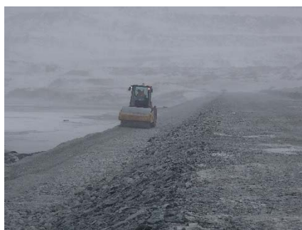
CD-1835 (2018-05-08), looking N from Sta. 0+830/-20 m. Compaction of the first 0.5 m lift (approx.) of fine and coarse filters material at El. 143.5 m with a 10-tonne smooth-drum compactor with vibration (6 passes) from Sta 0+490 m to 0+835 m.
