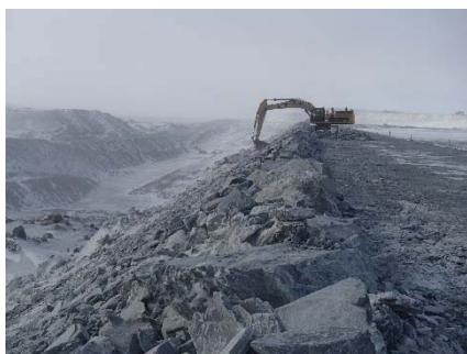
CD-1821 (2018-05-04), looking S from Sta. 0+175/+3 m. Profiling of the downstream slope (1.5H:1V) from El. 143 to 145 m with an excavator between Sta. 0+250 m and 0+330 m.
