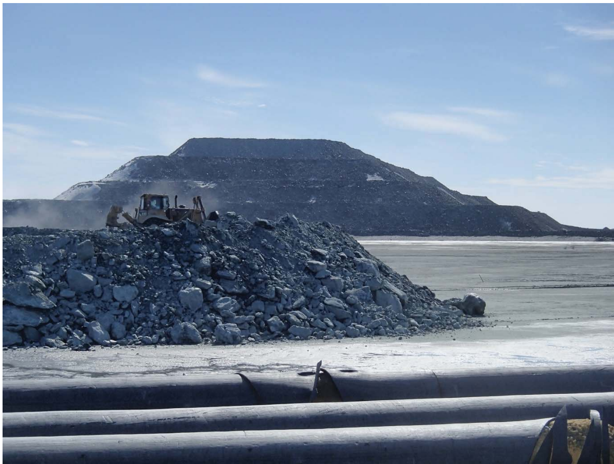
Photograph NCIS-027: From Sta. 1+360/+67 m, looking S. Placement of a 2 m thick (approx.) lift of UM rockfill from El. 150 m to El. 152 m (approx.) with a dozer from Sta. 1+365 m to 1+360 m (offset +9 m to -28 m).
