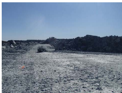
NCIS-100 (2018-07-20), looking E from Sta. 1+960/+10 m (approx.). Placement of a 2 m thick (approx.) lift of UM rockfill from El. 152 m to El. 154 m (approx.) with a dozer from Sta. 1+984 m to 1+947 m (+14 m to -26 m). The material is of good quality and is well graded.
