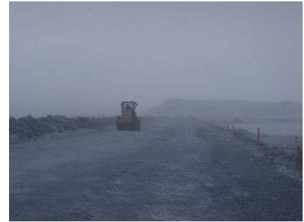
CD-1810 (2018-04-30), looking S from Sta. 0+335/-15 m. Compaction of the 2 m lift (approx.) of IV rockfill at El. 145 m with a 10-tonne smooth-drum compactor with vibration (6 passes) from Sta. 0+350 to 0+540 m (o.s. -19 to -7 m).
