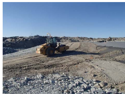
SD3-340 (2018-07-15), looking S from Sta. 20+750/-40 m. Compaction of the third 0.5 m thick lift of compacted sieved till on the upstream toe liner tie-in with an excavator from Sta. 20+760 m to 20+820 m.
