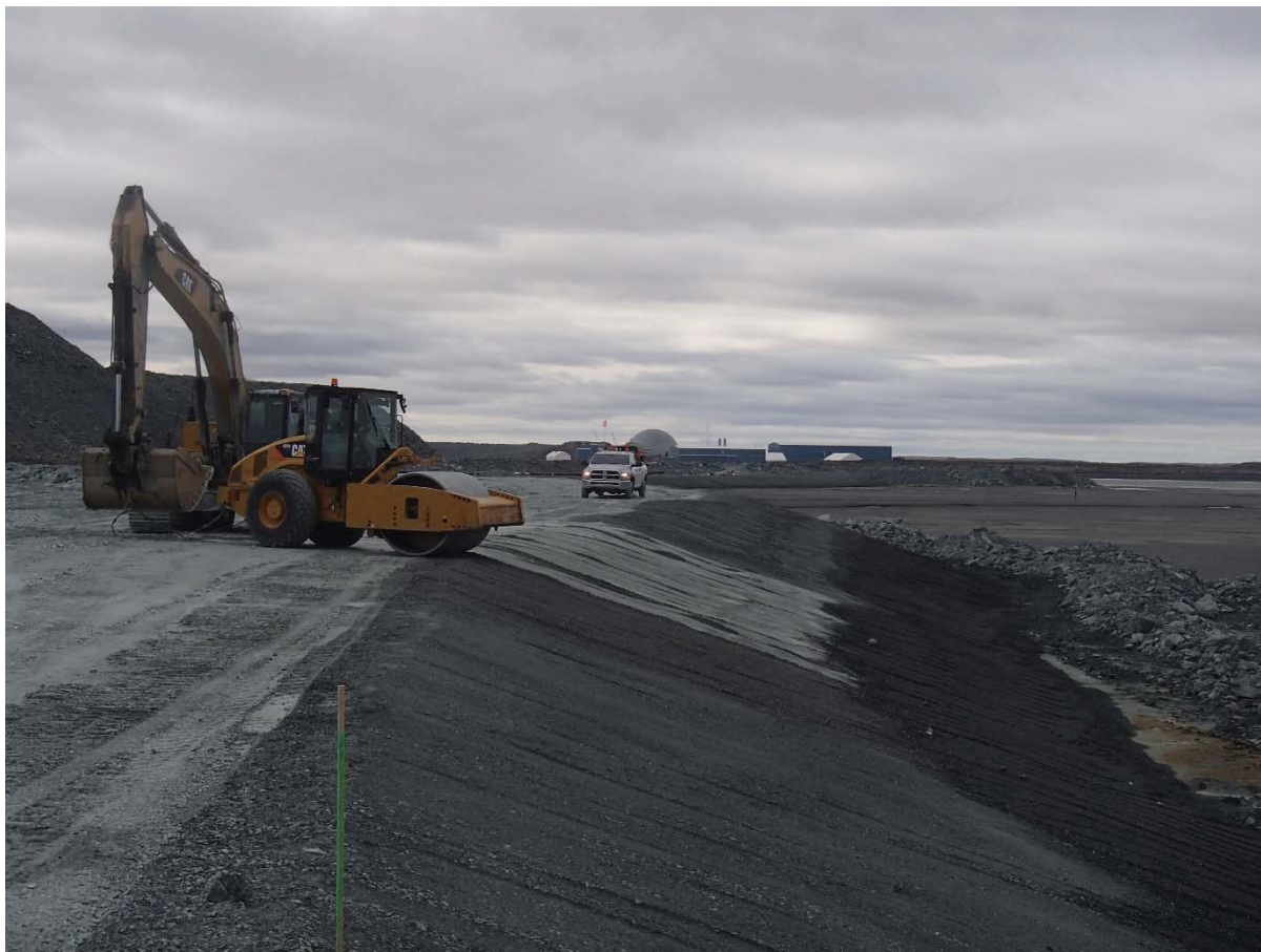
Photograph NCIS-129: From Sta. 2+450/-21 m (approx.), looking S. Compaction of the 0.5 m lift (approx.) of fine filter between El. 152 m and 154 m with a 10-tonne smooth-drum compactor with vibration (4 passes) in the upstream slope from Sta. 2+220 m to 1+940 m.
