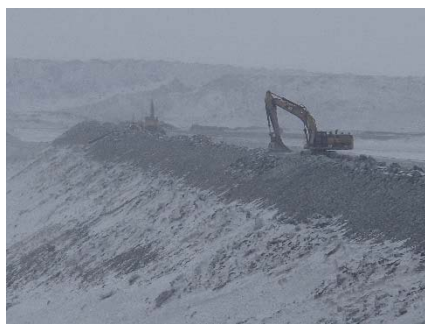
CD-1850 (2018-05-13), looking SW from Sta. 0+160/+20 m. Profiling of the downstream slope (1.5H:1V) from El. 143 to 145 m with an excavator between Sta. 0+440 m and 0+530 m and between Sta. 0+745 m and 0+835 m.
