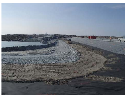
SD3-327 (2018-07-11), looking S from Sta. 20+610/-43 m. Compaction of the 0.5 m lift of low quality till (0-150 mm) at El. 142.5 m with a 10-tonne smooth-drum compactor with vibration (4 passes) from Sta. 20+610 m to 20+615 m and from Sta. 20+635 m to 20+760 m.
