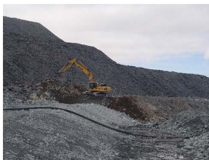
NCIS-046 (2018-06-26), looking SE from Sta. 2+680/-18 m. Removal of till material mixed with the UM rockfill of the capping (about 1 to 2 m thick along the slope) with an excavator from Sta. 2+760 m to 2+850 m (o.s. -35 to -17 m).
