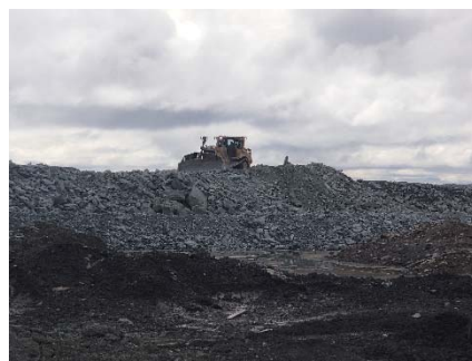
NCIS-084 (2018-07-08), looking E from Sta. 1+080/+47 m (approx.). Placement of a 2 m thick (approx.) lift of UM rockfill from El. 150 m to El. 152 m (approx.) with a dozer from Sta. 1+160 m to 1+130 m (-55 m to -102 m).
