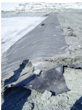
CD-1796 (2018-04-23), looking N from Sta. 0+650/-28 m. Damaged geomembrane near a deposition finger on Central Dike.
