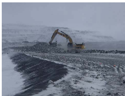
CD-1814 (2018-05-01), looking NE from Sta. 0+970/-10 m. Placement of intermediate volcanic (IV) rockfill around the instruments at approx. Sta. 0+830 m with the excavator.
