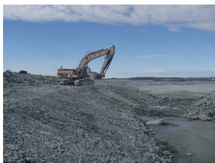
NCIS-067 (2018-07-01), looking N from Sta. 2+880/-26 m. Profiling of the upstream slope (3H:1V) from El. 150 to 152 m with an excavator from Sta. 2+860 m to 2+975 m.
