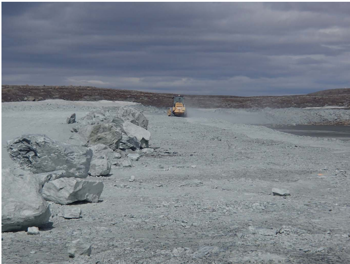
Photograph NCIS-032: From Sta. 1+400/-24 m (approx.), looking N. Compaction of the 2 m lift (approx.) of ultramafic (UM) rockfill at El. 152 m with a 10-tonne smooth-drum compactor with vibration (6 passes) between the haul truck traffic lane and the upstream slope from Sta. 1+660 to 1+380 m (offset -45 to -24 m).
