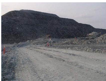
NCIS-086 (2018-07-10), looking E from Sta. 2+750/+14 m (approx.). Placement of a 2 m thick (approx.) lift of UM rockfill from El. 152 m to El. 154 m (approx.) with a dozer from Sta. 2+780 m to 2+760 m (-60 m to -44 m).
