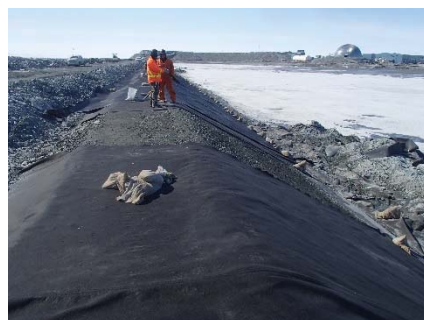
CD-1882 (2018-06-02), looking S from Sta. 0+510/-25 m. View of the emplacement of the geotextile panel with a horizontal weld in the slope at Sta. 0+520 following its removal.
