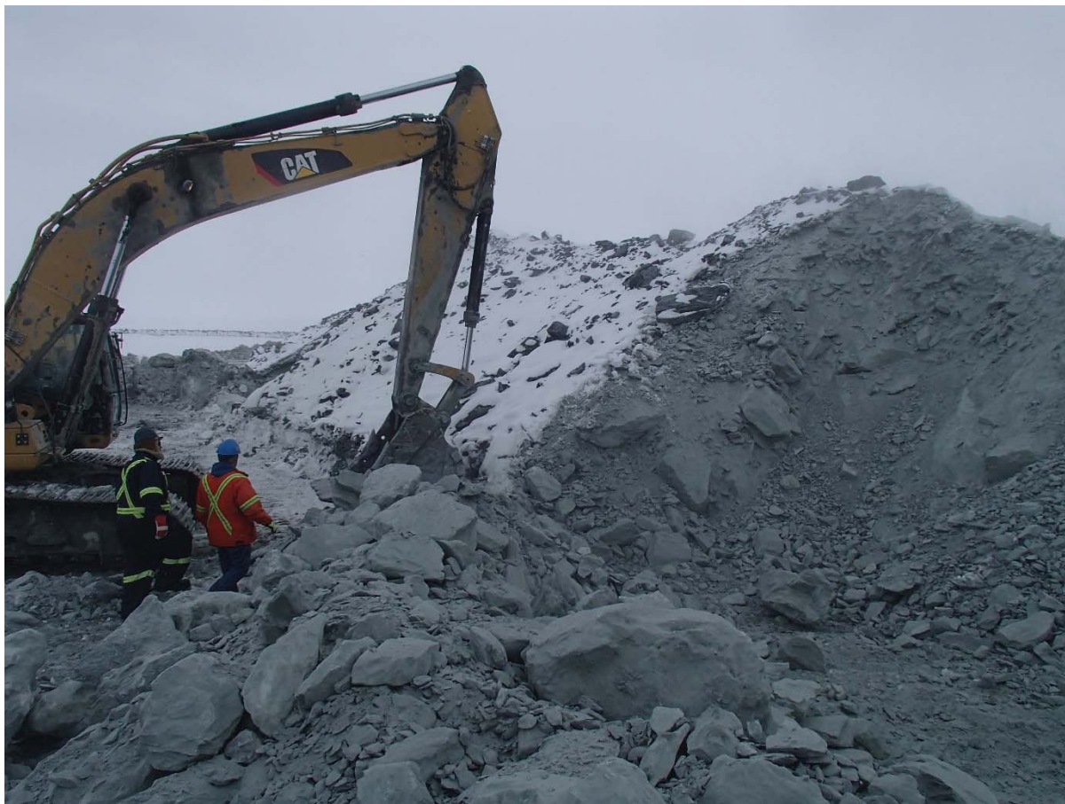
Photograph NCIS-003: Excavation of the snow-rich upstream toe material on an average width of 2 to 3 m with an excavator.
