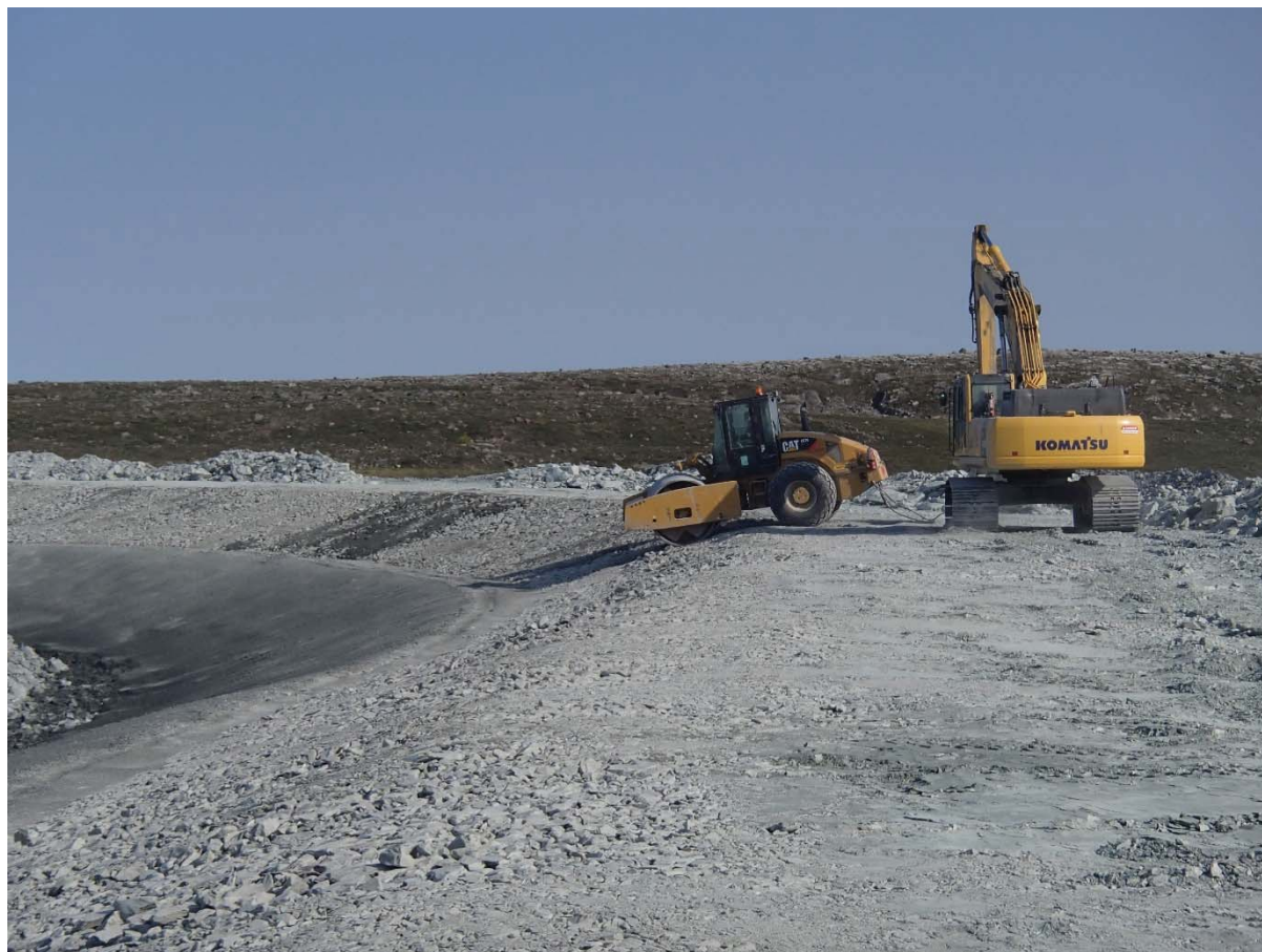
Photograph NCIS-110: From Sta. 2+320/-22 m (approx.), looking N. Compaction of the 0.5 m lift (approx.) of coarse filter between El. 152 m and 154 m with a 10-tonne smooth-drum compactor with vibration (4 passes) in the upstream slope from Sta. 2+293 m to 2+080 m.
