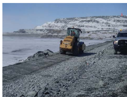
CD-1840 (2018-05-09), looking NW from Sta. 0+575/-15 m. Compaction of the second 0.5 m lift (approx.) of fine and coarse filters material at El. 144 m with a 10-tonne smooth-drum compactor with vibration (4 passes) from Sta 0+500 m to 40+730 m.
