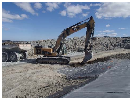
SD3-332 (2018-07-12), looking SE from Sta. 20+775/-23 m. Placement of a first 0.5 m thick lift of compacted sieved till over the LLDPE geomembrane on the upstream toe liner tie-in with an excavator from Sta. 20+775 m to 20+800 m.
