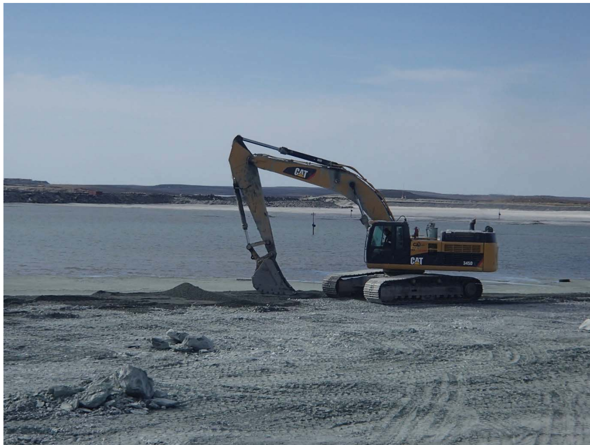
Photograph NCIS-068: From Sta. 1+150/-62 m (approx.), looking S. Placement of a 0.5 m thick lift of fine filter over the coarse filter in the upstream slope from El. 148 m to 150 m with an excavator from Sta. 1+180 m to 1+100 m.
