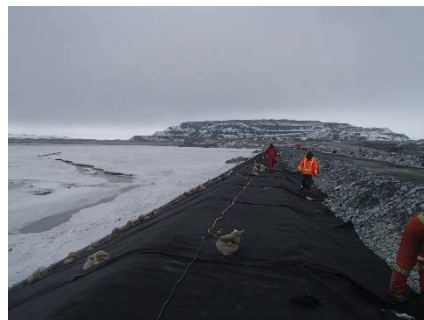
CD-1873 (2018-05-29), looking N from Sta. 0+760/-26 m. Installation of the geotextile on the upstream slope 2H:1V between El. 143 m and 145 m from Sta. 0+760 m to 0+740 m.
