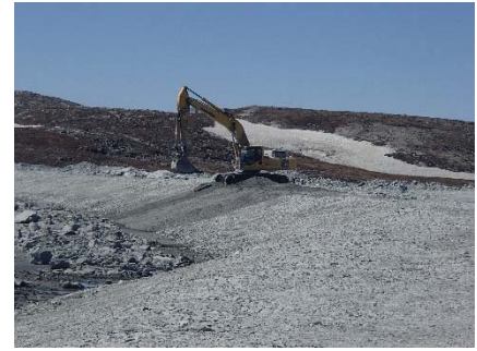
NCIS-039 (2018-06-23), looking W from Sta. 2+200/-24 m. Placement of a 0.5 m thick lift of fine filter over the coarse filter in the upstream slope from El. 150 m to 152 m with an excavator from Sta. 2+460 m to 2+475 m and from Sta. 2+065 m to 1+980 m.
