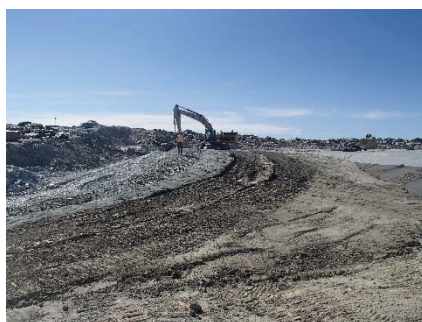
SD3-336 (2018-07-14), looking S from Sta. 20+755/-48 m. Placement of a fourth 0.5 m thick lifts of fine filter, coarse filter and fine rockfill on the upstream slope of the upstream toe liner tie-in with an excavator from Sta. 20+770 to 20+800 m.
