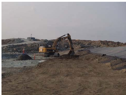
SD3-324 (2018-07-10), looking S from Sta. 20+680/-39 m. Placement of a 0.5 m thick lift of low quality till (0-150 mm) from El. 142 m to 142.5 m from Sta. 20+715 m to 20+760 m.
