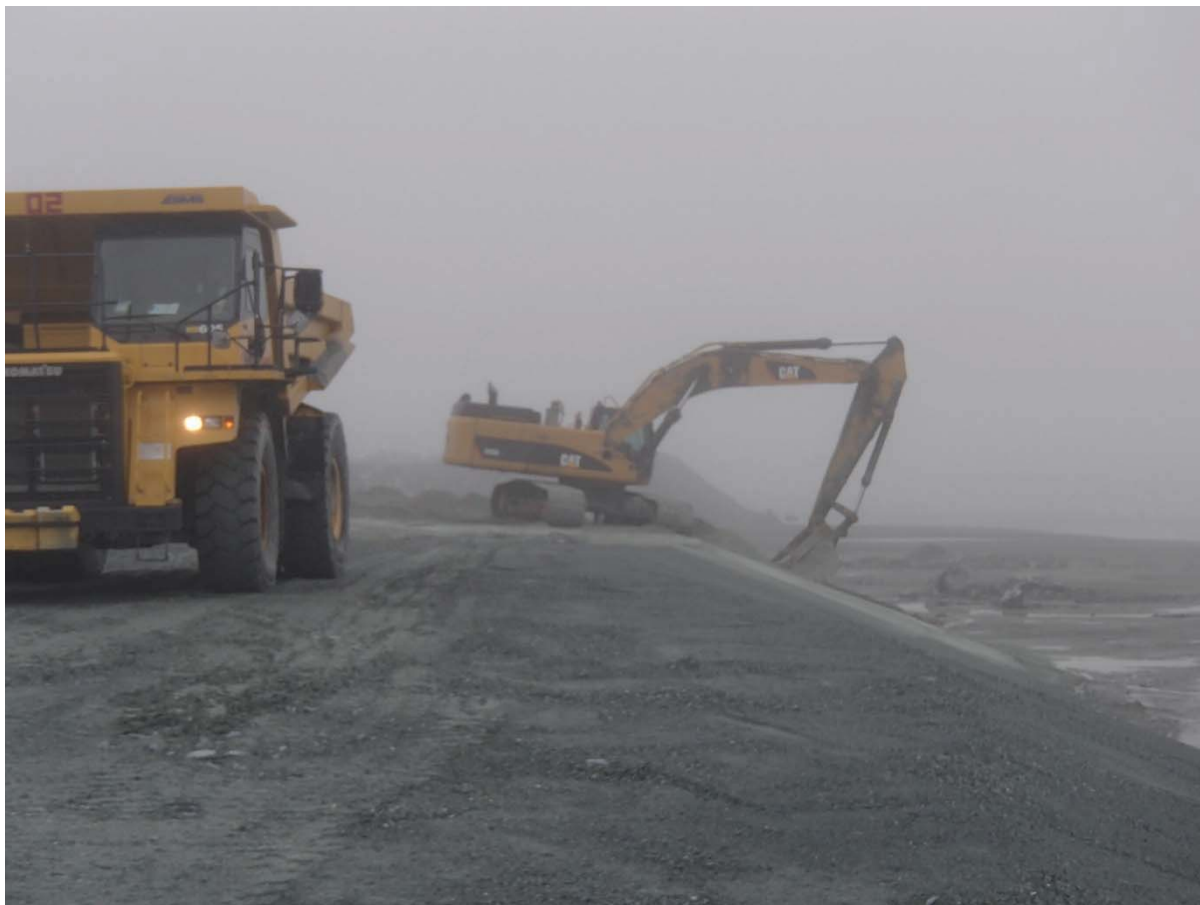
Photograph NCIS-082: From Sta 3+060/-33 m (approx.), looking S. Placement of a 0.5 m thick lift of fine filter over the coarse filter in the upstream slope from El. 150 m to 152 m with an excavator from Sta. 3+120 m to 3+160 m.
