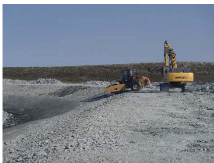
NCIS-110 (2018-07-23), looking N from Sta. 2+320/-22 m (approx.). Compaction of the 0.5 m lift (approx.) of coarse filter between El. 152 m and 154 m with a 10-tonne smooth-drum compactor with vibration (4 passes) in the upstream slope from Sta. 2+293 m to 2+080 m.
