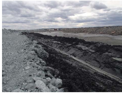
NCIS-137 (2018-07-31), looking SW from Sta. 1+380/+14 m (approx.). Excavation of a 0.8 m (approx.) deep, 1 m wide shallow ditch in the tailings with an excavator from Sta. 1+300 m to 1+200 m.
