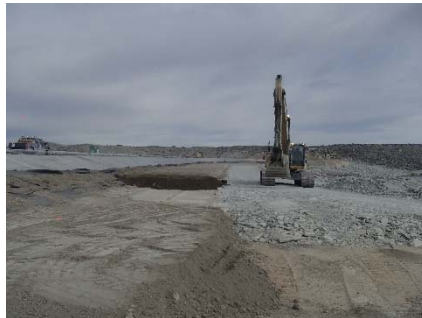
SD3-345 (2018-07-17), looking NW from Sta. 20+760/-42 m. Placement of a fourth 0.5 m thick lift of low quality till (0-150 mm) from El. 143 m to 143.5 m from Sta. 20+619 m to 20+777 m.
