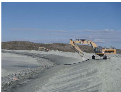
NCIS-113 (2018-07-24), looking SW from Sta. 2+220/-26 m (approx.). Profiling of the upstream slope (3H:1V) from El. 152 to 154 m with an excavator from Sta. 2+000 m to 1+185 m and placement of a 0.5 m thick lift of fine filter in the upstream slope from El. 152 m to 154 m with an excavator from Sta. 2+300 m to 2+090 m.
