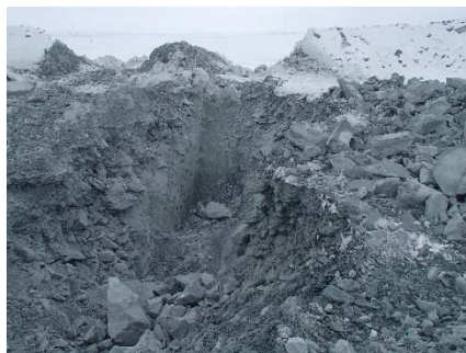
NCIS-001 (2018-05-19). View of a test pit in the UM rockfill lift at El. 152 m: a thick layer of snow (2 m) underlies the rockfill.
