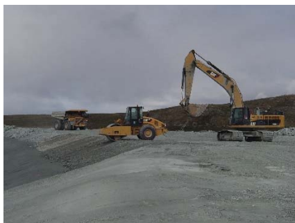
NCIS-131 (2018-07-29), looking W from Sta. 1+940/-20 m (approx.). Compaction of the 0.5 m lift (approx.) of coarse filter between El. 152 m and 154 m with a 10-tonne smooth-drum compactor with vibration (4 passes) in the upstream slope from Sta. 1+890 m to 1+826 m.
