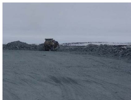
NCIS-021 (2018-05-28), looking S from Sta. 1+550 m. Placement a 2 m thick (approx.) lift of UM rockfill from El. 150 m to El. 152 m (approx.) with a dozer from Sta. 1+535 m to 1+500 m (o.s. unavailable).
