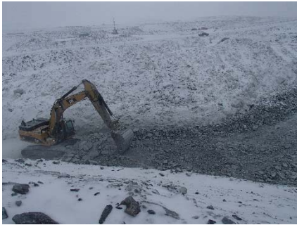
CD-1808 (2018-04-28), looking E from Sta. 40+790/-14 m. Placement a 2 m thick (approx.) lift of intermediate volcanic (IV) rockfill from approx. Sta. 40+780 to 40+805 m (o.s. -6 to 9 m).
