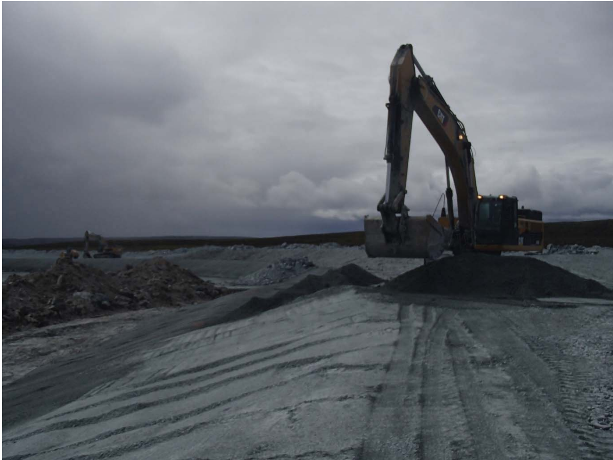
Photograph NCIS-135: From Sta. 1+860/-12 m (approx.), looking SW. Placement of a 0.5 m thick lift of fine filter in the upstream slope from El. 152 m to 154 m with an excavator from Sta. 1+830 m to 1+700 m.
