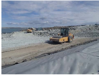
SD3-351 (2018-07-18), looking SE from Sta. 20+740/-24 m. Compaction of the m lift of low quality till (0-150 mm) at El. 143.5 m with a 10-tonne smooth-drum compactor with vibration (4 passes) from Sta. 20+619 m to 20+777 m.
