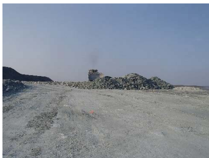
NCIS-089 (2018-07-12), looking S from Sta. 2+525/+4 m (approx.). Placement of a 2 m thick (approx.) lift of UM rockfill from El. 152 m to El. 154 m (approx.) with a dozer from Sta. 2+605 m to 2+455 m (+3 m to -23 m).
