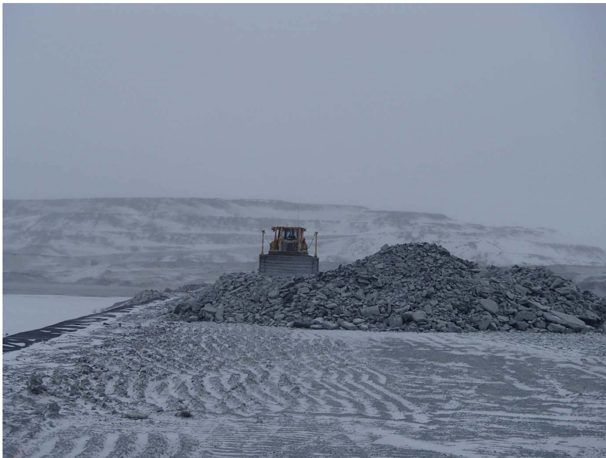
Photograph CD-1806: From Sta. 0+800/-27 m looking N. Placement a 2 m thick (approx.) lift of intermediate volcanic (IV) rockfill from El. 143 m to El. 145 m from approx. Sta. 0+710 to 0+760 m (o.s. -28 to 3 m).
