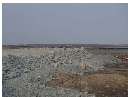
NCIS-085 (2018-07-09), looking SW from Sta. 1+150/-67 m (approx.). Placement of a 2 m thick (approx.) lift of UM rockfill from El. 150 m to El. 152 m (approx.) with a dozer from Sta. 1+130 m to 1+100 m (-55 m to -78 m).
