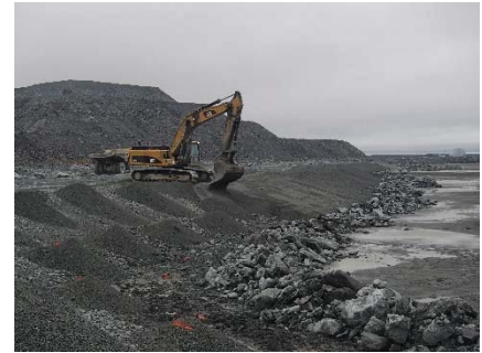
NCIS-042 (2018-06-25), looking SE from Sta. 2+210/-27 m. Placement of a 0.5 m thick lift of fine filter over the coarse filter in the upstream slope from El. 150 m to 152 m with an excavator from Sta. 2+305 m to 2+040 m.
