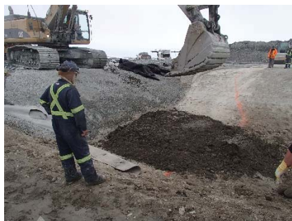
SD3-312 (2018-06-08), looking W from Sta. 20+610/-48 m. Placement of a 0.15 m thick lift of compacted sieved till from Sta. 20+596.4 m to 20+601.6 m (o.s. -42.6 to -46.3 m) to fill the depression in the compacted sieved till layer.
