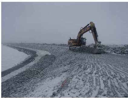
CD-1826 (2018-05-06), looking NE from Sta. 40+770/-27 m. Placement of a 0.5 m thick lift of coarse filter from El. 143 m to 143.5 m with an excavator from Sta. 40+730 m to 0+775 m.
