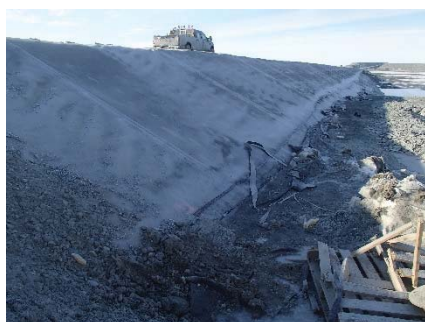
CD-1892 (2018-06-06), looking S from Sta. 0+155/-32 m. View of the liner panel 933 overlapping the underlying liner that has been cut at around Sta. 0+160 m to drain the water.
