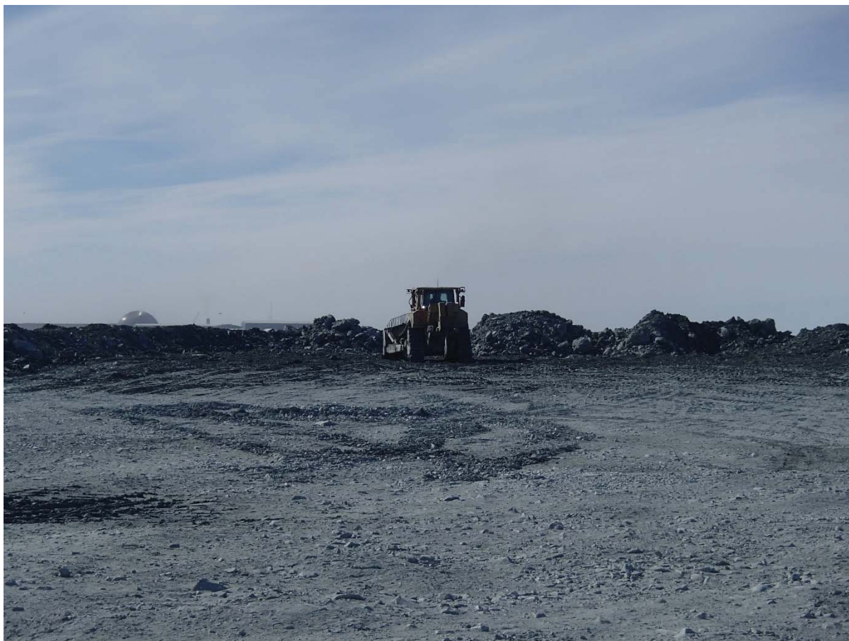
Photograph NCIS-026: From Sta. 1+440/+2 m, looking S. Placement of a 2 m thick (approx.) lift of UM rockfill from El. 150 m to El. 152 m (approx.) with a dozer from Sta. 1+390 m to 1+365 m (offset +10 m to -29 m).
