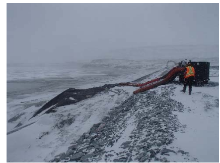
CD-1828 (2018-05-06), looking N from Sta. 0+410/-22 m. Defrosting of the deposition point finger materials with two Frost Fighters at Sta. 0+390 m.
