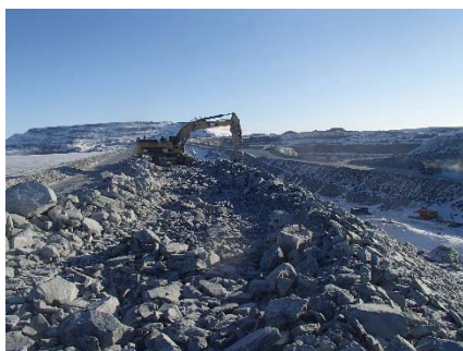
CD-1854 (2018-05-15), looking N from Sta. 0+860/-13 m. Profiling of the downstream slope (1.5H:1V) from El. 143 to 145 m with an excavator between Sta. 0+940 m and 0+990 m.
