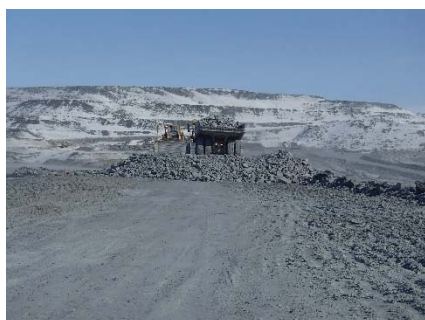
CD-1802 (2018-04-27), looking N from Sta. 0+770/-16 m. Placement a 2 m thick (approx.) lift of intermediate volcanic (IV) rockfill from El. 143 m to El. 145 m from approx. Sta. 0+625 to 0+710 m (o.s. -28 to -18 m).
