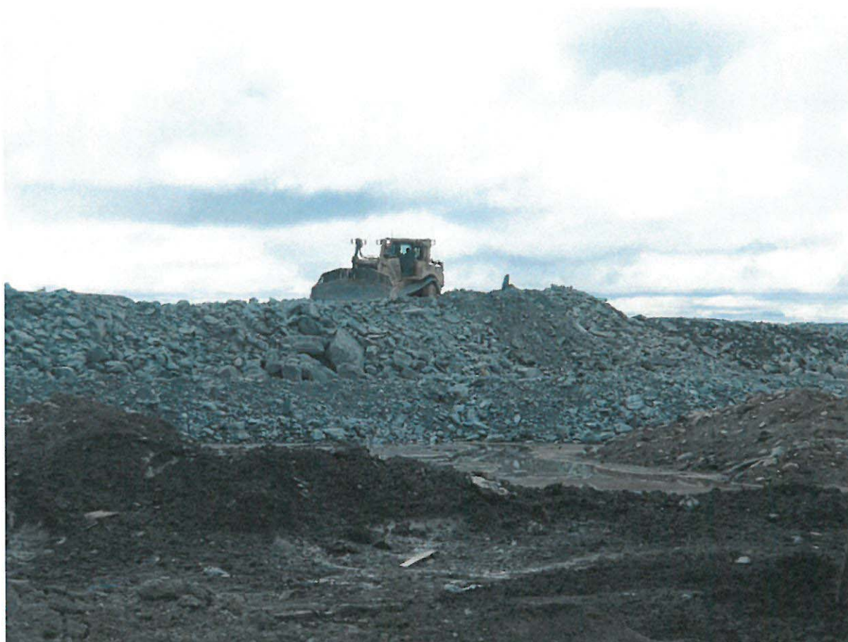
Photograph NCIS-084: From Sta 1+080/+47 m (approx.), looking E. Placement of a 2 m thick (approx.) lift of UM rockfill from El. 150 m to El. 152 m (approx.) with a dozer from Sta. 1+160 m to 1+130 m (-55 m to -102 m).
