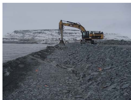
CD-1837 (2018-05-08), looking N from Sta. 0+940/-25 m. Placement of a second 0.5 m thick lift of coarse filter from El. 143.5 m to 144 m with an excavator from Sta. 0+290 m to 0+500 and from Sta. 0+835 m to 0+930 m.
