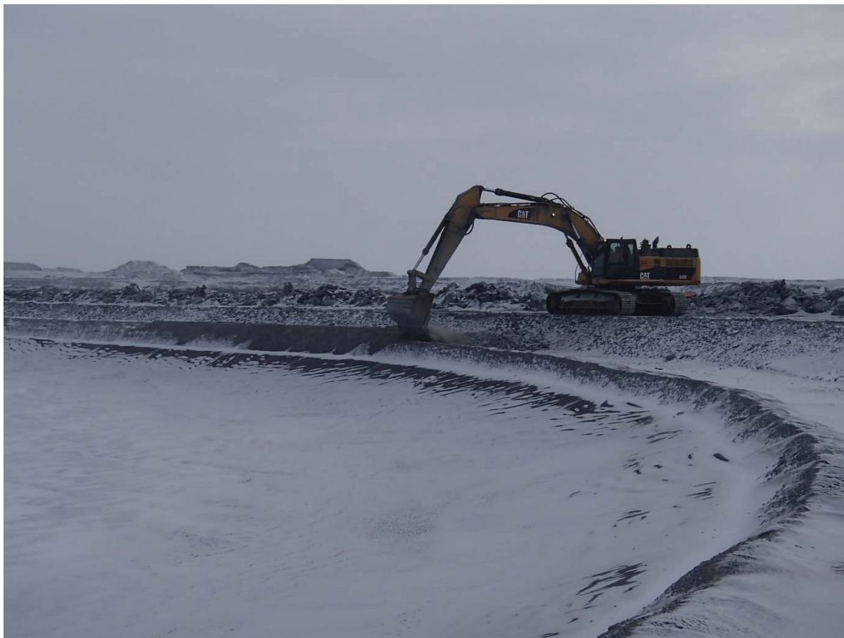
Photograph CD-1838: From Sta. 40+750/-31 m, looking NE. Placement of a second 0.5 m thick lift of fine filter from El. 143.5 m to 144 m upstream of the coarse filter with an excavator from Sta. 0+500 m to 0+835 m and from Sta. 0+930 to 40+730 m.
