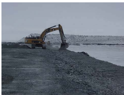
CD-1842 (2018-05-10), looking S from Sta. 0+380/-16 m. Placement of a third 0.5 m thick lift of fine filter from El. 143.5 m to 144 m upstream of the coarse filter with an excavator from Sta. 0+335 m to 0+940 m.
