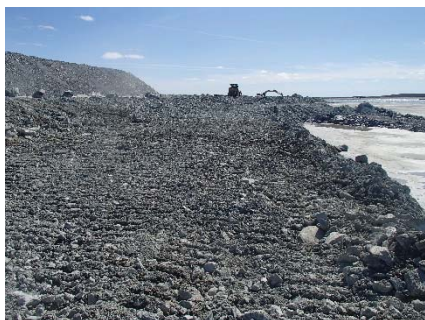
NCIS-053 (2018-06-27), looking S from Sta. 2+840/-37 m. Removing of UM rockfill material from the capping with a dozer to level the surface to El. 152 m from Sta. 2+850 m to 2+980 m (o.s. -38 to -24 m).
