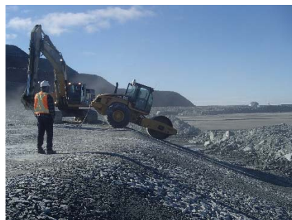
NCIS-054 (2018-06-28), looking SE from Sta. 2+580/-31 m. Compaction of the 0.5 m lift (approx.) of coarse filter between El. 150 and 152 m with a 10-tonne smooth-drum compactor with vibration (4 passes) in the upstream slope from Sta. 2+560 m to 2+815 m.
