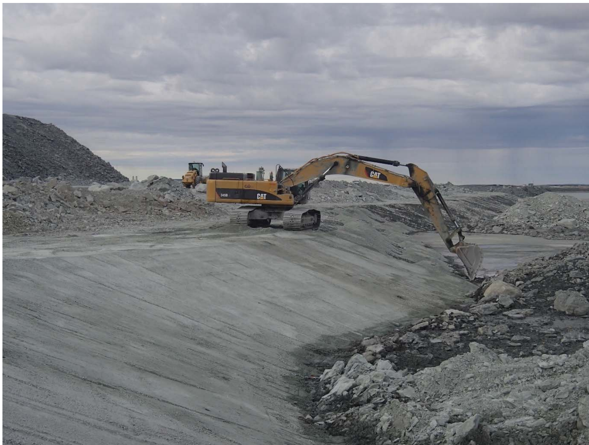
Photograph NCIS-078: From Sta. 2+760/-39 m (approx.), looking S. Placement of a 0.5 m thick lift of fine filter over the coarse filter in the upstream slope from El. 150 m to 152 m with an excavator from Sta. 2+800 m to 2+980 m.
