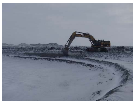
CD-1838 (2018-05-09), looking NE from Sta. 40+750/-31 m. Placement of a second 0.5 m thick lift of fine filter from El. 143.5 m to 144 m upstream of the coarse filter with an excavator from Sta. 0+500 m to 0+835 m and from 0+930 to 40+730 m.
