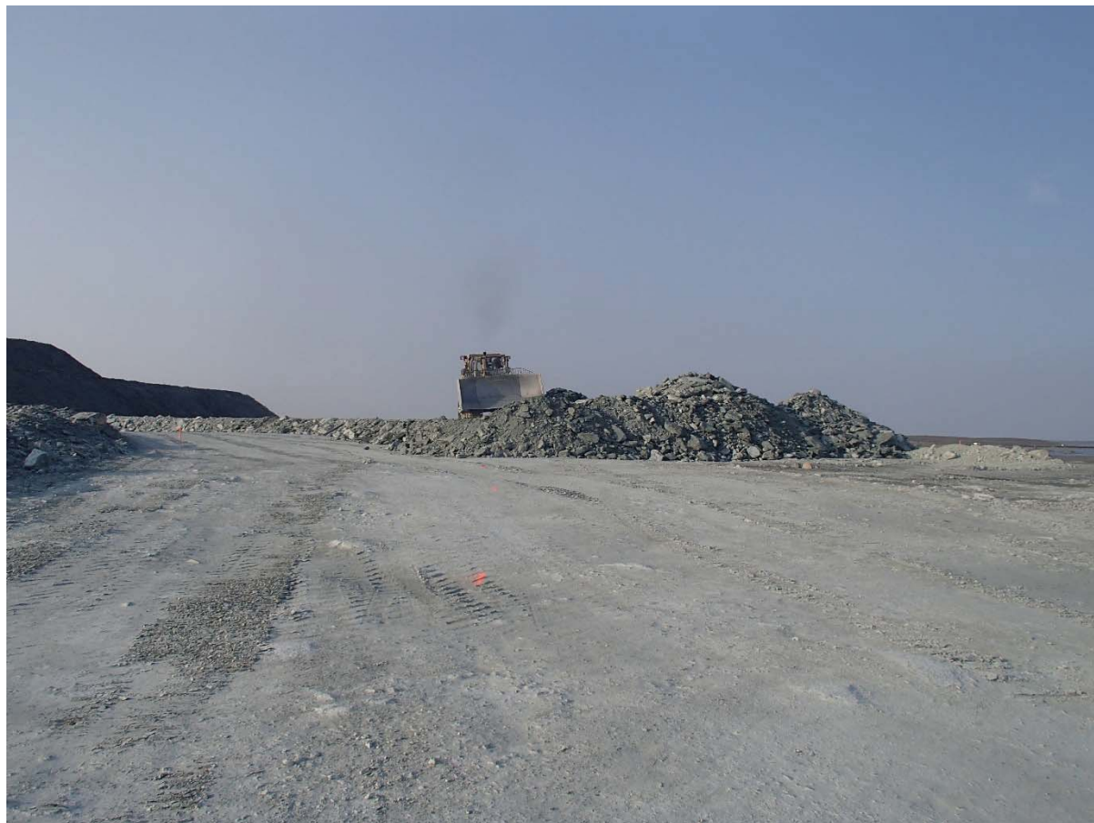
Photograph NCIS-089: From Sta 2+525/+4 m (approx.), looking S. Placement of a 2 m thick (approx.) lift of UM rockfill from El. 152 m to El. 154 m (approx.) with a dozer from Sta. 2+605 m to 2+455 m (+3 m to -23 m).
