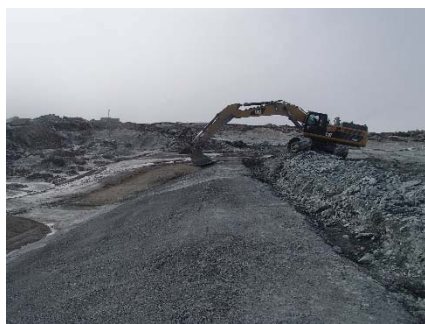
SD3-306 (2018-06-06), looking S from Sta. 20+780/-25 m. Correction of the surface of the fine filter in the upstream slope and the top of the first class compacted sieved till layer with an excavator from Sta. 20+803 m to 20+793 m.
