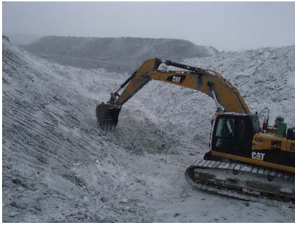
CD-1805 (2018-04-28), looking NE from Sta. 40+780/+2 m. Placement a 1.5 m thick (approx.) lift of intermediate volcanic (IV) rockfill from approx. Sta. 40+780 to 40+805 m (o.s. -6 to 9 m).
