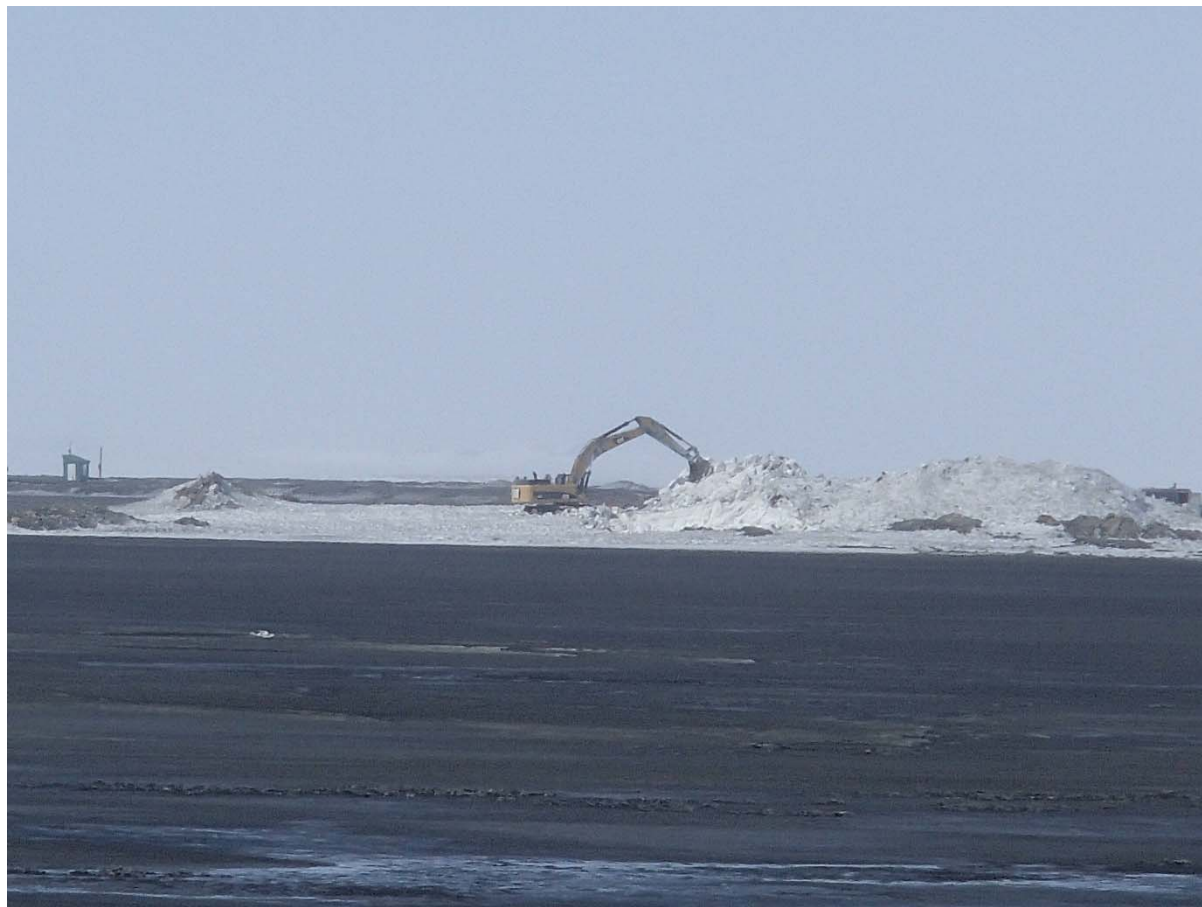
Photograph NCIS-024: From Sta. 2+570 m (approx.), looking SW. Removal of the snow bank in the footprint with an excavator from Sta. 1+160 m to 1+120 m (approx.).
