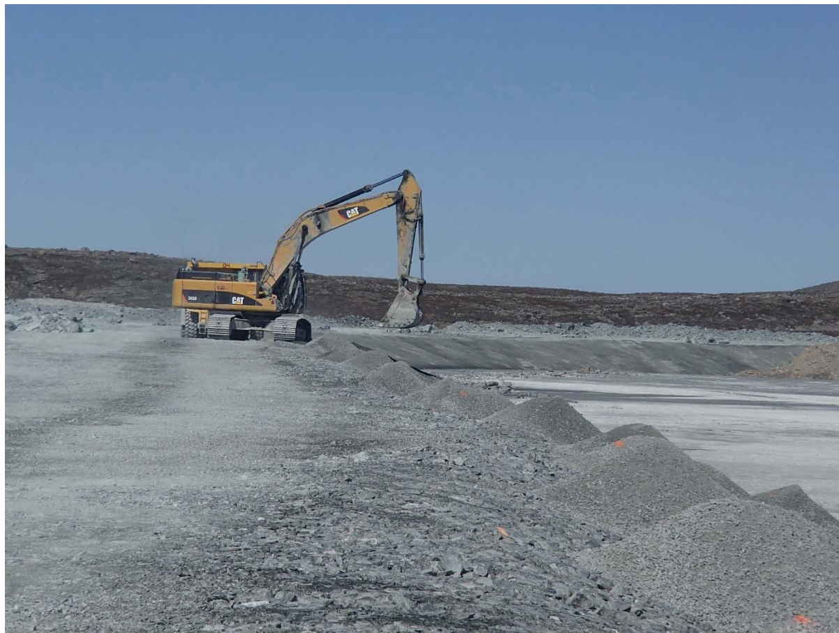
Photograph NCIS-066: From Sta. 1+400/-34 m (approx.), looking N. Placement of a 0.5 m thick lift of fine filter over the coarse filter in the upstream slope from El. 150 m to 152 m with an excavator from Sta. 1+595 m to 1+550 m.
