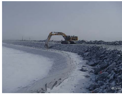
CD-1824 (2018-05-05), looking NE from Sta. 40+760/-25 m. Profiling of the upstream slope (2H:1V) from El. 143 to 145 m with an excavator between Sta. 0+830 m and 40+730 m.
