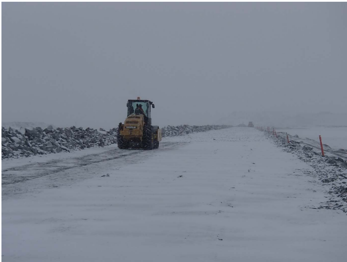
Photograph CD-1807: From Sta. 0+200/-15 m looking S. Compaction of the 2 m lift (approx.) of IV rockfill at El. 145 m with a 10-tonne smooth-drum compactor with vibration (6 passes) from Sta. 0+150 to 0+280 m (o.s. -21 to 11 m).
