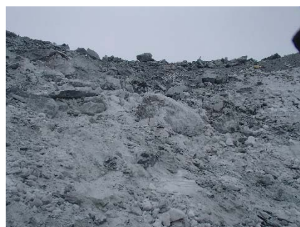
CD-1804 (2018-04-28), looking S from Sta. 40+790/-2 m. Presence of oversized boulders on the existing slope at the junction between SD5 and Central Dike.
