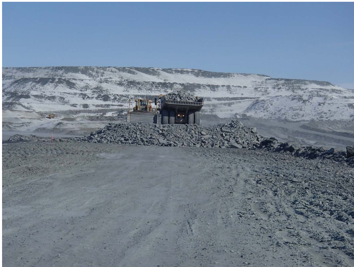
Photograph CD-1802: From Sta. 0+770/-16 m looking N. Placement of a 2 m thick (approx.) lift of intermediate volcanic (IV) rockfill from El. 143 m to El. 145 m from approx. Sta. 0+525 to 0+710 m (o.s. -28 to -18 m).
