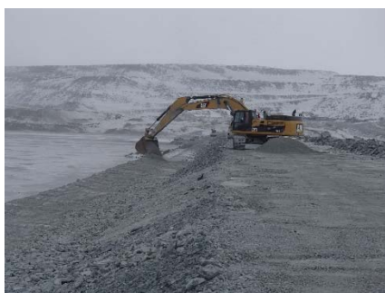
CD-1836 (2018-05-08), looking N from Sta. 0+580/-18 m. Placement of a first 0.5 m thick lift of fine filter from El. 143 m to 143.5 m upstream of the coarse filter with an excavator from Sta. 0+490 m to 0+835 m.
