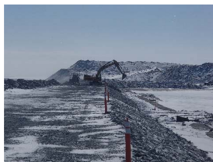
CD-1819 (2018-05-03), looking S from Sta. 0+560/-21 m. Profiling of the upstream slope (2H:1V) from El. 143 to 145 m with an excavator between Sta. 0+560 m and 0+830 m.
