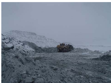
NCIS-005 (2018-05-19). Removal of the excavated material, pushed with a dozer towards the center of the North Cell to clear the upstream toe.
