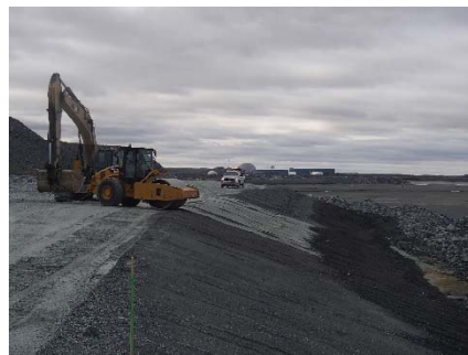
NCIS-129 (2018-07-28), looking S from Sta. 2+450/-21 m (approx.). Compaction of the 0.5 m lift (approx.) of fine filter between El. 152 m and 154 m with a 10-tonne smooth-drum compactor with vibration (4 passes) in the upstream slope from Sta. 2+220 m to 1+940 m.
