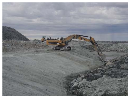
NCIS-078 (2018-07-05), looking S from Sta. 2+760/-39 m. Placement of a 0.5 m thick lift of fine filter over the coarse filter in the upstream slope from El. 150 m to 152 m with an excavator from Sta. 2+800 m to 2+980 m.
