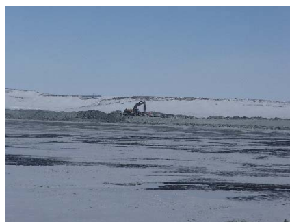
NCIS-018 (2018-05-25), looking NW from Sta. 2+310 m. Profiling of the upstream slope (3H:1V) from El. 150 to 152 m with an excavator from Sta. 1+989 m to 1+860 m.
