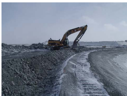
CD-1851 (2018-05-13), looking S from Sta. 0+910/-18 m. Excavation of the LLDPE geomembrane crest anchoring trench from Sta. 40+730 m to 0+830 m.
