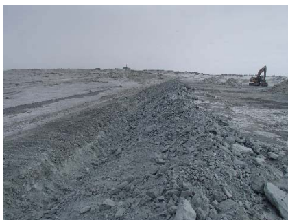
SD3-301 (2018-05-17), looking SE from Sta. 20+660/-22 m. Excavation of the LLDPE geomembrane crest anchoring trench with an excavator from Sta. 20+655 m to 20+675 m.
