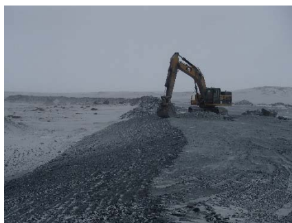
NCIS-019 (2018-05-26), looking SW from Sta. 2+100 m. Profiling of the upstream slope (3H:1V) from El. 150 to 152 m with an excavator from Sta. 1+860 m to 1+678 m. The portion between Sta. 1+900 m and 1+800 m, where the structure is built on the natural ground, was not profiled.
