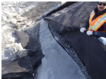
CD-1889 (2018-06-04), looking N from Sta. 0+150/-28 m. View of the underlying liner that has been cut at around Sta. 0+160 m to drain the water.
