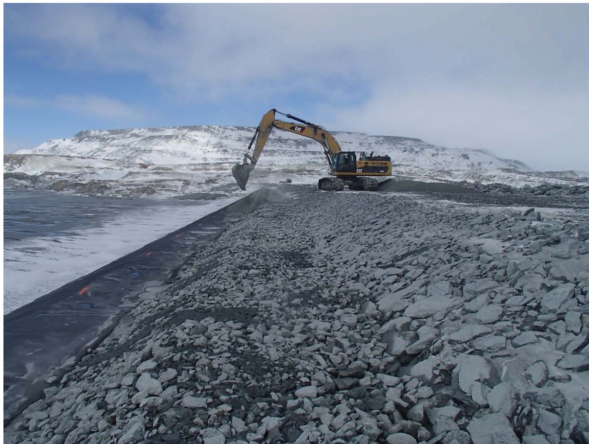
Photograph CD-1829: From Sta 0+410/-22 m, looking N. Placement of a 0.5 m thick lift of coarse filter from El. 143 m to 143.5 m with an excavator from Sta. 0+170 m to 0+460 m and placement of a 0.5 m thick lift of fine filter from Sta. 0+170 m to 0+380 m.
