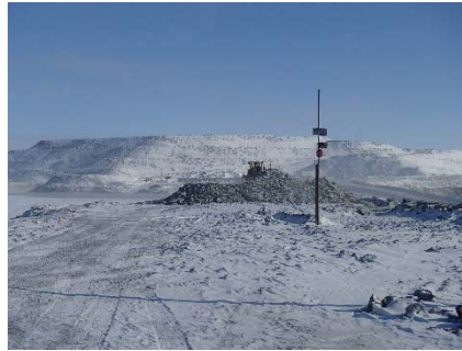
CD-1809 (2018-04-29), looking N from Sta. 0+870/-16 m. Placement a 2 m thick (approx.) lift of intermediate volcanic (IV) rockfill from El. 143 m to El. 145 m from approx. Sta. 0+760 to 0+835 m (o.s. -28 to 3 m).
