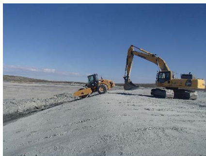
NCIS-112 (2018-07-24), looking N from Sta. 2+610/-29 m (approx.). Compaction of the 0.5 m lift (approx.) of coarse filter between El. 152 m and 154 m with a 10-tonne smooth-drum compactor with vibration (4 passes) in the upstream slope from Sta. 2+080 m to 2+000 m.
