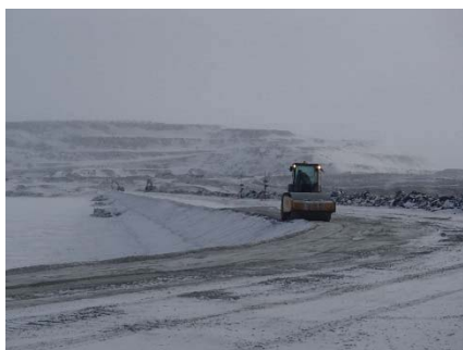
CD-1848 (2018-05-13), looking N from Sta. 40+780/-15 m. Compaction of the fourth 0.5 m lift (approx.) of fine and coarse filters material at El. 145 m with a 10-tonne smooth-drum compactor with vibration (4 passes) from Sta 0+930 m to 40+730 m.
