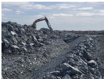
NCIS-130 (2018-07-28), looking S from Sta. 1+445/+16 m (approx.). Excavation of a 0.8 m (approx.) deep, 1 m wide shallow ditch in the rockfill capping with an excavator from Sta. 1+380 m to 1+300 m.
