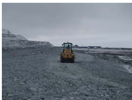
NCIS-022 (2018-05-30), looking SE from Sta. 2+245 m. Compaction of the 2 m lift (approx.) of ultramafic (UM) rockfill at El. 152 m with a 10-tonne smooth-drum compactor with vibration (6 passes) between the haul truck traffic lane and the upstream slope from Sta. 2+625 to 1+625 m (o.s. unavailable).
