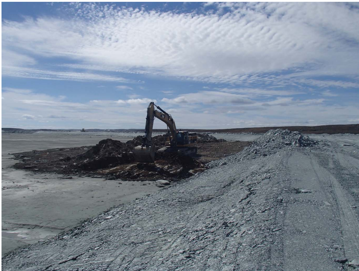
Photograph NCIS-031: From Sta. 1+880/-21 m (approx.), looking SW. Final clean-up of the dike footprint with an excavator to reach a good quality bedrock from Sta. 1+800 to 1+850 m (offset -42 to -33 m).
