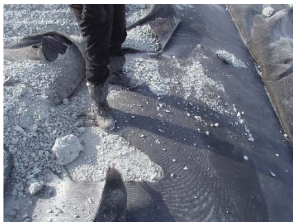
CD-1833 (2018-05-07), looking S from Sta. 0+390/-25 m. Damaged geomembrane near a deposition finger on Central Dike at Sta. 0+390 m.
