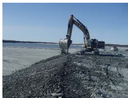
NCIS-063 (2018-06-30), looking SW from Sta. 1+200/-65 m. Placement of a 0.5 m thick lift of coarse filter in the upstream slope from El. 148 m to 150 m with an excavator from Sta. 1+270 m to 1+100 m.
