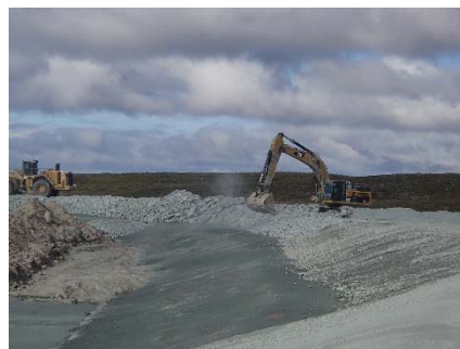
NCIS-132 (2018-07-29), looking W from Sta. 1+940/-20 m (approx.). Profiling of the upstream slope (3H:1V) from El. 152 to 154 m with an excavator from Sta. 1+780 m to 1+660 m.
