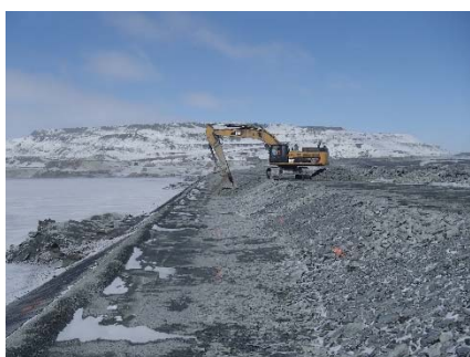
CD-1839 (2018-05-09), looking N from Sta. 0+835/-20 m. Placement of a second 0.5 m thick lift of coarse filter from El. 143.5 m to 144 m with an excavator from Sta. 0+500 m to 0+835 m and from 0+930 to 40+730 m.
