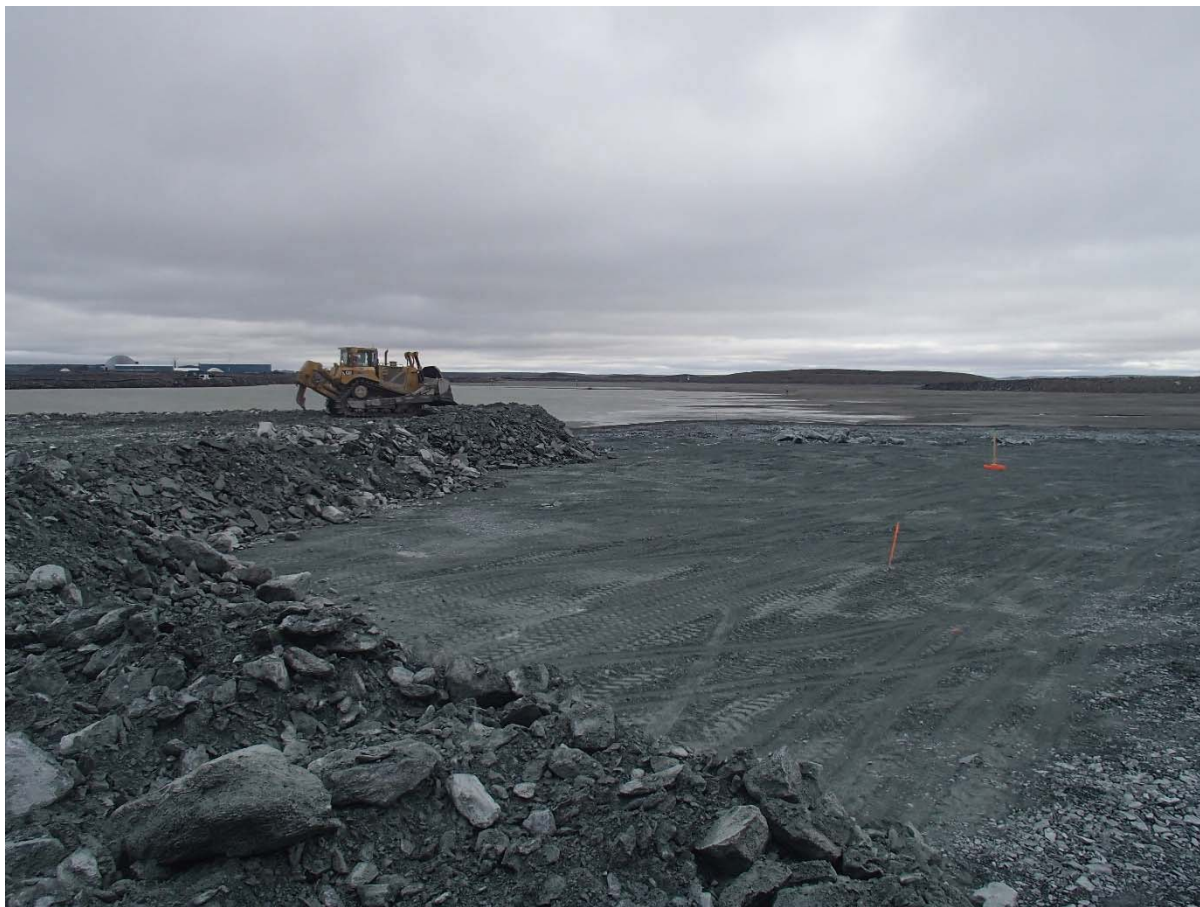
Photograph NCIS-083: From Sta 1+140/-52 m (approx.), looking SW. Placement of a 2 m thick (approx.) lift of IV rockfill from El. 150 m to El. 152 m (approx.) with a dozer from Sta. 1+160 m to 1+170 m (-64 m to -111 m). The material is of good quality and is well graded.
