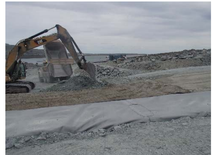
SD3-346 (2018-07-17), looking E from Sta. 20+760/-21 m. Placement of a third 0.5 m thick lift of fine UM rockfill (0-500 mm) upstream of the low quality till (0-150mm) from El. 143 m to 143.5 m from Sta. 20+668 m to 20+777 m.
