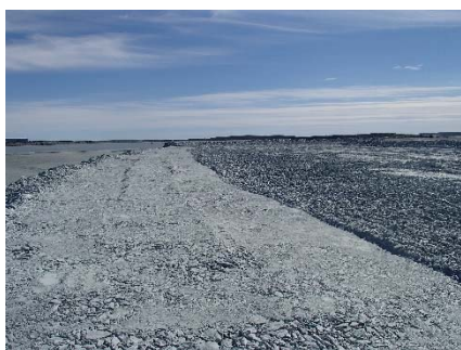
NCIS-050 (2018-06-26), looking S from Sta. 1+230/-55 m. Compaction of the 1.5 to 2 m lift (approx.) of ultramafic (UM) rockfill at El. 150 m with a 10-tonne smooth-drum compactor with vibration (6 passes) between the haul truck traffic lane and the upstream slope from Sta. 1+220 to 1+130 m (o.s. -91 to -44 m).
