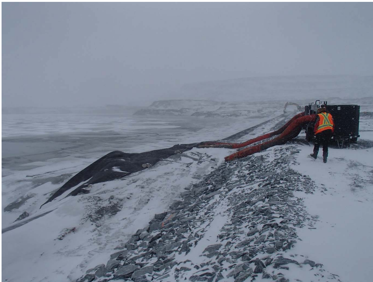
Photograph CD-1828: From Sta 0+410/-22 m, looking N. Defrosting of the deposition finger materials with two Frost Fighters at Sta. 0+390 m.
