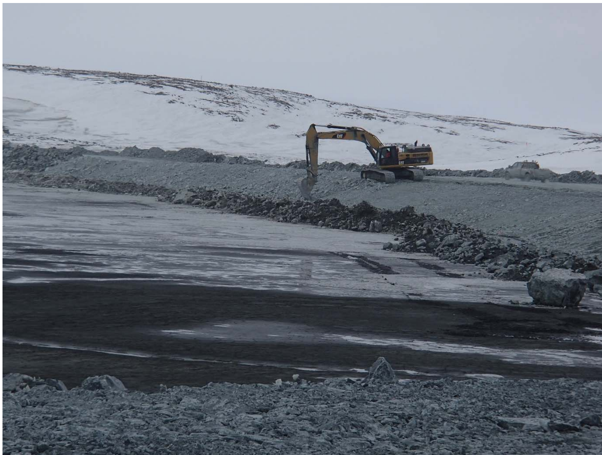
Photograph NCIS-017: From Sta. 2+290 m (approx.), looking SW. Profiling of the upstream slope (3H:1V) from El. 150 to 152 m with an excavator from Sta. 2+138 m to 1+989 m.
