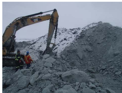
NCIS-003 (2018-05-19). Excavation of the snow-rich upstream toe material on an average width of 2 to 3 m with an excavator.
