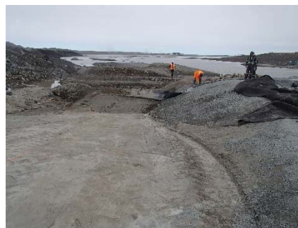
SD3-314 (2018-06-08), looking E from Sta. 20+590/-32 m. View of the liner bedding ready for geosynthetics installation.
