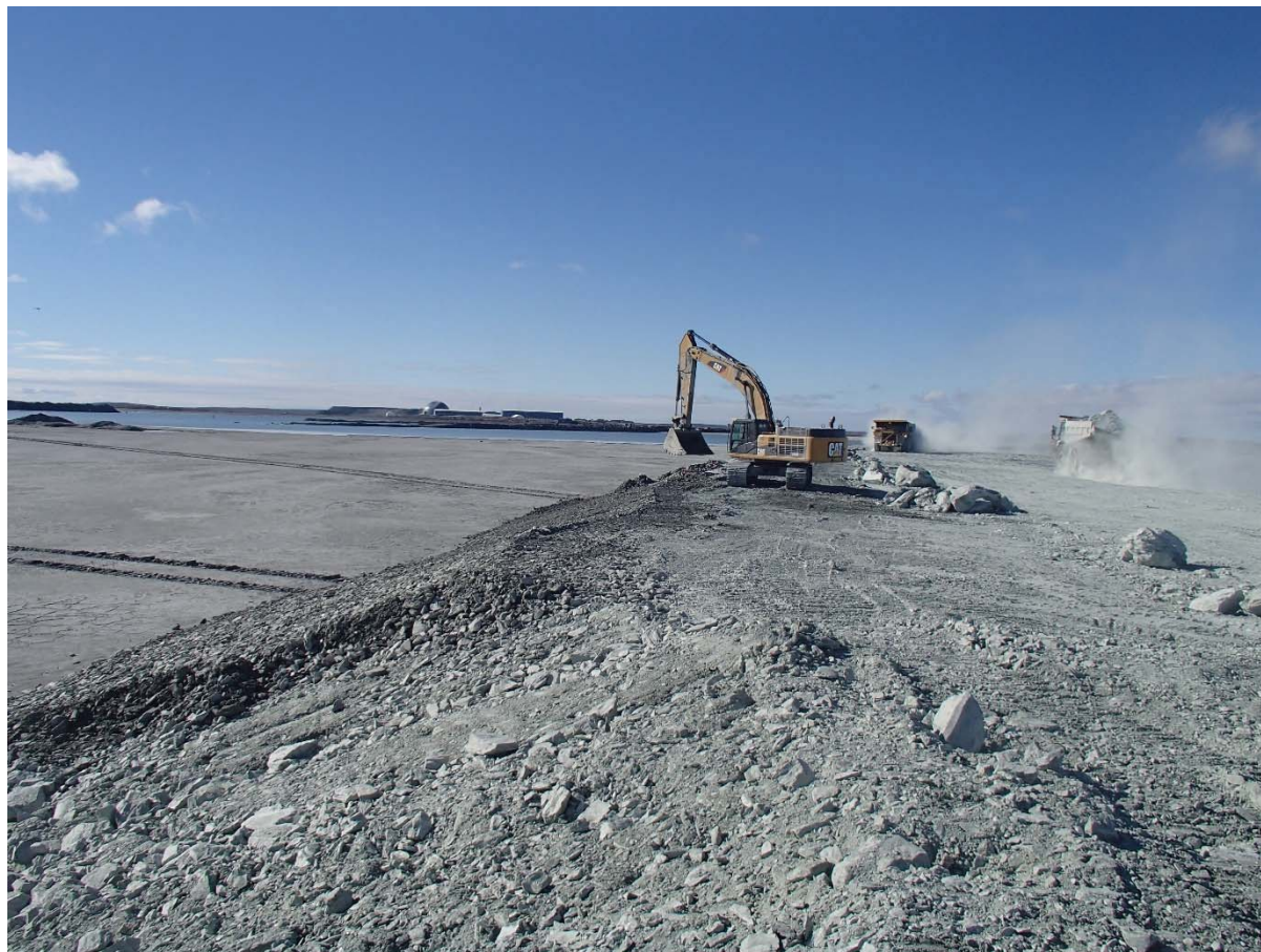
Photograph NCIS-058: From Sta. 1+340/-34 m (approx.), looking S. Placement of a 0.5 m thick lift of coarse filter in the upstream slope from El. 148 m to 152 m with an excavator from Sta. 1+340 m to 1+270 m.
