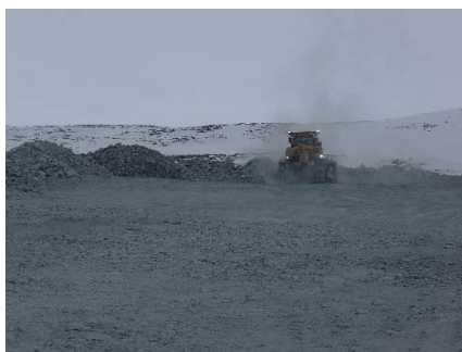
NCIS-011 (2018-05-22), looking SW from Sta. 2+000 m. Placement a 2 m thick (approx.) lift of UM rockfill from El. 150 m to El. 152 m (approx.) with a dozer from Sta. 1+880 m to 1+767 m (o.s. unavailable).
