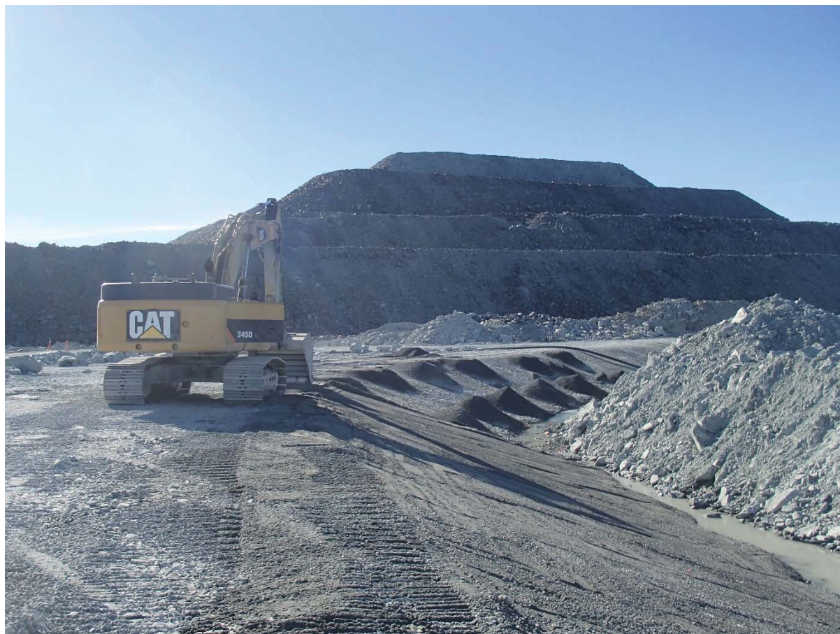
Photograph NCIS-071: From Sta. 2+670/-28 m (approx.), looking SE. Placement of a 0.5 m thick lift of fine filter over the coarse filter in the upstream slope from El. 150 m to 152 m with an excavator from Sta. 1+550 m to 1+320 m and 1+630 m to 1+610 m.
