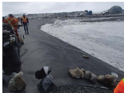
CD-1870 (2018-05-27), looking S from Sta. 0+900/-26 m. Installation of the LLDPE liner on the upstream slope 2H:1V between El. 143 m and 145 m from Sta. 0+935 m to 0+900 m (panel numbers 820 to 823).
