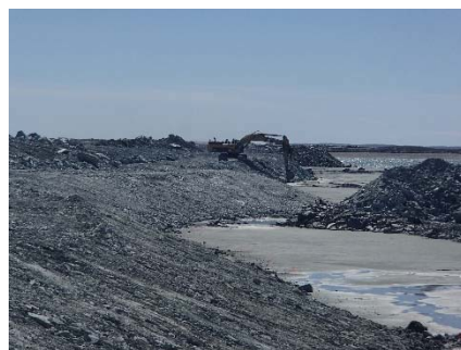
NCIS-072 (2018-07-02), looking W from Sta. 2+790/-38 m. Profiling of the upstream slope (3H:1V) from El. 150 to 152 m with an excavator from Sta. 2+975 m to 3+070 m.
