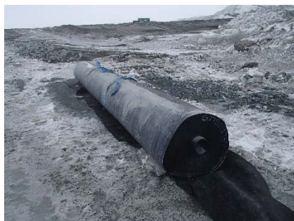
SD3-303 (2018-05-21), looking N from Sta. 20+780/-15 m. View of a LLDPE liner roll stored on geotextile.
