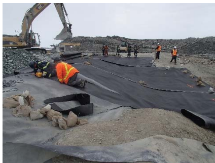
SD3-315 (2018-06-08), looking W from Sta. 20+615/-46 m. Installation of the geotextile on the upstream slope 3H:1V between El. 143 m and 145 m from Sta. 20+593 m to 20+610 m and installation of the LLDPE liner on the upstream slope 3H:1V between El. 143 m and 145 m from Sta. 20+593 m to 20+610 m (panel numbers 965 to 967).
