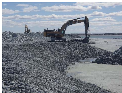
NCIS-075 (2018-07-03), looking S from Sta. 2+860/-36 m. Placement of a 0.5 m thick lift of coarse filter in the upstream slope from El. 150 m to 152 m with an excavator from Sta. 2+815 m to 2+980 m.
