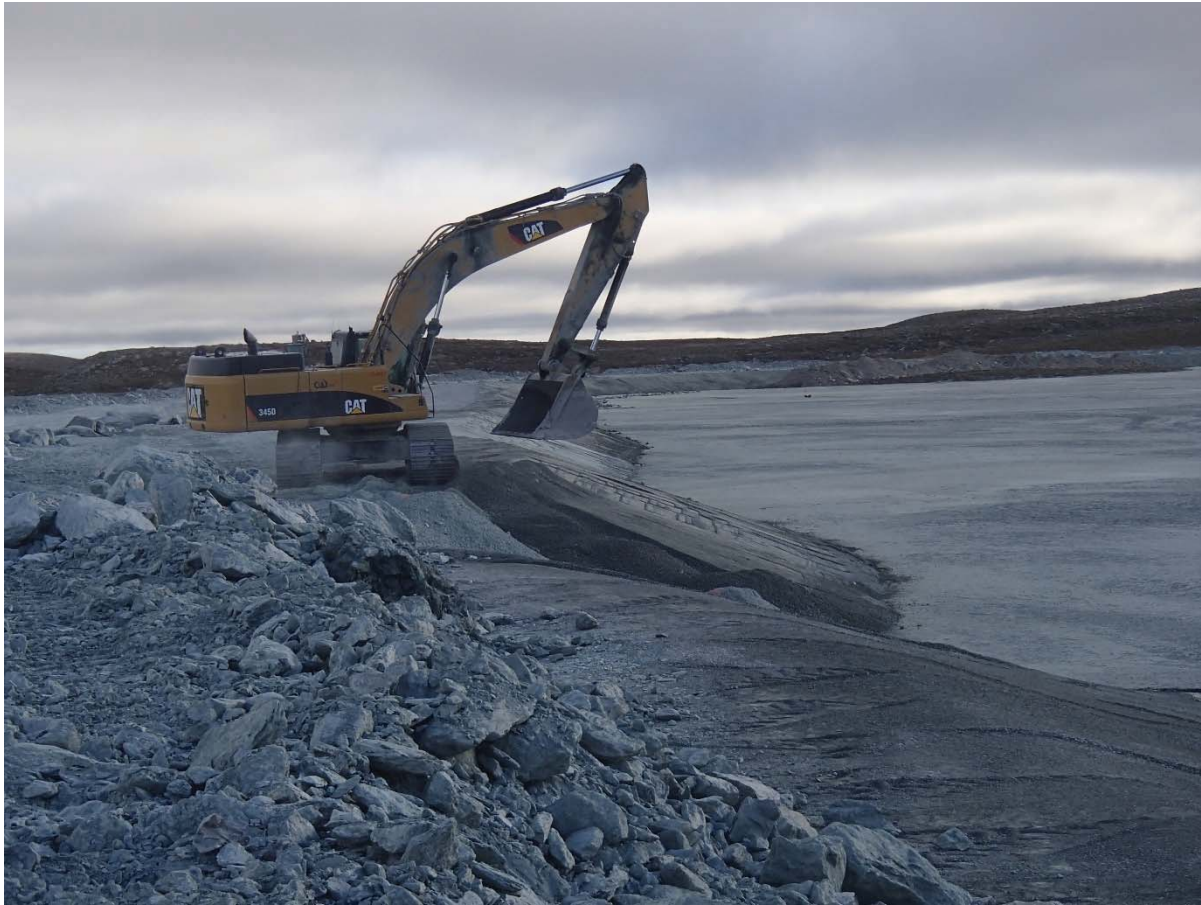
Photograph NCIS-073: From Sta. 1+300/-33 m (approx.), looking N. Placement of a 0.5 m thick lift of fine filter over the coarse filter in the upstream slope from El. 150 m to 152 m with an excavator from Sta. 1+320 m to 1+300 m.
