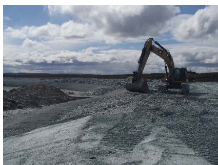
NCIS-133 (2018-07-29), looking W from Sta. 1+820/-28 m (approx.). Placement of a 0.5 m thick lift of coarse filter in the upstream slope from El. 152 m to 154 m with an excavator from Sta. 1+890 m to 1+826 m.
