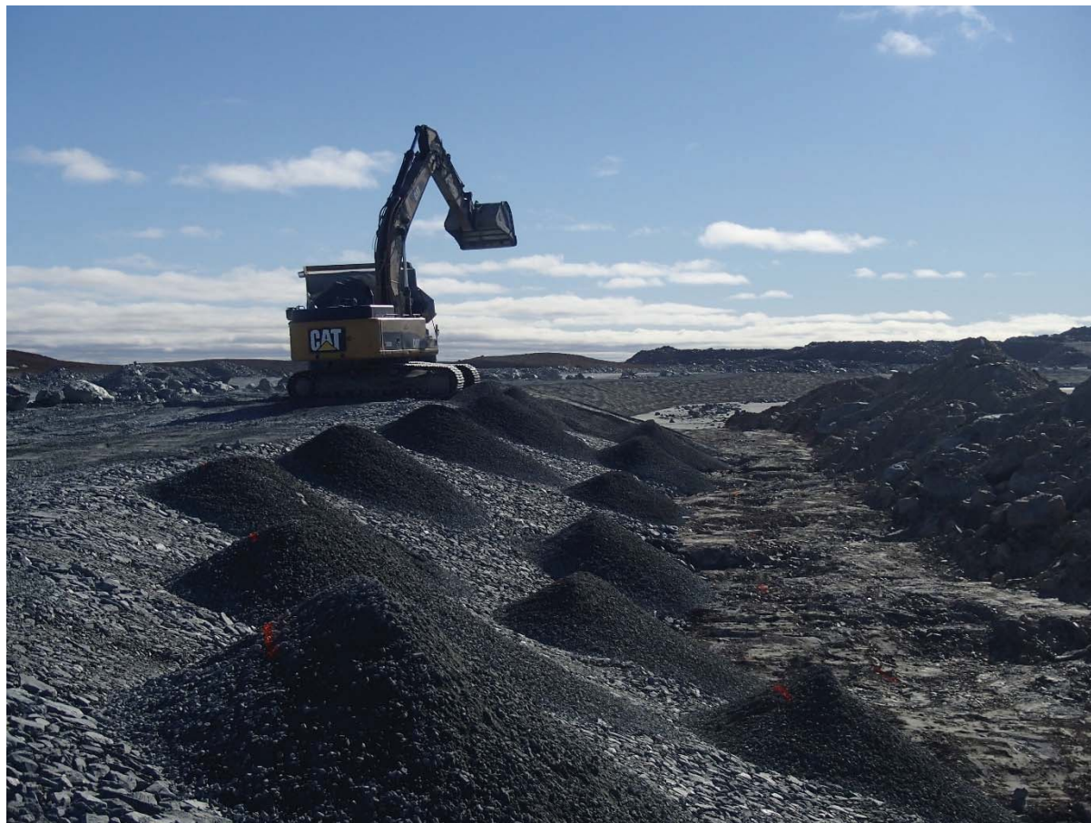
Photograph NCIS-055: From Sta. 1+730/-42 m (approx.), looking NE. Placement of a 0.5 m thick lift of fine filter over the coarse filter in the upstream slope from El. 150 m to 152 m with an excavator from Sta. 1+820 m to 1+595 m.
