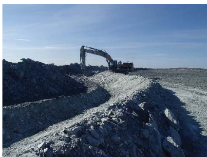
NCIS-116 (2018-07-25), looking SE from Sta. 1+700/+37 m (approx.). Excavation of a 0.8 m (approx.) deep, 1 m wide shallow ditch in the rockfill capping with an excavator from Sta. 1+500 m to 1+455 m.
