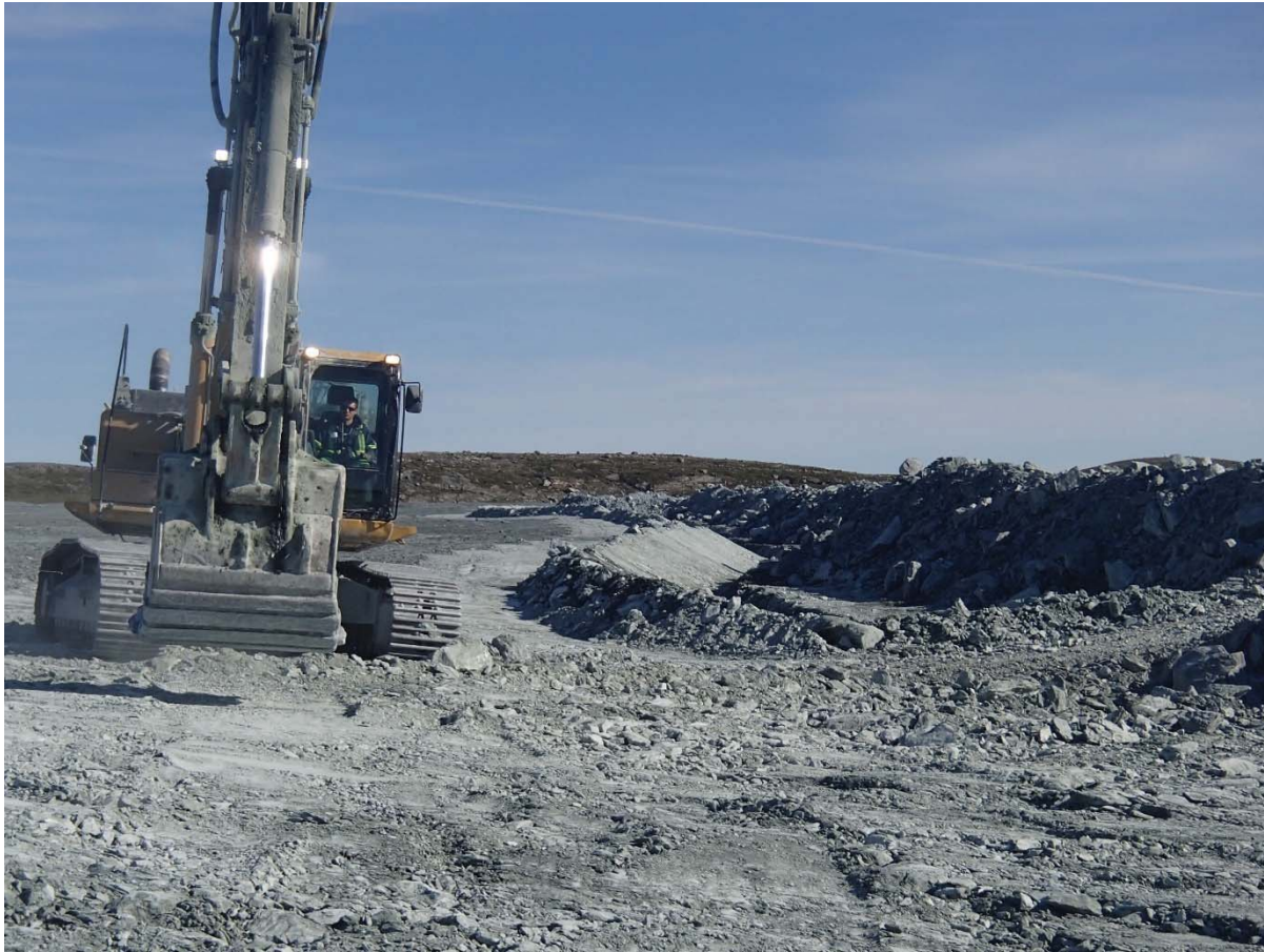
Photograph NCIS-119: From Sta. 1+430/-22 m (approx.), looking N. Excavation of a 0.8 m (approx.) deep, 1 m wide shallow ditch in the rockfill capping with an excavator from Sta. 1+455 m to 1+400 m.
