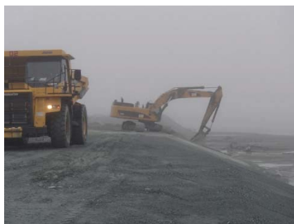
NCIS-082 (2018-07-07), looking S from Sta. 3+060/-33 m. Placement of a 0.5 m thick lift of fine filter over the coarse filter in the upstream slope from El. 150 m to 152 m with an excavator from Sta. 3+120 m to 3+160 m.
