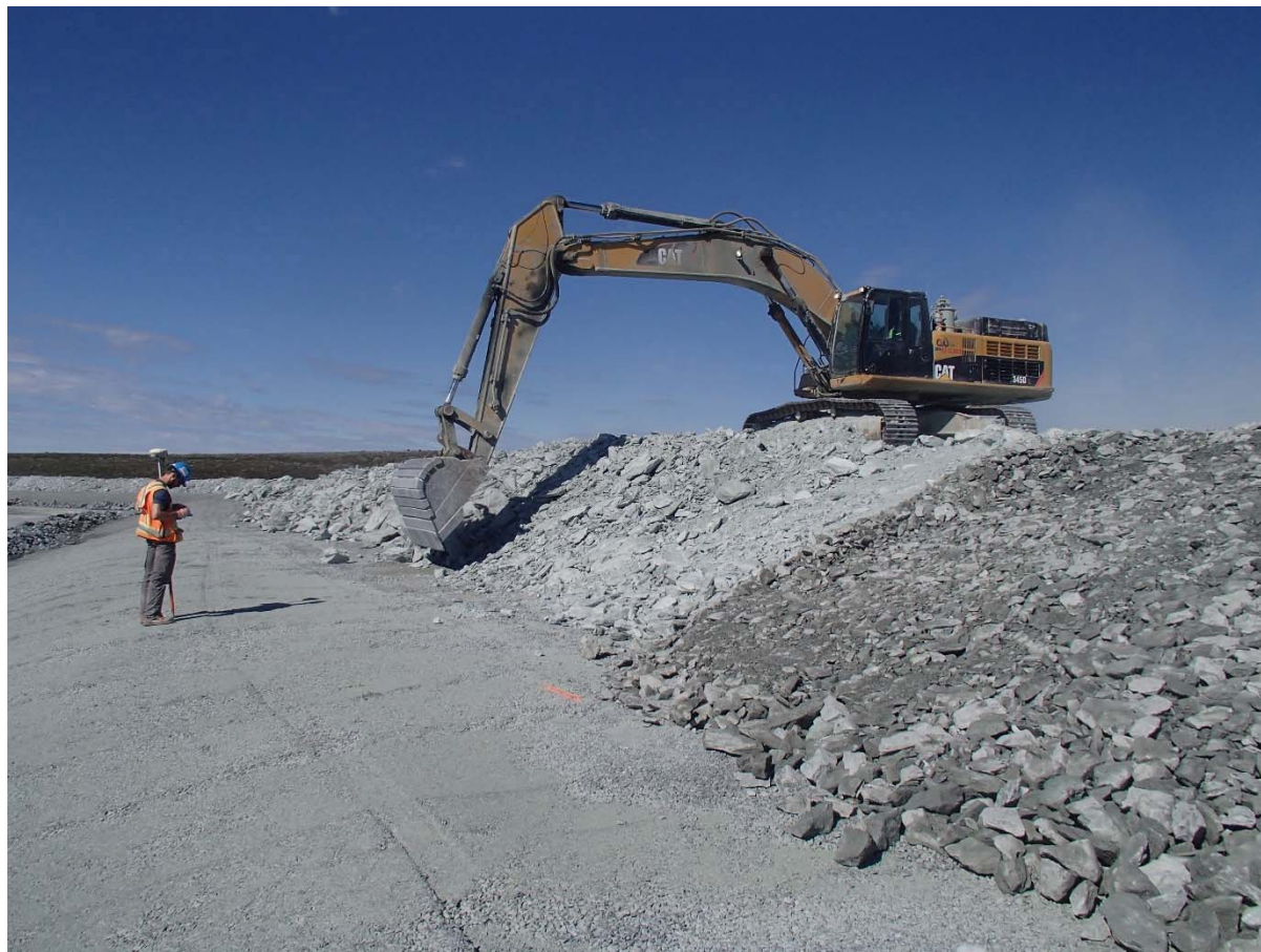
Photograph NCIS-103: From Sta. 2+420/-27 m (approx.), looking NE. Profiling of the upstream slope (3H:1V) from El. 152 to 154 m with an excavator from Sta. 2+400 m to 2+410 m. Oversize boulders were removed.
