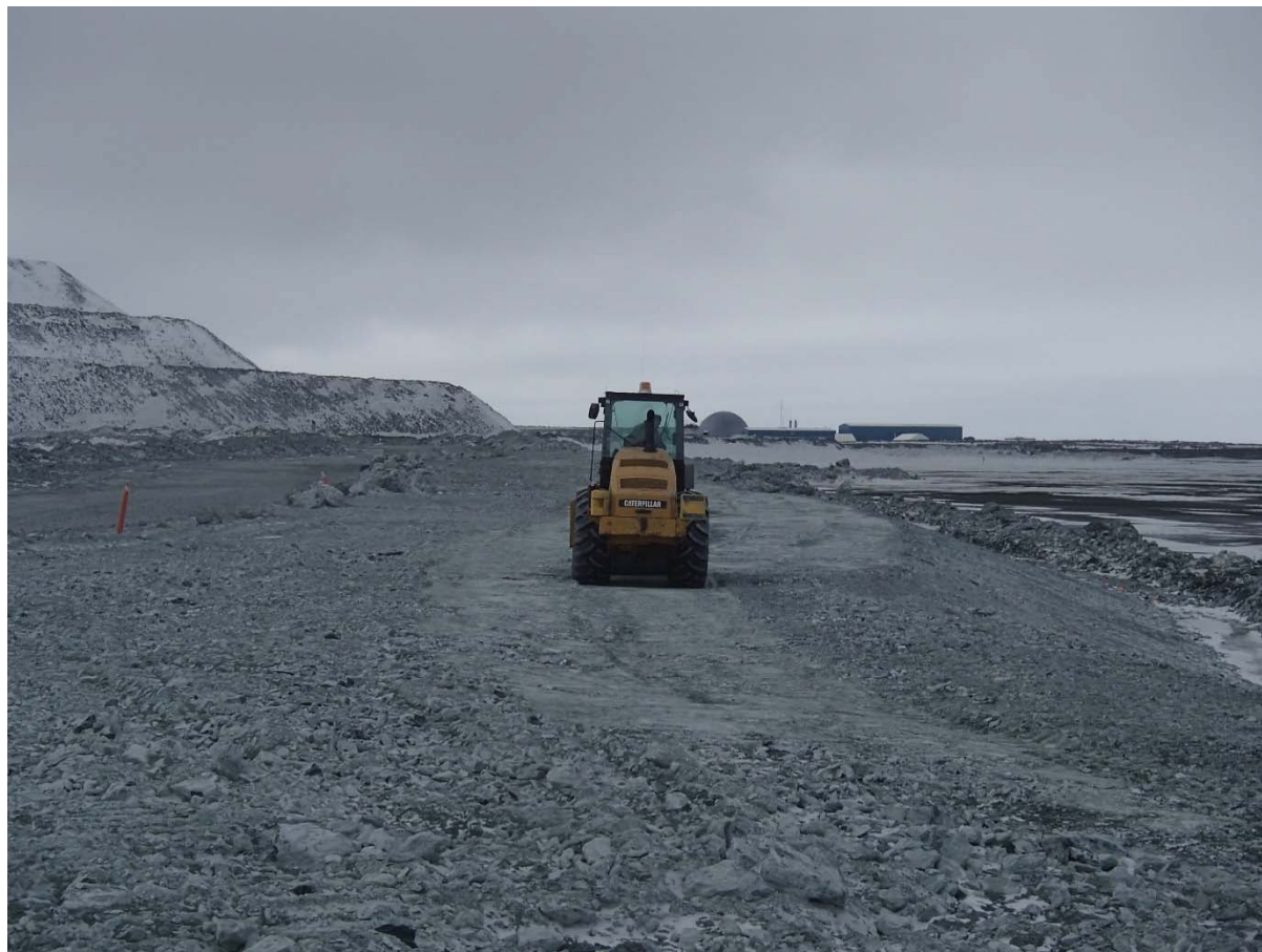
Photograph NCIS-022: From Sta. 2+245 m (approx.), looking SE. Compaction of the 2 m lift (approx.) of ultramafic (UM) rockfill at El. 152 m with a 10-tonne smooth-drum compactor with vibration (6 passes) between the haul truck traffic lane and the upstream slope from Sta. 2+625 to 1+625 m (offset unavailable).
