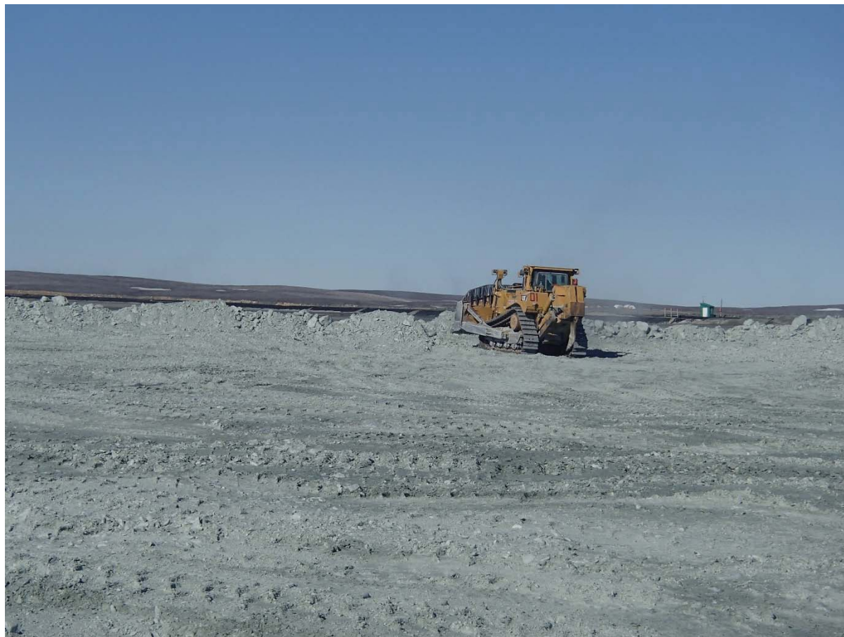
Photograph NCIS-052: From Sta. 1+120/-87 m (approx.), looking SW. Placement of a 1.5 to 2 m thick (approx.) lift of UM rockfill from El. 148 m to El. 150 m (approx.) with a dozer from Sta. 1+115 m to 1+100 m (-107 m to -45 m). The material is of good quality and is well graded.
