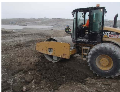
SD3-313 (2018-06-08), looking S from Sta. 20+600/-52 m. Compaction of the 0.15 m-thick lift of compacted sieved till with a 10-tonne smooth-drum compactor without vibration (4 passes) from Sta. 20+596 m to 20+601 m.
