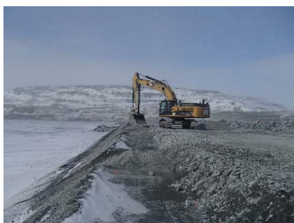
CD-1845 (2018-05-11), looking N from Sta. 0+660/-20 m. Profiling of the upstream slope (2H:1V) from El. 143 to 145 m with an excavator between Sta. 0+175 and 0+330 m and between Sta. 0+600 m and 0+715 m.
