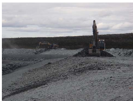
NCIS-109 (2018-07-22), looking N from Sta. 2+450/-21 m (approx.). Placement of a 0.5 m thick lift of coarse filter in the upstream slope from El. 152 m to 154 m with an excavator from Sta. 2+293 m to 2+411 m.
