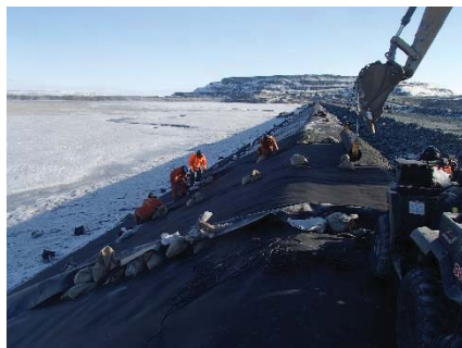
CD-1871 (2018-05-28), looking N from Sta. 0+910/-25 m. Installation of the geotextile on the upstream slope 2H:1V between El. 143 m and 145 m from Sta. 0+900 m to 0+870 m.
