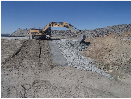
SD3-341 (2018-07-15), looking W from Sta. 20+600/-59 m. Placement of a first 0.5 m thick lift of fine rockfill on the upstream slope of the upstream toe liner tie-in with an excavator from Sta. 20+588 m to 20+599 m.
