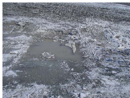
SD3-302 (2018-05-18), looking NE from Sta. 20+595/-42 m. View of water ponding on the first compacted sieved till layer of upstream toe liner tie-in. A portion of exposed damaged LLDPE liner is visible.
