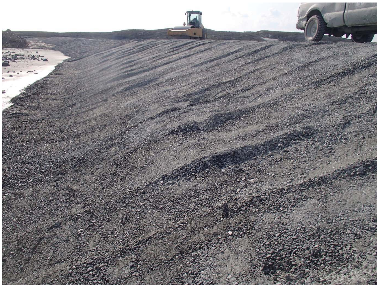
Photograph NCIS-087: From Sta 1+950/-34 m (approx.), looking W. Compaction of the 0.5 m lift (approx.) of fine filter between El. 150 and 152 m with a 10-tonne smooth-drum compactor (4 passes) in the upstream slope from Sta. 2+000 m to 1+930 m. Vibration is used except for the first pass down the slope in order to stabilize the material and limit deformation of the lift.
