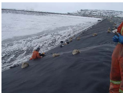
CD-1866 (2018-05-25), looking NW from Sta. 0+940/-25 m. Installation of the LLDPE liner on the upstream slope 2H:1V between El. 143 m and 145 m from Sta. 0+950 m to 0+935 m (panel numbers 818 and 819).
