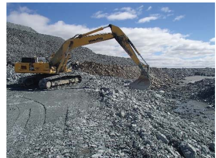
NCIS-045 (2018-06-25), looking S from Sta. 2+760/-40 m. Profiling of the upstream slope (3H:1V) from El. 150 to 152 m with an excavator from Sta. 2+715 m to 2+825 m.
