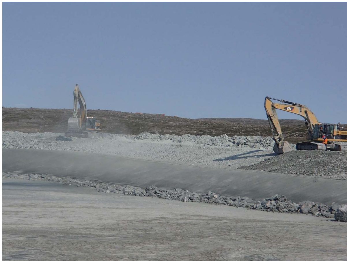
Photograph NCIS-111: From Sta. 2+320/-22 m (approx.), looking NW. Profiling of the upstream slope (3H:1V) from El. 152 to 154 m with an excavator from Sta. 2+159 m to 2+000 m and placement of a 0.5 m thick lift of coarse filter in the upstream slope from El. 152 m to 154 m with an excavator from Sta. 2+293 m to 2+080 m.
