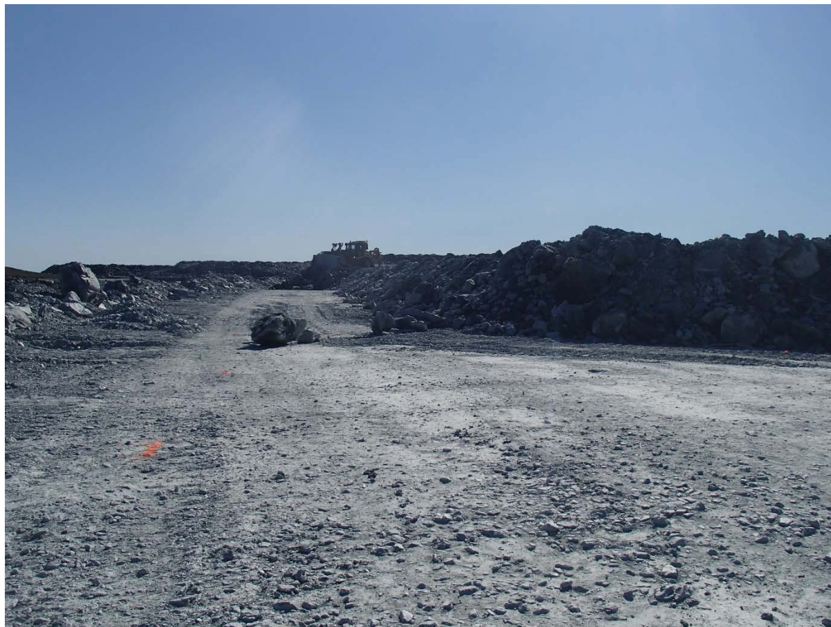
Photograph NCIS-100: From Sta. 1+960/+10 m (approx.), looking E. Placement of a 2 m thick (approx.) lift of UM rockfill from El. 152 m to El. 154 m (approx.) with a dozer from Sta. 1+984 m to 1+947 m (+14 m to -26 m). The material is of good quality and is well graded.
