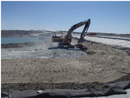
SD3-344 (2018-07-16), looking S from Sta. 20+610/-43 m. Placement of a third 0.5 m thick lift of low quality till (0-150 mm) from El. 142.5 m to 143 m from Sta. 20+570 m to 20+590 m.
