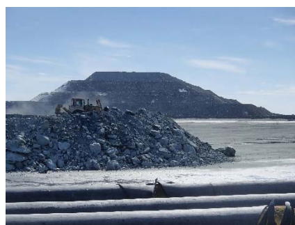
NCIS-027 (2018-06-07), looking E from Sta. 1+360/+67 m. Placement of a 2 m thick (approx.) lift of UM rockfill from El. 150 m to El. 152 m (approx.) with a dozer from Sta. 1+365 m to 1+360 m (+9 m to -28 m).
