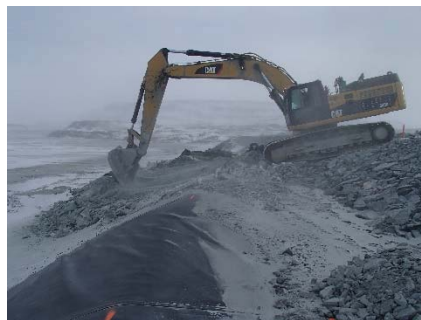
CD-1830 (2018-05-07), looking N from Sta. 0+420/-26 m. Removal of the deposition finger materials with an excavator at Sta. 0+390 m.
