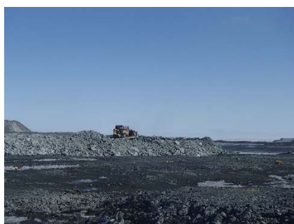
NCIS-025 (2018-06-01), looking SE from Sta. 1+475 m. Placement of a 2 m thick (approx.) lift of UM rockfill from El. 150 m to El. 152 m (approx.) with a dozer from Sta. 1+450 m to 1+390 m (o.s. unavailable). The material is of good quality and is well graded.
