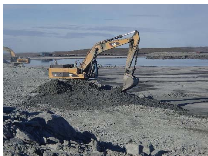
NCIS-076 (2018-07-04), looking SW from Sta. 2+940/-15 m. Placement of a 0.5 m thick lift of coarse filter in the upstream slope from El. 150 m to 152 m with an excavator from Sta. 2+980 m to 3+160 m.
