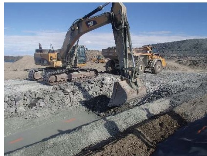
CD-1897 (2018-07-22), looking NW from Sta. 0+145/-30 m. Placement of a 0.5 m thick lift of coarse filter on the top of the fine filter on the top of the upstream toe liner tie-in and on the upstream slope with an excavator from Sta. 0+147 m to 0+177 m.
