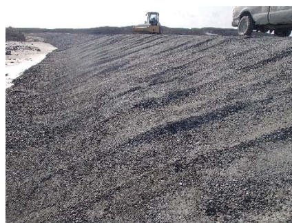
NCIS-087 (2018-07-11), looking W from Sta. 1+950/-34 m (approx.). Compaction of the 0.5 m lift (approx.) of fine filter between El. 150 and 152 m with a 10-tonne smooth-drum compactor (4 passes) in the upstream slope from Sta. 2+000 m to 1+930 m.
