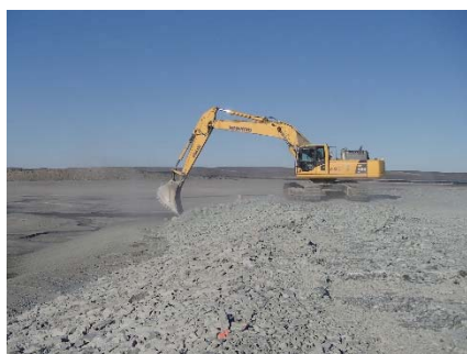
NCIS-094 (2018-07-15), looking SW from Sta. 1+125/-109 m (approx.). Profiling of the upstream slope (3H:1V) from El. 150 to 152 m with an excavator from Sta. 1+135 m to 1+115 m.
