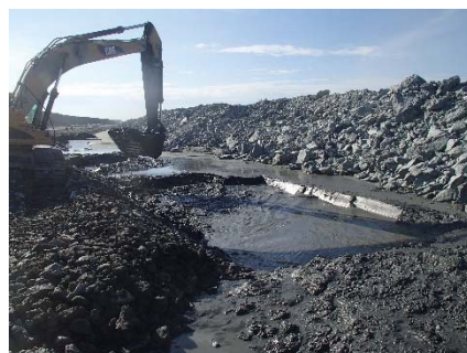
NCIS-123 (2018-07-27), looking S from Sta. 3+340/+33 m (approx.). Excavation of a 1 m (approx.) deep sump (south sump) in the tailings with an excavator from Sta. 3+345 m to 3+365 m (o.s. +24 to +32 m).
