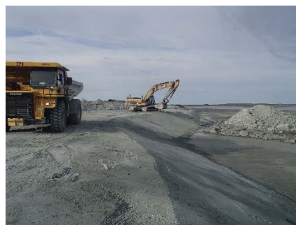
NCIS-081 (2018-07-06), looking SE from Sta. 2+975/-37 m (approx.). Placement of a 0.5 m thick lift of fine filter over the coarse filter in the upstream slope from El. 150 m to 152 m with an excavator from Sta. 1+300 m to 1+210 m and from Sta. 2+940 m to 3+120 m.
