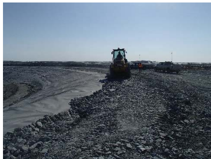
CD-1895 (2018-06-11), looking E from Sta. 40+670/-15 m. Compaction of the geosynthetics tie-in material at El. 145 m with a 10-tonne smooth-drum compactor with vibration (4 passes) from Sta. 40+670 m to 0+950 m.
