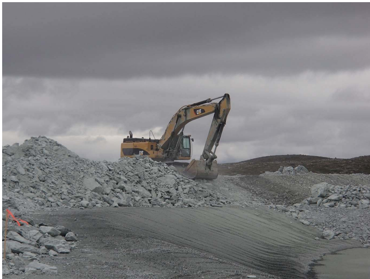
Photograph NCIS-134: From Sta. 1+630/-32 m (approx.), looking NE. Completion of the profiling of the upstream slope (3H:1V) from El. 152 to 154 m with an excavator from Sta. 1+700 m to 1+660 m.
