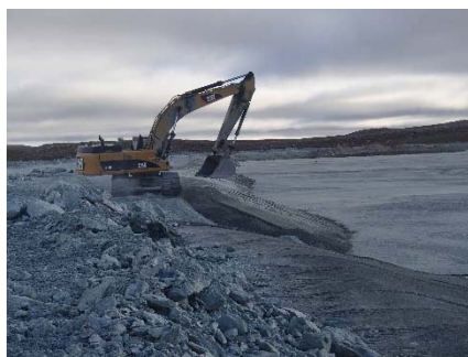
NCIS-073 (2018-07-03), looking N from Sta. 1+300/-33 m. Placement of a 0.5 m thick lift of fine filter over the coarse filter in the upstream slope from El. 150 m to 152 m with an excavator from Sta. 1+320 m to 1+300 m.
