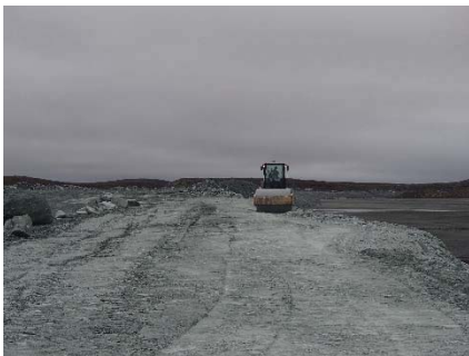
NCIS-043 (2018-06-25), looking N from Sta. 1+250/-38 m. Compaction of the 1.5 to 2 m lift (approx.) of ultramafic (UM) rockfill at El. 150 m with a 10-tonne smooth-drum compactor with vibration (6 passes) between the haul truck traffic lane and the upstream slope from Sta. 1+330 to 1+200 m (o.s. -53 to -24 m).
