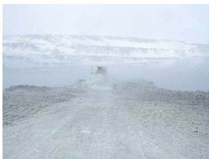
CD-1800 (2018-04-25), looking N from Sta. 0+500/-14 m. Placement a 2 m thick (approx.) lift of intermediate volcanic (IV) rockfill from El. 143 m to El. 145 m from 0+435 to 0+535m (o.s. -28 to -18 m).
