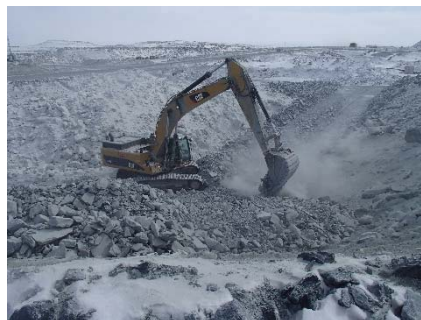
CD-1812 (2018-04-30), looking SE from Sta. 0+985/-11 m. Placement of intermediate volcanic (IV) rockfill on the existing downstream slope up to approx. El. 140 m, from approx. Sta. 0+985 to 40+780 m.
