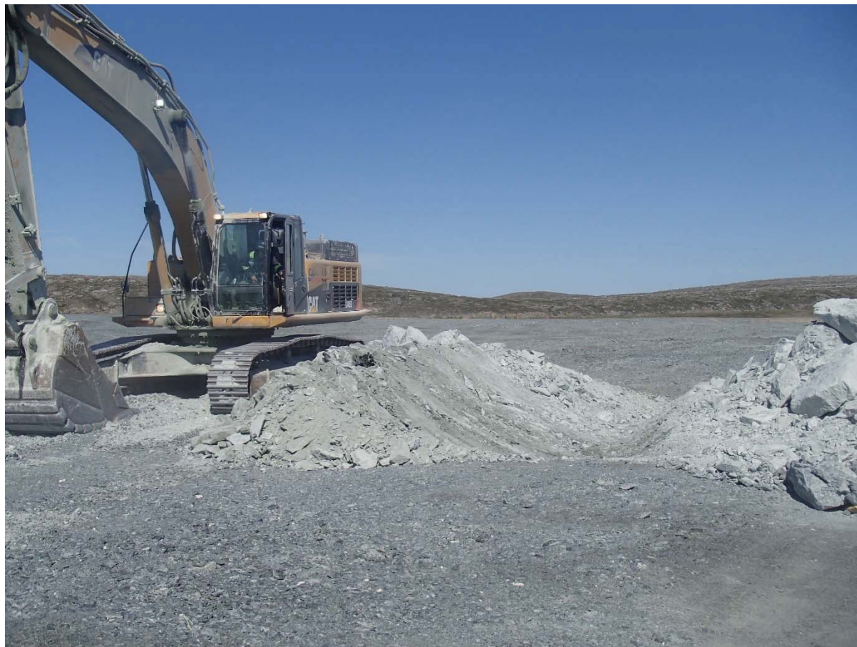
Photograph NCIS-114: From Sta. 1+700/-34 m (approx.), looking N. Excavation of a 0.8 m (approx.) deep, 1 m wide shallow ditch in the rockfill capping with an excavator from Sta. 1+500 m to 1+650 m.
