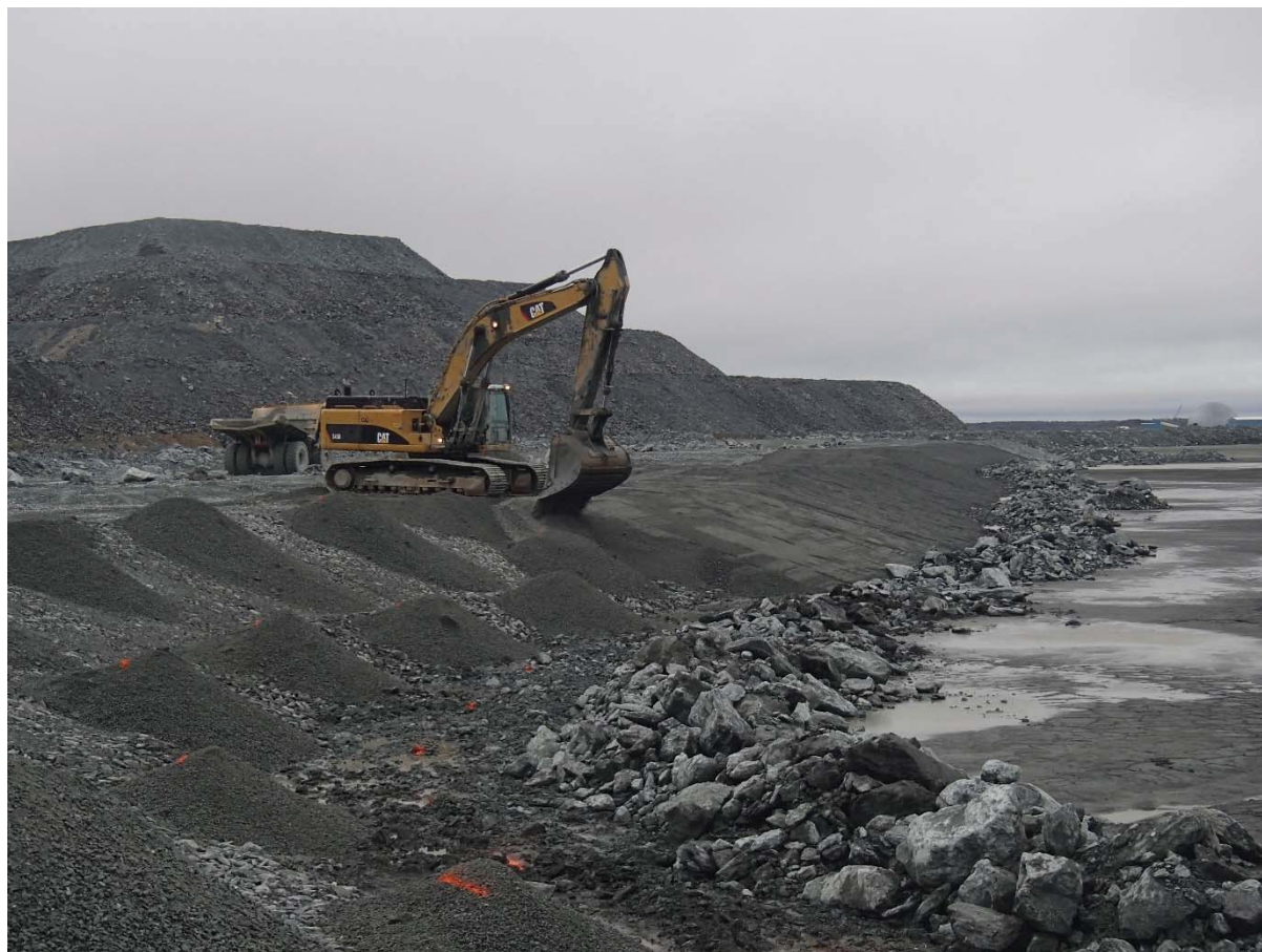
Photograph NCIS-042: From Sta. 2+210/-27 m (approx.), looking SE. Placement of a 0.5 m thick lift of fine filter over the coarse filter in the upstream slope from El. 150 m to 152 m with an excavator from Sta. 2+305 m to 2+040 m.
