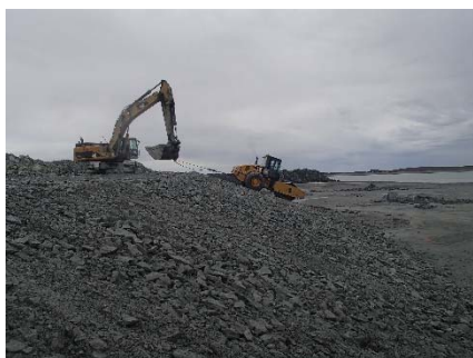
NCIS-080 (2018-07-05), looking S from Sta. 2+800/-38 m. Compaction of the 0.5 m lift (approx.) of coarse filter between El. 150 and 152 m with a 10-tonne smooth-drum compactor (4 passes) in the upstream slope from Sta. 2+925 m to 3+160 m and from Sta. 1+300 m to 1+200 m.
