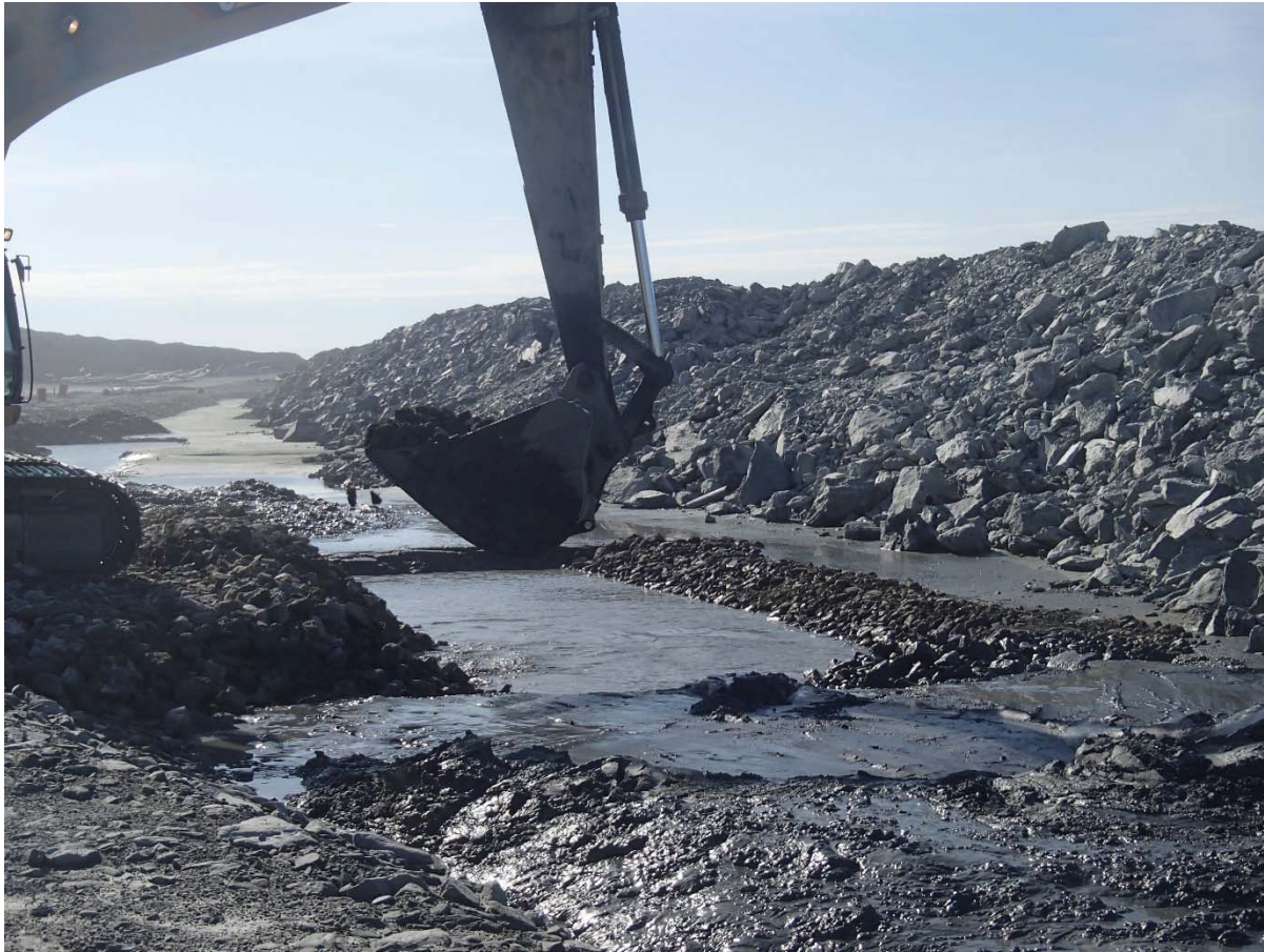
Photograph NCIS-124: From Sta. 3+340/+33 m (approx.), looking S. Placement of a 0.3 m thick (approx.) layer of till sieving reject material on the bottom and on the slopes of the south sump.
