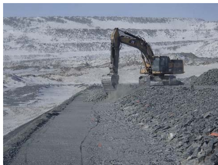
CD-1832 (2018-05-07), looking N from Sta. 0+280/-25 m. Placement of a second 0.5 m thick lift of coarse filter from El. 143.5 m to 144 m with an excavator from Sta. 0+175 m to 0+280 m.
