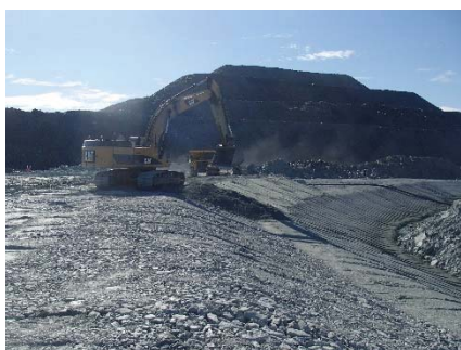
NCIS-104 (2018-07-21), looking SE from Sta. 2+650/-23 m (approx.). Placement of a 0.5 m thick lift of fine filter in the upstream slope from El. 152 m to 154 m with an excavator from Sta. 2+710 m to 2+445 m.
