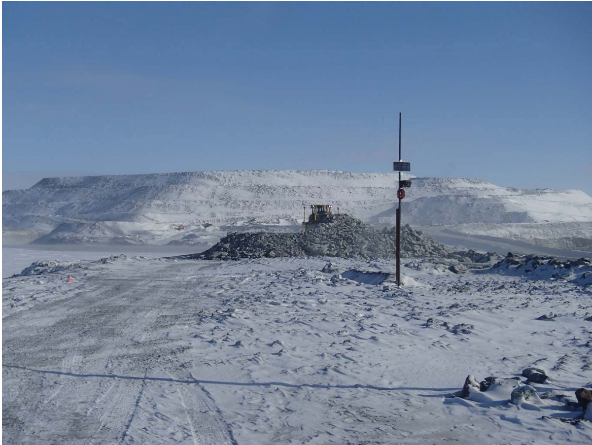
Photograph CD-1809: From Sta. 0+870/-16 m looking N. Placement of a 2 m thick (approx.) lift of intermediate volcanic (IV) rockfill from El. 143 m to El. 145 m from approx. Sta. 0+760 to 0+835 m (o.s. -28 to 3 m).
