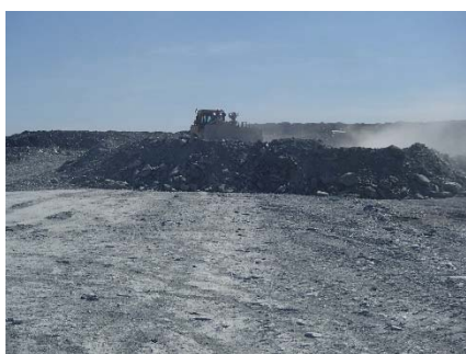
NCIS-098 (2018-07-19), looking E from Sta. 2+040/-9 m (approx.). Placement of a 2 m thick (approx.) lift of UM rockfill from El. 152 m to El. 154 m (approx.) with a dozer from Sta. 2+103 m to 1+984 m (+7 m to -22 m). The material is of good quality and is well graded.
