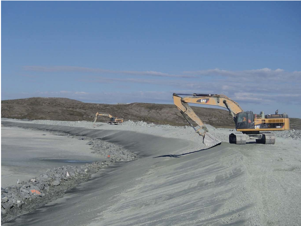
Photograph NCIS-113: From Sta. 2+220/-26 m (approx.), looking SW. Profiling of the upstream slope (3H:1V) from El. 152 to 154 m with an excavator from Sta. 2+000 m to 1+185 m and placement of a 0.5 m thick lift of fine filter in the upstream slope from El. 152 m to 154 m with an excavator from Sta. 2+300 m to 2+090 m.
