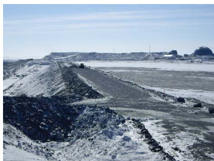
CD-1799 (2018-04-24), looking S from Sta. 0+080/-25 m. Placement a 2 m thick (approx.) lift of intermediate volcanic rockfill from El. 143 m to El. 145 m from 0+340 to 0+435 m (o.s. -28 to -18 m).
