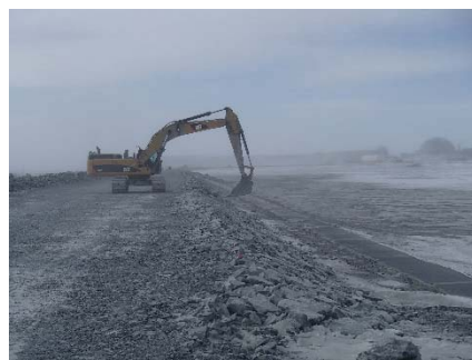
CD-1816 (2018-05-02), looking S from Sta. 0+175/-27 m. Profiling of the upstream slope (2H:1V) from El. 143 to 145 m with an excavator between Sta. 0+175 and 0+560 m.
