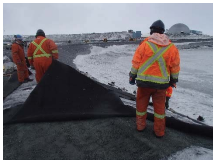
CD-1868 (2018-05-27), looking S from Sta. 0+915/-24 m. Removal of the wet geotextile in place from Sta. 0+935 m to 0+900 m.
