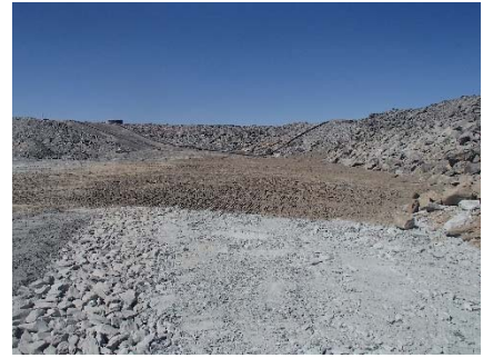
SD3-343 (2018-07-16), looking W from Sta. 20+590/-40 m. View of the depression between SD2 and SD3 backfilled with low quality till up to El. 145 m.
