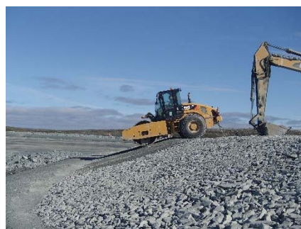
NCIS-105 (2018-07-21), looking NW from Sta. 2+630/-34 m (approx.). Compaction of the 0.5 m lift (approx.) of coarse filter between El. 152 m and 154 m with a 10-tonne smooth-drum compactor with vibration (4 passes) in the upstream slope from Sta. 2+710 m to 2+411 m.
