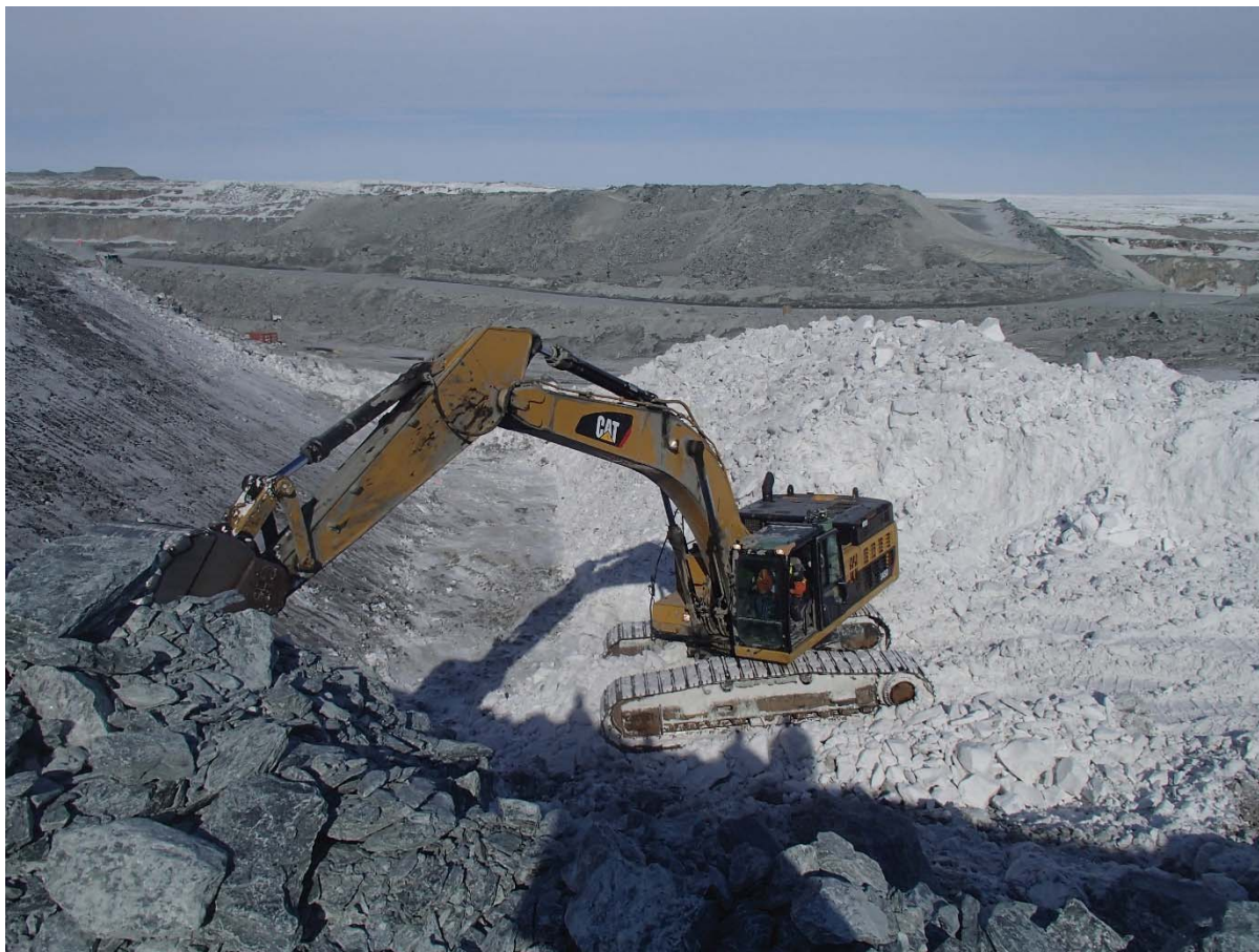
Photograph CD-1803: From Sta. 40+750/27 m looking NE. Removal of snow to expose the foundation bedrock with an excavator between approx. Sta. 40+780 and 40+800 m (o.s. 7 to 10 m).
