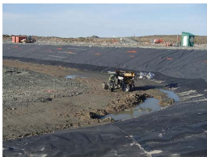
SD3-321 (2018-07-09), looking SW from Sta. 20+610/-56 m. Water ponding at El. 142m on the compacted sieved till layer of the upstream toe liner tie-in at approx. Sta. 20+620 m to 20+630 m was pumped.
