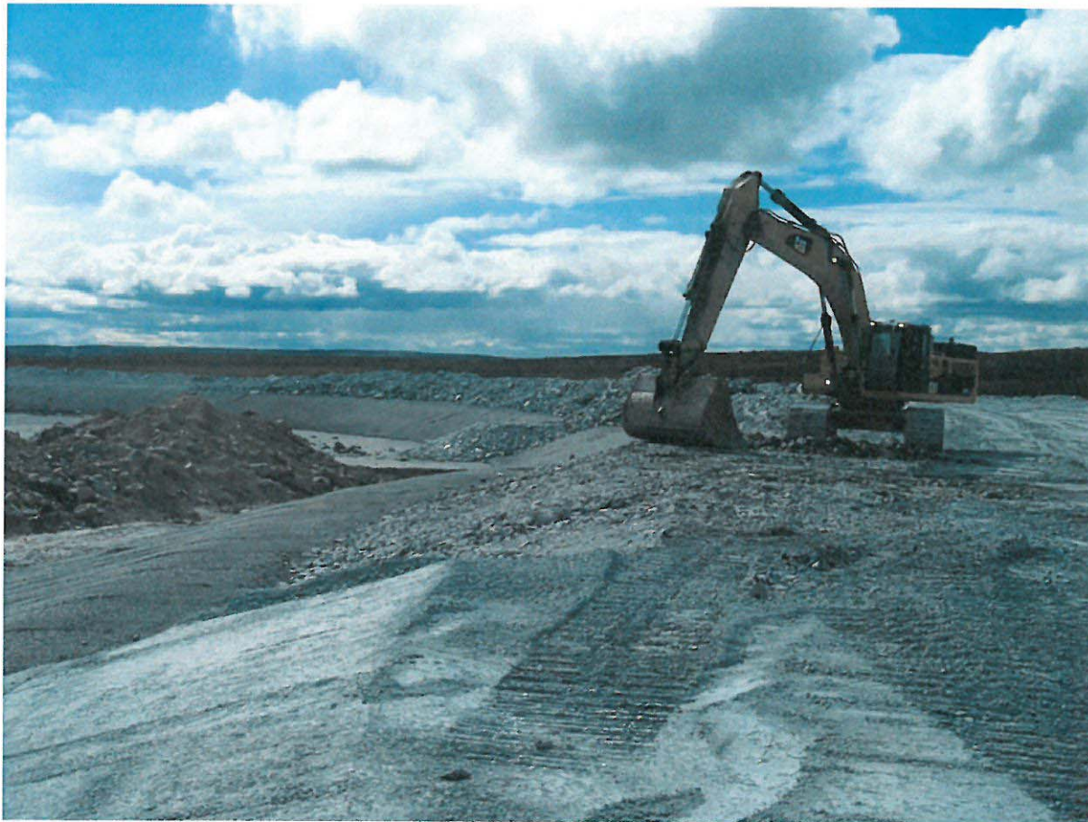
Photograph NCIS-133: From Sta. 1+820/-28 m (approx.), looking W. Placement of a 0.5 m thick lift of coarse filter in the upstream slope from El. 152 m to 154 m with an excavator from Sta. 1+890 m to 1+826 m.
