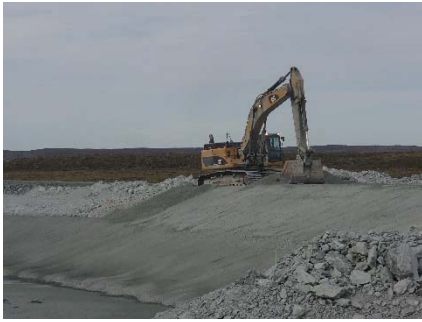
NCIS-136 (2018-07-31), looking SW from Sta. 1+800/-33 m (approx.). Placement of a 0.5 m thick lift of fine filter in the upstream slope from El. 152 m to 154 m with an excavator from Sta. 1+700 m to 1+660 m.
