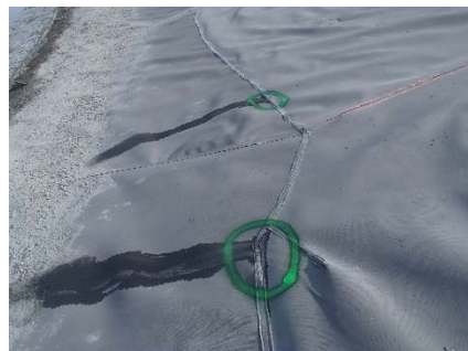
CD-1891 (2018-06-05), looking NE from Sta. 0+960/-28 m. View of leaking extrusion fillet seams before their repair on panel 816 and 818.
