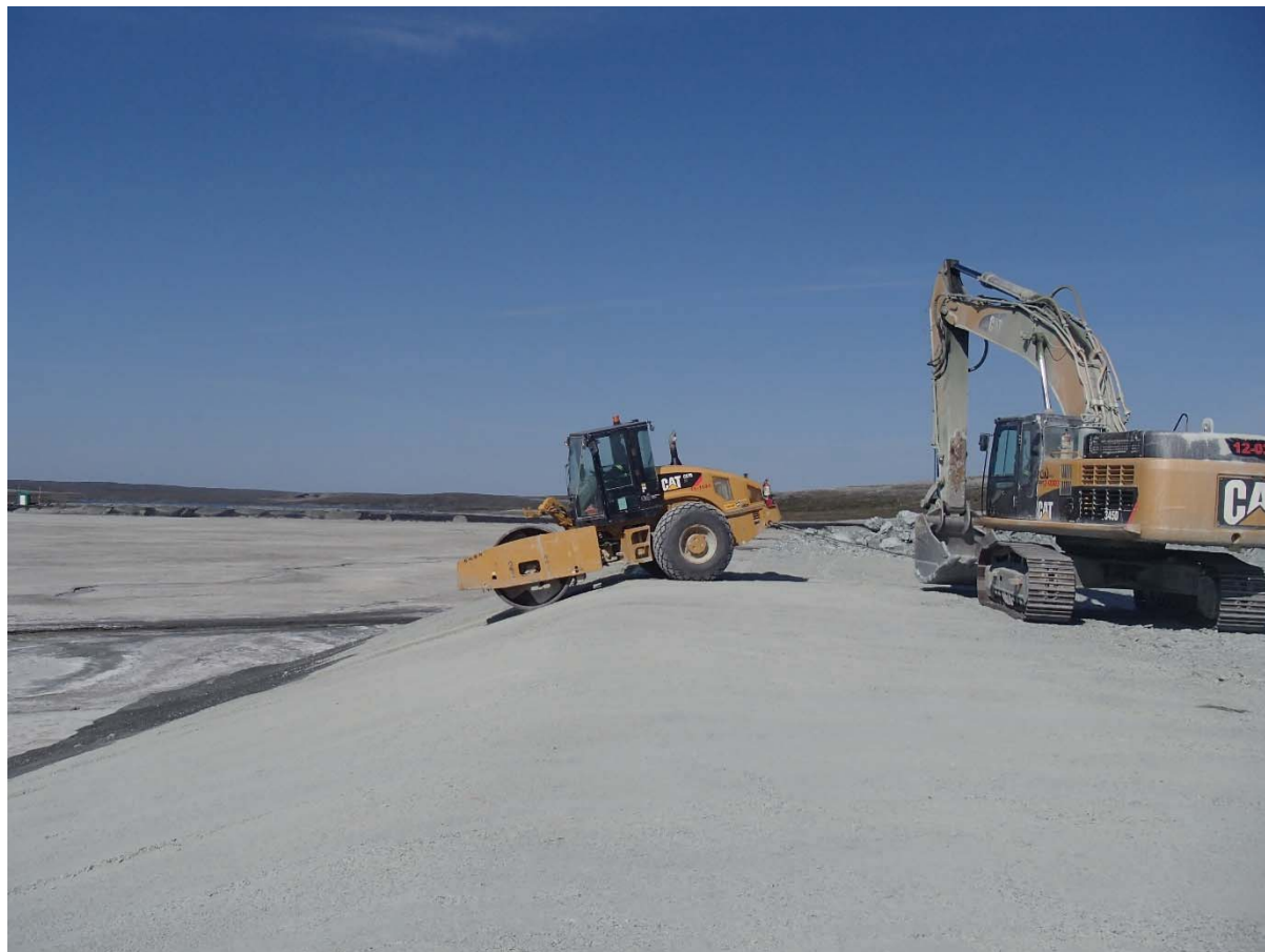
Photograph NCIS-126: From Sta. 1+140/-98 m (approx.), looking W. Compaction of the 0.5 m lift (approx.) of coarse filter between El. 150 m and 152 m with a 10-tonne smooth-drum compactor with vibration (4 passes) in the upstream slope from Sta. 1+240 m to 1+100 m.
