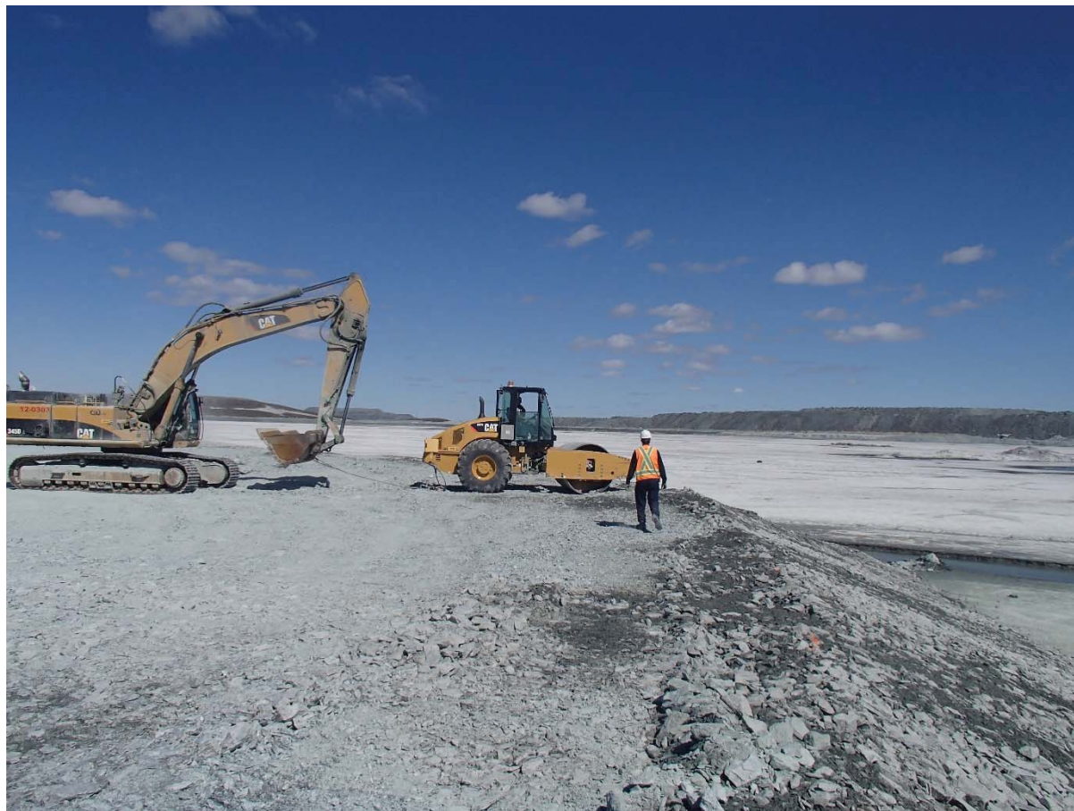
Photograph NCIS-065: From Sta. 1+140/-96 m (approx.), looking NE. Compaction of the 0.5 m lift of coarse filter between El. 148 and 152 m with a 10-tonne smooth-drum compactor with vibration (4 passes) in the upstream slope from Sta. 1+270 m to 1+100 m.
