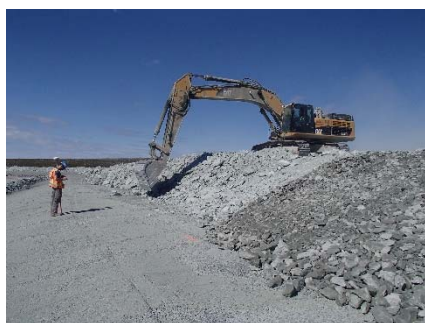
NCIS-103 (2018-07-20), looking NE from Sta. 2+420/-27 m (approx.). Profiling of the upstream slope (3H:1V) from El. 152 to 154 m with an excavator from Sta. 2+400 m to 2+410 m. Oversize boulders were removed.
