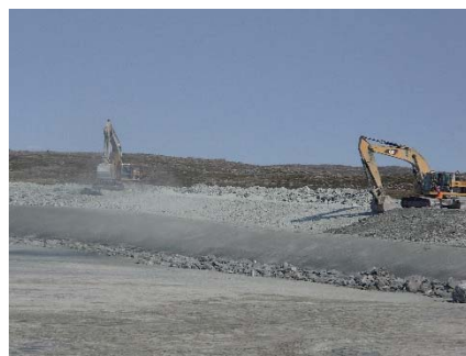
NCIS-111 (2018-07-23), looking NW from Sta. 2+320/-22 m (approx.). Profiling of the upstream slope (3H:1V) from El. 152 to 154 m with an excavator from Sta. 2+159 m to 2+000 m and placement of a 0.5 m thick lift of coarse filter in the upstream slope from El. 152 m to 154 m with an excavator from Sta. 2+293 m to 2+080 m.
