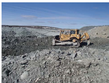
NCIS-049 (2018-06-26), looking N from Sta. 2+870/-28 m. Removing of UM rockfill material from the capping with a dozer to level the surface to El. 150 m from Sta. 2+760 m to 2+850 m (o.s. -29 to -17 m).
