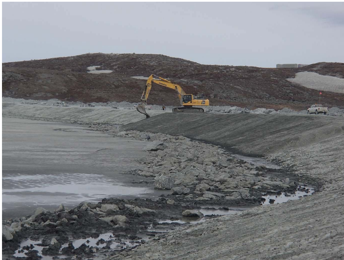
Photograph NCIS-040: From Sta. 2+185/-25 m (approx.), looking W. Placement of a 0.5 m thick lift of fine filter over the coarse filter in the upstream slope from El. 150 m to 152 m with an excavator from Sta. 2+305 m to 2+460 m and from Sta. 1+980 m to 1+835 m.
