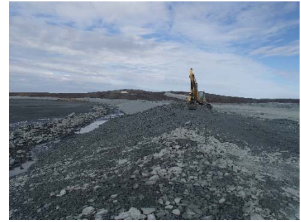
NCIS-030 (2018-06-20), looking W from Sta. 2+140/-29 m. Placement of a 0.5 m thick lift of coarse filter in the upstream slope from El. 150 m to 152 m with an excavator from Sta. 2+105 m to 1+930 m. Notice the presence of water ponding at the bottom of the slope.
