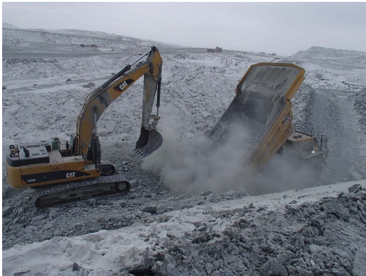
Photograph CD-1811: From Sta. 0+985/-11 m looking SE. Placement the second, third, fourth and fifth 1 m thick (approx.) lifts of intermediate volcanic (IV) rockfill from approx. Sta. 0+985 to 40+780 m (o.s. -8 to 8 m) with the excavator.
