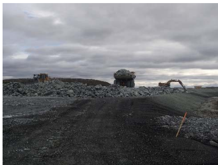
NCIS-128 (2018-07-28), looking NE from Sta. 1+680/-42 m (approx.). Placement of a 2 m thick (approx.) lift of UM rockfill from El. 152 m to El. 154 m (approx.) with a dozer from Sta. 1+830 m to 1+660 m (+8 m to -31 m) and profiling of the upstream slope (3H:1V) from El. 152 to 154 m with an excavator from Sta. 1+880 m to 1+780 m.
