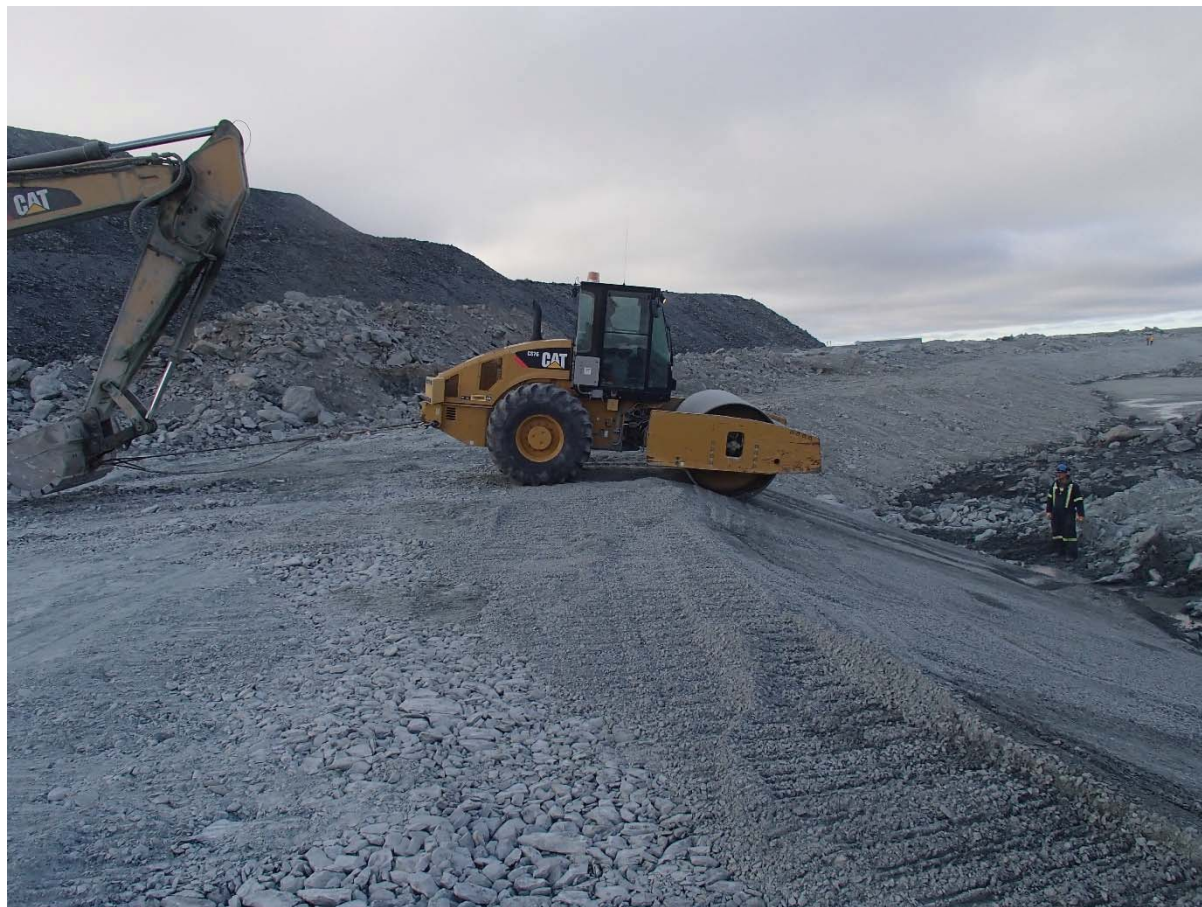
Photograph NCIS-074: From Sta. 2+750/-37 m (approx.), looking SE. Compaction of the 0.5 m lift (approx.) of fine filter between El. 150 m and 152 m with a 10-tonne smooth-drum compactor (4 passes) in the upstream slope from Sta. 2+810 m to 2+095 m. Vibration is used except for the first pass down the slope in order to stabilize the material and limit deformation of the lift.
