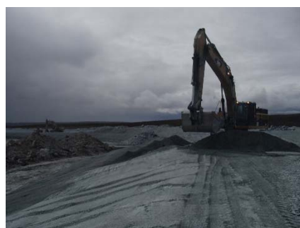
NCIS-135 (2018-07-30), looking SW from Sta. 1+860/-12 m (approx.). Placement of a 0.5 m thick lift of fine filter in the upstream slope from El. 152 m to 154 m with an excavator from Sta. 1+830 m to 1+700 m.
