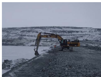
CD-1846 (2018-05-12), looking N from Sta. 0+835/-25 m. Profiling of the upstream slope (2H:1V) from El. 143 to 145 m with an excavator between Sta. 0+330 and 0+600 m and between Sta. 0+715 m and 40+730 m.
