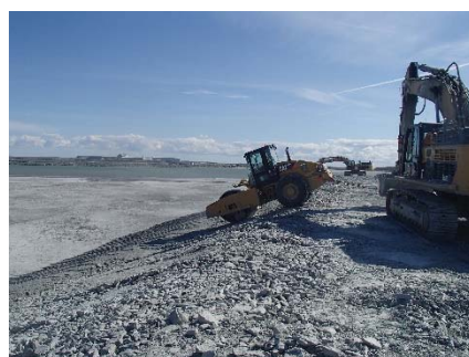
NCIS-099 (2018-07-19), looking SE from Sta. 1+180/-76 m (approx.). Compaction of the 0.5 m lift (approx.) of coarse filter between El. 150 m and 152 m with a 10-tonne smooth-drum compactor with vibration (4 passes) in the upstream slope from Sta. 1+200 m to 1+170 m.
