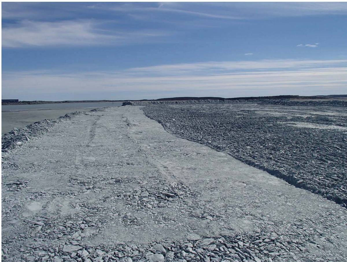
Photograph NCIS-050: From Sta. 1+230/-55 m (approx.), looking S. Compaction of the 1.5 to 2 m lift (approx.) of ultramafic (UM) rockfill at El. 150 m with a 10-tonne smooth-drum compactor with vibration (6 passes) between the haul truck traffic lane and the upstream slope from Sta. 1+220 to 1+130 m (offset -91 to -44 m).
