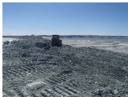
NCIS-057 (2018-06-28), looking SW from Sta. 3+010/-15 m. Removing of UM rockfill material from the capping with a dozer to level the surface to El. 152 m from Sta. 2+980 m to 3+050 m (o.s. -30 to -20 m).
