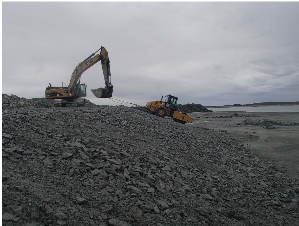
Photograph NCIS-080: From Sta. 2+800/-38 m (approx.), looking S. Compaction of the 0.5 m lift (approx.) of coarse filter between El. 150 and 152 m with a 10-tonne smooth-drum compactor (4 passes) in the upstream slope from Sta. 2+925 m to 3+160 m and from Sta. 1+300 m to 1+200 m.
