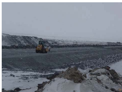
CD-1847 (2018-05-12), looking SE from Sta. 0+085/-48 m. Compaction of the fourth 0.5 m lift (approx.) of fine and coarse filters material at El. 145 m with a 10-tonne smooth-drum compactor with vibration (4 passes) from Sta 0+170 m to 0+930 m.
