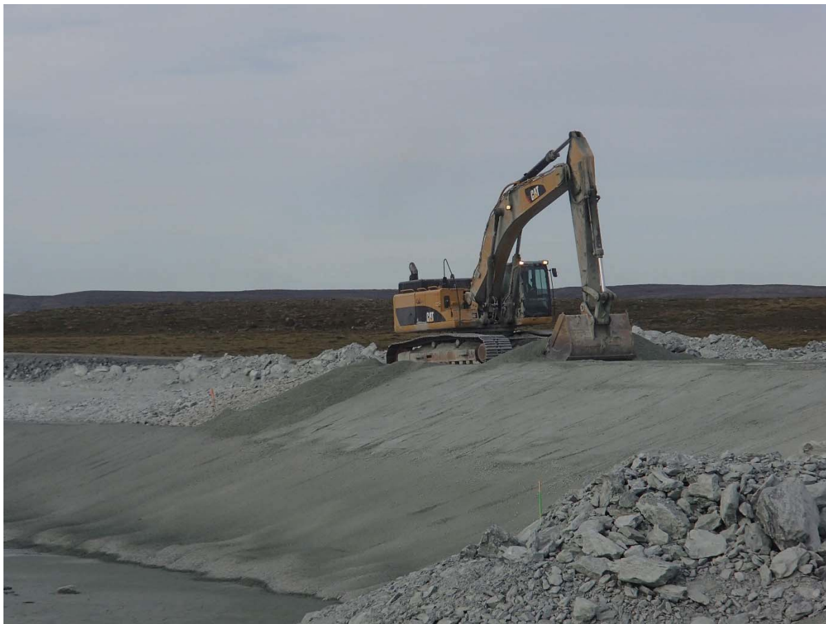
Photograph NCIS-136: From Sta. 1+800/-33 m (approx.), looking SW. Placement of a 0.5 m thick lift of fine filter in the upstream slope from El. 152 m to 154 m with an excavator from Sta. 1+700 m to 1+660 m.
