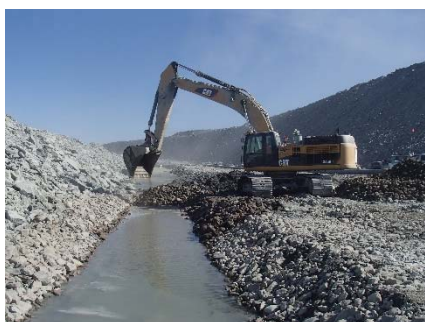
NCIS-125 (2018-07-27), looking NE from Sta. 3+050/+26 m (approx.). Corrections to the north sump: removal of approx. 0.5 m of tailing and till sieving reject material on the bottom of the excavation. The erosion protection material was replaced.
