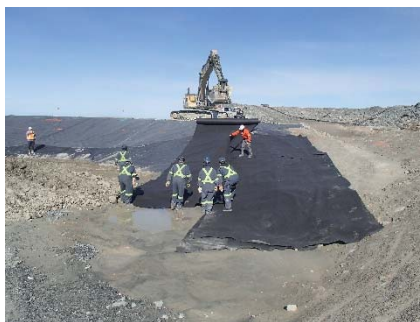
SD3-322 (2018-07-09), looking W from Sta. 20+625/-63 m. Installation of two layers of geotextile on the upstream slope 3H:1V between El. 142 m and 143 m (approx.) from Sta. 20+610 m to 20+800 m.
