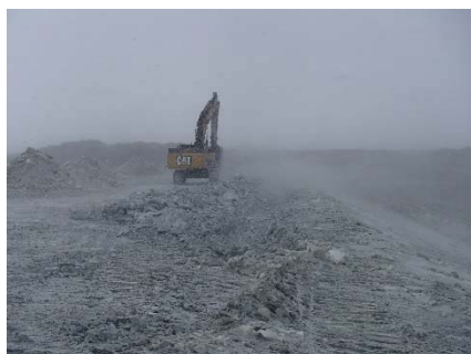
SD3-300 (2018-05-16), looking NW from Sta. 20+790/-33 m. Excavation of the LLDPE geomembrane crest anchoring trench with an excavator from Sta. 20+675 m to 20+780 m.
