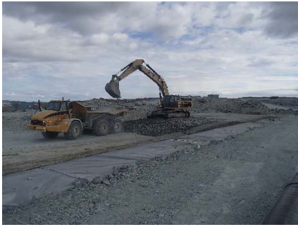
SD3-350 (2018-07-18), looking SE from Sta. 20+740/-24 m. Placement of a 0.5 m thick lift of coarse filter on the top of 0.5 m lift of low quality till (0-150 mm) the fine filter on the upstream toe liner at El. 143.5 m with an excavator from Sta. 20+777 m to 20+807 m.
