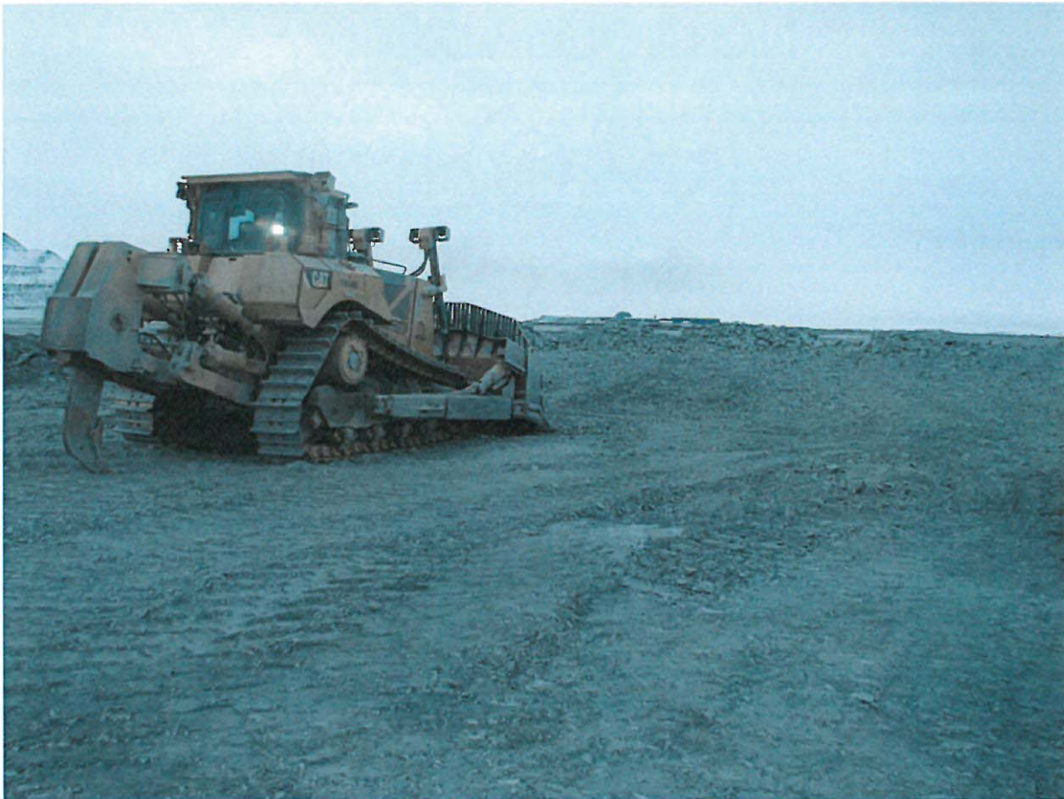
Photograph NCIS-020: From Sta. 1+570 m (approx.), looking S. Placement of a 2 m thick (approx.) lift of UM rockfill from El. 150 m to El. 152 m (approx.) with a dozer from Sta. 1+564 m to 1+535 m (offset unavailable).
