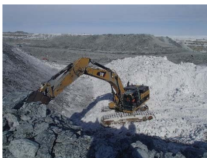
CD-1803 (2018-04-27), looking NE from Sta. 40+750/+27 m. Removal of snow to expose the foundation bedrock with an excavator between approx. Sta. 40+780 and 40+800 m (o.s. 7 to 10 m).
