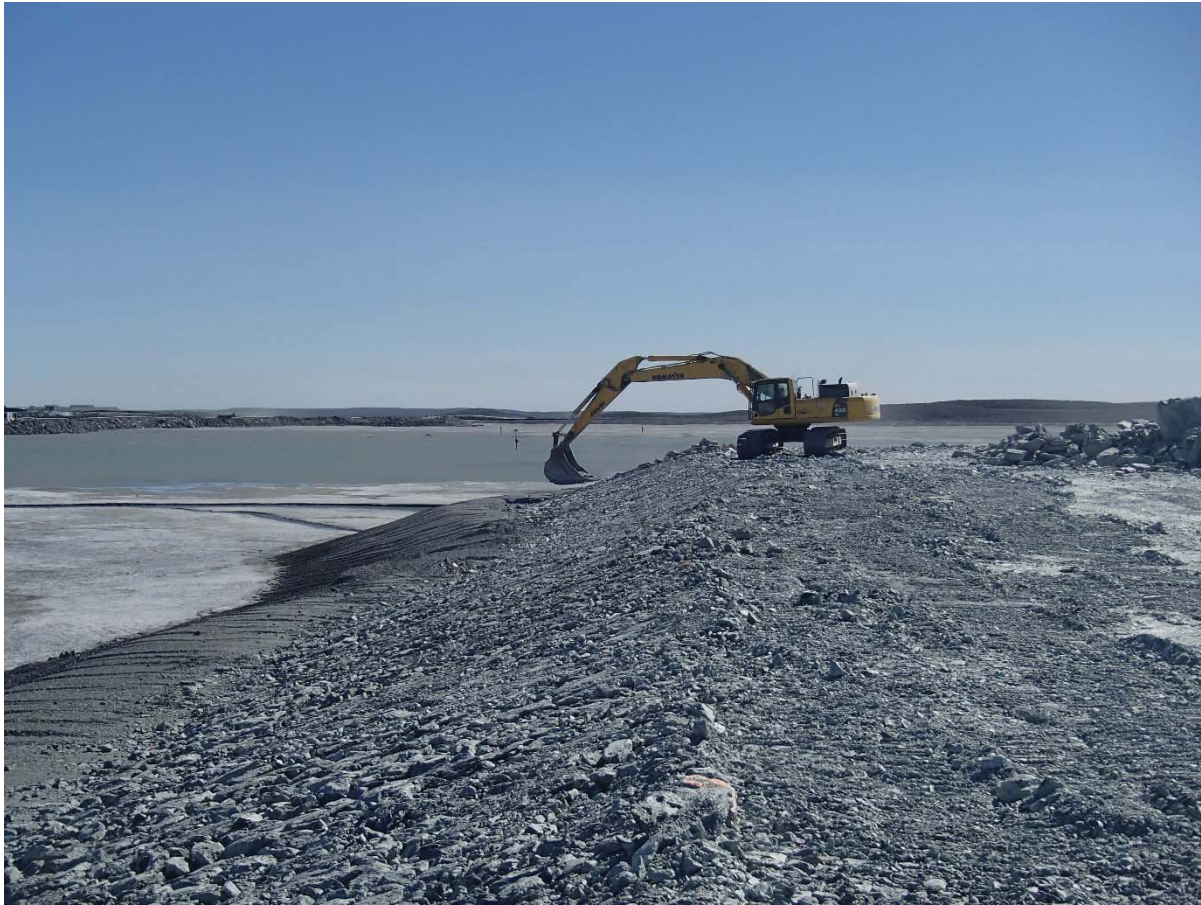
Photograph NCIS-092: From Sta 1+160/-77 m (approx.), looking S. Profiling of the upstream slope (3H:1V) from El. 150 to 152 m with an excavator from Sta. 1+185 m to 1+135 m.
