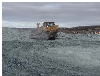
NCIS-048 (2018-06-26), looking SW from Sta. 1+120/-92 m. Placement of a 1.5 to 2 m thick (approx.) lift of UM rockfill from El. 148 m to El. 150 m (approx.) with a dozer from Sta. 1+125 m to 1+115 m (-92 m to -47 m).
