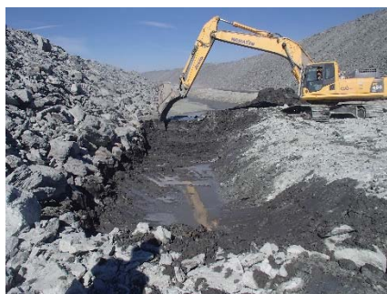
NCIS-115 (2018-07-24), looking NE from Sta. 3+040/-33 m (approx.). Excavation of a 1 m (approx.) sump in the tailings with an excavator from Sta. 3+010 m to 3+030 m (o.s. +27 to +30 m).
