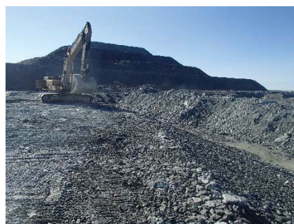
NCIS-051 (2018-06-27), looking SE from Sta. 2+630/-34 m. Placement of a 0.5 m thick lift of coarse filter in the upstream slope from El. 150 m to 152 m with an excavator from Sta. 2+640 m to 2+815 m.
