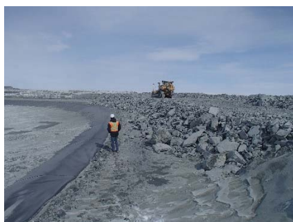
CD-1817 (2018-05-02), looking NE from Sta. 40+700/-10 m. View of the rockfill lift thickness at the junction of Saddle Dam 5 and Central Dike, approx. 2.5 m thick..
