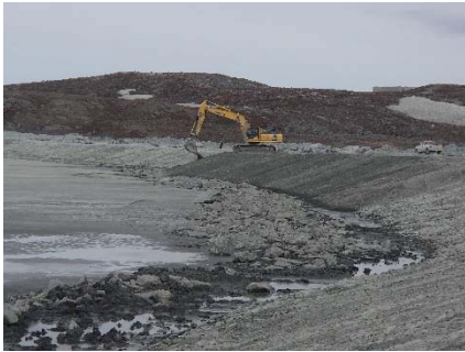
NCIS-040 (2018-06-24), looking W from Sta. 2+185/-25 m. Placement of a 0.5 m thick lift of fine filter over the coarse filter in the upstream slope from El. 150 m to 152 m with an excavator from Sta. 2+305 m to 2+460 m and from Sta. 1+980 m to 1+835 m.
