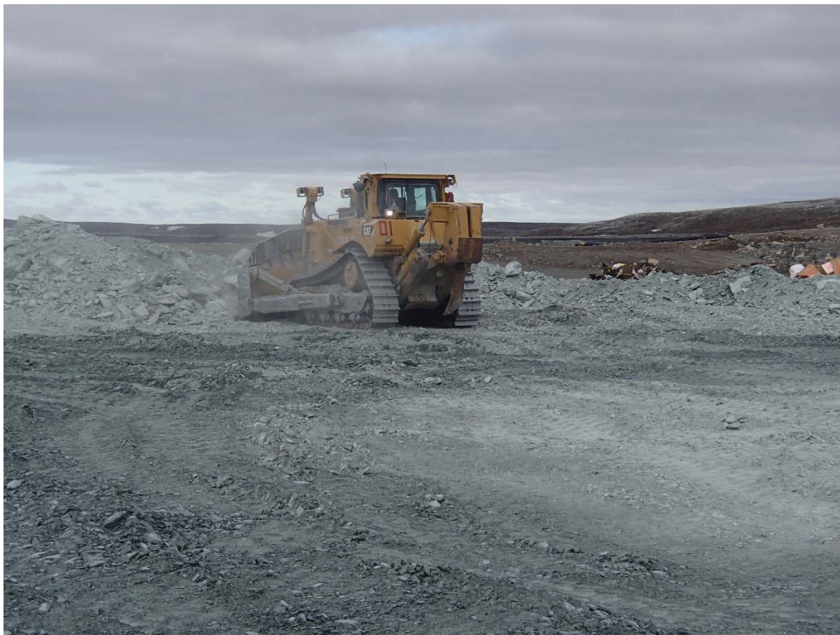
Photograph NCIS-048: From Sta. 1+120/-92 m (approx.), looking SW. Placement of a 1.5 to 2 m thick (approx.) lift of UM rockfill from El. 148 m to El. 150 m (approx.) with a dozer from Sta. 1+125 m to 1+115 m (-92 m to -47 m). The material is of good quality and is well graded.
