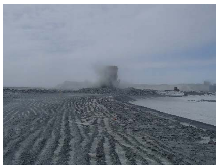
CD-1815 (2018-05-02), looking S from Sta. 0+920/-25 m. Placement of a 2 m thick (approx.) lift of intermediate volcanic (IV) rockfill from El. 143 m to El. 145 m from approx. Sta. 40+740 to 0+980 m (o.s. -28 to -11 m).
