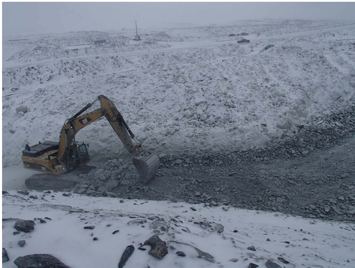
Photograph CD-1808: From Sta. 40+790/-14 m looking E. Placement of a 1.5 m thick (approx.) lift of intermediate volcanic (IV) rockfill from approx. Sta. 40+780 to 40+805 m (o.s. -6 to 9 m).
