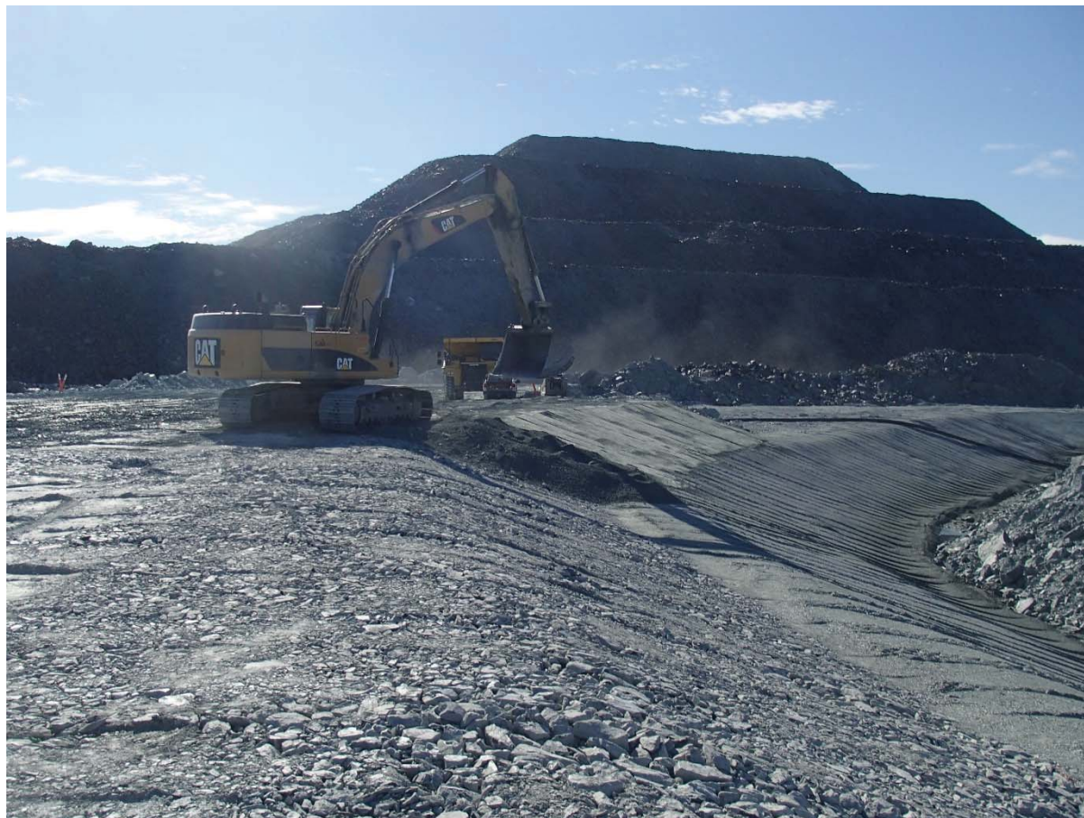
Photograph NCIS-104: From Sta. 2+650/-23 m (approx.), looking SE. Placement of a 0.5 m thick lift of fine filter in the upstream slope from El. 152 m to 154 m with an excavator from Sta. 2+710 m to 2+445 m.
