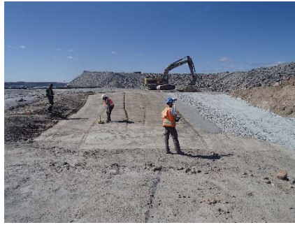
SD3-342 (2018-07-15), looking W from Sta. 20+600/-58 m. View of the compaction test and view of the filling of the depression between SD2 and SD3 with low quality till up to El. 145 m.
