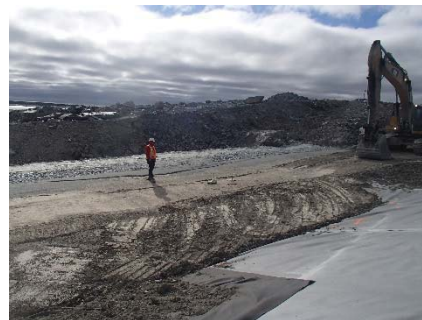
SD3-334 (2018-07-13), looking SE from Sta. 20+780/-26 m. Compaction of the second 0.5 m thick lift of compacted sieved till and third lift of fine filter, coarse filter and fine rockfill of the upstream toe liner tie-in with a 10 tonne smooth-drum compactor with vibrations from Sta. 20+770 m to 20+800 m.
