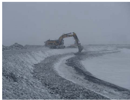
CD-1827 (2018-05-06), looking SW from Sta. 0+940/-16 m. Placement of a 0.5 m thick lift of fine filter from El. 143 m to 143.5 m with an excavator from Sta. 40+730 m to 0+835 m.
