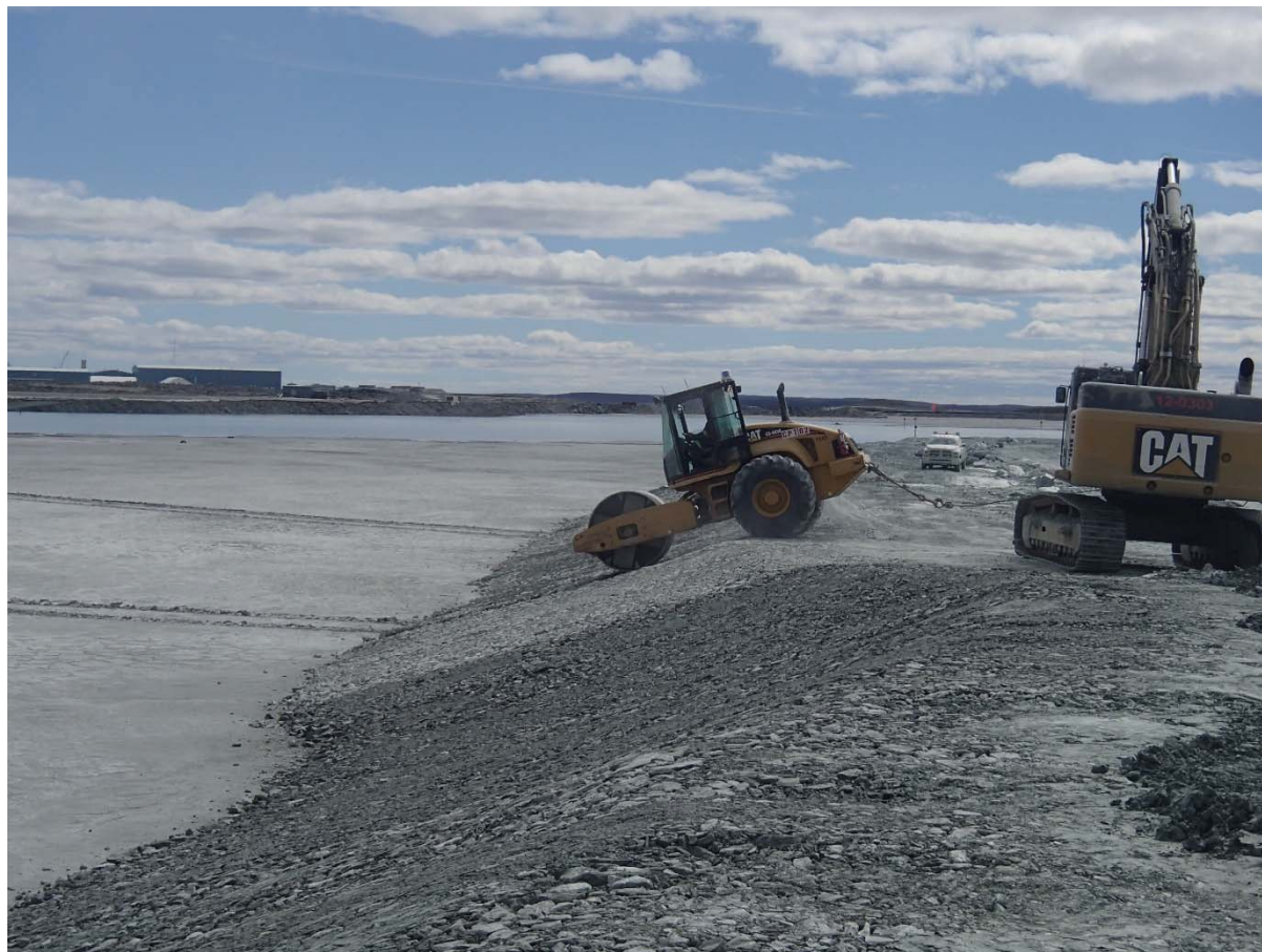
Photograph NCIS-061: From Sta. 1+365/-35 m (approx.), looking S. Compaction of the 0.5 m lift of coarse filter between El. 148 and 152 m with a 10-tonne smooth-drum compactor with vibration (4 passes) in the upstream slope from Sta. 1+340 m to 1+270 m.
