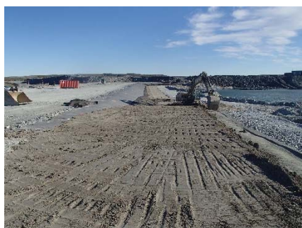
SD3-335 (2018-07-14), looking N from Sta. 20+815/-27 m. Placement of a third 0.5 m thick lift of compacted sieved till on the upstream toe liner tie-in with an excavator from Sta. 20+760 m to 20+810 m.
