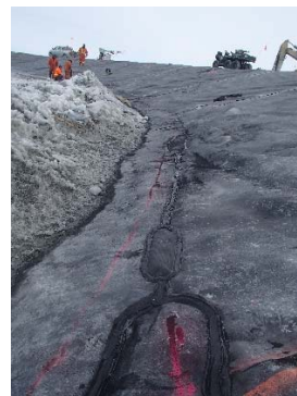
CD-1867 (2018-05-25), looking E from Sta. 40+680/-37 m. View of repair patches on the extrusion weld at the bottom of the panels.
