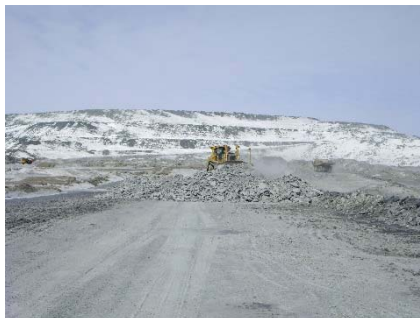
CD-1797 (2018-04-23), looking N from Sta. 0+380/-20 m. Placement a 2 m thick (approx.) lift of intermediate volcanic rockfill from El. 143 m to El. 145 m from 0+250 to 0+400 m (o.s. -28 to -18 m).
