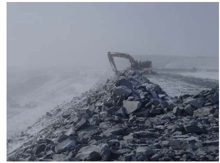
CD-1825 (2018-05-05), looking S from Sta. 0+430/+9 m. Profiling of the downstream slope (1.5H:1V) from El. 143 to 145 m with an excavator between Sta. 0+330 m and 0+440 m and between Sta. 0+530 m and 0+745 m.
