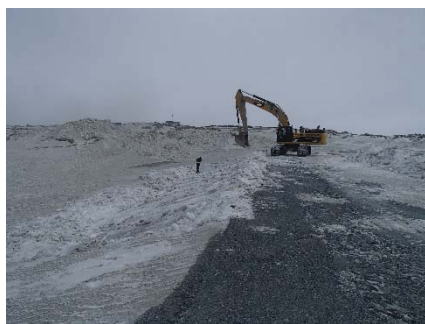
SD3-297 (2018-05-14), looking SE from Sta. 20+730/-10 m. Removal of snow on the upstream slope of SD3 with an excavator, from Sta. 20+640 to 20+760 m.
