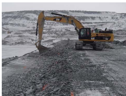
CD-1841 (2018-05-10), looking N from Sta. 0+475/-14 m. Placement of a third 0.5 m thick lift of coarse filter from El. 144 m to 144.5 m with an excavator from Sta. 0+335 m to 40+730 m.
