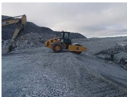
NCIS-074 (2018-07-03), looking SE from Sta. 2+750/-37 m. Compaction of the 0.5 m lift (approx.) of fine filter between El. 150 and 152 m with a 10-tonne smooth-drum compactor (4 passes) in the upstream slope from Sta. 2+810 m to 2+095 m.
