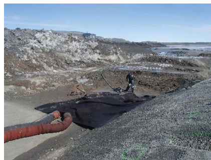
SD3-305 (2018-06-05), looking NE from Sta. 20+590/-48 m. Dewatering of the water ponding on the first compacted sieved till layer of upstream toe liner tie-in. A Genset Frost-fighter is heating the sieved till layer and a pump is evacuating the water.
