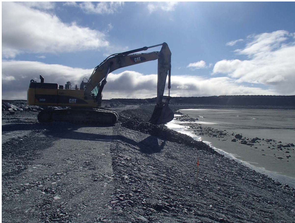
Photograph NCIS-033: From Sta. 1+900/-21 m (approx.), looking E. Placement of a 0.5 m thick lift of coarse filter in the upstream slope from El. 150 m to 152 m with an excavator from Sta. 1+930 m to 1+715 m.
