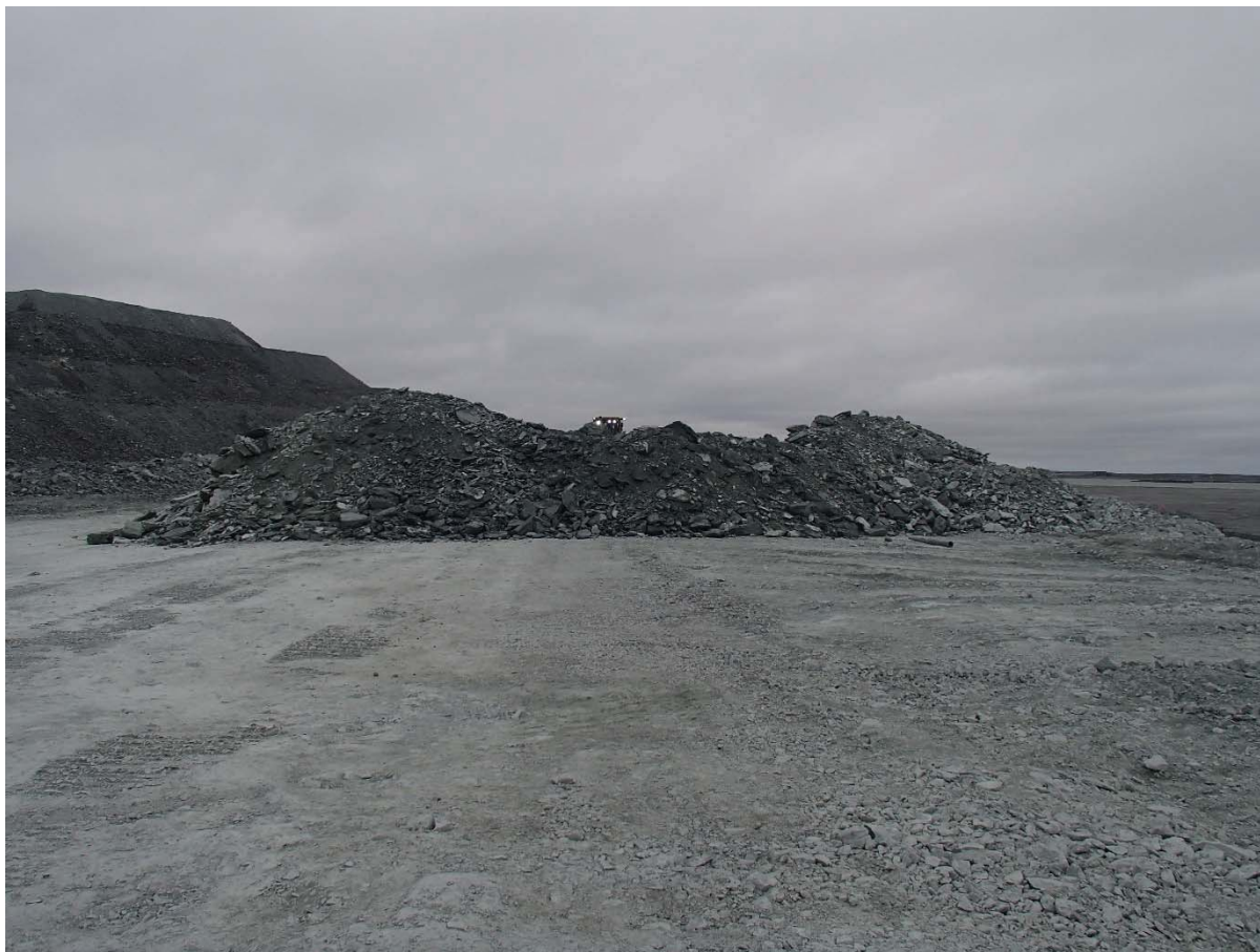
Photograph NCIS-090: From Sta 2+440/-1 m (approx.), looking SE. Placement of a 2 m thick (approx.) lift of UM rockfill from El. 152 m to El. 154 m (approx.) with a dozer from Sta. 2+455 m to 2+370 m (+4 m to -24 m).
