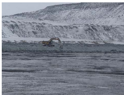
NCIS-010 (2018-05-21). Profiling of the upstream slope (3H:1V) from El. 150 to 152 m with an excavator from Sta. 2+777 m to 2+400 m.
