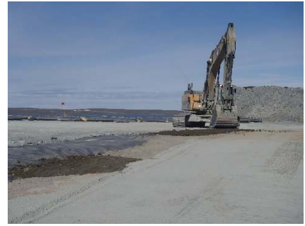
SD3-352 (2018-07-19), looking SW from Sta. 20+600/-59 m. Corrections to the layer of compacted sieved till placed against the upstream slope from Sta. 20+599 m to 20+613 m.
