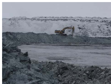
NCIS-012 (2018-05-22), looking NW from Sta. 2+000 m. Profiling of the upstream slope (3H:1V) from El. 150 to 152 m with an excavator from Sta. 2+325 m to 2+275 m (approx.).
