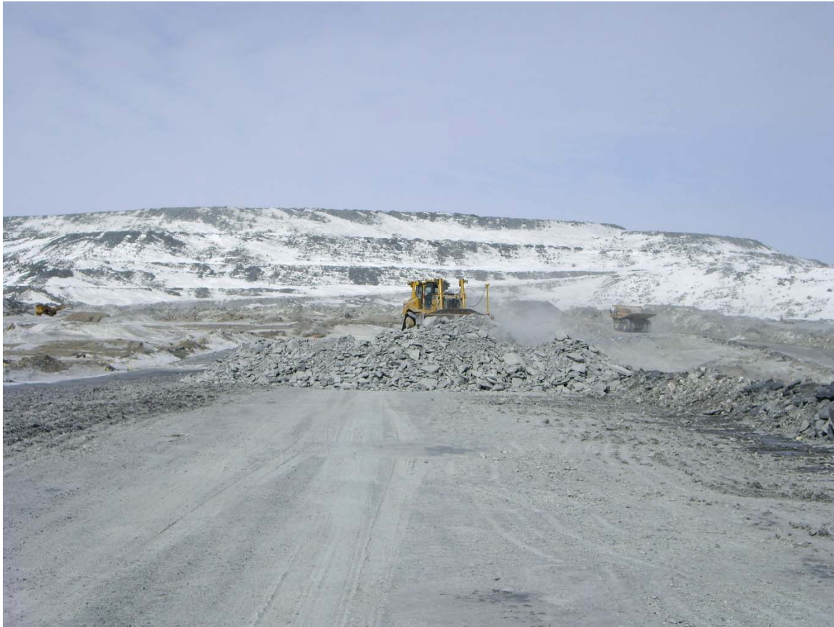
Photograph CD-1797: From Sta. 0+320/-20 m, looking N. Placement of a 2 m thick (approx.) lift of intermediate volcanic (IV) rockfill from El. 143 m to El. 145 m from 0+250 to 0+400 m (o.s. -28 to -18 m).
