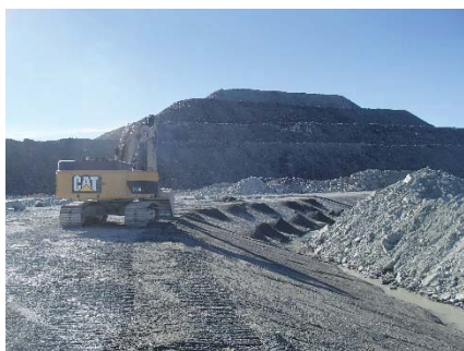
NCIS-071 (2018-07-02), looking SE from Sta. 2+670/-28 m. Placement of a 0.5 m thick lift of fine filter over the coarse filter in the upstream slope from El. 150 m to 152 m with an excavator from Sta. 1+550 m to 1+320 m and 1+630 m to 1+610 m.
