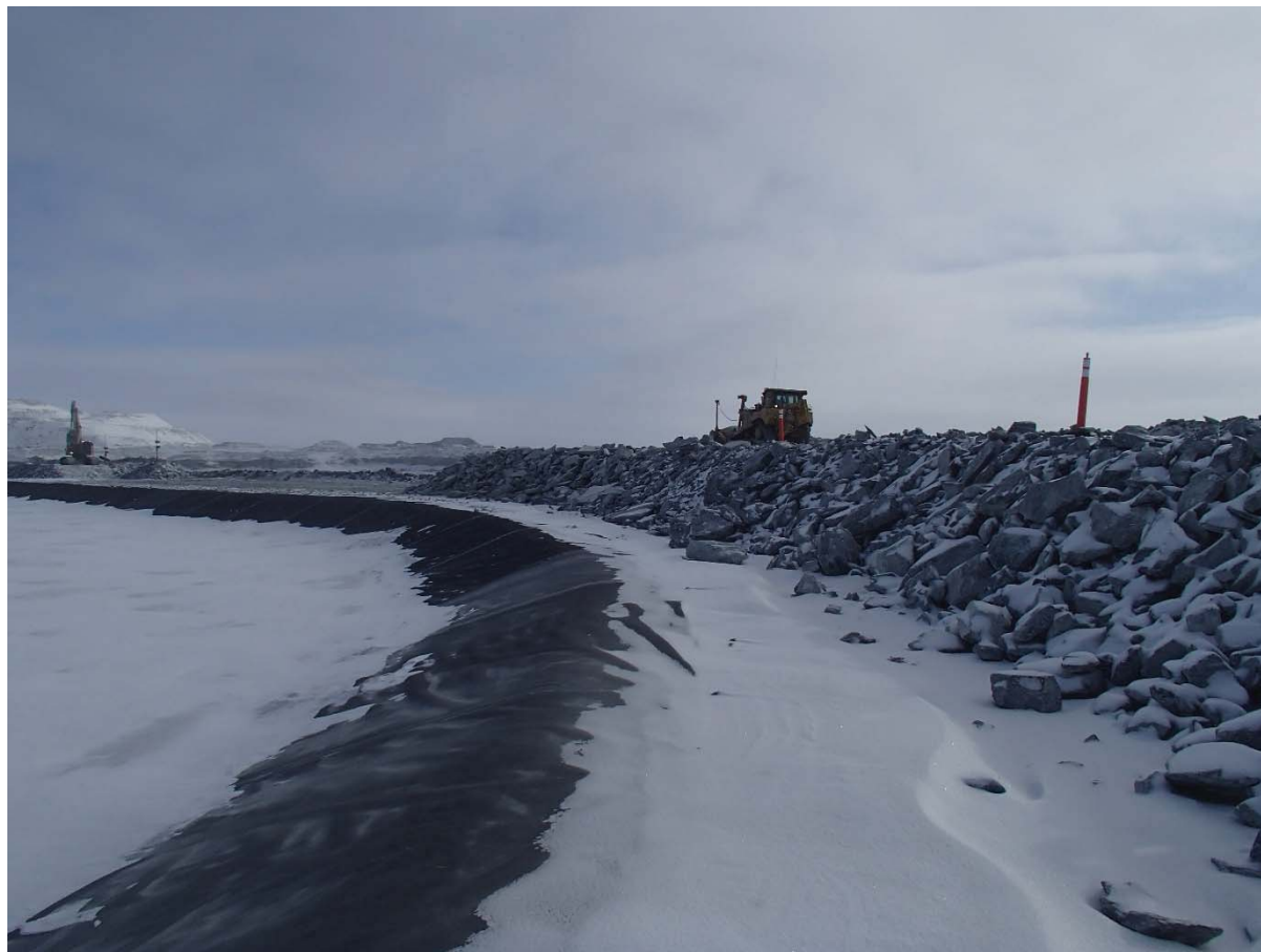
Photograph CD-1818: From Sta. 40+770/-25, looking NE. Placement of a 2 m thick (approx.) lift of intermediate volcanic (IV) rockfill from El. 143 m to El. 145 m from approx. Sta. 0+980 m to 0+880 m (o.s. -28 to -11 m).
