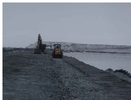
CD-1843 (2018-05-10), looking S from Sta. 0+460/-23 m. Compaction of the third 0.5 m lift (approx.) of fine and coarse filters material at El. 144.5 m with a 10-tonne smooth-drum compactor with vibration (4 passes) from Sta 0+335m to 0+900 m.
