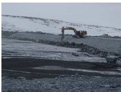
NCIS-017 (2018-05-24), looking SW from Sta. 2+290 m. Profiling of the upstream slope (3H:1V) from El. 150 to 152 m with an excavator from Sta. 2+138 m to 1+989 m.
