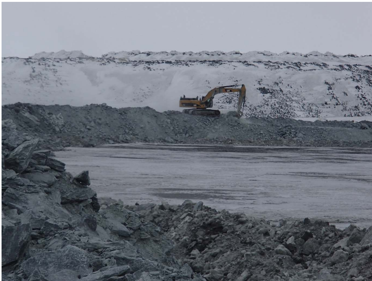
Photograph NCIS-012: From Sta. 2+000 m (approx.), looking NW. Profiling of the upstream slope (3H:1V) from El. 150 to 152 m with an excavator from Sta. 2+325 m to 2+275 m (approx.).
