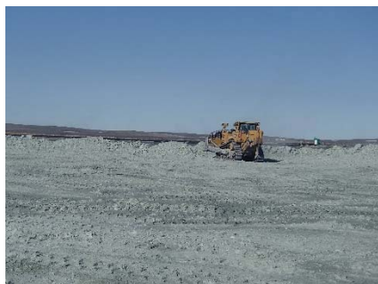
NCIS-052 (2018-06-27), looking SW from Sta. 1+120/-87 m. Placement of a 1.5 to 2 m thick (approx.) lift of UM rockfill from El. 148 m to El. 150 m (approx.) with a dozer from Sta. 1+115 m to 1+100 m (-107 m to -45 m).
