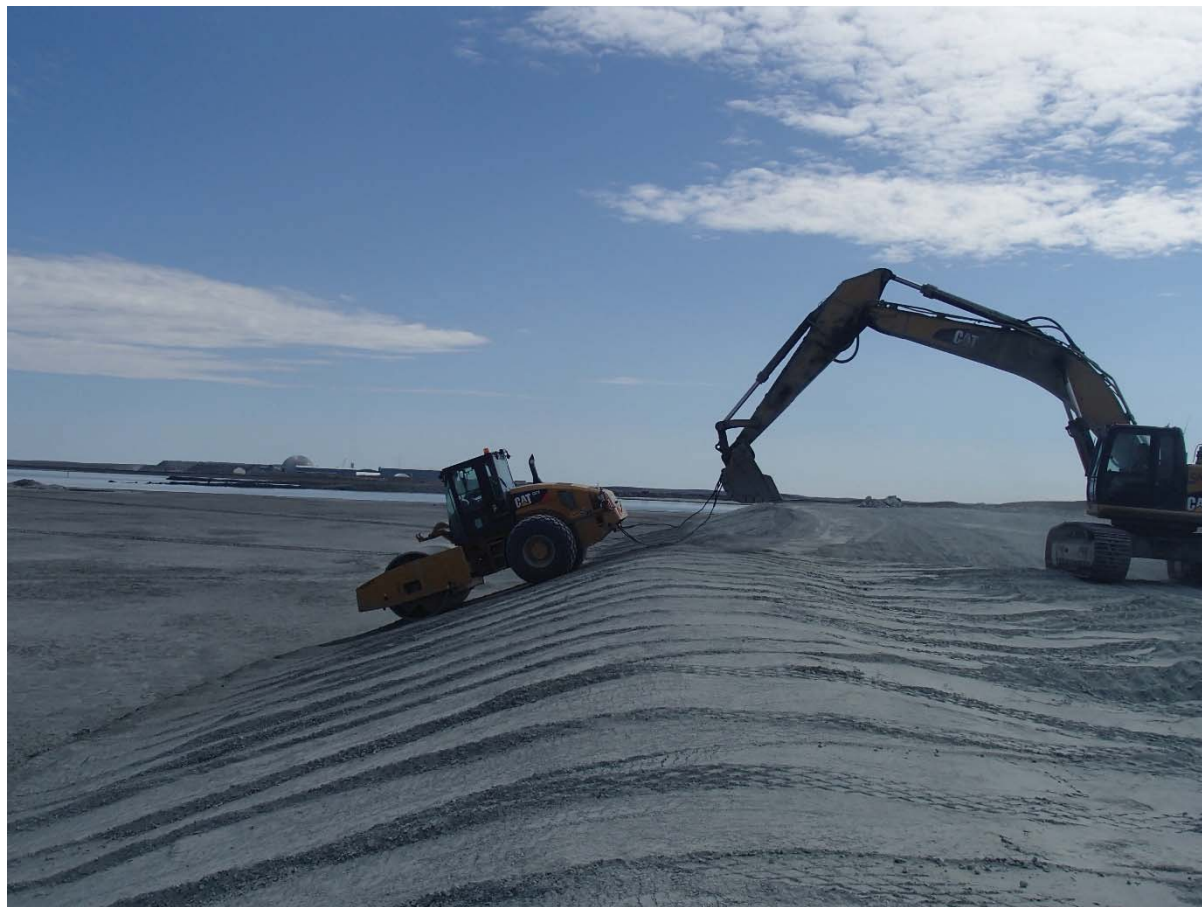
Photograph NCIS-107: From Sta. 1+380/-38 m (approx.), looking S. Compaction of the 0.5 m lift (approx.) of fine filter between El. 150 m and 152 m with a 10-tonne smooth-drum compactor with vibration (4 passes) in the upstream slope from Sta. 1+251 m to 1+1+660 m.
