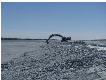
NCIS-056 (2018-06-28), looking S from Sta. 1+290/-39 m. Profiling of the upstream slope (3H:1V) from El. 148 to 150 m with an excavator from Sta. 1+340 m to 1+130 m.
