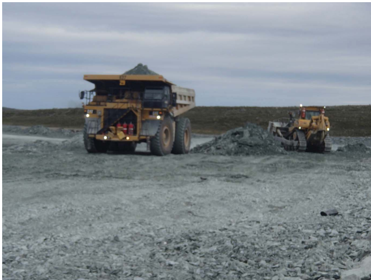
Photograph NCIS-096: From Sta 2+355/+9 m (approx.), looking N. Placement of a 2 m thick (approx.) lift of UM rockfill from El. 152 m to El. 154 m (approx.) with a dozer from Sta. 2+190 m to 2+103 m (+7 m to -22 m). The material is of good quality and is well graded.
