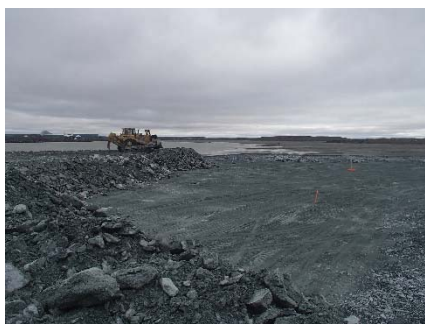
NCIS-083 (2018-07-07), looking SW from Sta. 1+140/52 m. Placement of a 2 m thick (approx.) lift of IV rockfill from El. 150 m to El. 152 m (approx.) with a dozer from Sta. 1+160 m to 1+170 m (-64 m to -111 m).
