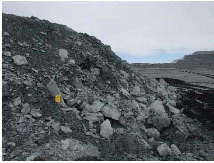
NCIS-028 (2018-06-09), looking E from Sta. 1+340/+3 m. View of the UM rockfill lift approximately 3.2 m thick.
