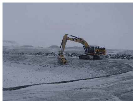
CD-1849 (2018-05-13), looking NE from Sta. 40+750/-17 m. Final rolling of the upstream slope in view of the LLDPE geomembrane installation from Sta. 0+170 m to 40+730 m.
