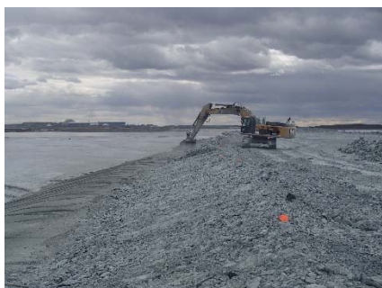
NCIS-077 (2018-07-04), looking S from Sta. 1+310/-32 m. Profiling of the upstream slope (3H:1V) from El. 150 m to 152 m with an excavator from Sta. 1+300 m to 1+175 m and from 3+070 m to 3+160 m.
