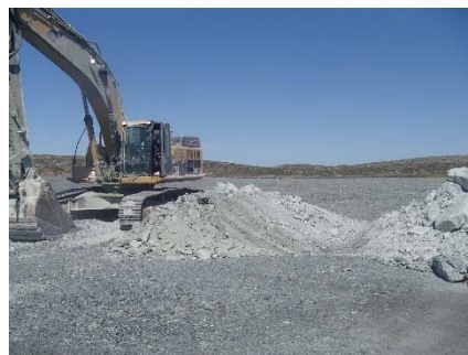
NCIS-114 (2018-07-24), looking N from Sta. 1+700/-34 m (approx.). Excavation of a 0.8 m (approx.) deep, 1 m wide shallow ditch in the rockfill capping with an excavator from Sta. 1+500 m to 1+650 m.
