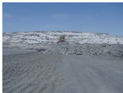
CD-1801 (2018-04-26), looking N from Sta. 0+650/-10 m. Placement a 2 m thick (approx.) lift of intermediate volcanic (IV) rockfill from El. 143 m to El. 145 m from 0+535 to 0+625m (o.s. -28 to -18 m).
