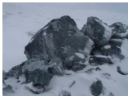
NCIS-006 (2018-05-19). View of oversize boulders on the UM rockfill lift at El. 152 m.
