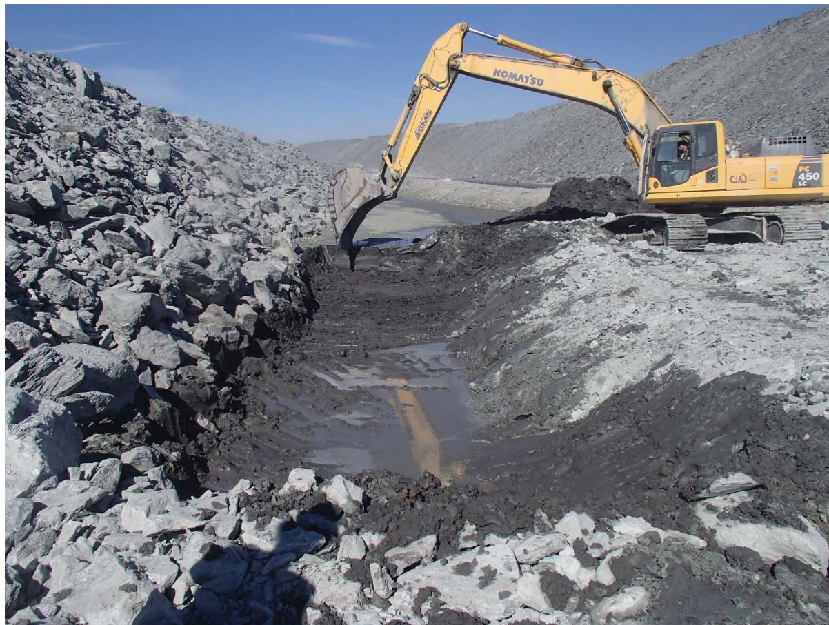
Photograph NCIS-115: From Sta. 3+040/-33 m (approx.), looking NE. Excavation of a 1 m (approx.) sump in the tailings with an excavator from Sta. 3+010 m to 3+030 m (o.s. +27 to +30 m). The bottom of the excavation was frozen.
