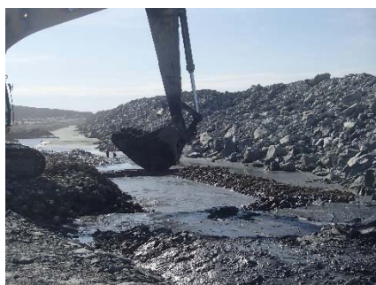
NCIS-124 (2018-07-27), looking S from Sta. 3+340/+33 m (approx.). Placement of a 0.3 m thick (approx.) layer of till sieving reject material on the bottom and on the slopes of the south sump.
