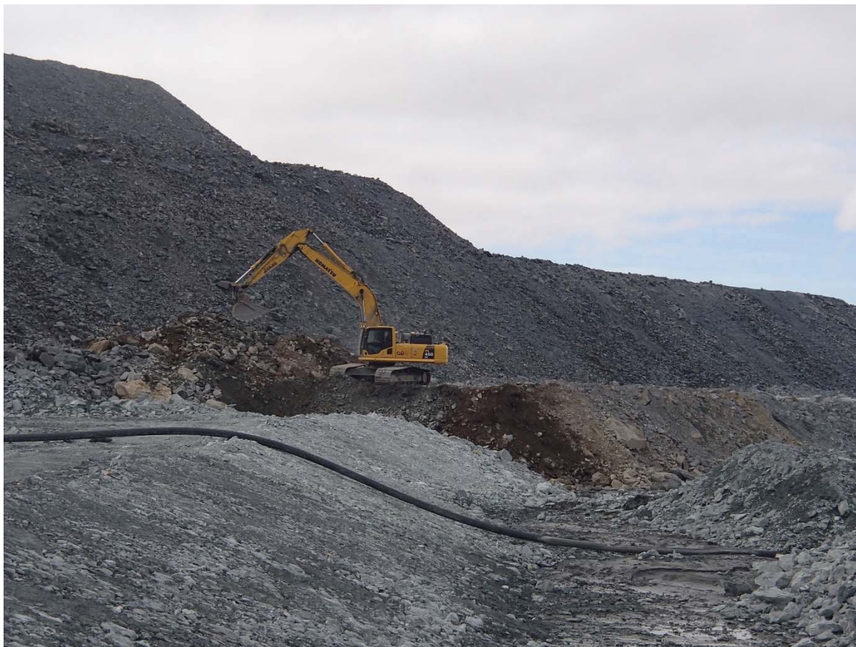
Photograph NCIS-046: From Sta. 2+680/-18 m (approx.), looking SE. Removal of till material mixed with the UM rockfill of the capping (about 1 to 2 m thick along the slope) with an excavator from Sta. 2+760 m to 2+850 m (offset -35 to -17 m).
