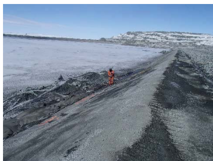
CD-1856 (2018-05-18), looking N from Sta. 0+670/-24 m. Clean-up of the fine filter placed against the slope at the deposition finger at approx. Sta. 0+670 m with pressurized air stream to expose 1 m of LLDPE liner, in preparation for the new liner installation.
