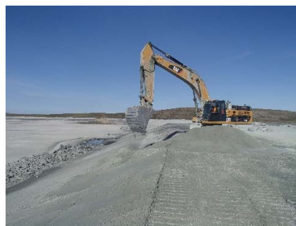
NCIS-117 (2018-07-25), looking SW from Sta. 2+050/-25 m (approx.). Placement of a 0.5 m thick lift of fine filter in the upstream slope from El. 152 m to 154 m with an excavator from Sta. 2+090 m to 1+890 m.
