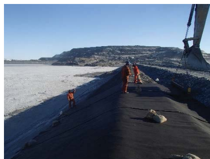
CD-1885 (2018-06-03), looking N from Sta. 0+460/-26 m. Installation of the geotextile on the upstream slope 2H:1V between El. 143 m and 145 m from Sta. 0+480 m to 0+320 m. compactor with vibration (4 passes) from Sta. 0+610 to 0+480 m.
