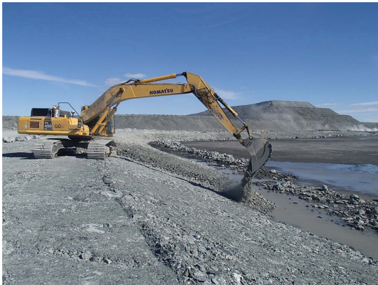
Photograph NCIS-029: From Sta. 2+120/-27 m (approx.), looking SE. Placement of a 0.5 m thick lift of coarse filter in the upstream slope from El. 150 m to 152 m with an excavator from Sta. 2+280 m to 2+105 m.
