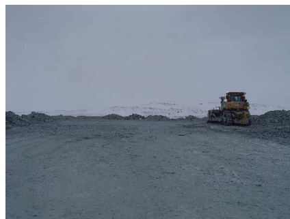
NCIS-009 (2018-05-21). Placement a 2 m thick (approx.) lift of UM rockfill from El. 150 m to El. 152 m (approx.) with a dozer from Sta. 1+880 m to 1+825 m (o.s. unavailable).
