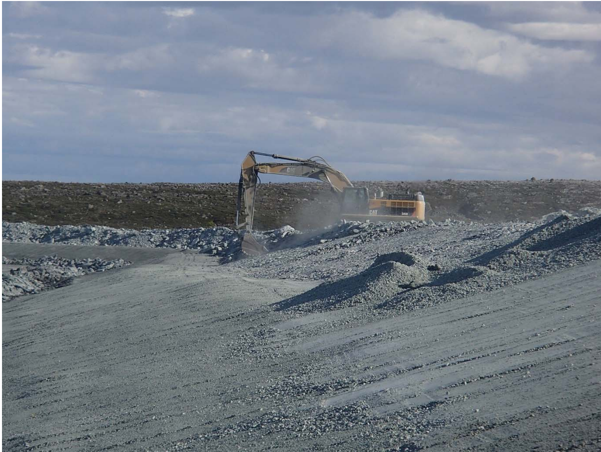
Photograph NCIS-108: From Sta. 2+490/-32 m (approx.), looking N. Profiling of the upstream slope (3H:1V) from El. 152 to 154 m with an excavator from Sta. 2+159 m to 2+409 m.
