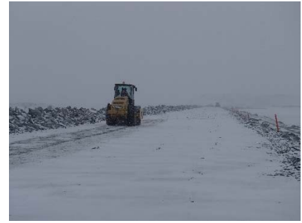
CD-1807 (2018-04-28), looking S from Sta. 0+200/-15 m. Compaction of the 2 m lift (approx.) of IV rockfill with a 10-tonne smooth-drum compactor with vibration (6 passes) from Sta. 0+150 to 0+280 m (o.s. -21 to 11 m).
