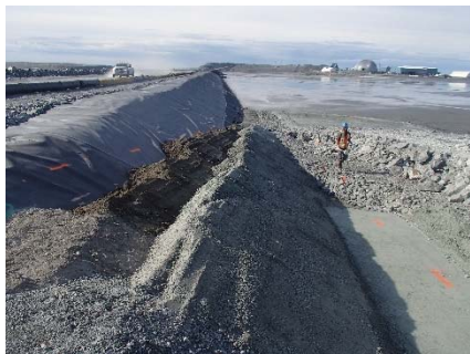
CD-1896 (2018-07-22), looking S from Sta. 0+140/-30 m. Placement of 0.5 m thick layers of compacted sieved till and fine filter on the upstream slope of Central Dike with an excavator from Sta. 0+147 m to 0+177 m.
