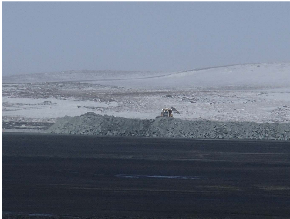
Photograph NCIS-023: From Sta. 2+570 m (approx.), looking W. Placement of a 2 m thick (approx.) lift of UM rockfill from El. 150 m to El. 152 m (approx.) with a dozer from Sta. 1+500 m to 1+450 m (offset unavailable). The material is of good quality and is well graded.
