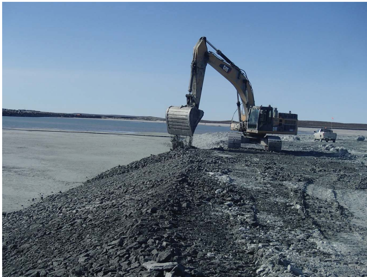
Photograph NCIS-063: From Sta. 1+200/-65 m (approx.), looking SW. Placement of a 0.5 m thick lift of coarse filter in the upstream slope from El. 148 m to 152 m with an excavator from Sta. 1+270 m to 1+100 m.
