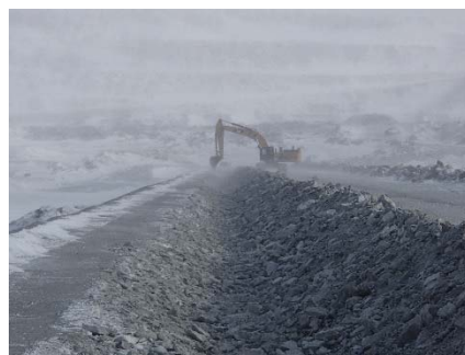
CD-1852 (2018-05-14), looking N from Sta. 0+500/-25 m. Excavation of the LLDPE geomembrane crest anchoring trench from Sta. 0+830 m to 0+170 m.
