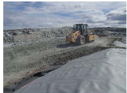
SD3-349 (2018-07-18), looking SE from Sta. 20+765/-29 m. Compaction of the 0.5 m thick lift of fine filter on the top of the upstream toe liner tie-in with a 10 tonne smooth-drum compactor with vibration (4 passes) from Sta. 20+777 m to 20+807 m.
