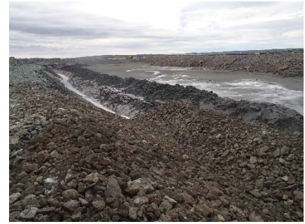
NCIS-138 (2018-08-01), looking SW from Sta. 1+365/+15 m (approx.). Excavation of a 0.8 m (approx.) deep, 1 m wide shallow ditch in the tailings and placement of a 0.3 m thick (approx.) layer of till sieving reject material on the bottom and on the slopes of the ditch from Sta. 1+200 m to 1+100 m.
