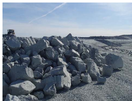
NCIS-120 (2018-07-26), looking NE from Sta. 1+830/-27 m (approx.). View of an accumulation of boulders on the upstream slope of the NCIS.
