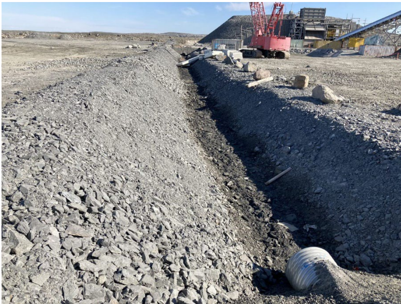
Photograph H12-6 UG Ore Stockpile Saline Ditch
