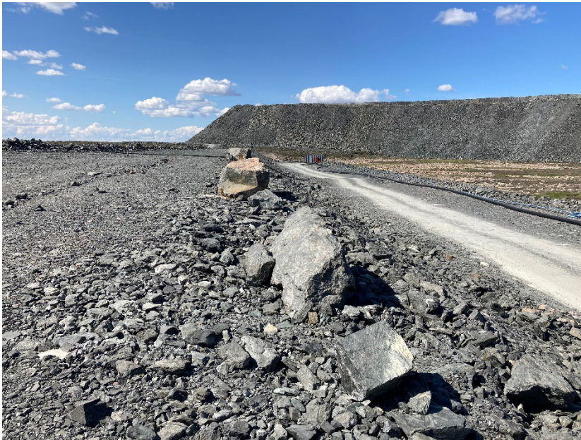
Photograph A7-4 WRSF Dike
