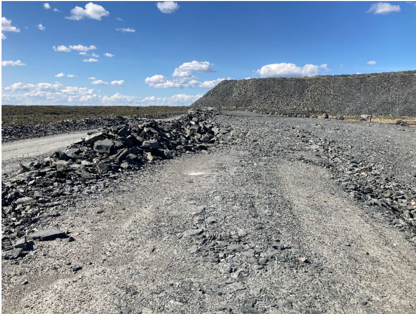
Photograph A7-3 WRSF Dike
