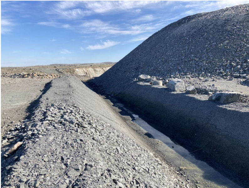
Photograph H12-7 UG Ore Stockpile Saline Ditch
