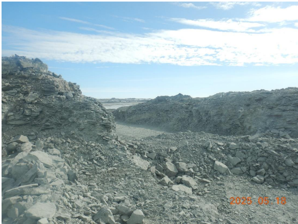
Blast to 5140, progressive mucking
