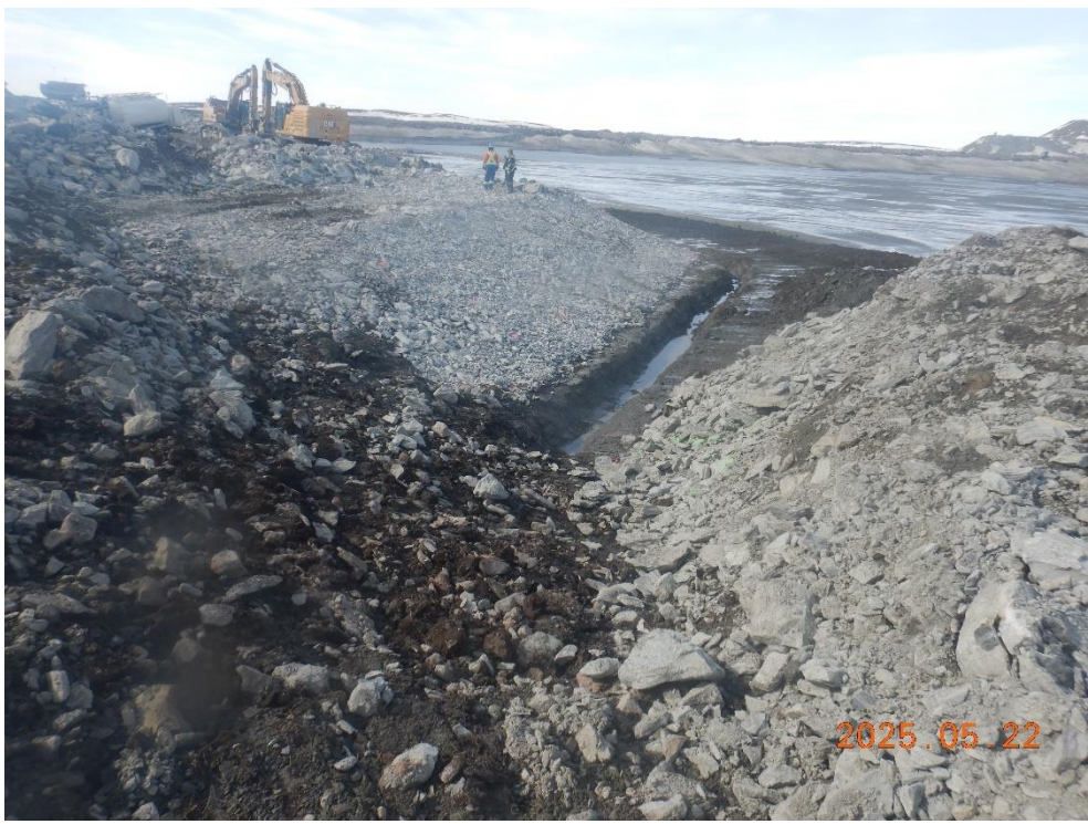
Excavation of key trench at east abutment
