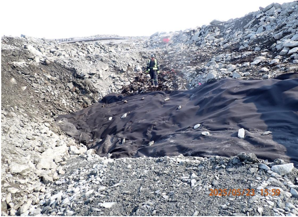
Geotextile placement on natural ground at east abutment
