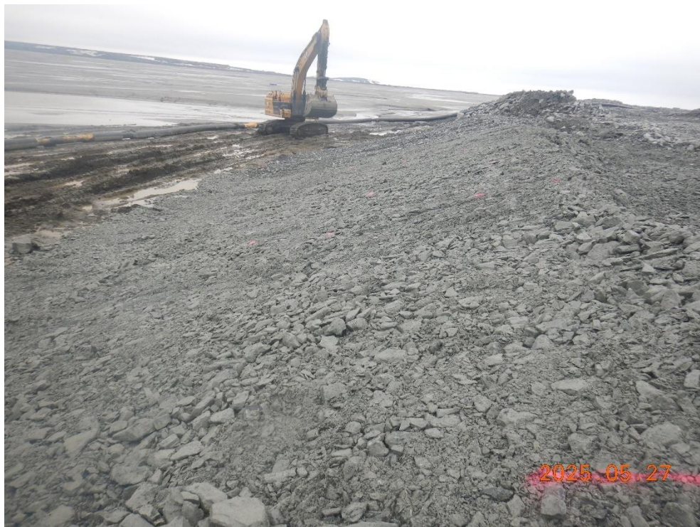
Completion of coarse filter placement and sloping
