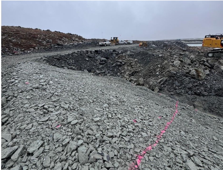
Survey markings indicating continuation of road cover at El. 145 masl
