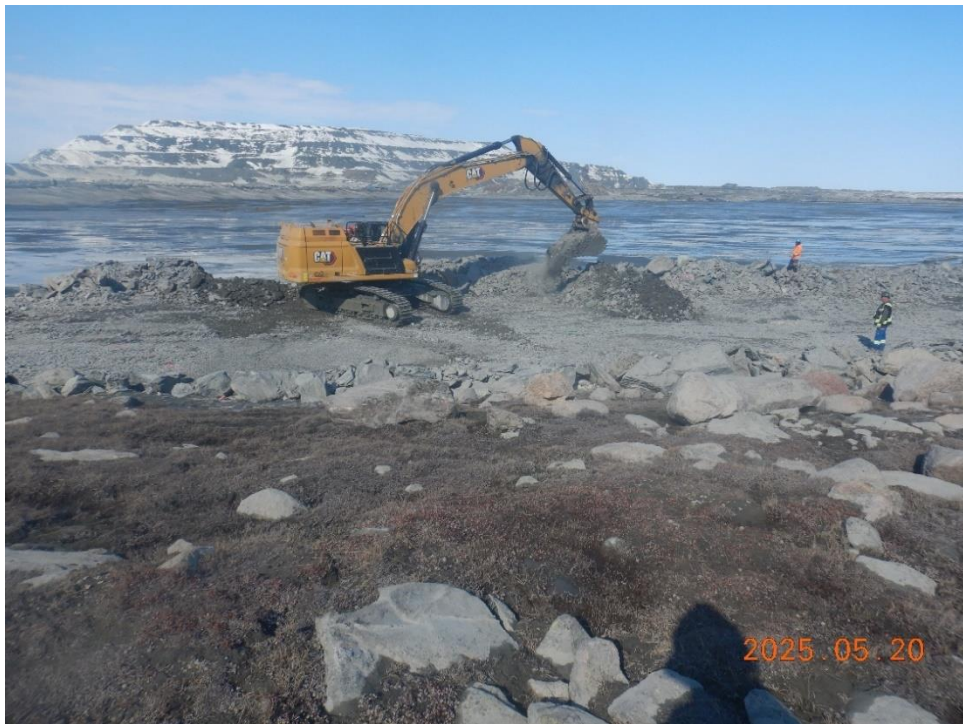
Beginning of removal of access road at El. 145
