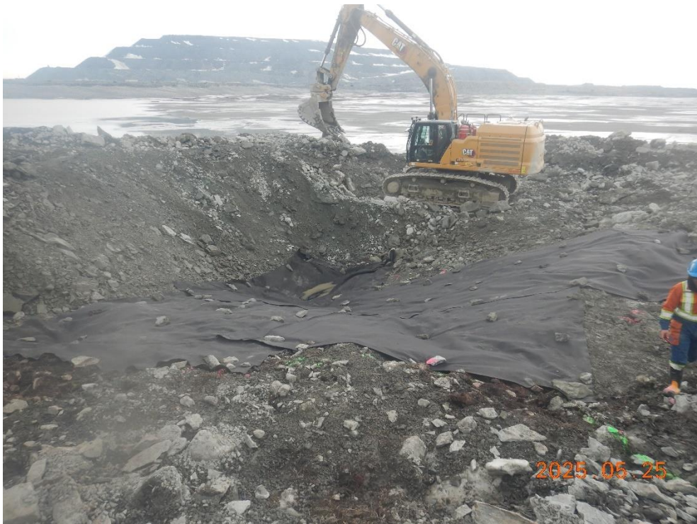
Geotextile placement at west abutment
