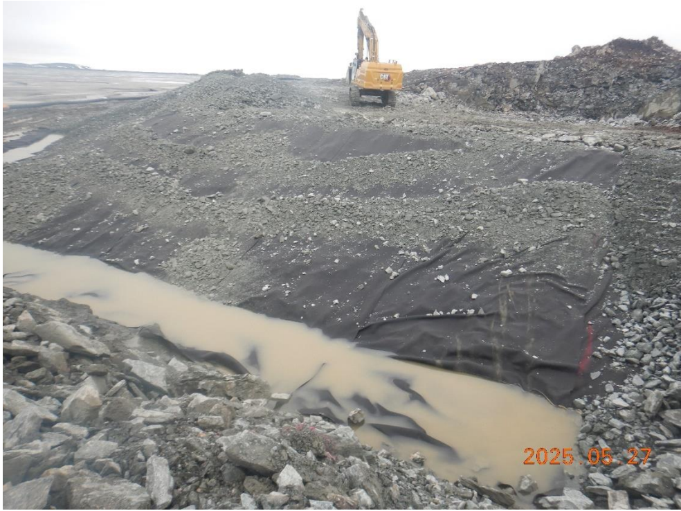
Geotextile placement on upstream slope, near west abutment
