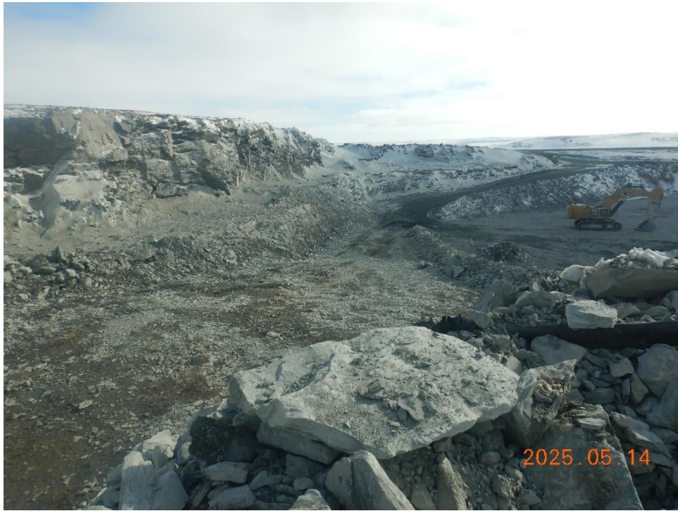
Status of southern access ramp, looking south
