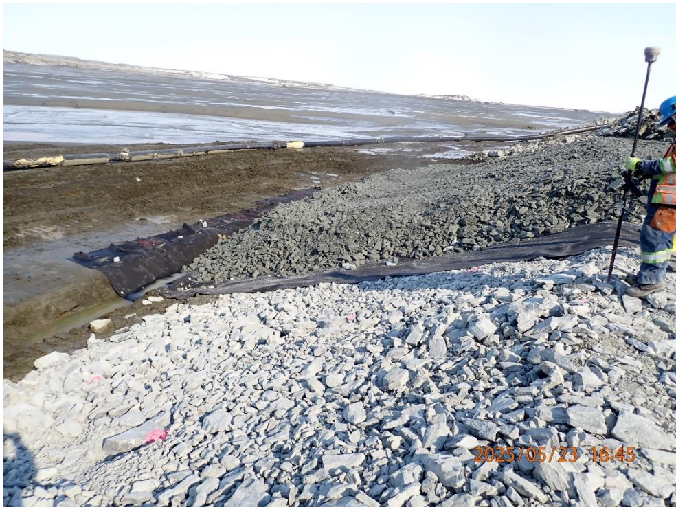
Coarse filter placed over geotextile near eastern slope
