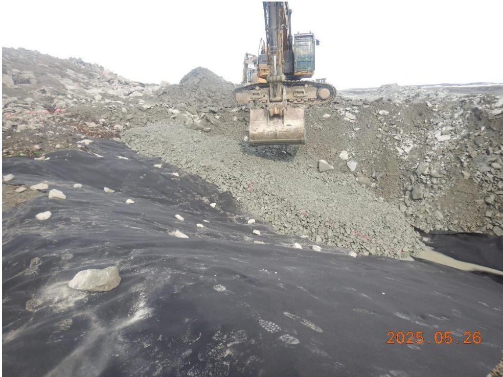
Coarse filter placement at west abutment
