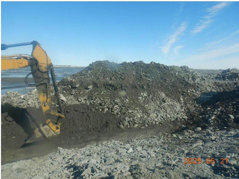
Preparation of key trench at east abutment
