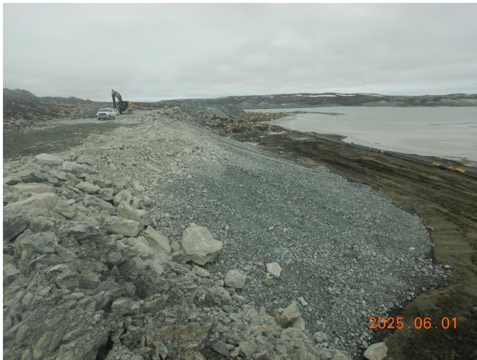
Completed upstream slope
