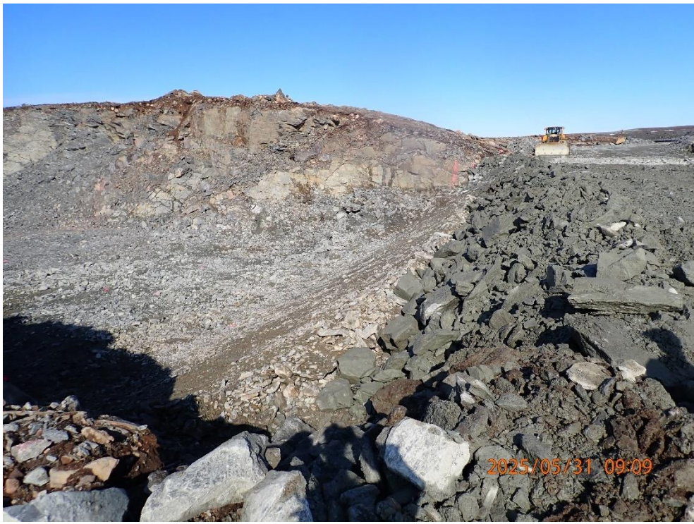
Progress of second lift of rockfill on downstream slope
