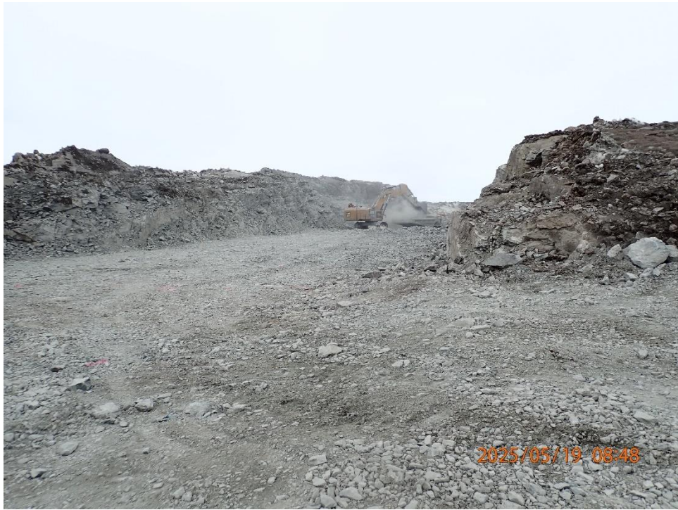
Progress of mucking 5149 floor
