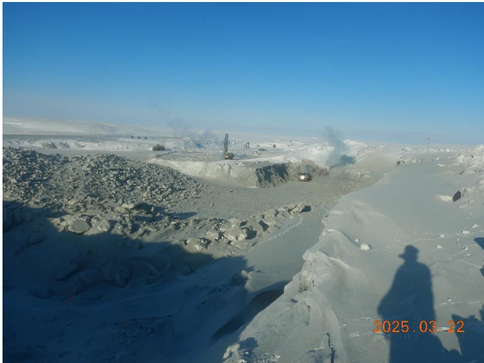
Routine drilling and mucking activities in the western sector
