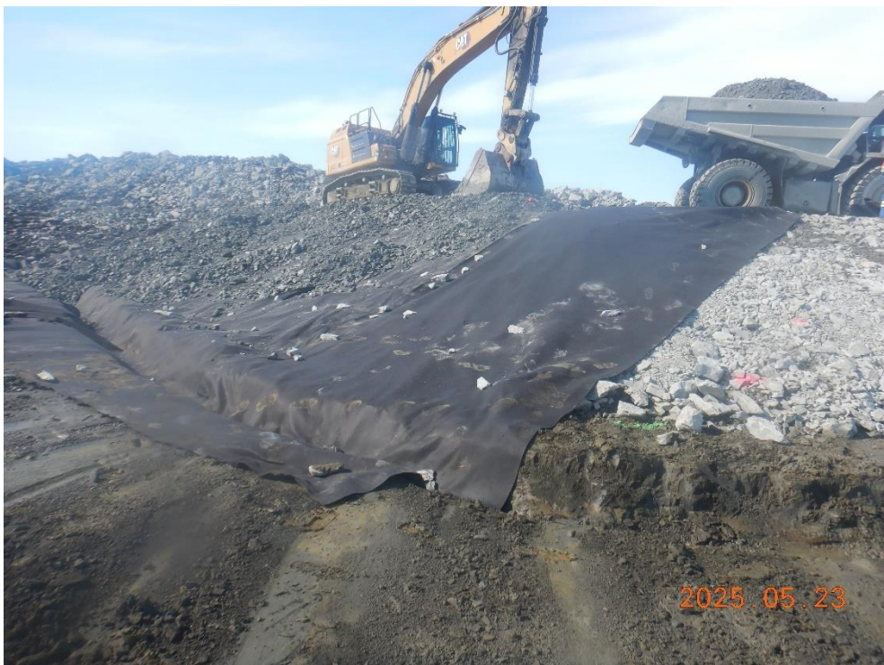
Continuation of geotextile placement and key trench excavation at upstream slope
