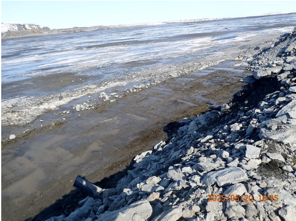
Preparation of upstream foundation in tailings
