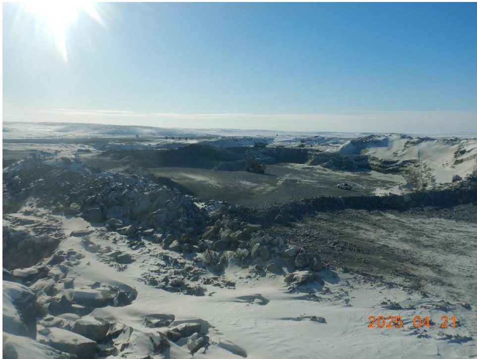
Progress of 5135 floor
