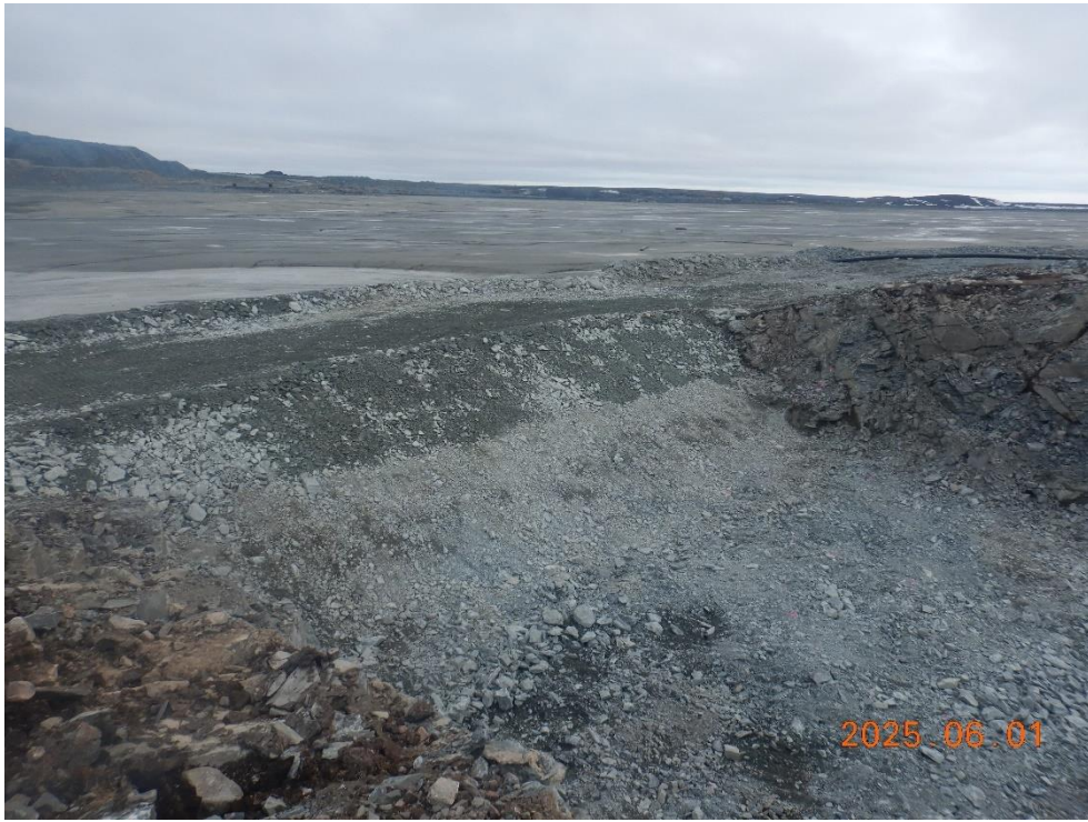
Completed downstream slope
