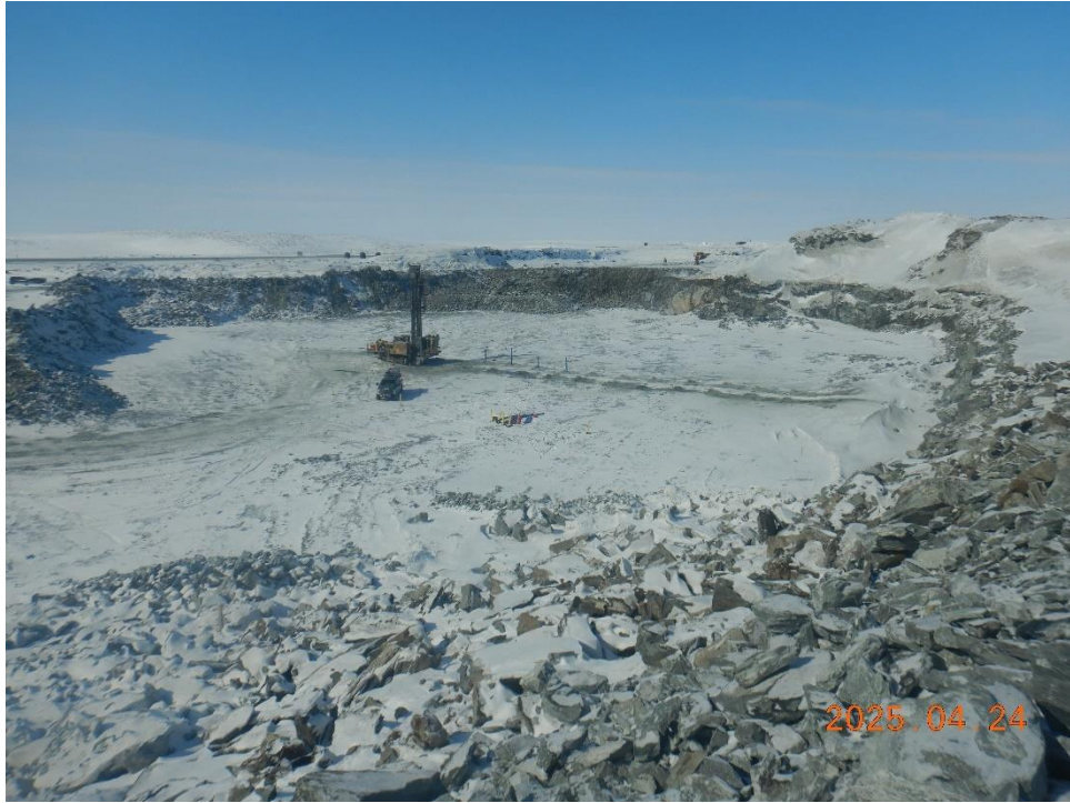
Drilling of 5128 temporary sump
