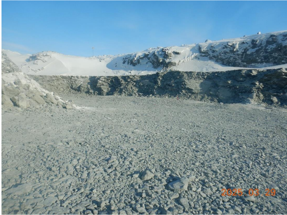
Clean floor of 5142 prior to blasting to 5135
