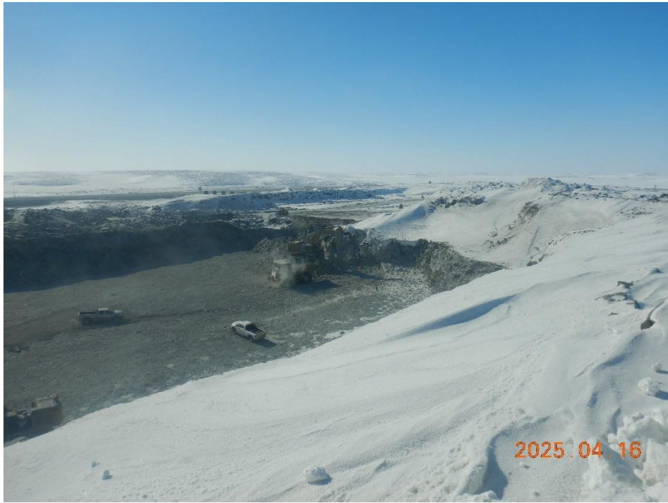
Progress of routine mucking activities, looking southwest
