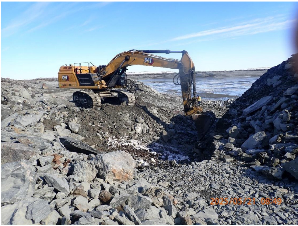
Preparation of east abutment tie-in to natural ground. Removal of snow.
