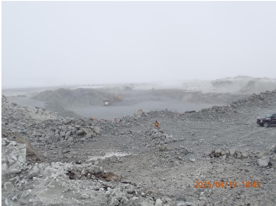
Survey preparation of drill patterns in spillway on 5149 bench
