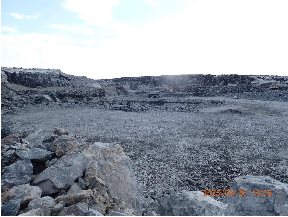
Completed Phase 1, looking northeast and 5135 floor
