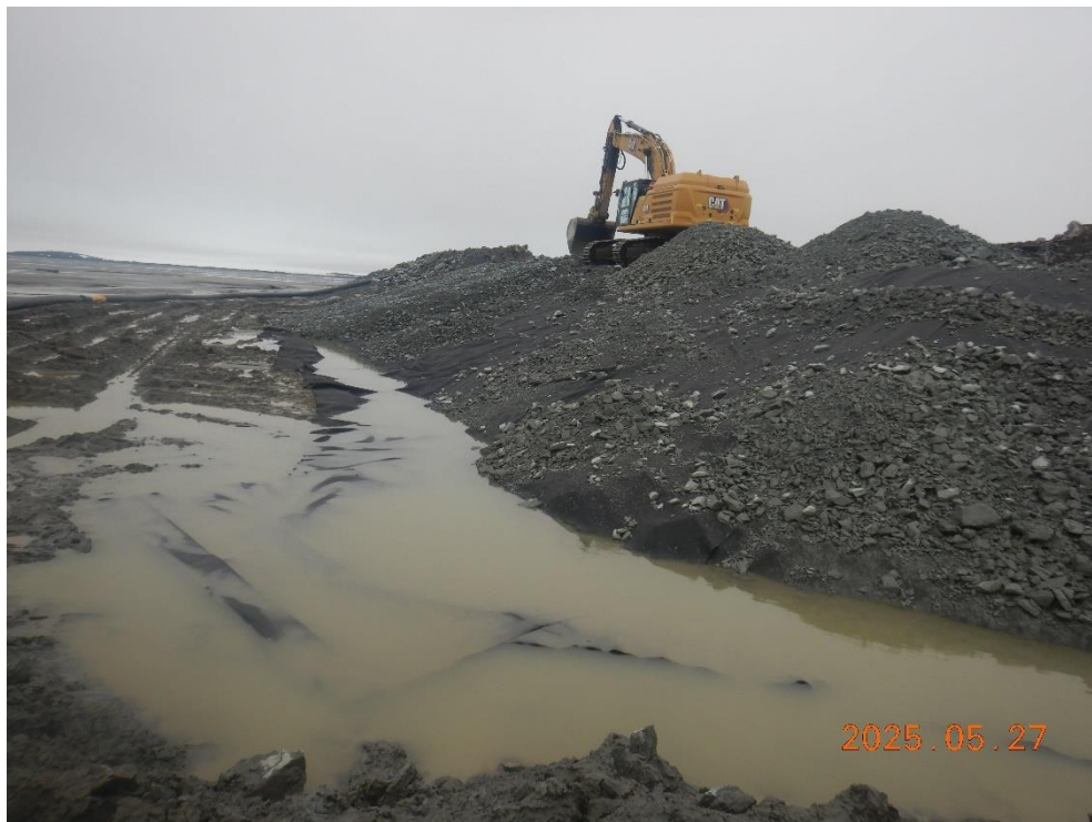
Continuation of coarse filter placement over geotextile
