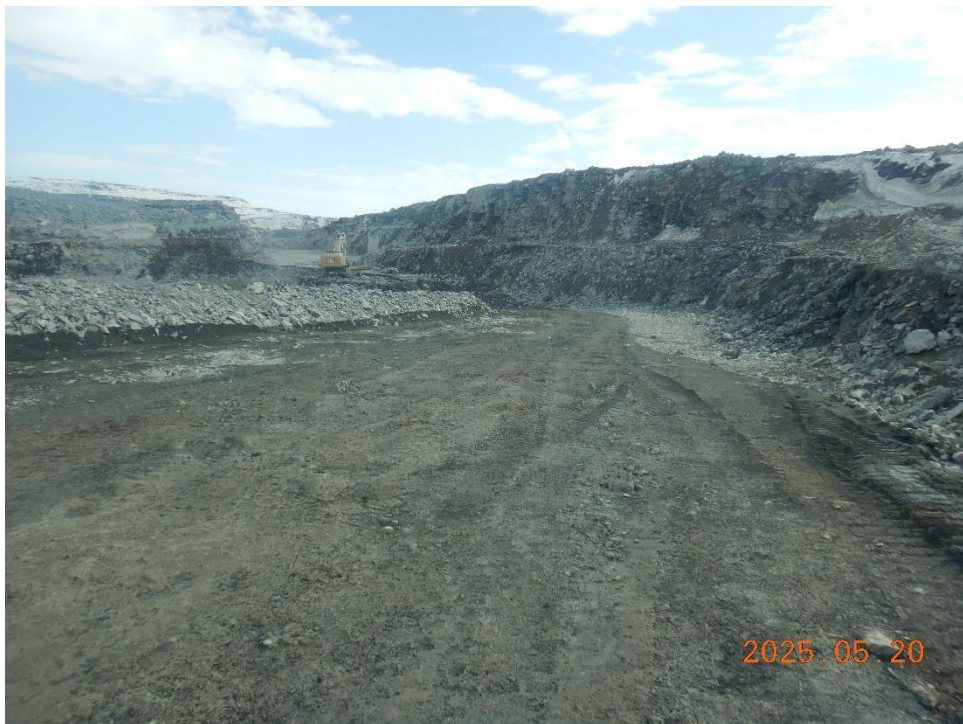
Status of southern access ramp, looking north
