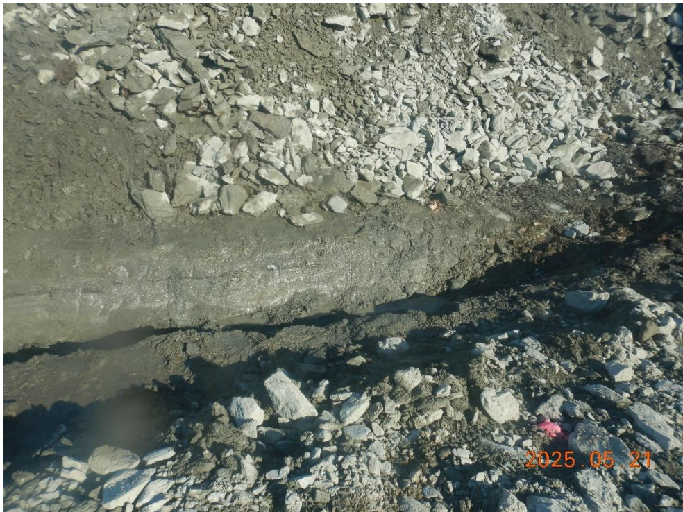
Condition of key trench excavation in tailings near east abutment
