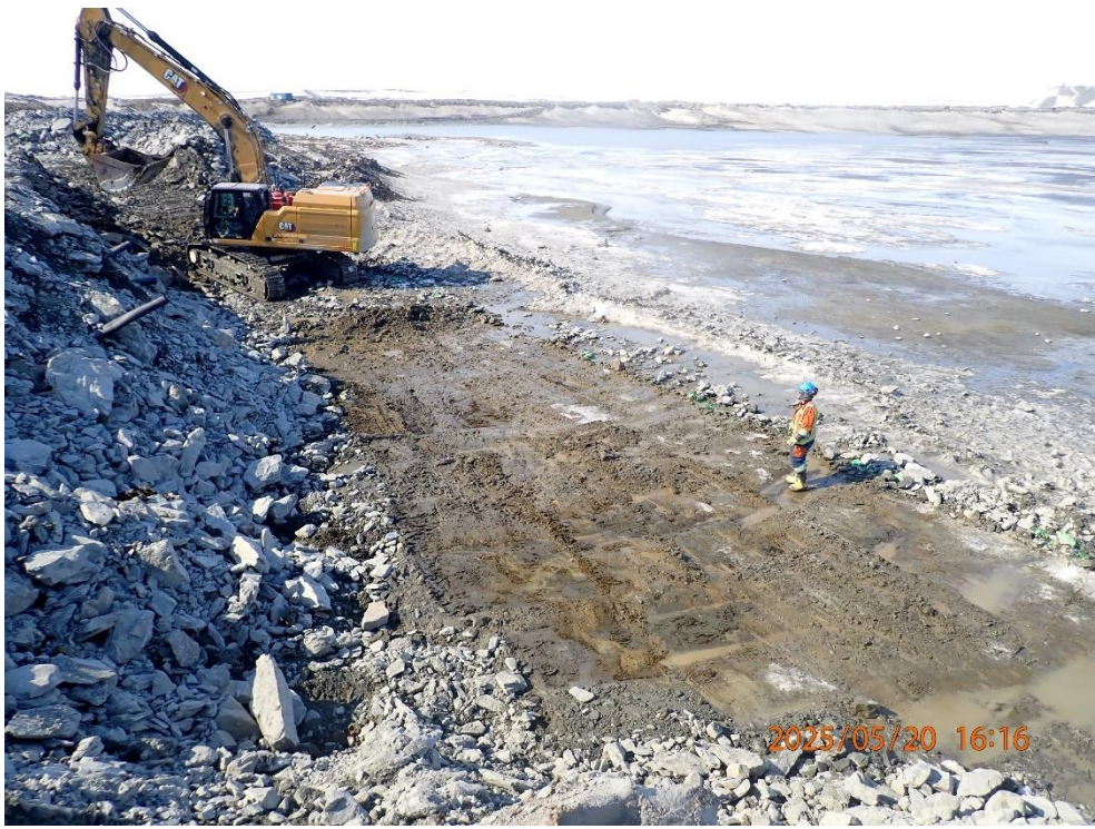
Preparation of upstream foundation in tailings
