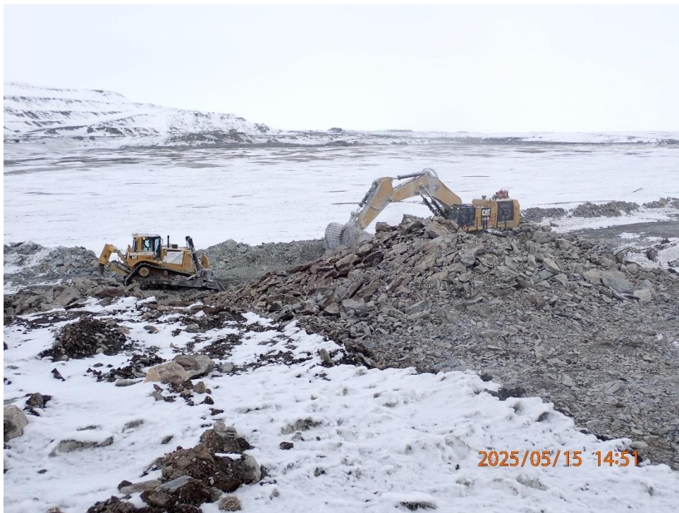
Mucking of 5140 material and creation of temporary drilling pad
