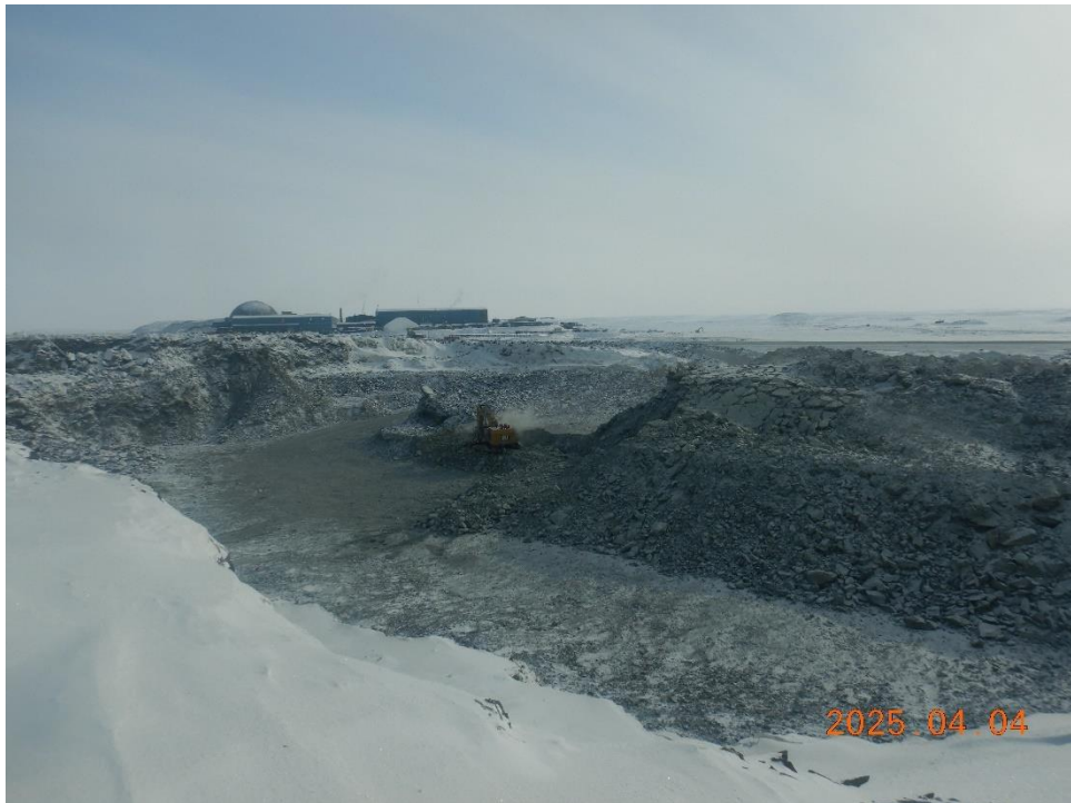
Progress of routine mucking activities, looking southeast
