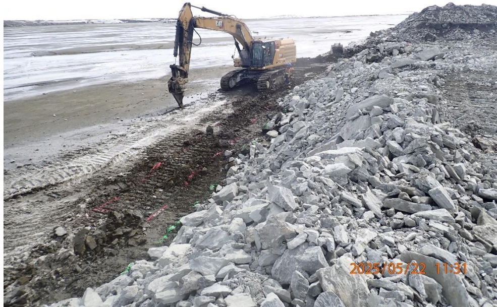
Preparation and survey markings for key trench excavation upstream
