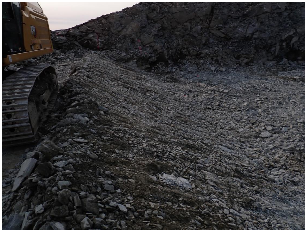
Progress of first lift of rockfill on downstream slope
