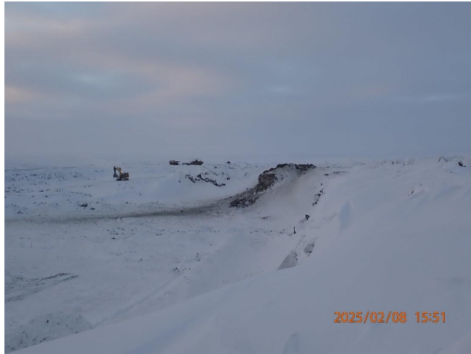
West wall of collection pond; signature blast
