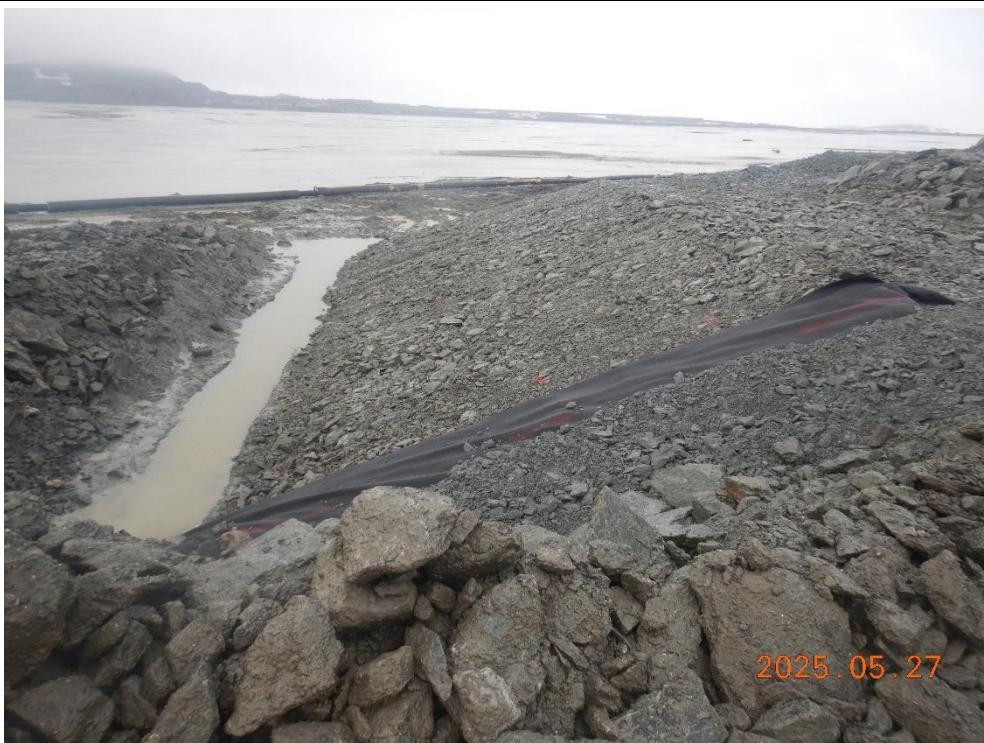
Rockfill slope preparation and key trench excavation continuing past west abutment
