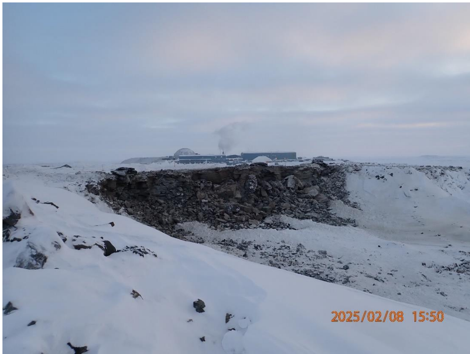
East wall of collection pond; signature blast
