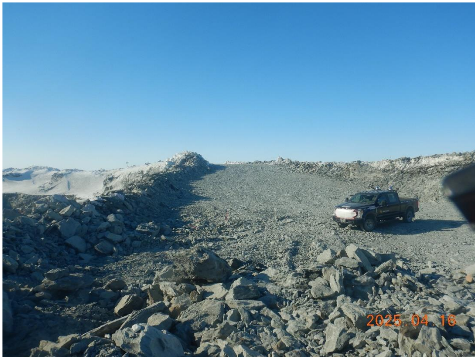
Ramp from west created to 5149 to access spillway footprint
