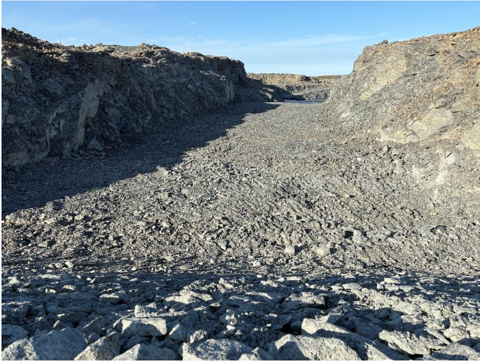
Completed spillway, looking south from temporary reclaim berm
