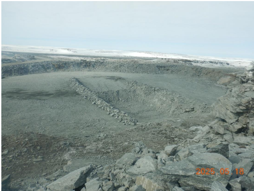
Completed 5128 sump with safety berms in place
