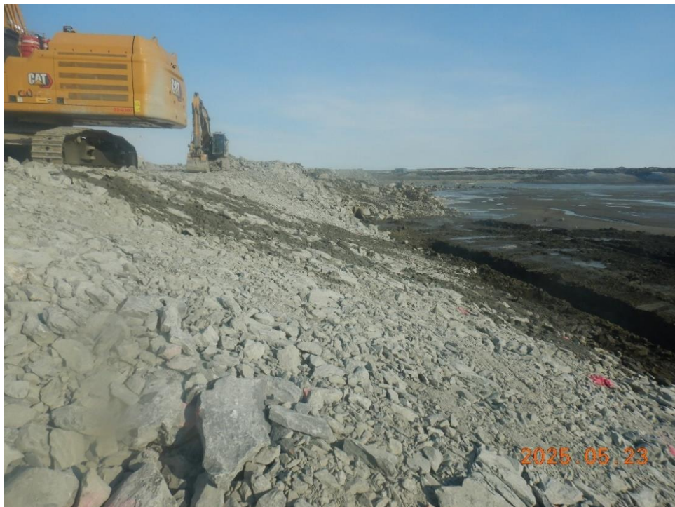
Preparation of upstream rockfill slope towards west abutment
