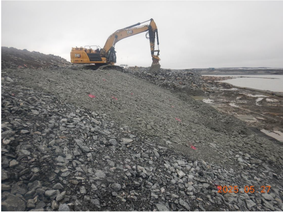
Completion of coarse filter placement and sloping
