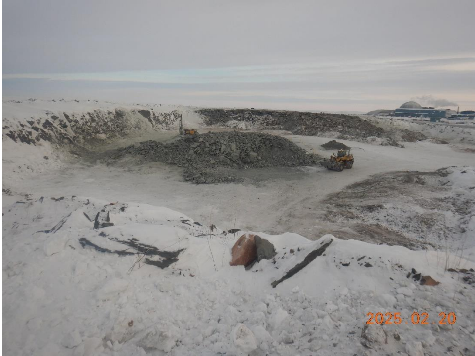
Mucking of 5142 blast material
