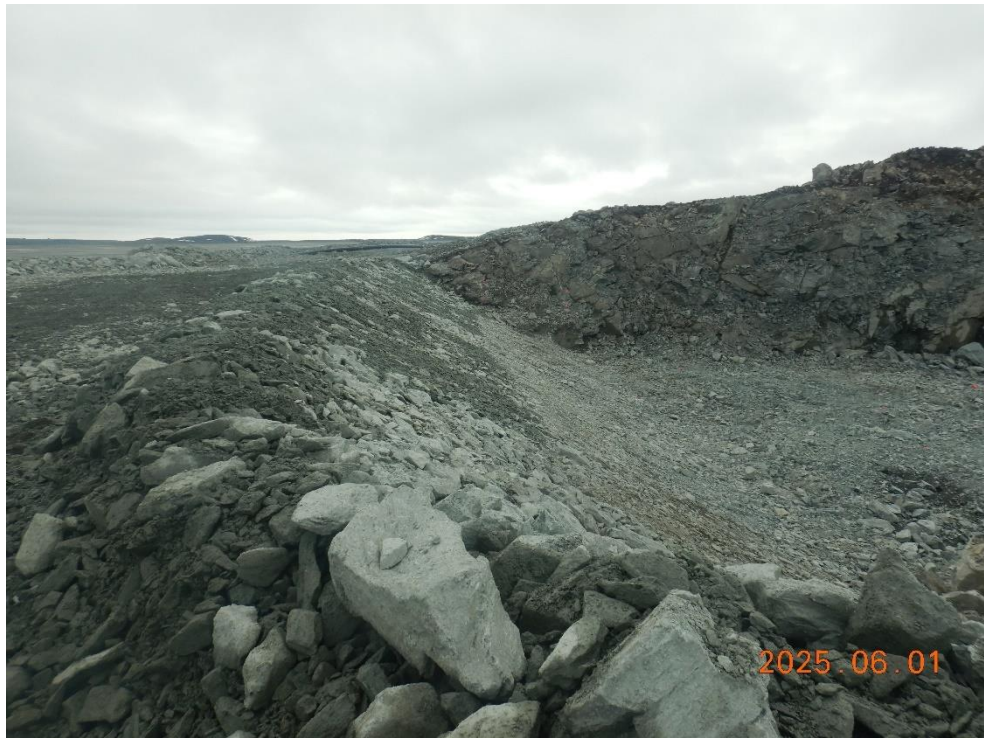
Completed downstream slope
