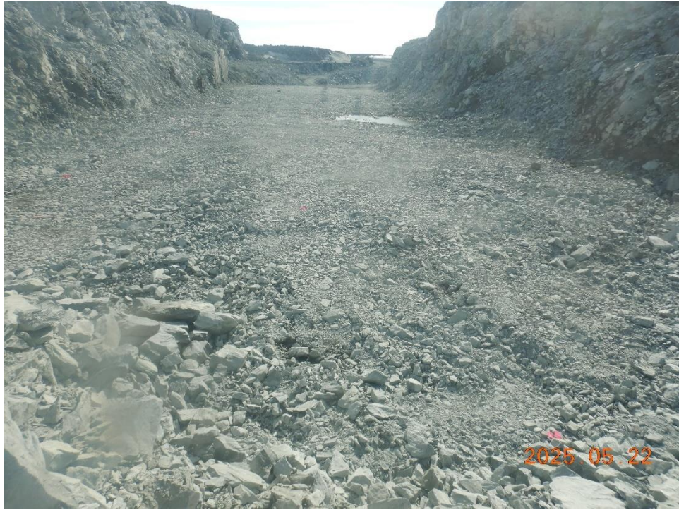
Completed mucking of spillway to 5140 floor, looking south towards CP23
