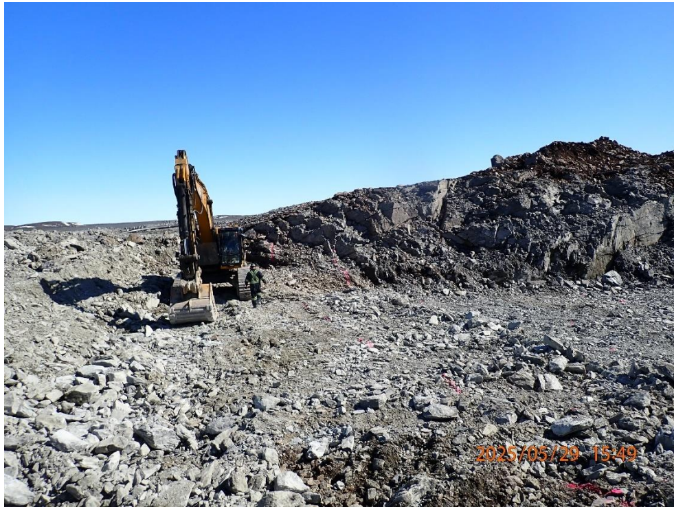
Preparation of downstream slope within spillway
