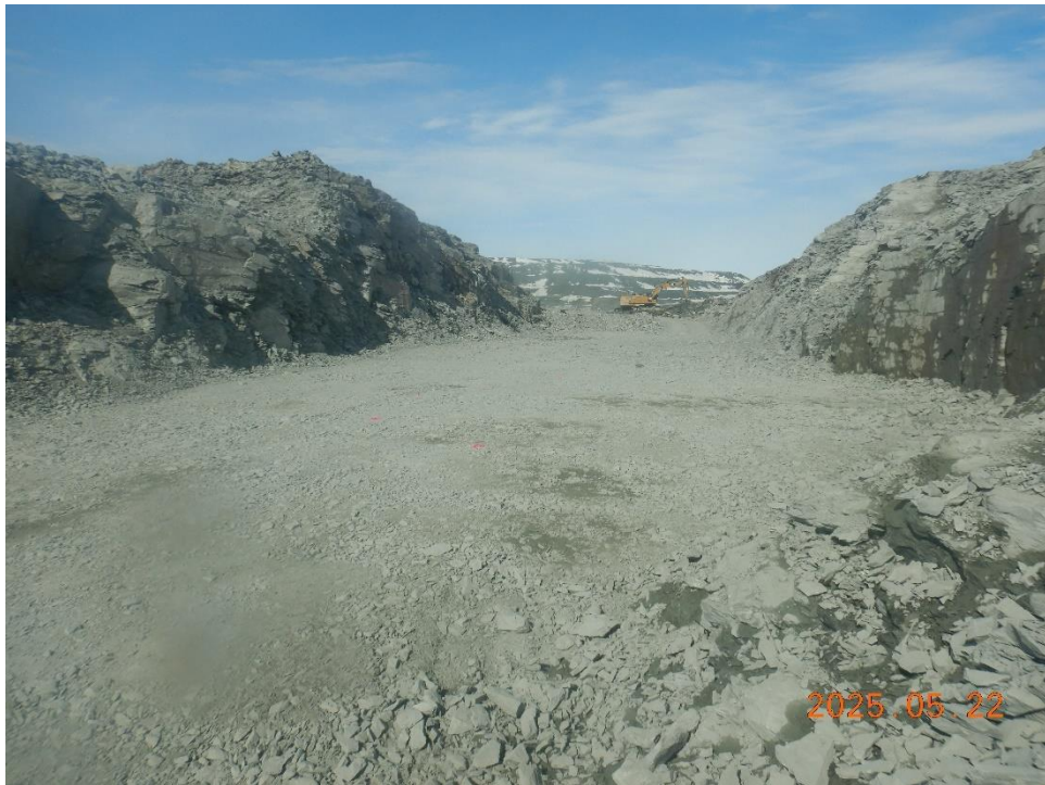
Completed mucking of spillway to 5140 floor, looking north towards South Cell
