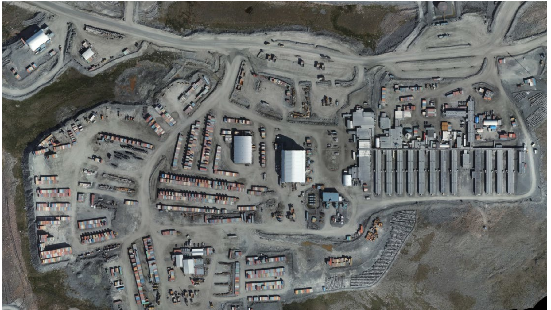
Figure 1-3 Aerial photo showing Whale Tail camp infrastructure (Summer 2025)
