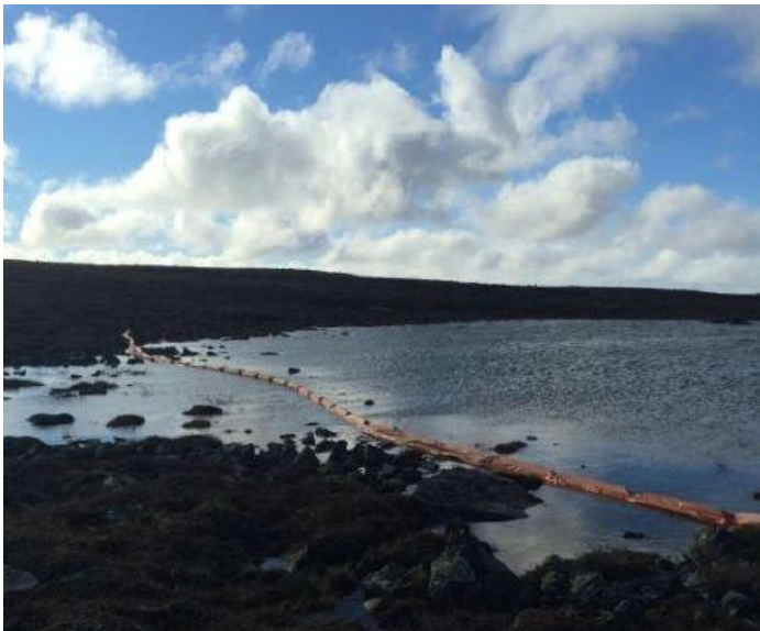
Figure 2-11: Turbidity barriers at the inlet of Dogleg Lake
