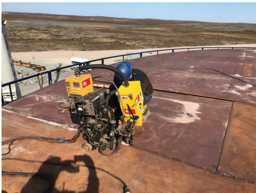
Tank roof plate welding
