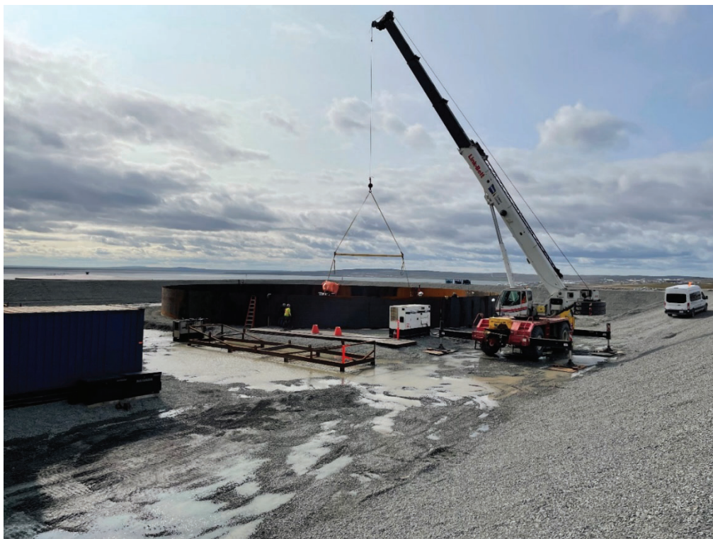
Tank wall welding
