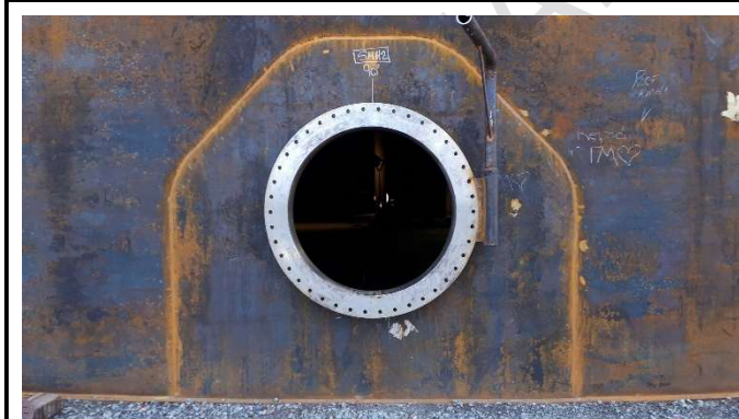
Photo #6: Manway (90 degree)
