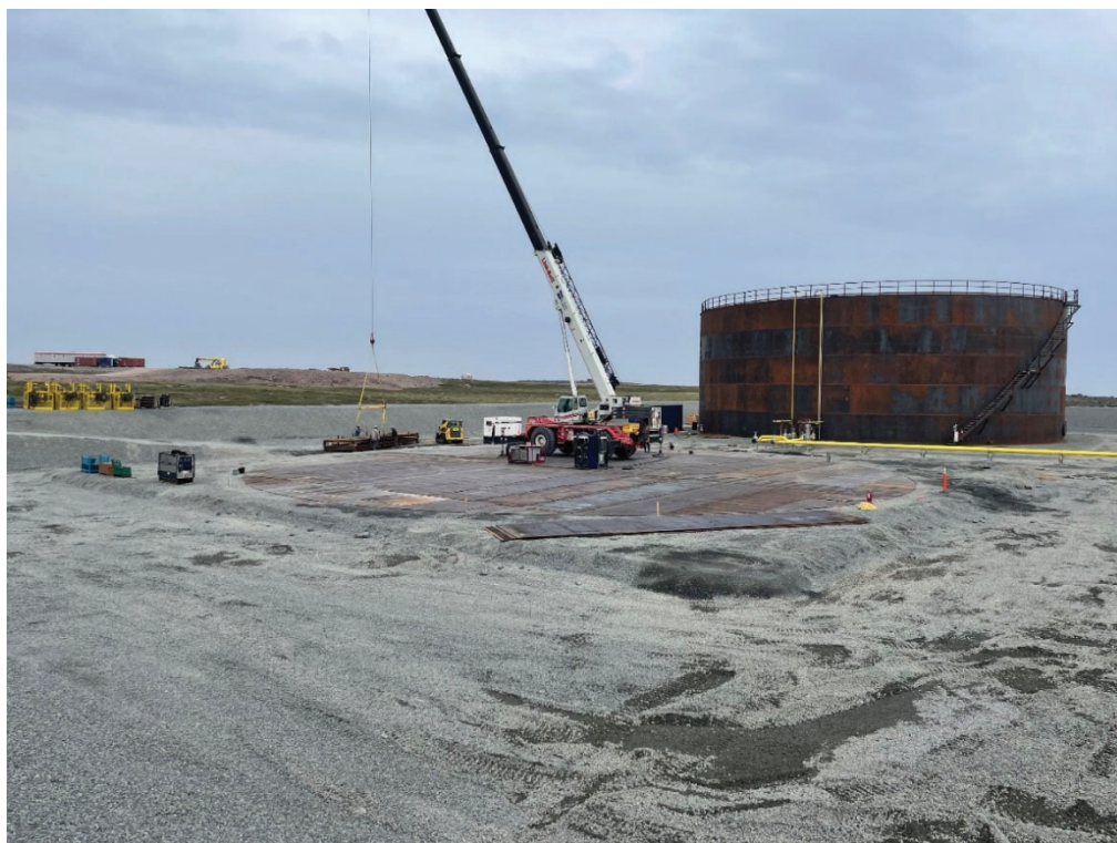
Tank floor construction
