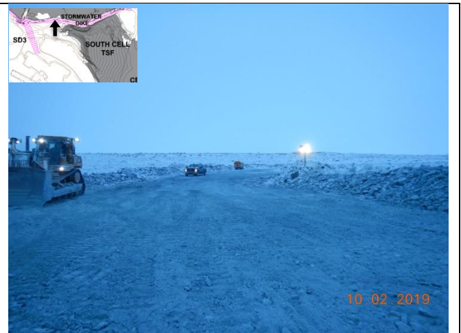
Photo 8: View of the berm
