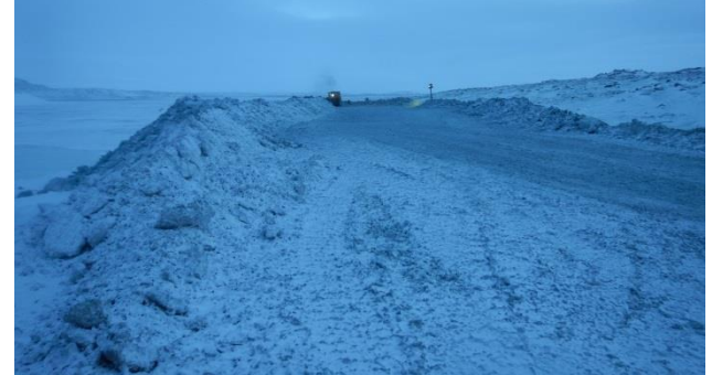
Photo 2: Construction of the access road
