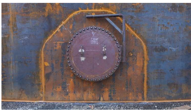
Photo #8: Manway (180 degree)
