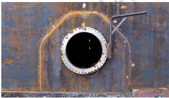
Photo #12: Manway (270 degree)
