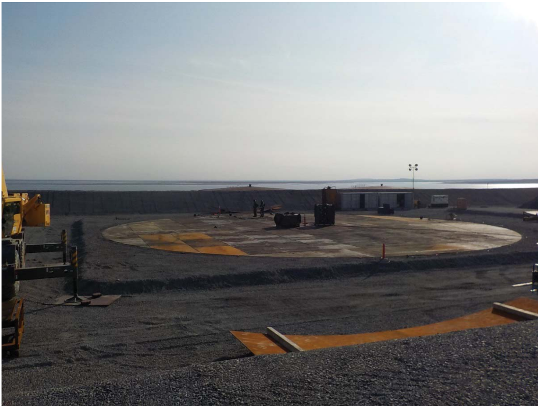
Tank floor construction
