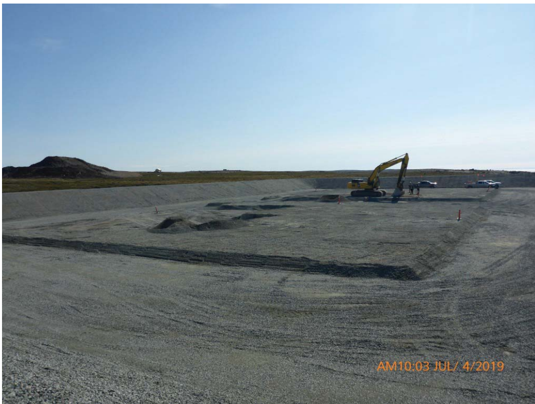
Tank pad construction
