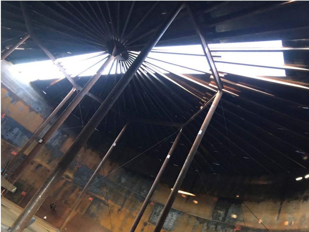
Tank roof structure
