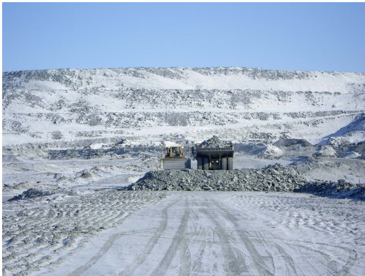
Photograph CD-1798: From Sta. 0+500/-15 m looking N. Placement of a 2 m thick (approx.) lift of intermediate volcanic (IV) rockfill from El. 143 m to El. 145 m from 0+340 to 0+435 m (o.s. -28 to -18 m).
