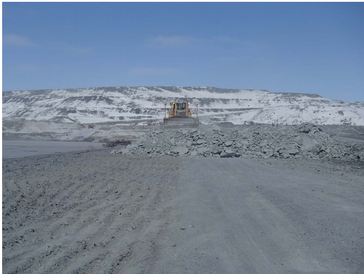
Photograph CD-1801: From Sta. 0+650/-10 m looking N. Placement of a 2 m thick (approx.) lift of intermediate volcanic (IV) rockfill from El. 143 m to El. 145 m from 0+535 to 0+625m (o.s. -28 to -18 m).
