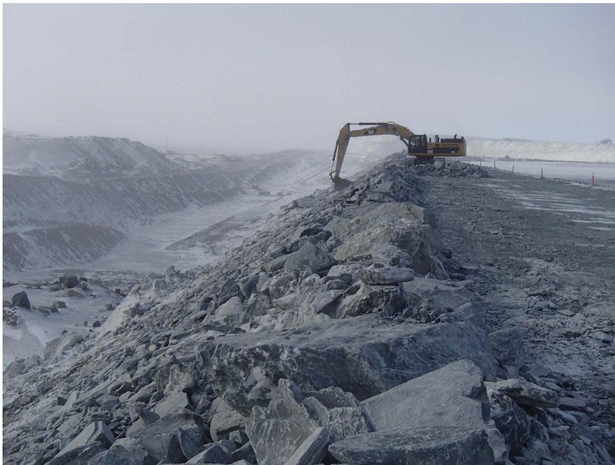
Photograph CD-1821: From Sta. 0+175/+3, looking S. Profiling of the downstream slope (1.5H:1V) from El. 143 to 145 m with an excavator between Sta. 0+250 m and 0+330 m.
