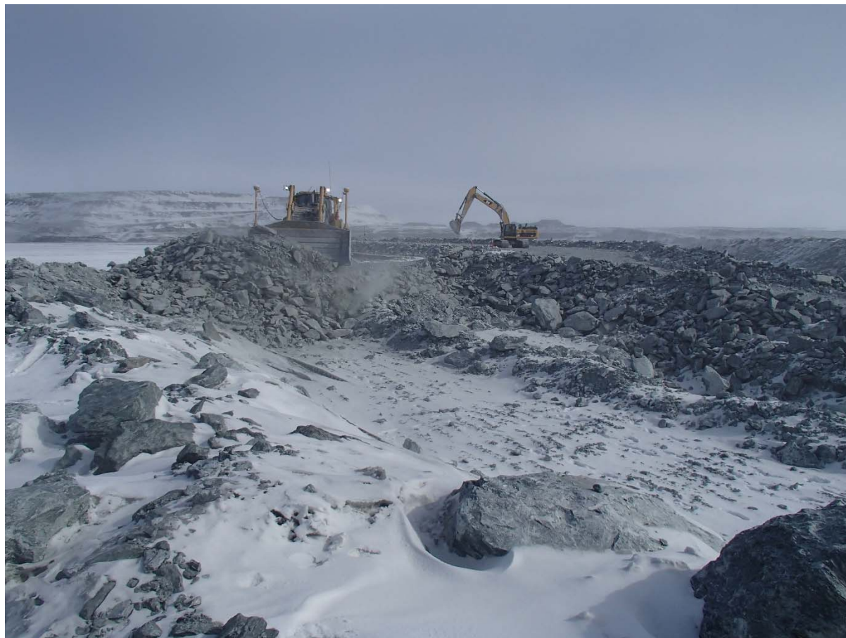
Photograph CD-1822: From Sta. 40+725/+7, looking N. Placement of two 2 m thick (approx.) lifts of intermediate volcanic (IV) rockfill from El. 141 m to El. 145 m from approx. Sta. 40+720 m to 40+750 m (o.s. -10 to +10 m) and profiling of the upstream slope (2H:1V) from El. 143 to 145 m with an excavator between Sta. 0+830 m and 0+980 m.
