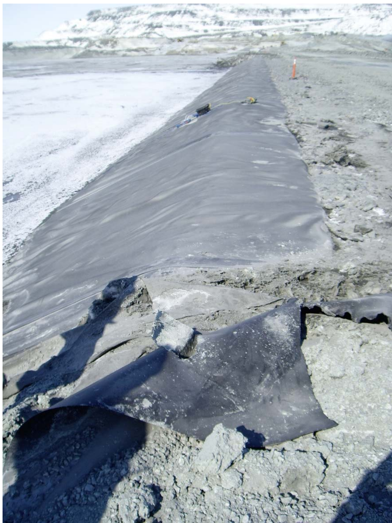
Photograph CD-1796: From Sta. 0+650/-28 m, looking N. Damaged geomembrane near a deposition finger on Central Dike.
