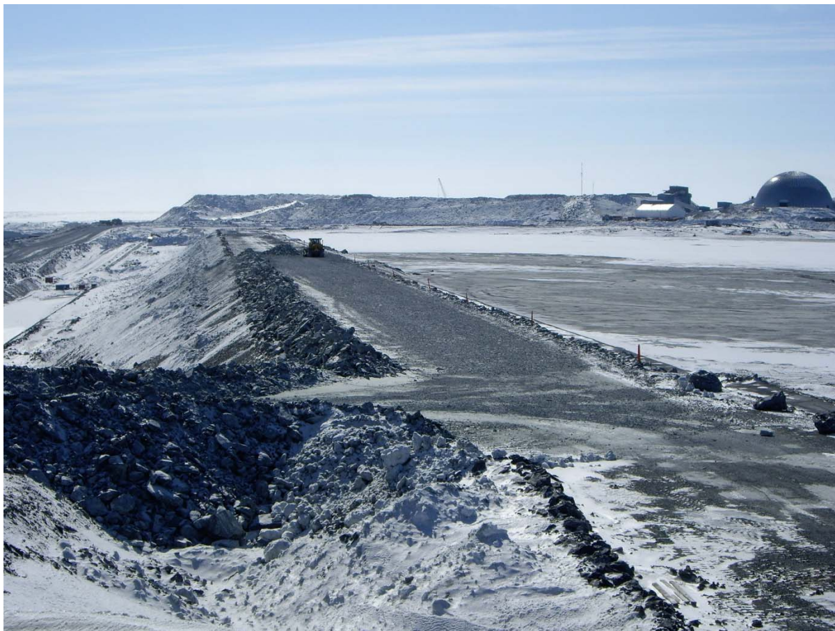
Photograph CD-1799: From Sta. 0+080/-25 m looking S. Placement of a 2 m thick (approx.) lift of intermediate volcanic (IV) rockfill from El. 143 m to El. 145 m from 0+340 to 0+435 m (o.s. -28 to -18 m).
