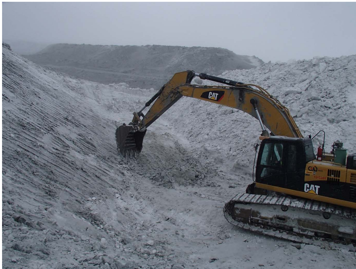
Photograph CD-1805: From Sta. 40+780/2 m looking NE. Final clean-up of footprint with an excavator to reach a good quality bedrock from Sta. 40+780 to 40+805 m (o.s. -6 to 9 m).
