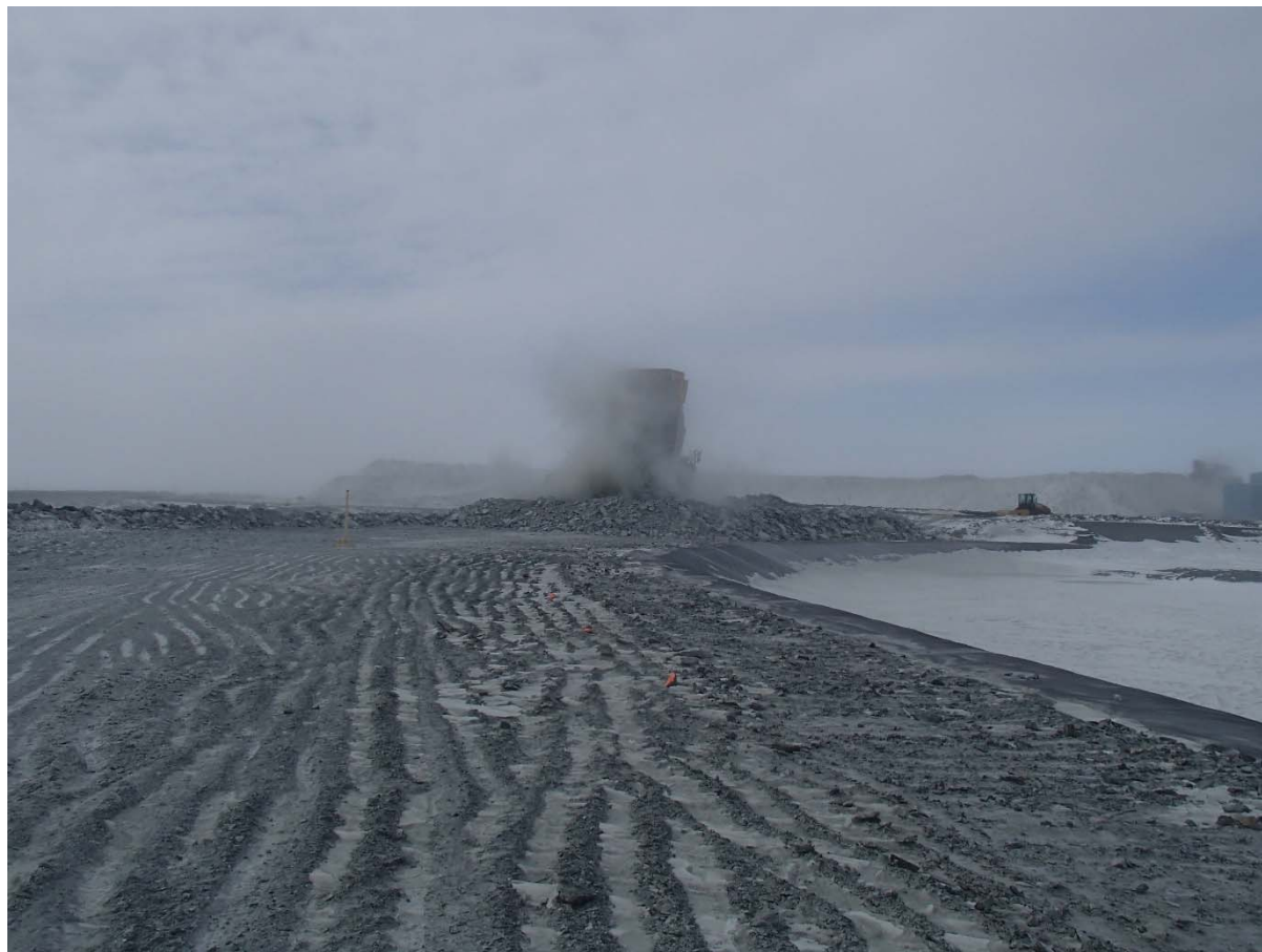
Photograph CD-1815: From Sta. 0+920/-25, looking S. Placement of a 2 m thick (approx.) lift of intermediate volcanic (IV) rockfill from El. 143 m to El. 145 m from approx. Sta. 40+740 to 0+980 m (o.s. -28 to -11 m).
