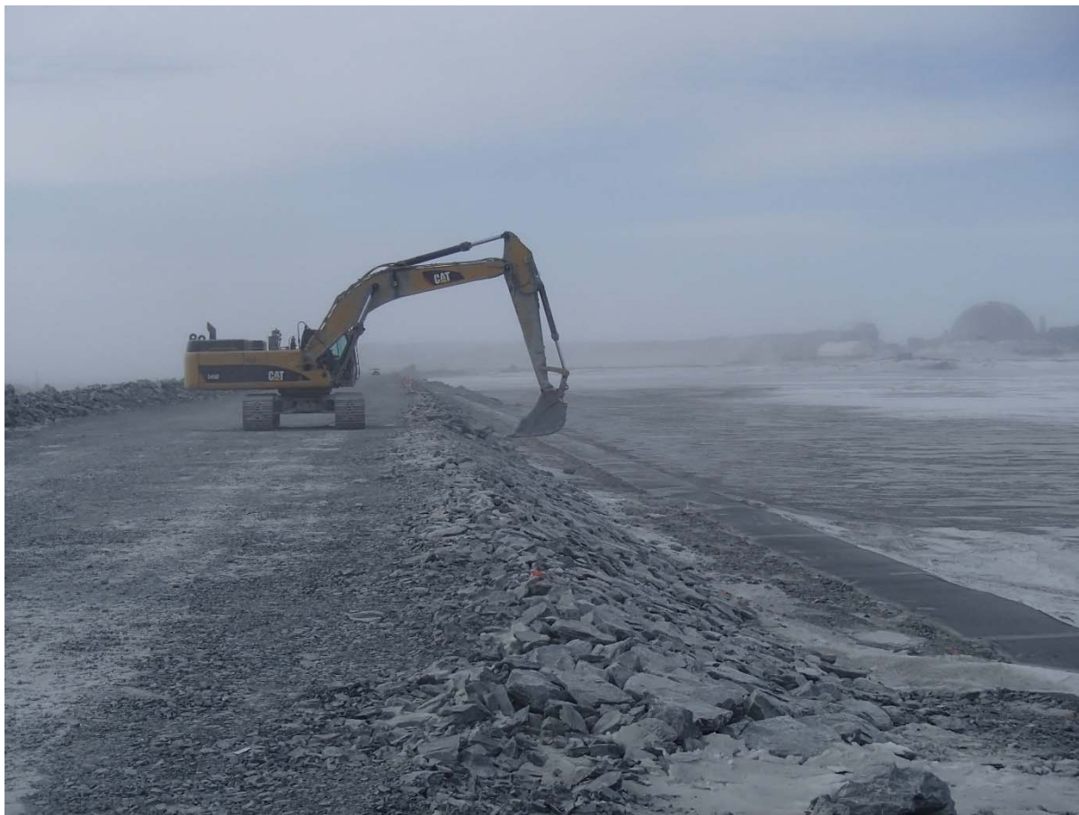
Photograph CD-1816: From Sta. 0+175/-27, looking S. Profiling of the upstream slope (2H:1V) from El. 143 to 145 m with an excavator between Sta. 0+175 and 0+560 m.
