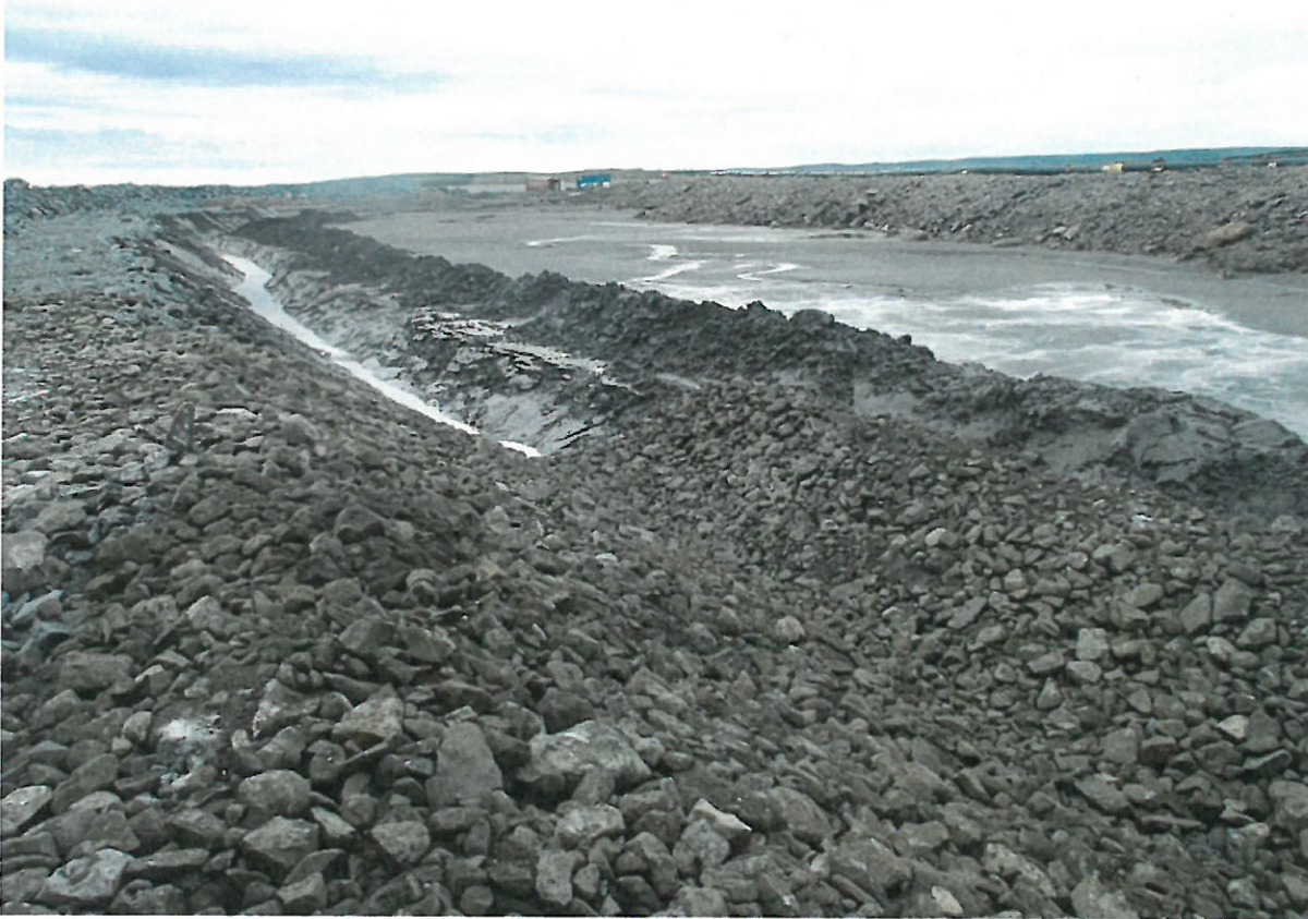
Photograph NCIS-138: From Sta. 1+365/+15 m (approx.), looking SW. Excavation of a 0.8 m (approx.) deep, 1 m wide shallow ditch in the tailings and placement of a 0.3 m thick (approx.) layer of till sieving reject material on the bottom and on the slopes of the ditch from Sta. 1+200 m to 1+100 m.
