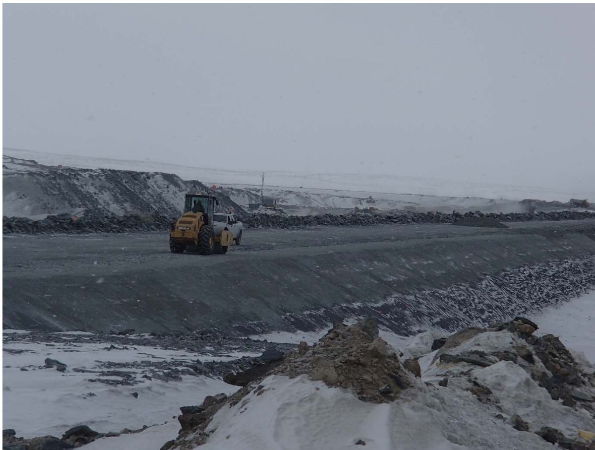
Photograph CD-1847: From Sta. 0+085/-48 m, looking SE. Compaction of the fourth 0.5 m lift (approx.) of fine and coarse filters material at El. 145 m with a 10-tonne smooth-drum compactor with vibration (4 passes) from Sta. 0+170 m to 40+730 m.
