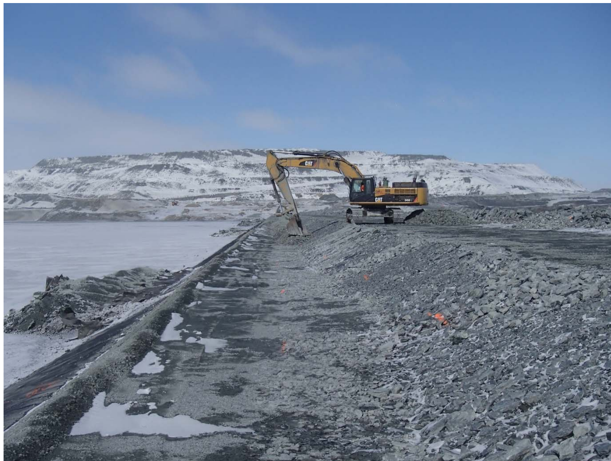
Photograph CD-1838: From Sta. 0+835/-20 m, looking N. Placement of a second 0.5 m thick lift of coarse filter from El. 143.5 m to 144 m with an excavator from Sta. 0+500 m to 0+835 m and from Sta. 0+930 to 40+730 m.
