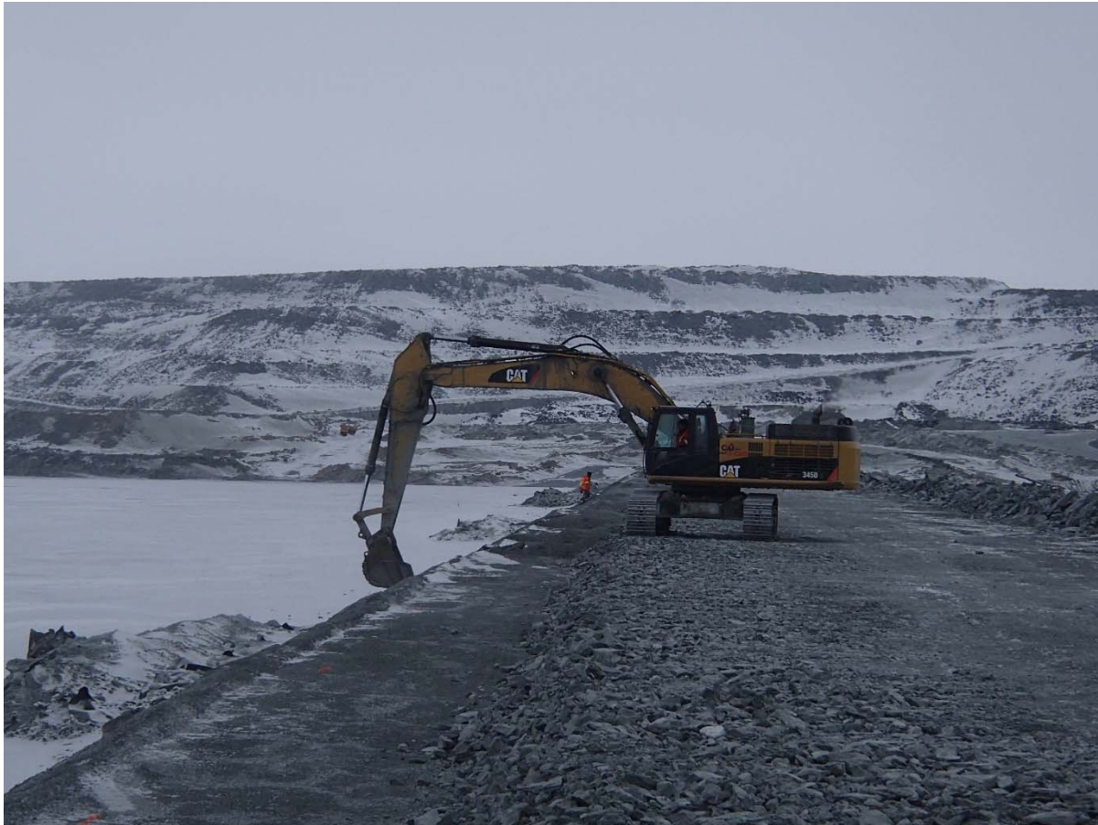
Photograph CD-1846: From Sta. 0+835/-25 m, looking N. Profiling of the upstream slope (2H:1V) from El. 143 to 145 m with an excavator between Sta. 0+330 and 0+600 m and between Sta. 0+715 m and 40+730 m. The removed material was placed with material from the fine filter stockpile on the fourth 0.5 m thick lift of fine filter from El. 144.5 m to 145 m upstream of the coarse filter with an excavator from Sta. 0+330 m to 0+600 m and between Sta. 0+715 m and 40+730 m.
