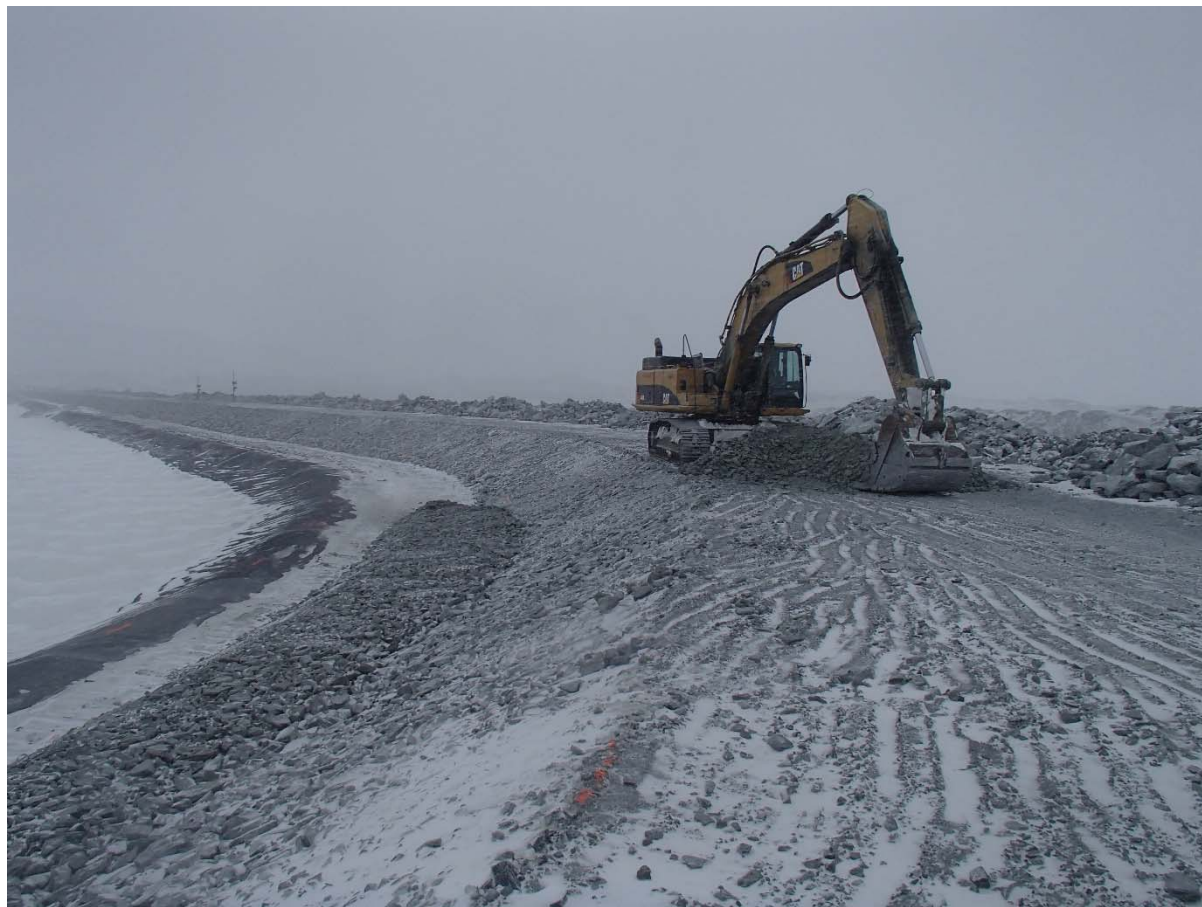
Photograph CD-1826: From Sta 40+770/-27 m, looking NE. Placement of a 0.5 m thick lift of coarse filter from El. 143 m to 143.5 m with an excavator from Sta. 40+730 m to 0+ 775 m.
