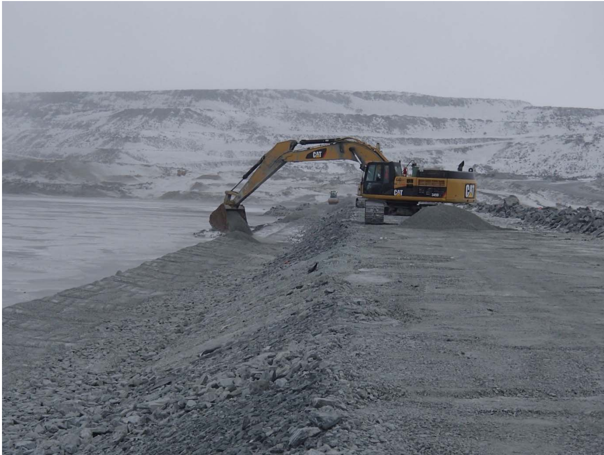
Photograph CD-1836: From Sta. 0+830/-20 m, looking N. Placement of a first 0.5 m thick lift of fine filter from El. 143 m to 143.5 m upstream of the coarse filter with an excavator from Sta. 0+490 to 0+835 m.
