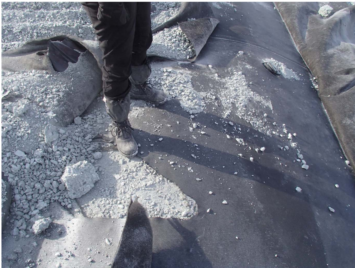
Photograph CD-1833: From Sta. 0+390/-25 m, looking S. Damaged geomembrane near a deposition finger on Central Dike at Sta. 0+390 m.
