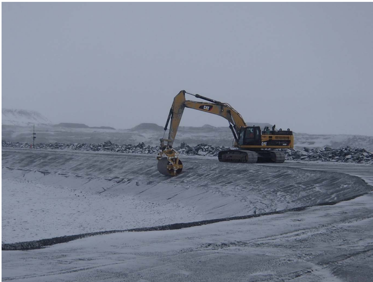
Photograph CD-1849: From Sta. 40+750/-17 m, looking NE. Final rolling of the upstream slope in view of the LLDPE geomembrane installation from Sta. 0+170 m to 40+730 m.
