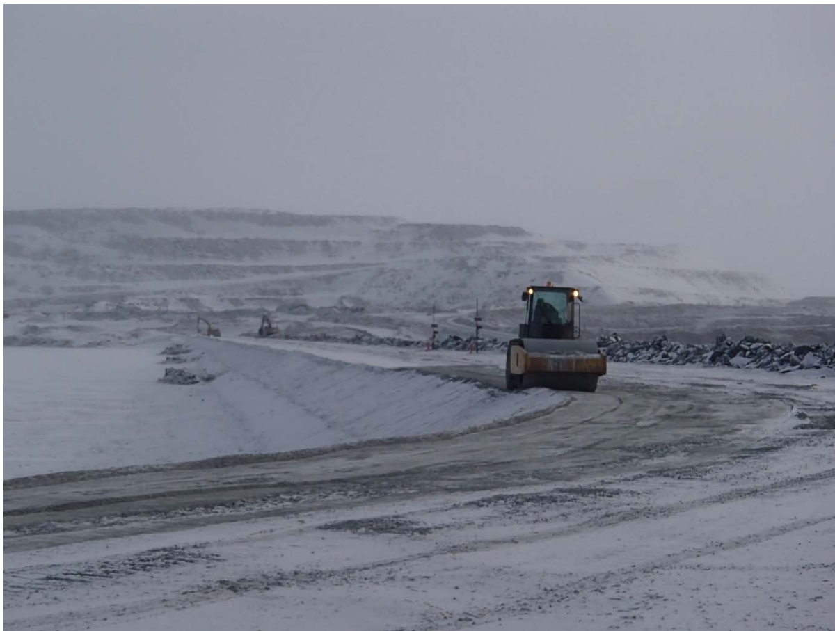
Photograph CD-1848: From Sta. 40+780/-15m, looking N. Compaction of the fourth 0.5 m lift (approx.) of fine and coarse filters material at El. 145 m with a 10-tonne smooth-drum compactor with vibration (4 passes) from Sta. 0+930 m to 40+730 m.
