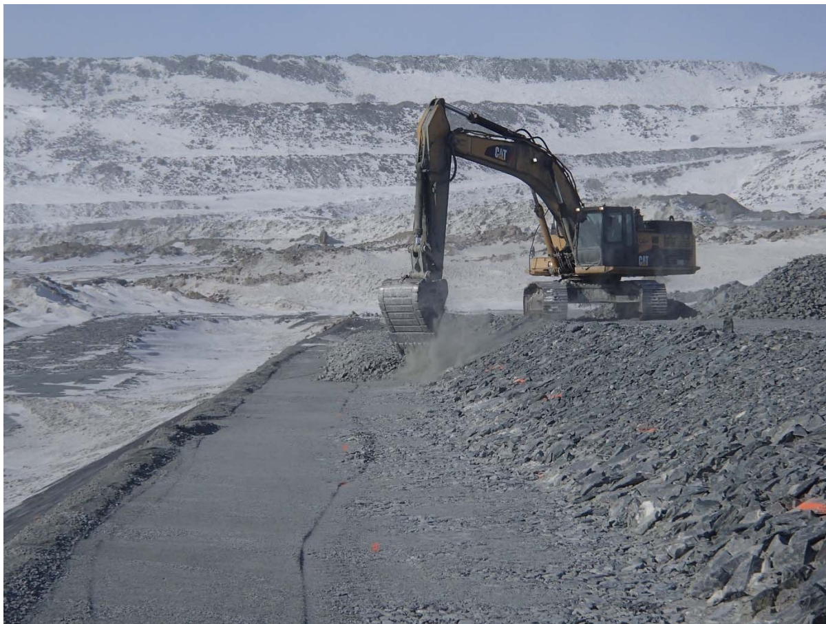
Photograph CD-1832: From Sta. 0+280/-25 m, looking N. Placement of a second 0.5 m thick lift of coarse filter from El. 143.5 m to 144 m with an excavator from Sta. 0+175 m to 0+280 m.
