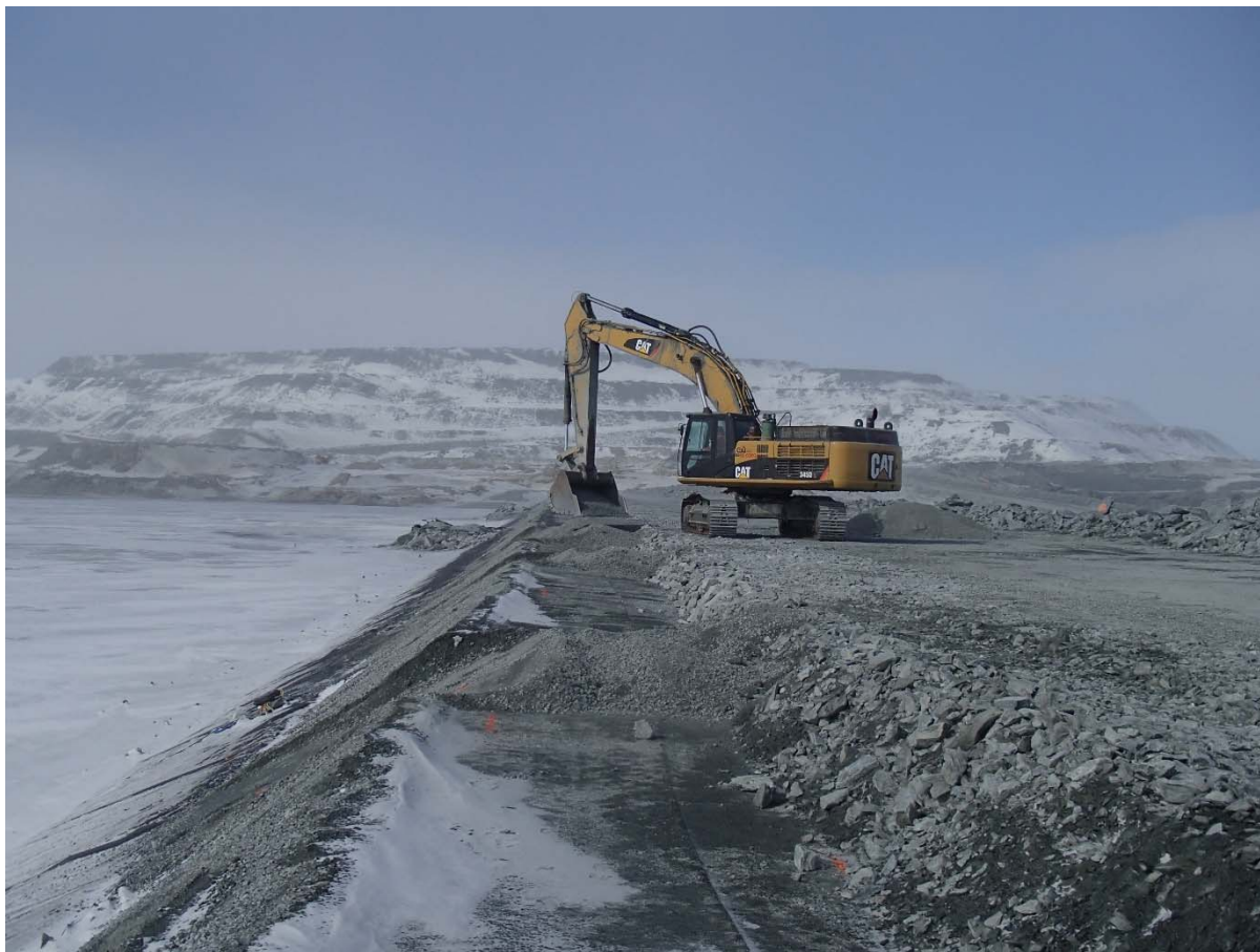
Photograph CD-1845: From Sta. 0+660/-20 m, looking N. Profiling of the upstream slope (2H:1V) from El. 143 to 145 m with an excavator between Sta. 0+175 and 0+330 m and between Sta. 0+600 m and 0+715 m. The removed material is placed on the fourth 0.5 m thick lift of fine filter from El. 144.5 m to 145 m upstream of the coarse filter with an excavator from Sta. 0+170 m to 0+330 m and between Sta. 0+600 m and 0+715 m.
