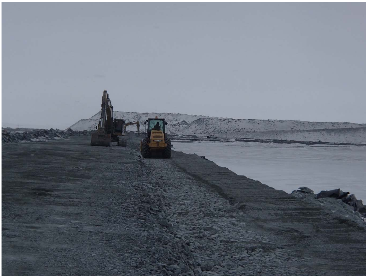
Photograph CD-1843: From Sta. 0+460/-23 m, looking S. Compaction of the third 0.5 m lift (approx.) of fine and coarse filters material at El. 144.5 m with a 10-tonne smooth-drum compactor with vibration (4 passes) from Sta 0+335m to 0+900 m.
