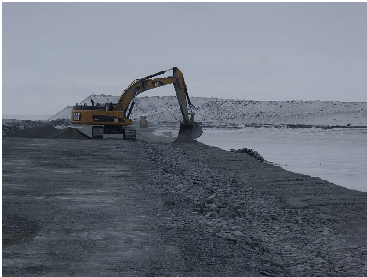
Photograph CD-1842: From Sta. 0+380/-16 m, looking S. Placement of a third 0.5 m thick lift of fine filter from El. 143.5 m to 144 m upstream of the coarse filter with an excavator from Sta. 0+335 m to 0+940 m.
