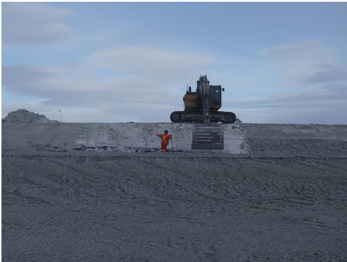
Photograph SD3-298: From Sta. 20+680/-88 m, looking S. Removal of snow on the upstream slope of SD3 above El. 142 m, from Sta. 20+620 m to 20+780 m.
