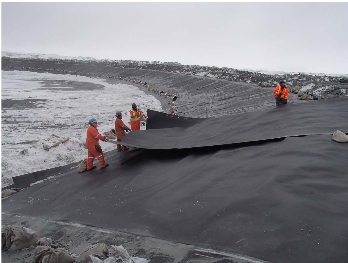
Photograph CD-1861: From Sta. 40+680/-28 m, looking NE. Installation of the LLDPE liner on the upstream slope 3H:1V (SD5 side) to 2H:1V (Central Dike side) between El. 143 m and 145 m from Sta. 40+680 m to 0+950 m (panel numbers 802 to 817).
