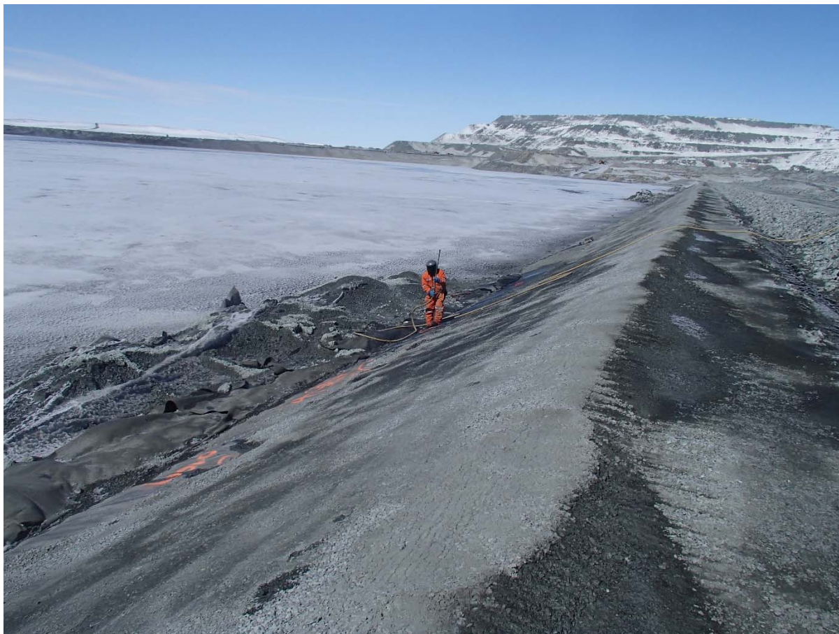
Photograph CD-1586: From Sta. 0+670/-24 m, looking N. Clean-up of the fine filter placed against the slope at the deposition finger at approx. Sta. 0+670 m with pressurized air stream to expose 1 m of LLDPE liner, in preparation for the new liner installation.
