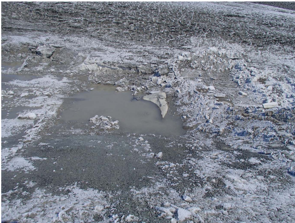
Photograph SD3-302: From Sta. 20+595/42 m, looking NE. View of water ponding on the first compacted sieved till layer of upstream toe liner tie-in. A portion of exposed damaged LLDPE liner is visible.
