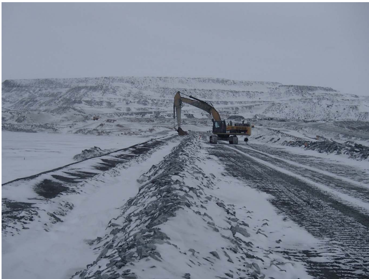
Photograph CD-1857: From Sta. 0+700/-20 m, looking N. Snow removal in the anchoring trench with an excavator between Sta. 0+170 m and 40+780 m.
