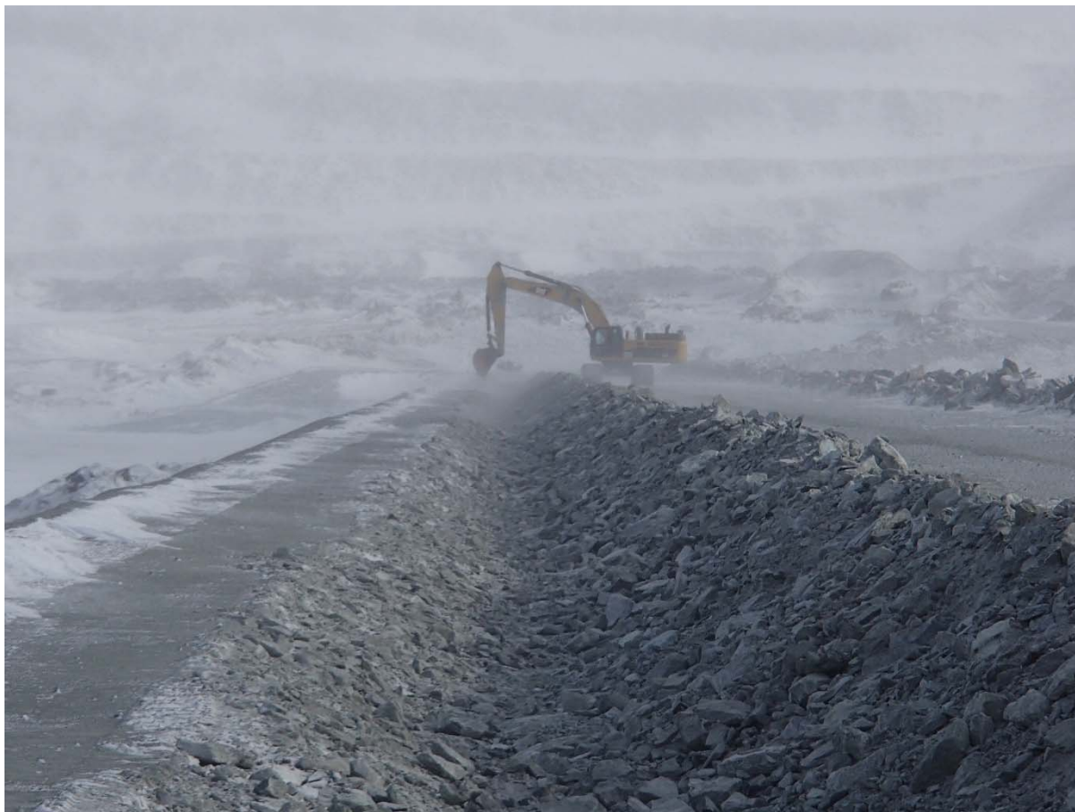
Photograph CD-1852: From Sta. 0+500/-25 m, looking N. Excavation of the LLDPE geomembrane crest anchoring trench from Sta. 0+830 m to 0+170 m.
