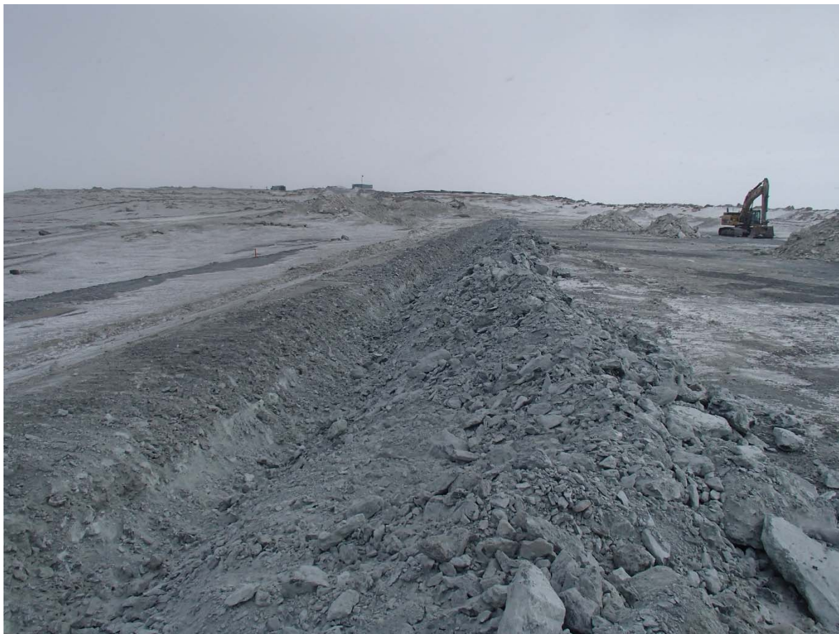
Photograph SD3-301: From Sta. 20+660/-22 m, looking SE. Excavation of the LLDPE geomembrane crest anchoring trench with an excavator from Sta. 20+655 m to 20+675 m.
