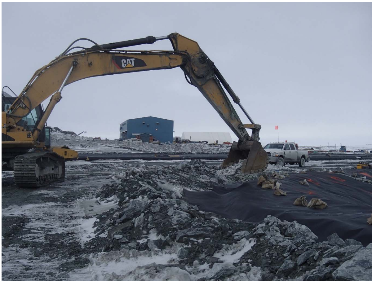
Photograph CD-1863: From Sta. 40+750/-18 m, looking SW. Backfilling of the geosynthetics tie-in from Sta. 40+680 m to 0+950 m.
