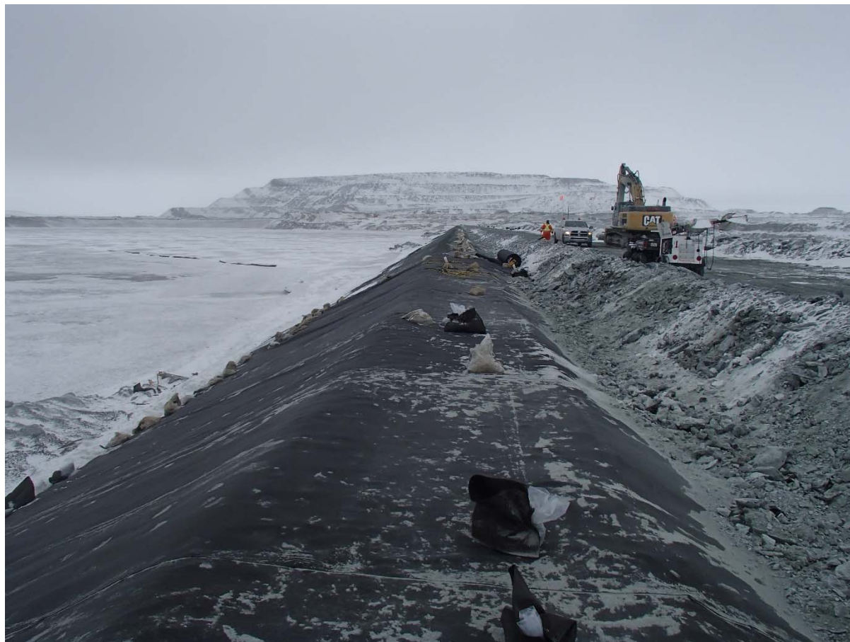
Photograph CD-1860: From Sta. 0+790/-26 m, looking N. Installation of the geotextile on the upstream slope 2H:1V between El. 143 m and 145 m from Sta. 0+830 m to 0+750 m.
