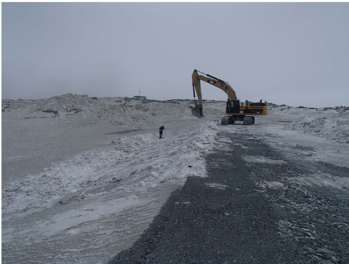
Photograph SD3-297: From Sta. 20+730/-10 m, looking SE. Removal of snow on the upstream slope of SD3 with an excavator, from Sta. 20+640 to 20+760 m.
