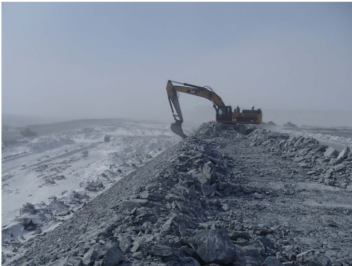
Photograph CD-1853: From Sta. 0+850/+3 m, looking S. Profiling of the downstream slope (1.5H:1V) from El. 143 to 145 m with an excavator between Sta. 0+835 m and 0+940 m.
