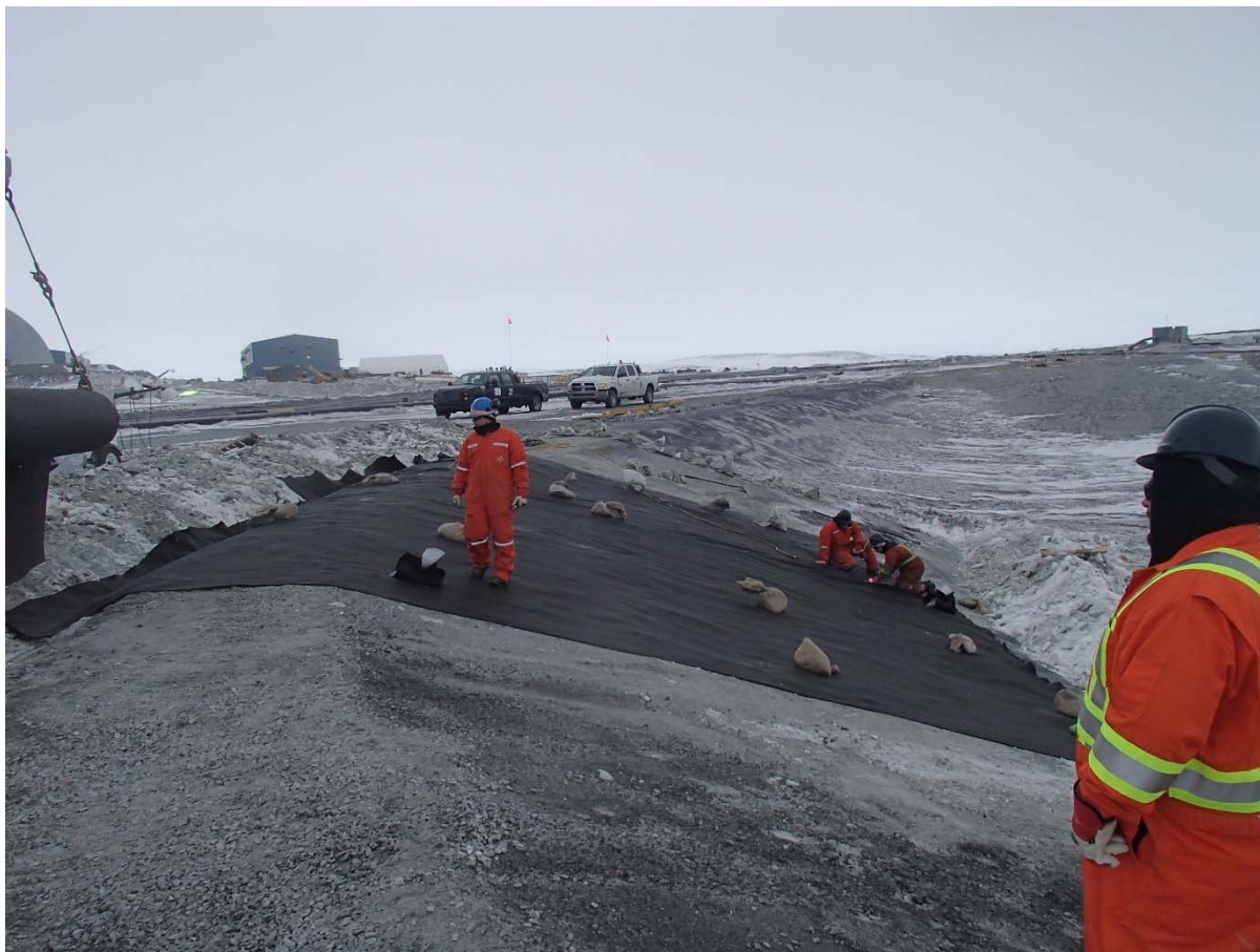
Photograph CD-1859: From Sta. 40+780/-38 m, looking SW. Installation of the geotextile on the upstream slope 3H:1V (SD5 side) to 2H:1V (Central Dike side) between El. 143 m and 145 m from Sta. 40+640 m to 0+830 m.
