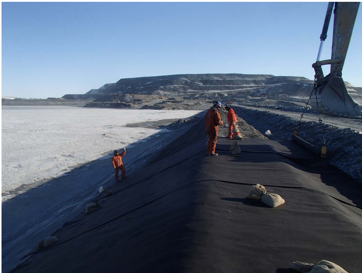
Photograph CD-1885: From Sta. 0+460/-26 m, looking N. Installation of the geotextile on the upstream slope 2H:1V between El. 143 m and 145 m from Sta. 0+480 m to 0+320 m.
