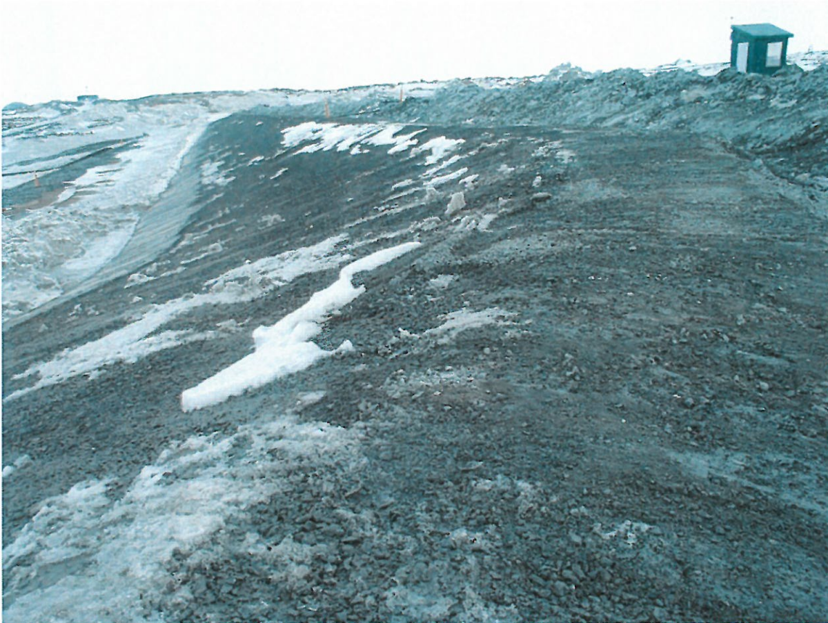
Photograph SD3-304: From Sta. 20+620/-36 m, looking SE. Smoothing of the surface of the fine filter with an excavator on top of the upstream slope from Sta. 20+600 m to 20+780 m.
