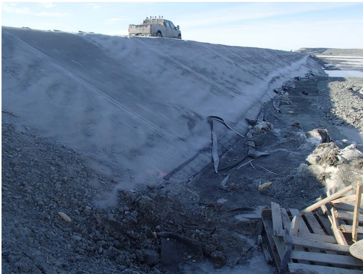
Photograph CD-1892: From Sta. 0+155/-32 m, looking S. View of the liner panel 933 overlapping the underlying liner that has been cut at around Sta. 0+160 m to drain the water.
