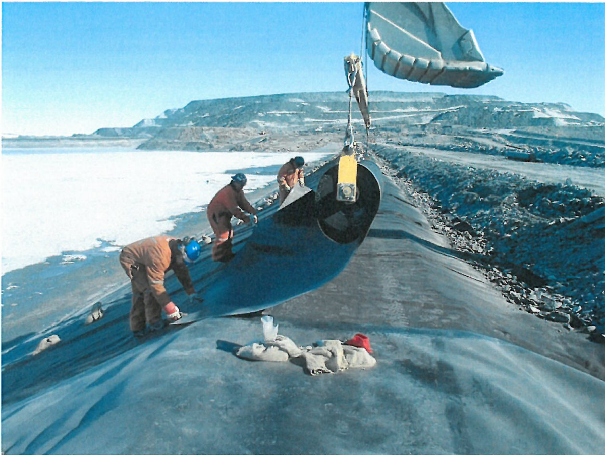
Photograph CD-1886: From Sta. 0+525/-26 m, looking N. Installation of the LLDPE liner on the upstream slope 2H:1V between El. 143 m and 145 m from Sta. 0+480 m to 0+320 m (panel numbers 887 to 910).
