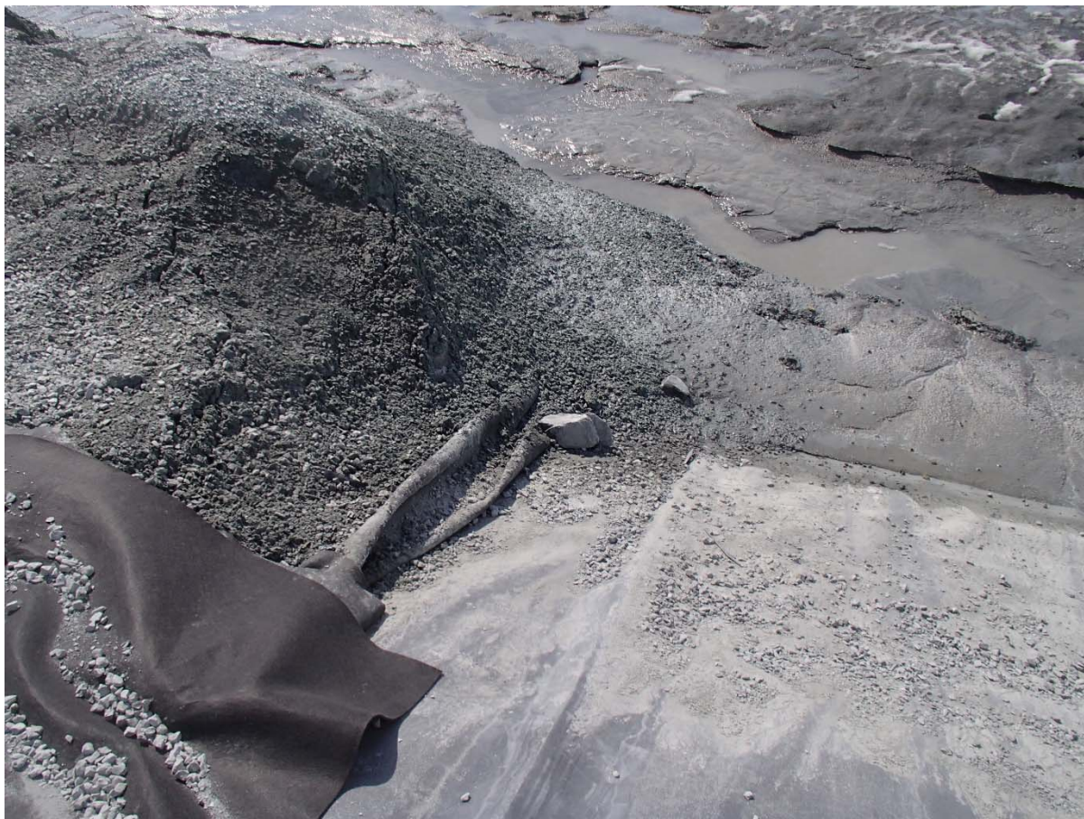
Photograph CD-1894: From Sta. 0+800/-28 m, looking E. View of a rock in direct contact with the LLDPE liner following the construction of the deposition fingers on Central Dike.
