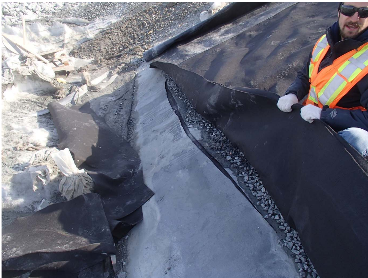
Photograph CD-1889: From Sta. 0+150/-28 m, looking N. View of the underlying liner that has been cut at around Sta. 0+160 m to drain the water.
