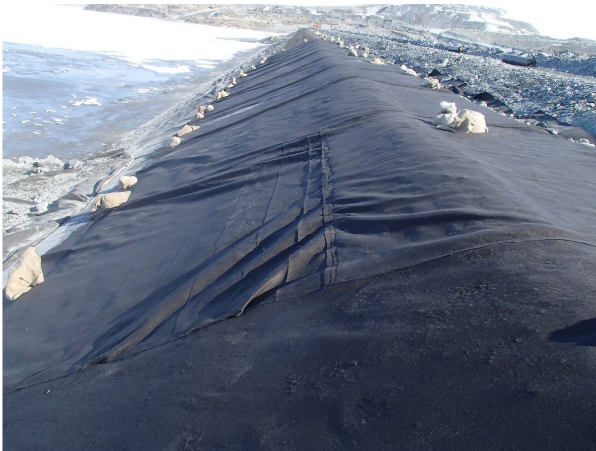
Photograph CD-1881: From Sta. 0+530/-27 m, looking N. View of a geotextile panel with a horizontal weld in the slope at Sta. 0+520 m before its removal.
