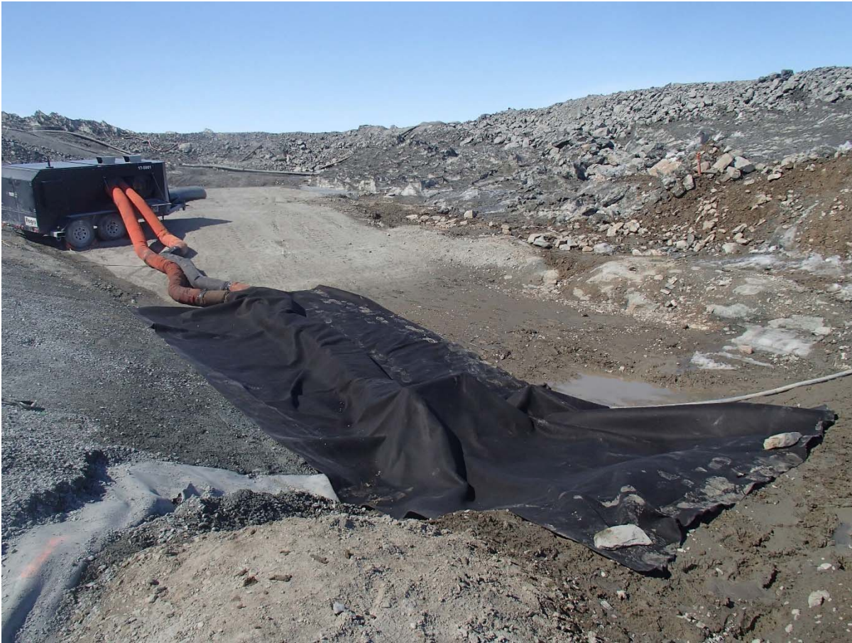
Photograph SD3-305: From Sta. 20+610/-48 m, looking NW. Dewatering of the water ponding on the first compacted sieved till layer of upstream toe liner tie-in. A Genset Frost-fighter is heating the sieved till layer and a pump is evacuating the water.
