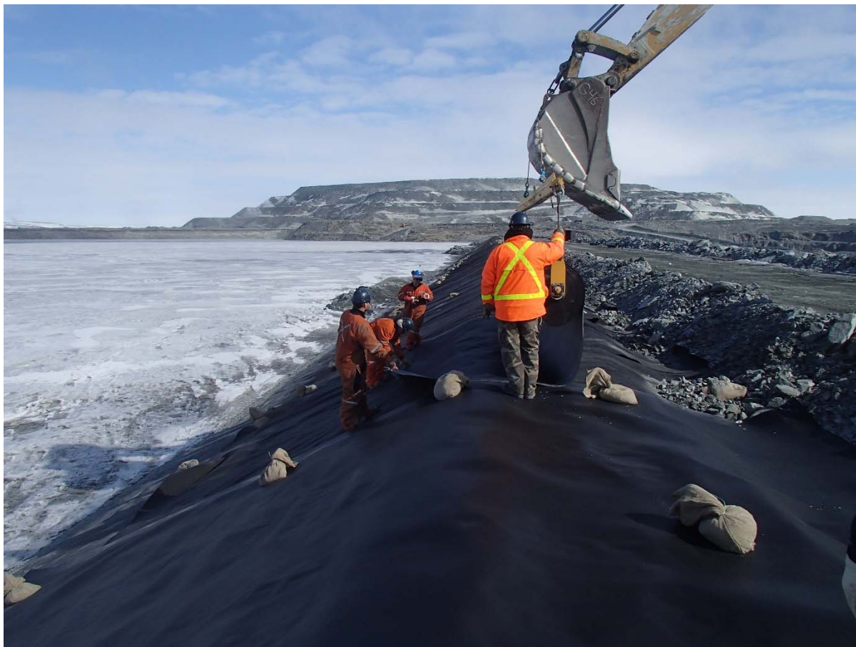
Photograph CD-1878: From Sta. 0+720/-24 m, looking N. Installation of the LLDPE liner on the upstream slope 2H:1V between El. 143 m and 145 m from Sta. 0+740 m to 0+610 m (panel numbers 849 to 867).
