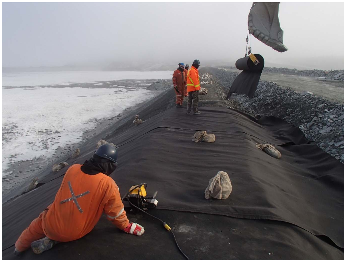
Photograph CD-1880: From Sta. 0+600/-25 m, looking N. Installation of the geotextile on the upstream slope 2H:1V between El. 143 m and 145 m from Sta. 0+610 m to 0+480 m.
