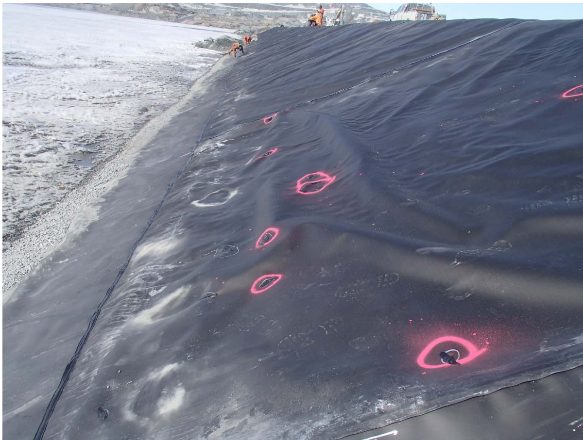
Photograph CD-1879: From Sta. 0+735/-28 m, looking N. View of the repaired holes on panel 850.
