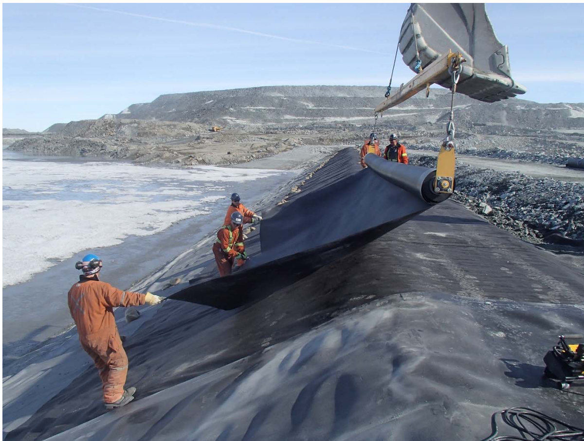
Photograph CD-1888: From Sta. 0+525/-26 m, looking N. Installation of the LLDPE liner on the upstream slope 2H:1V between El. 143 m and 145 m from Sta. 0+320 m to 0+150 m (panel numbers 911 to 933).
