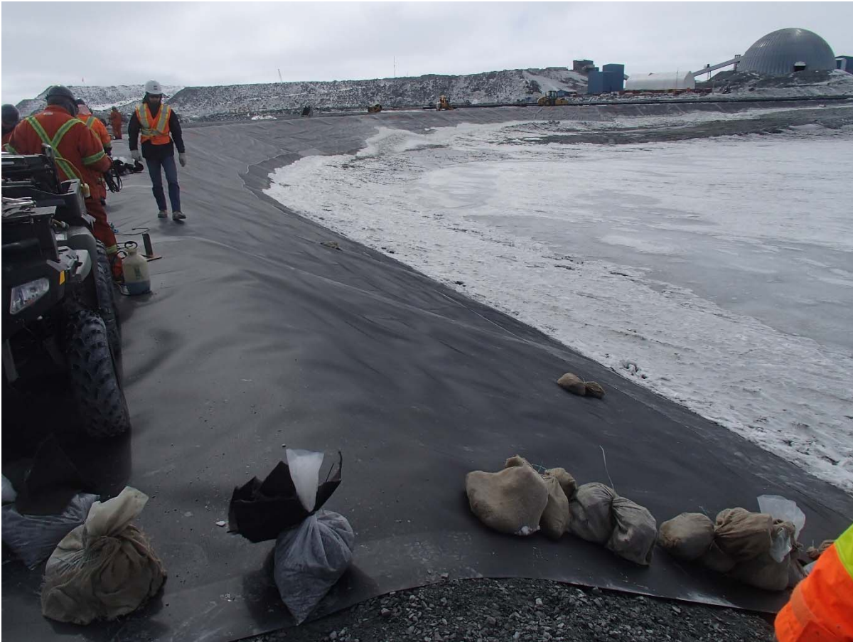
Photograph CD-1870: From Sta. 0+900/-26 m, looking S. Installation of the LLDPE liner on the upstream slope 2H:1V between El. 143 m and 145 m from Sta. 0+935 m to 0+900 m (panel numbers 820 to 823).
