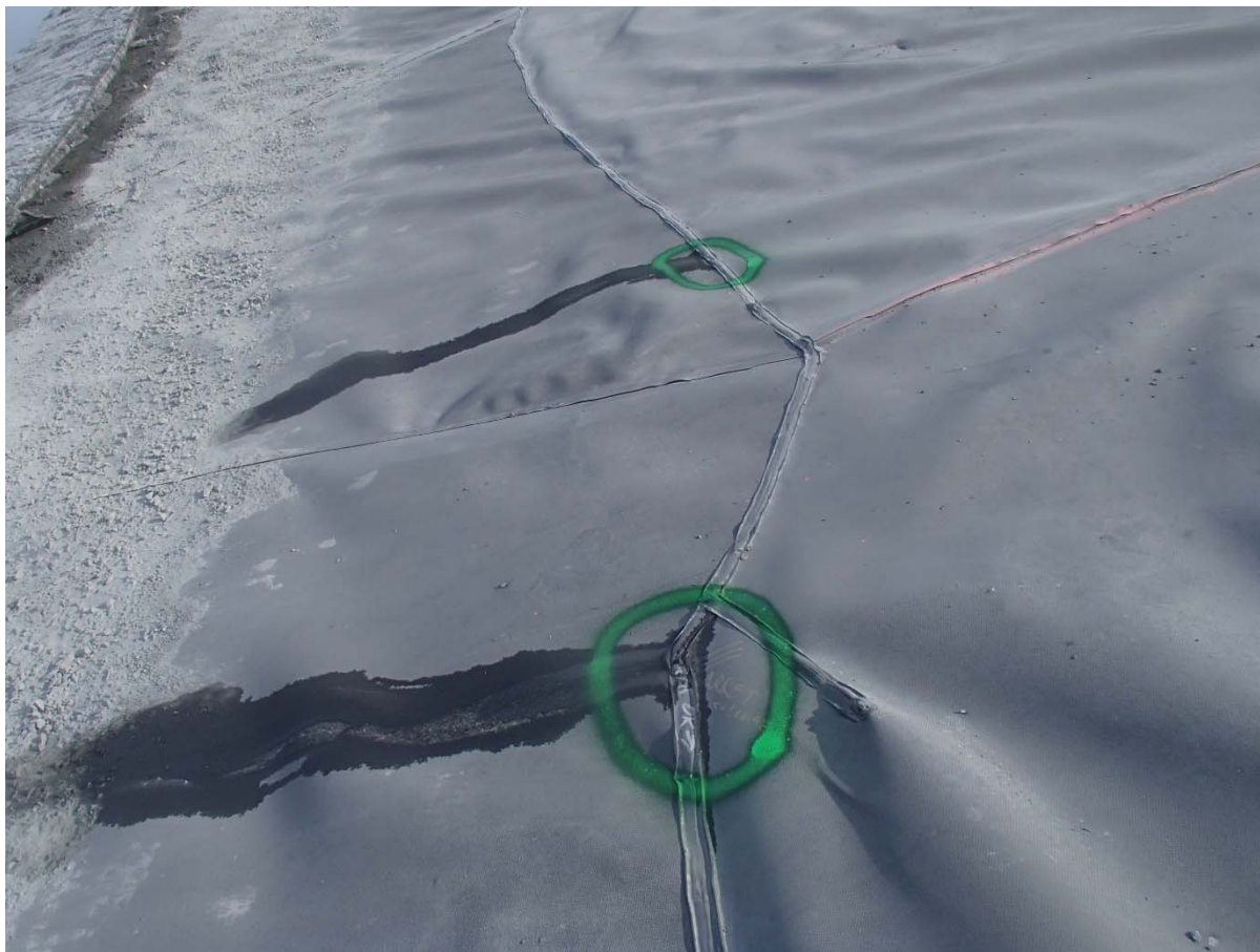
Photograph CD-1891: From Sta. 0+960/-28 m, looking N. View of leaking extrusion fillet seam before their repair on panels 816 and 818.
