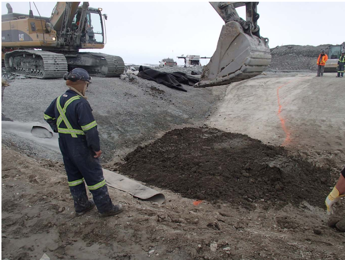
Photograph SD3-312: From Sta. 20+610/-48 m, looking W. Placement of a 0.15 m thick lift of compacted sieved till from Sta. 20+596.4 m to 20+601.6 m (offset -42.6 to -46.3 m) to fill the depression in the compacted sieved till layer.
