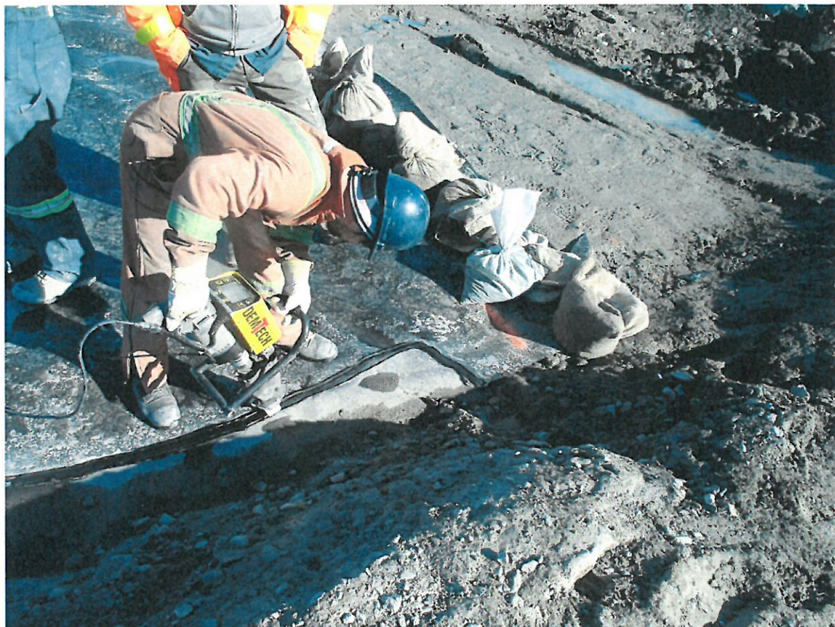
Photograph SD3-316: From Sta. 20+610/-45 m, looking NW. Repairs on the extrusion fillet seam between LLDPE panel 965 and the existing LLDPE panel at Sta. 20+600 m (approx.).
