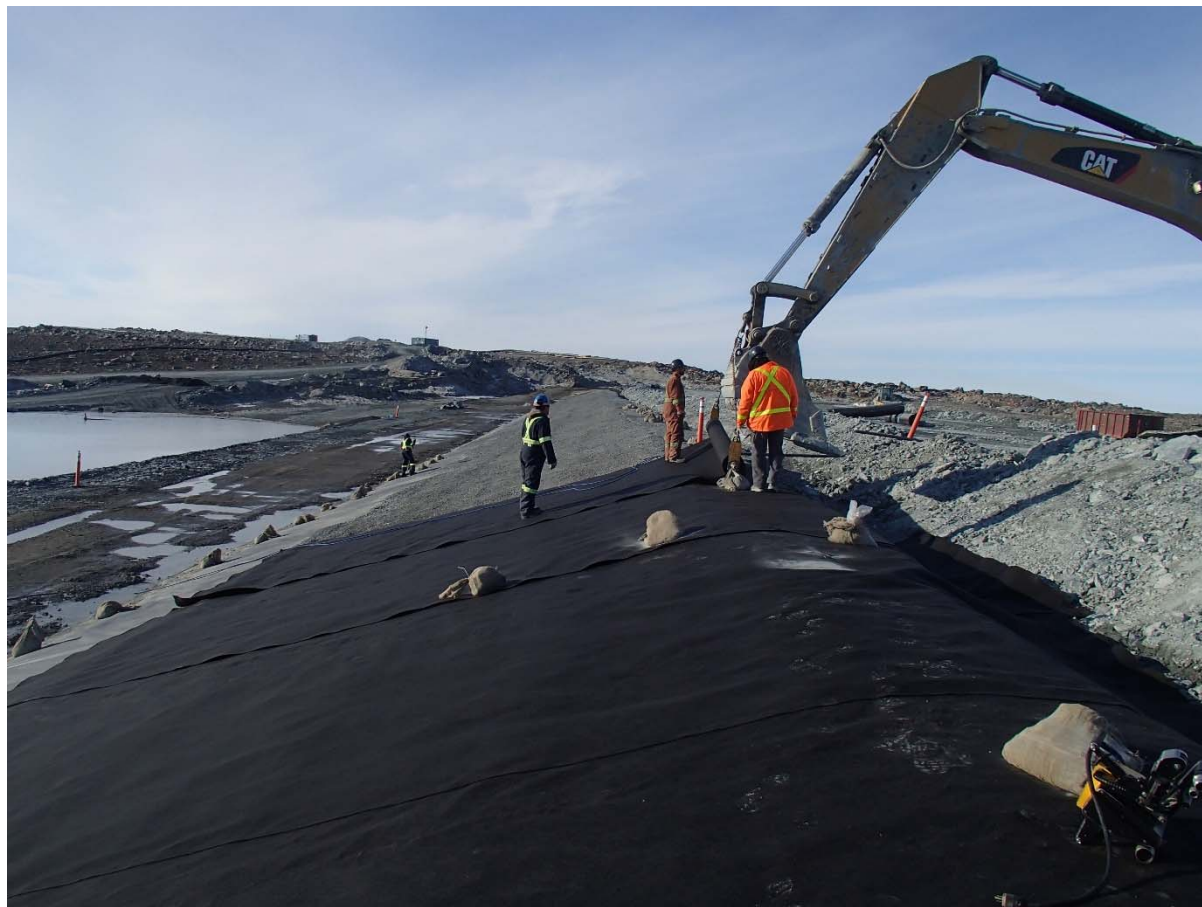
Photograph SD3-310: From Sta. 20+635/-24 m, looking S. Installation of the geotextile on the upstream slope 3H:1V between El. 143 m and 145 m from Sta. 20+630 m to 20+800 m.
