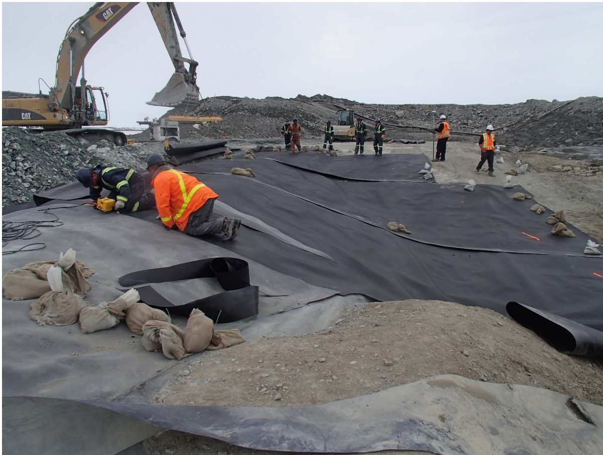
Photograph SD3-315: From Sta. 20+615/-46 m, looking W. Installation of the geotextile on the upstream slope 3H:1V between El. 143 m and 145 m from Sta. 20+593 m to 20+610 m and installation of the LLDPE liner on the upstream slope 3H:1V between El. 143 m and 145 m from Sta. 20+593 m to 20+610 m (panel numbers 965 to 967).
