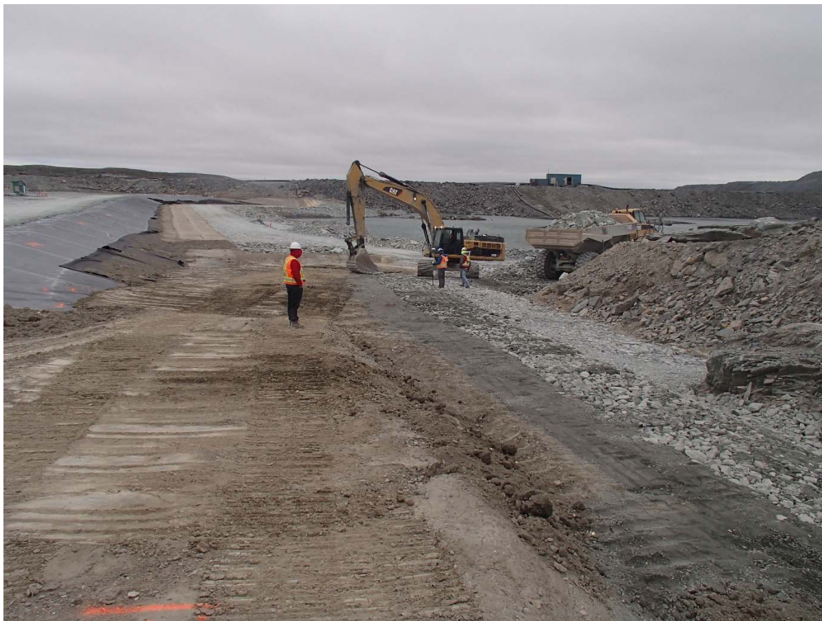
Photograph SD3-333: From Sta. 20+817/-29 m, looking N. Placement of a second 0.5 m thick lift of fine rockfill on the upstream slope of the upstream toe liner tie-in with an excavator from Sta. 20+775 m to 20+800 m.
