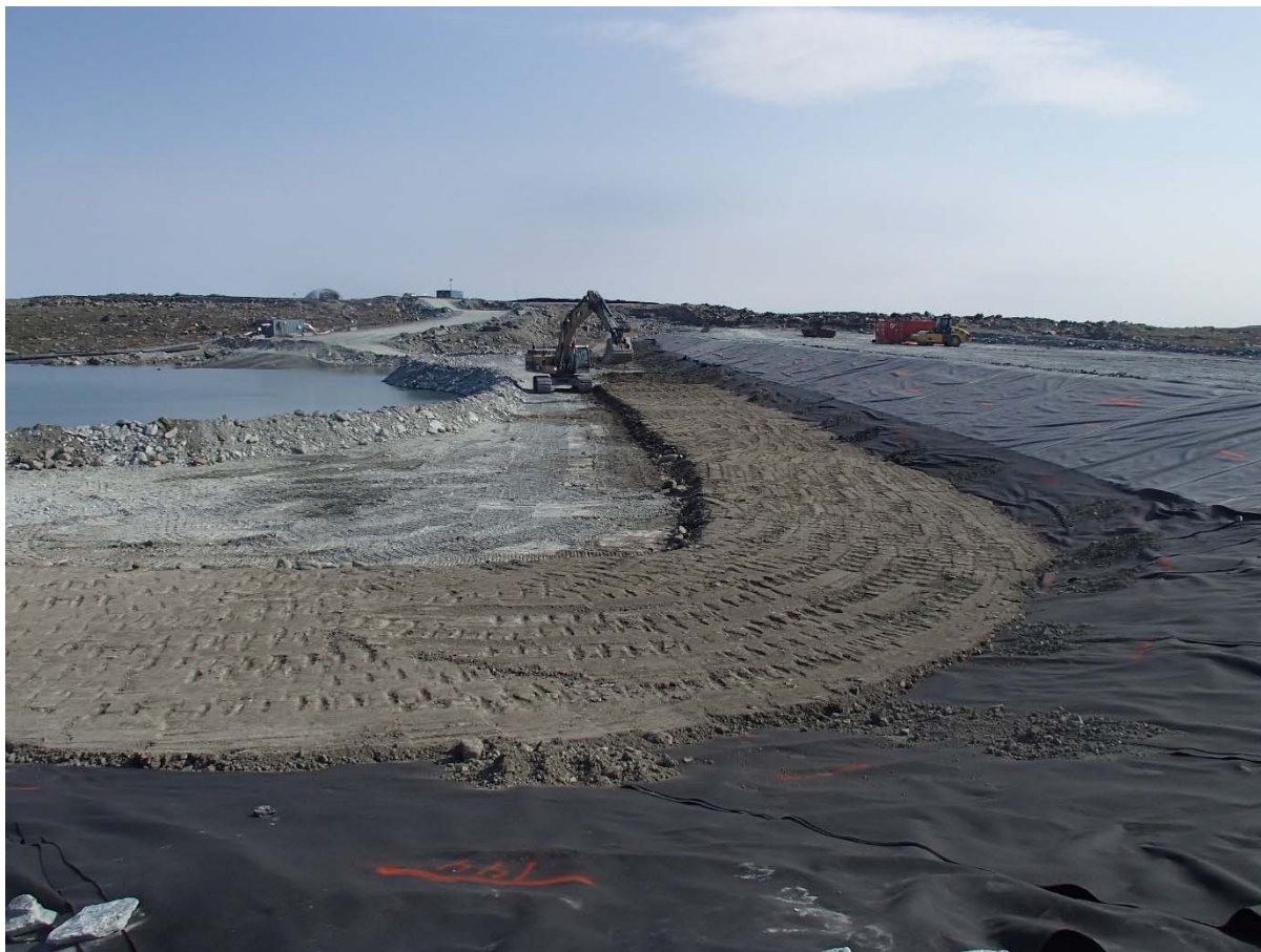
Photograph SD3-323: From Sta. 20+610/-43 m, looking S. Placement of the first lift of low quality till (0-150 mm) from El. 142 m to 142.5 m from Sta. 20+610 m to 20+715 m.
