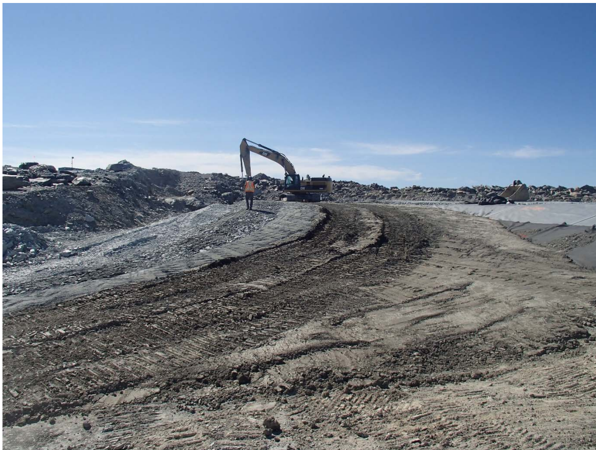
Photograph SD3-336: From Sta. 20+755/-48 m, looking S. Placement of a fourth 0.5 m thick lifts of fine filter, coarse filter and fine rockfill on the upstream slope of the upstream toe liner tie-in with an excavator from Sta. 20+770 to 20+800 m.
