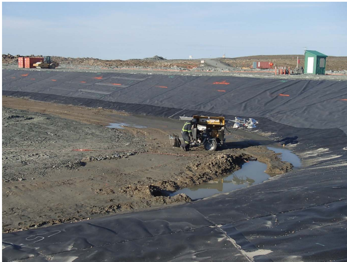
Photograph SD3-321: From Sta. 20+610/-56 m, looking SW. Water ponding at El. 142m on the compacted sieved till layer of the upstream toe liner tie-in at approx. Sta. 20+620 m to 20+630 m was pumped.
