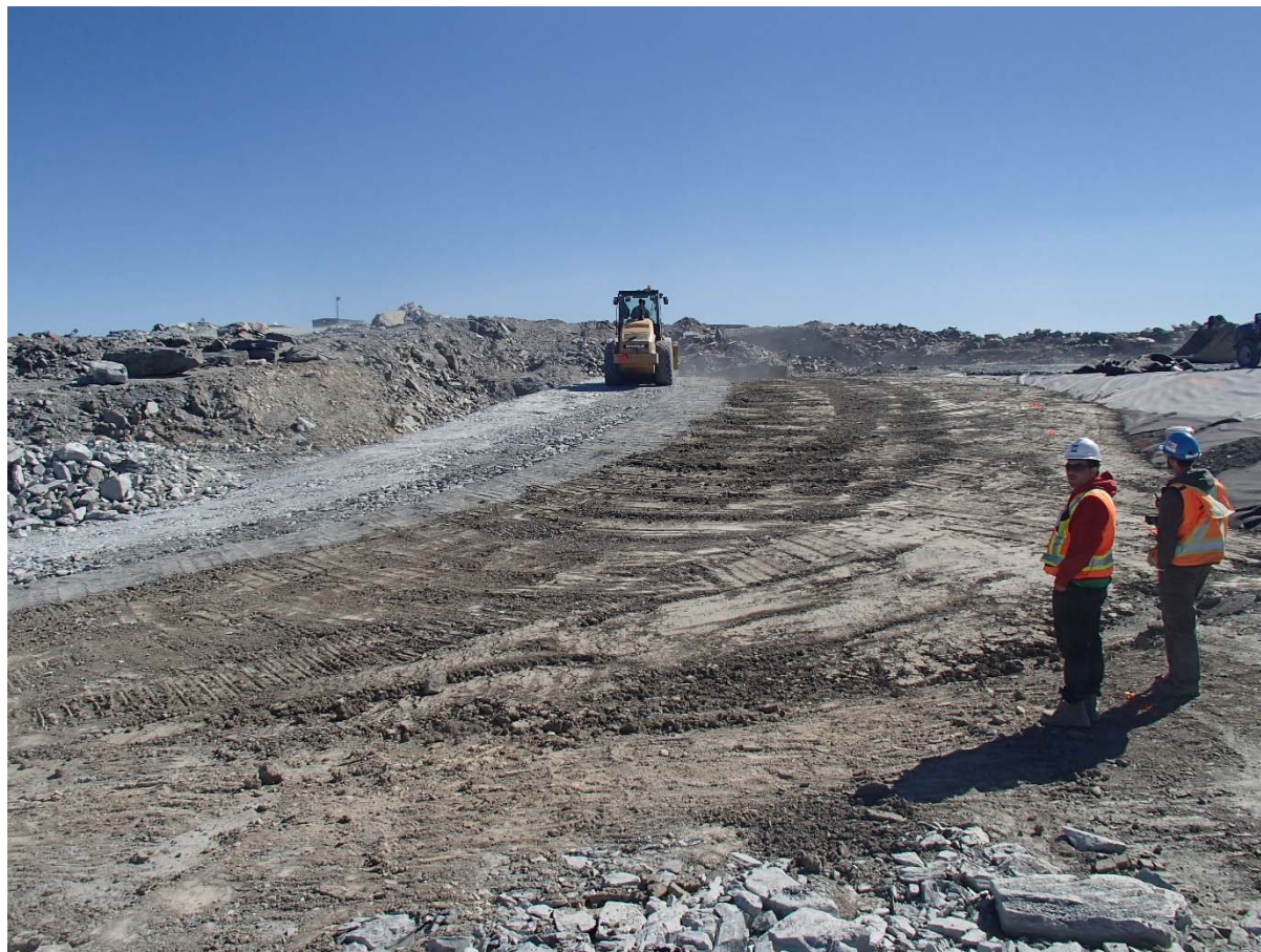
Photograph SD3-337: From Sta. 20+760/-37 m, looking S. Compaction of the fourth 0.5 m thick lifts of fine filter, coarse filter and fine rockfill on the upstream slope of the upstream toe liner tie-in with a 10-tonne smooth-drum compactor with vibrations (4 passes) from Sta. 20+770 to 20+800 m.
