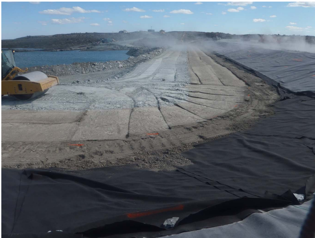
Photograph SD3-331: From Sta. 20+610/-43 m, looking S. Compaction of the 0.5 m lift of low quality till (0-150 mm) at El. 143 m with a 10-tonne smooth-drum compactor with vibration (4 passes) from Sta. 20+610 m to 20+760 m.
