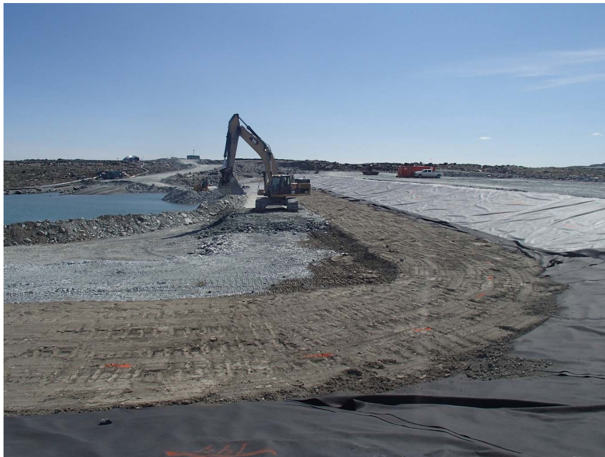
Photograph SD3-330: From Sta. 20+610/-43 m, looking S. Placement of a second 0.5 m thick lift of fine rockfill (0-500 mm) upstream of the low quality till (0-150 mm) from El. 142.5 m to 143 m from Sta. 20+610 m to 20+760 m.
