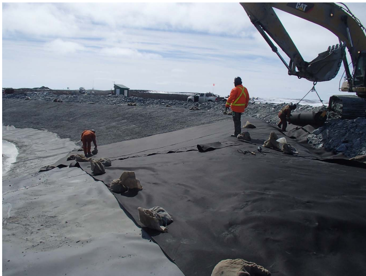
Photograph SD3-308: From Sta. 20+620/-48 m, looking SW. Installation of the geotextile on the upstream slope 3H:1V between El. 143 m and 145 m from Sta. 20+610 m to 20+810 m.
